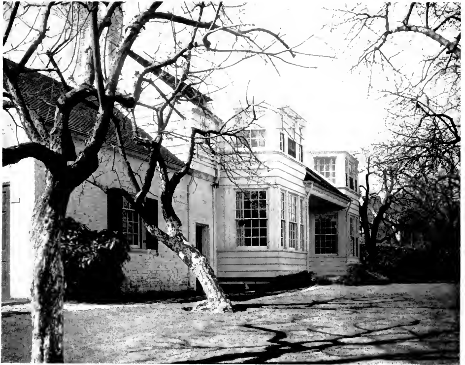
NEU RESIDENCE, PORTLAND, OREGON—1930 TERRACE SIDE
