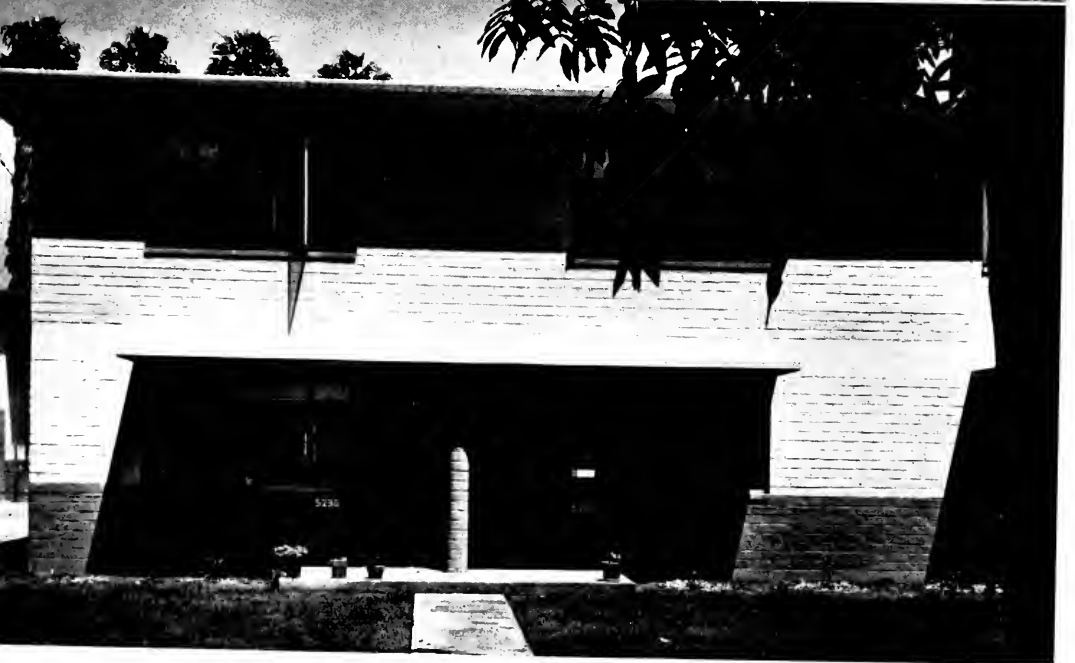
Close up of a twin apartment unit showing wide overhang flat roof and hooded entrances, the latter formed by a cantilevered extension of the second floor slab
