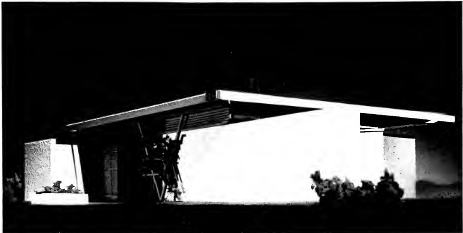
THE "V" HOUSE, WITH ITS GRACIOUS ENTRANCE AND PRIVATE PATIO. ITS MASSIVE WALLS ARE GROUPED FOR PRIVACY AND RELATIVE PROTECTION AGAINST BOMB FRAGMENTS AND FIRE
