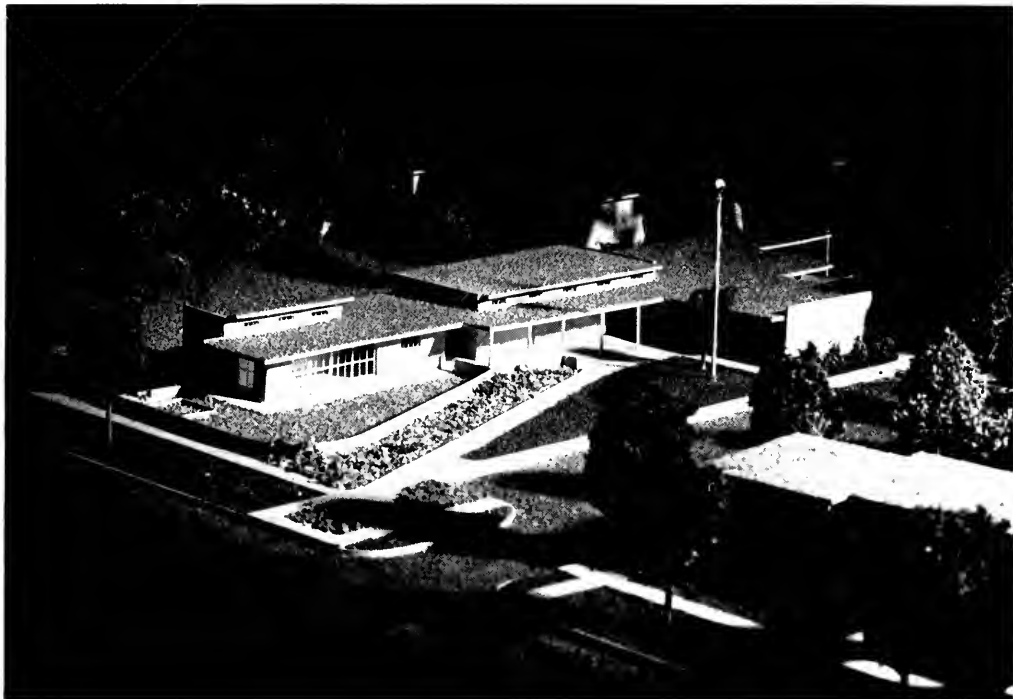
Administration building, a one-story structure with masonry walls. Building may also be used for community gatherings.
