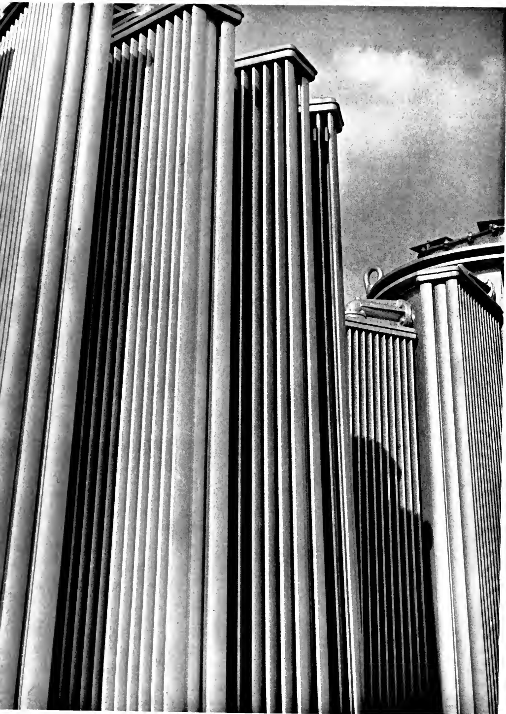
PHOTOGRAPH OF TRANSFORMERS AT EDISON SALVAGE YARDS, ALHAMBRA, CALIFORNIA, BY W. ELLIS TEAS
