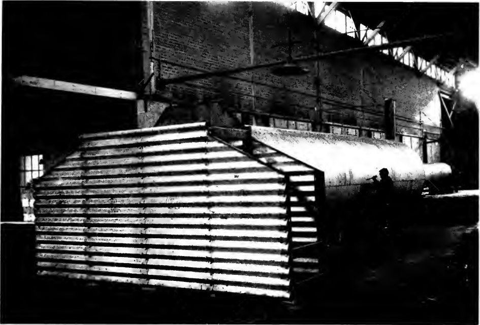
This Armo iron air-raid shelter is 50 ft. long and 7 1/2 ft. high and will accommodate 50 persons. Four unskilled workmen can erect the shelter with simple tools in a few hours.
