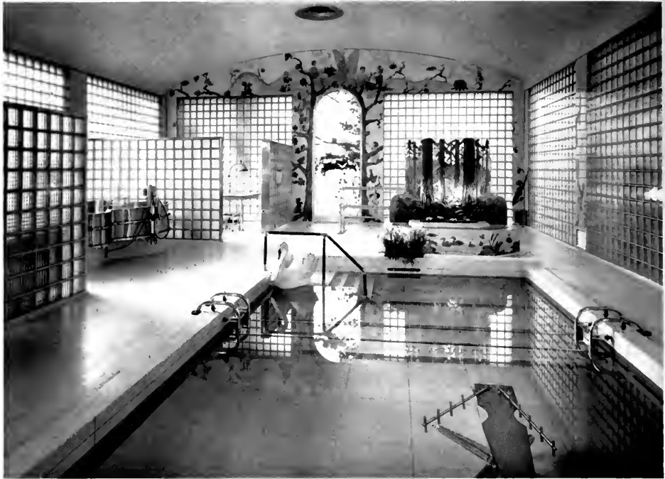
GLASS BLOCKS FOR WALL CONSTRUCTION WERE CHOSEN LARGELY BECAUSE ONLY DAYLIGHT WILL PENETRATE THEM AND THE PATIENTS ARE PROTECTED FROM DUST, DIRT AND MOISTURE
