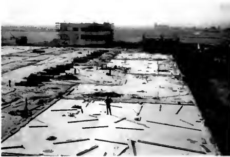
SISAL paper used to cure and protect concrete floor at United Airlines Terminal
