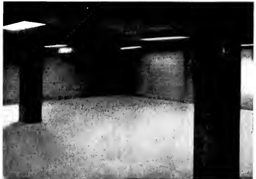
Government Cellar contains four 100-barrel and eleven 250-barrel glass lined tanks. The Wall Units are Kraftile Ceramic Glazed. Cellular, they are ideal for a refrigerated room like this. Kraftile Vitreous 8 x 8 Quarry Tile is used to finish the floor here, in the Meter Room, and the entire working area of Machinery Hall. 13,300 square feet were used—the largest quarry tile installation in San Francisco last year.
