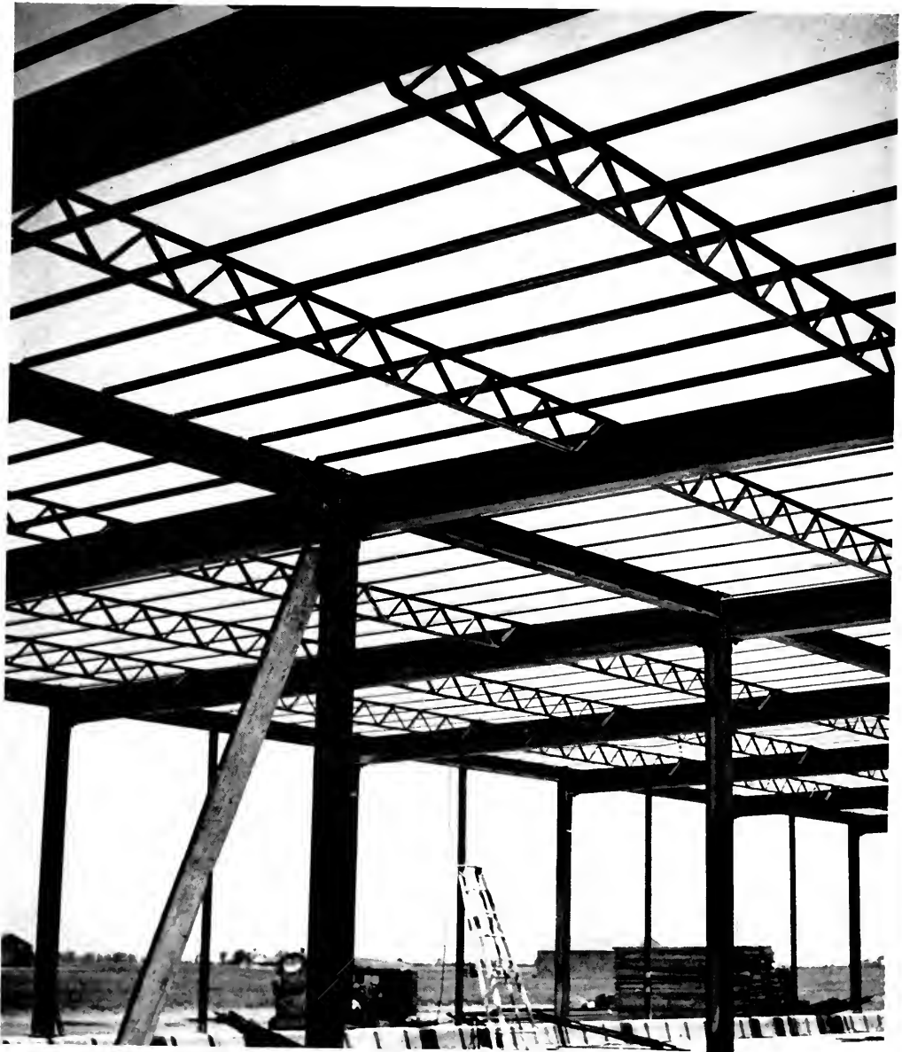
STEEL FRAME AND JOIST SYSTEM USED IN CONSTRUCTION OF INDUSTRIAL PLANT
