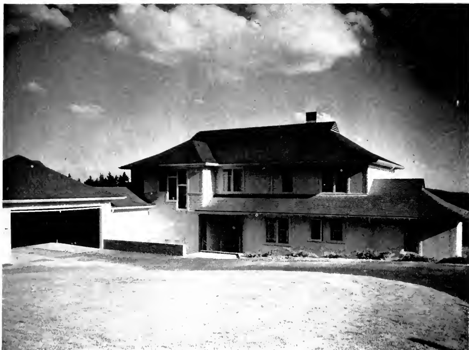
SCHLESSER RESIDENCE—1940—ENTRANCE FRONT
