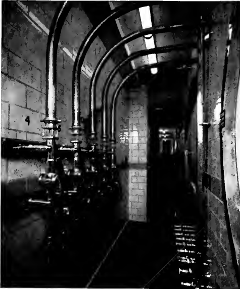
Government Cellar contains four 100-barrel and eleven 250-barrel glass lined tanks. The Wall Units are Kraftile Ceramic Glazed. Cellular, they are ideal for a refrigerated room like this. Kraftile Vitreous 8 x 8 Quarry Tile is used to finish the floor here, in the Meter Room, and the entire working area of Machinery Hall. 13,300 square feet were used—the largest quarry tile installation in San Francisco last year.
