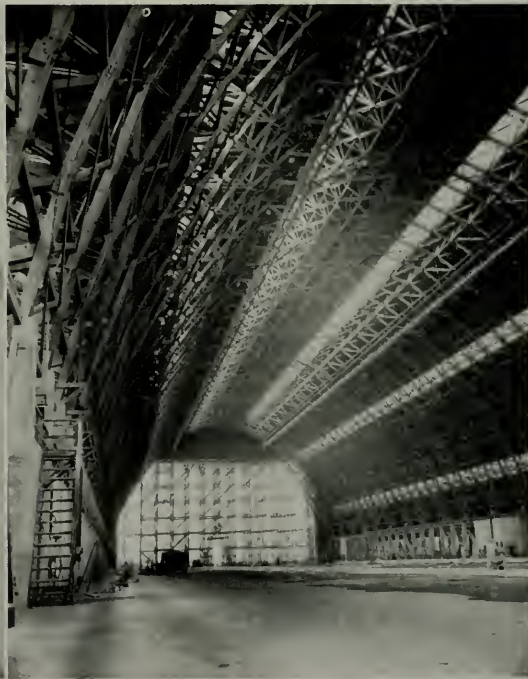
Left, folding doors at each end of hangar are supported by twin concrete pylons carrying an enormous built-up wooden "box beam." The doors fold up in recess between pylons.
