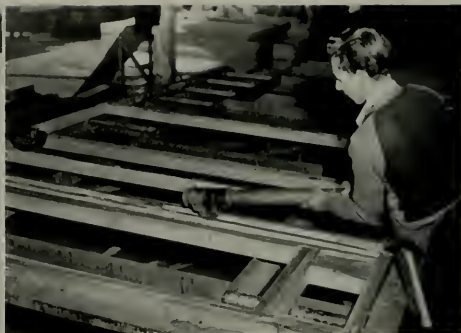
Modern methods of home construction are the result of planning by architects to facilitate erection and to make a better-built and more livable home for post-war living. Here the wall sections in a flat-bed jig are receiving glue applied by workman from a glue gun. Construction with glue not only makes stronger walls, but saves tons of nails which would ordinarily be used.
