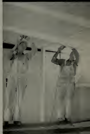
Fastening Roof Panel With Electric Screwdrivers
