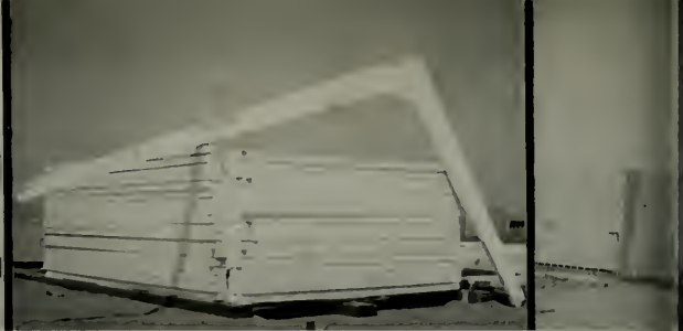
Laminated Three-Hinged Arches Before Erection
