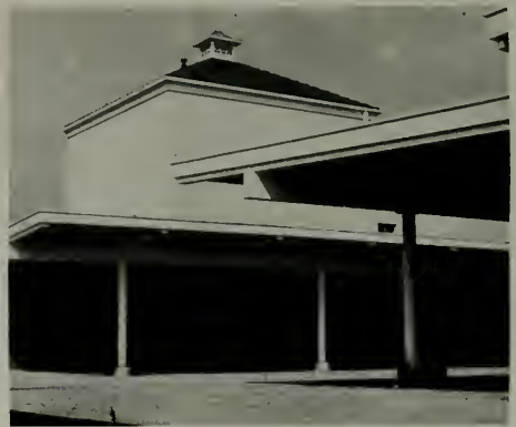
Typical private garage for tenants of Parklabrea Apartments, Los Angeles
