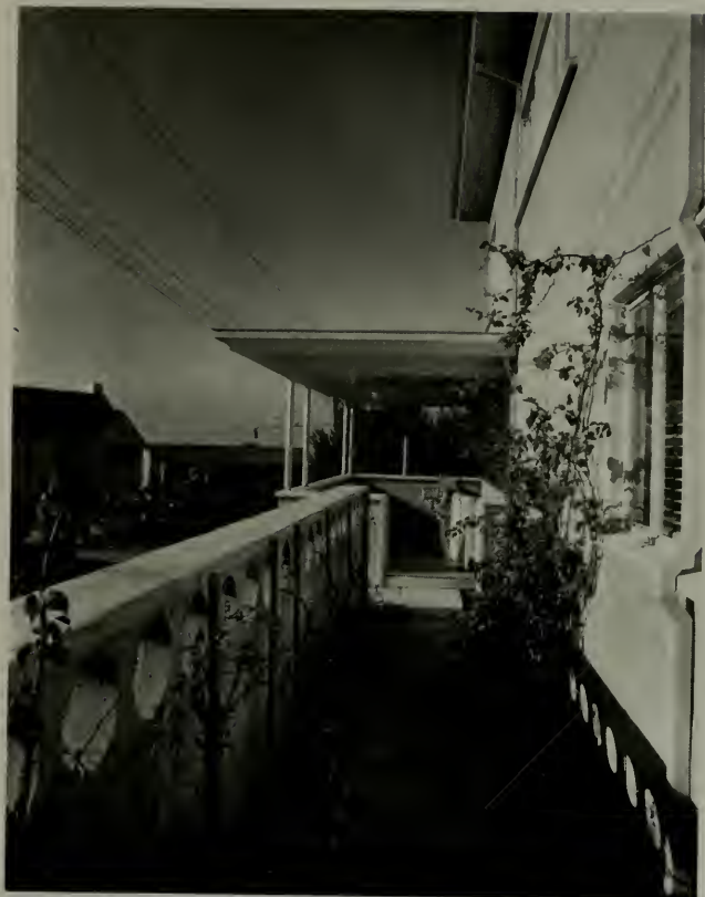
Left: Service walk, showing Concrete Grid Walls.
