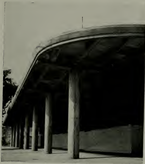
DETAIL OF ARCADE, LOCKHEED COMMISSARY BURBANK, CALIFORNIA
