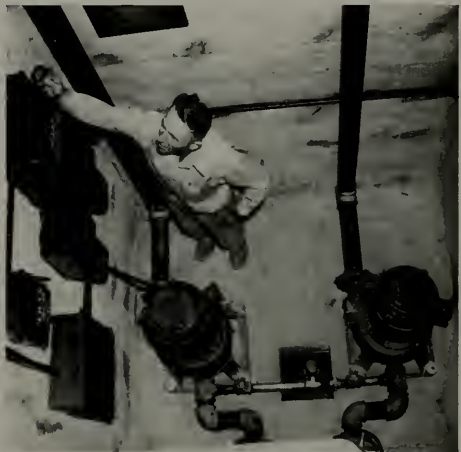
Sump Pit showing pump equipment
