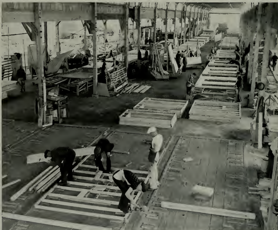
This is more evidence of planning on the technological front, to expedite delivery of houses to the consumer, as well as keep down costs of post-war homes. The model prefabrication plant shown here is so arranged that entire houses may be prefabricated at one time. In the foreground wall frames are being nailed together in the first step after the proper lengths have been cut. Wall is then glued to studding, progresses to delivery end of the plant where a complete building—roof, ceiling, wall and floor sections are loaded onto a single truck, transported to site to be erected.
