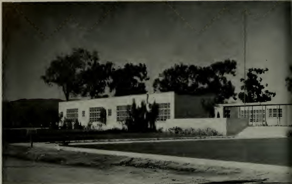
View from street. Buildings occupy an area 203 feet in depth by 419 feet in length. The set-back from street curb is approximately 80 feet.
