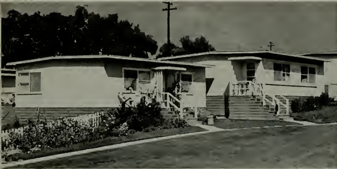
Row of houses placed to conform to contour of site, Bayview Heights, San Diego, California.
