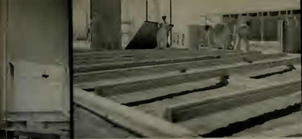
Mudsills and Floor Girders (foreground), Erecting Wall Panel (background)
