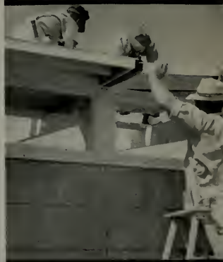
Dropping Roof Panel into Place
