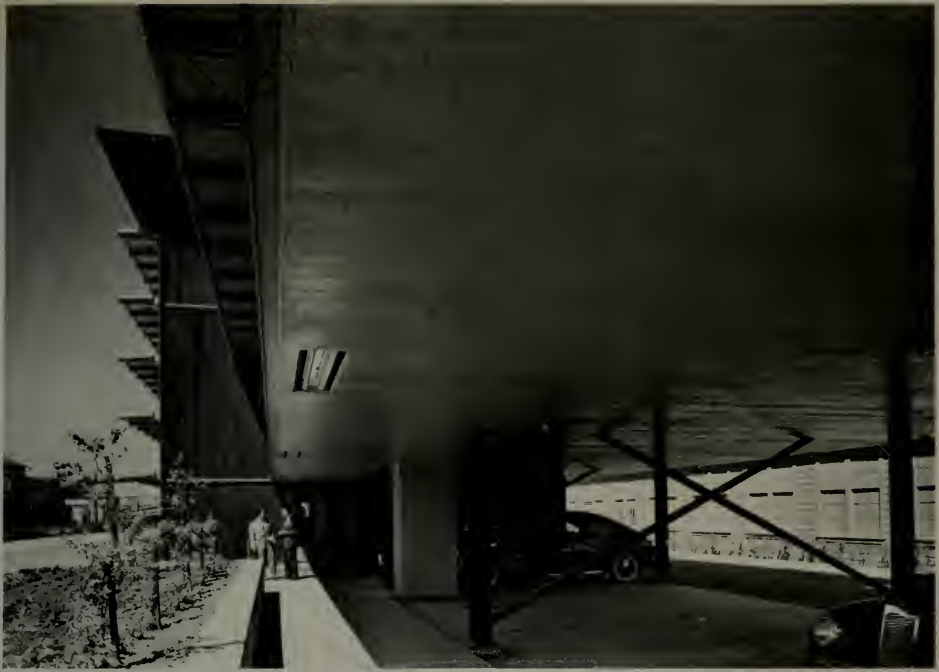
Steel columns and beams support this parking area at street level of main building. Company executives use space for parking, convenient in inclement weather.
