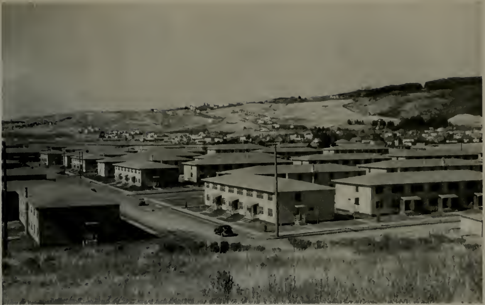
LATE PHOTO SHOWING LARGE GROUP OF THE 4,000-UNIT RICHMOND PROJECT ONLY THE PAVING REMAINS TO BE LAID
