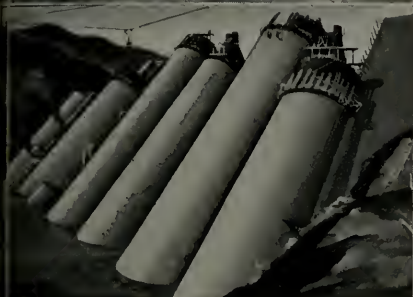
The Bartlett Dam, highest multiple arch construction in the world. Arizona.
