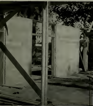
Showing wall panels in process of erection.
