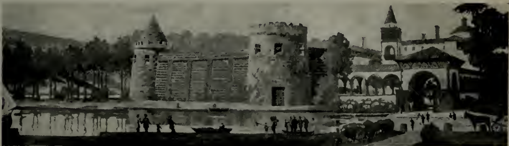
A wooden fort built at St. Augustine about 1678—taken from a Spanish sketch. Copies of a document are also extant in which the Spanish governor pleaded with the king of Spain to send him money with which to build an all-stone fort, saying that they could not fire off the cannon in the wooden fort because the fort would collapse.
