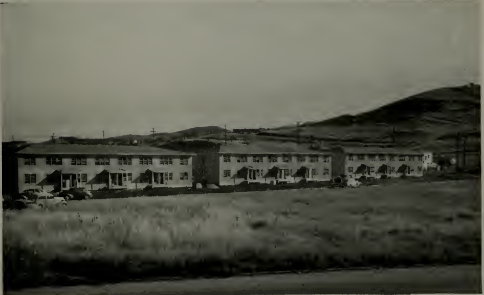
THREE OF 285 FOURTEEN-APARTMENT BUILDINGS AT RICHMOND, ALL OF WHICH WILL BE COMPLETED THIS MONTH—A 4,000-UNIT PROJECT FOR THE U. S. MARITIME COMMISSION
