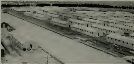
McCarthy-built barracks for housing alien evacuees at Tanforan Race Track. 170 barracks were built in 7 days against a time limit of 15 days.
