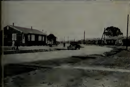
A city of 5000 homes for war workers. Erected in 180 days. Norfolk, Virginia.
