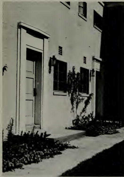
Two front entrances to apartments. Note ventilators over windows. Walks fringed with shrubbery.
