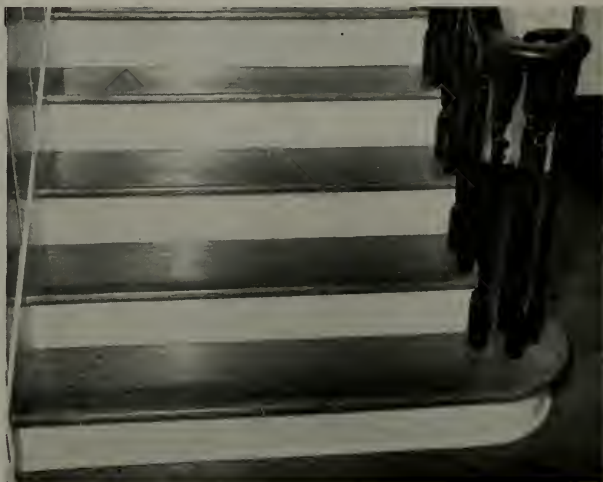
Dark stained treads and painted risers combined in a beautiful staircase of hemlock.
