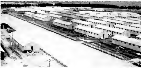
McCarthy-built barracks for housing alien evacuees at Tanforan Race Track. 170 barracks were built in 7 days against a time limit of 15 days.
