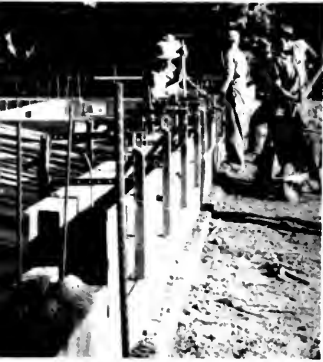
Tamping concrete into slip forms, showing lock with hard rock foundations.
