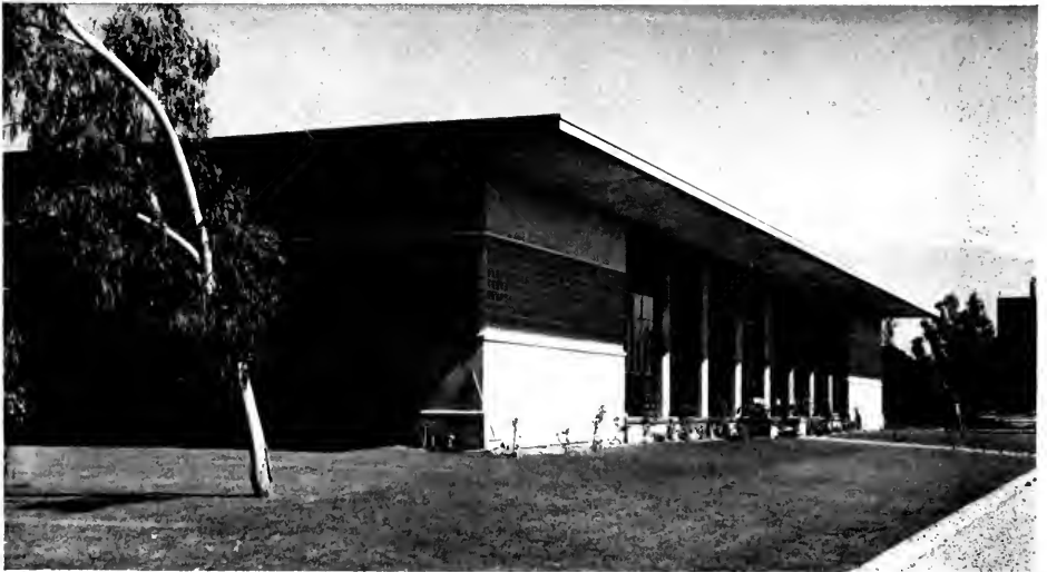
PHYSICAL TESTING LABORATORY, KAISER STEEL PLANT, FONTANA Birge M. and David B. Clark, Architects
