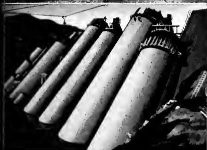
The Bartlett Dam, highest multiple arch construction in the world. Arizona.
