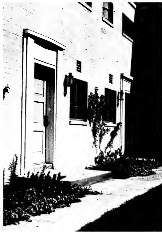
Two front entrances to apartments. Note ventilators over windows. Walks fringed with shrubbery.
