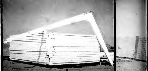
Laminated Three-Hinged Arches Before Erection
