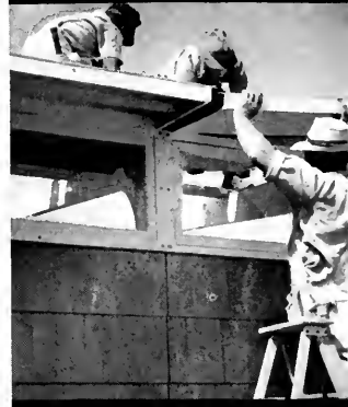
Dropping Roof Panel into Place
