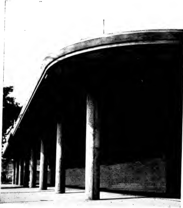
DETAIL OF ARCADE, LOCKHEED COMMISSARY BURBANK, CALIFORNIA
