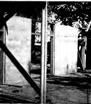
Showing wall panels in process of erection.
