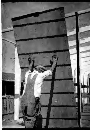
Assembling of Three-Hinged Arches
