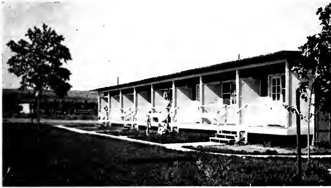
This duration city houses 6,000 persons. There are 2,000 apartments. Below, two close-ups and building site.
