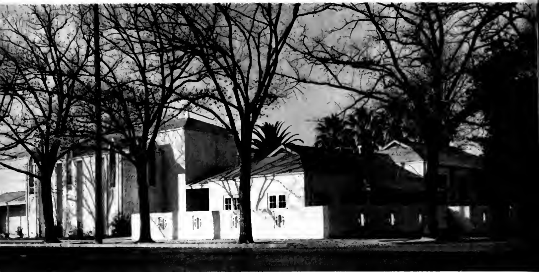
ST. JOHN'S EPISCOPAL CHURCH, MARYSVILLE, CALIFORNIA General view of group.
