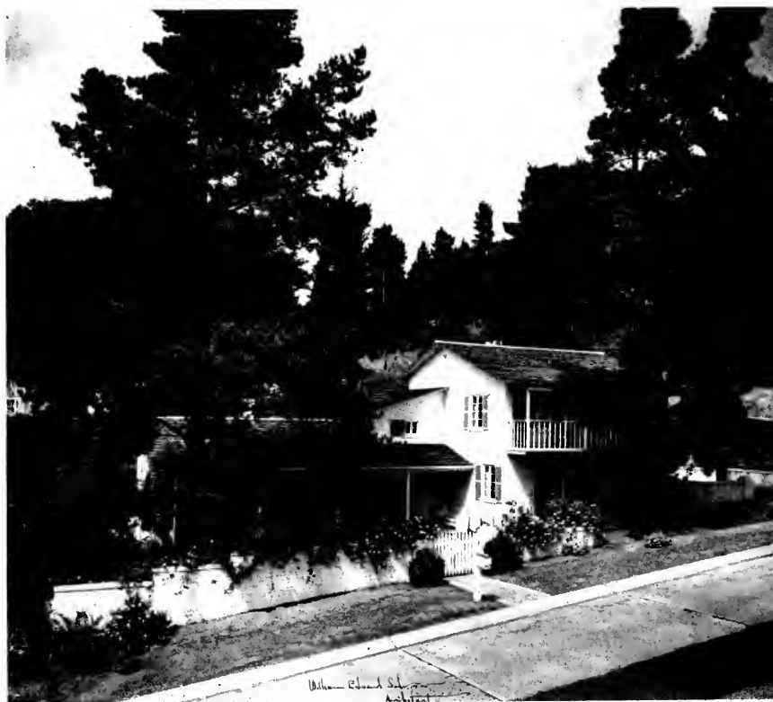
HILLSIDE HOUSE FOR MR. AND MRS. STUART HAWLEY, PIEDMONT William E. Schirmer, Architect
