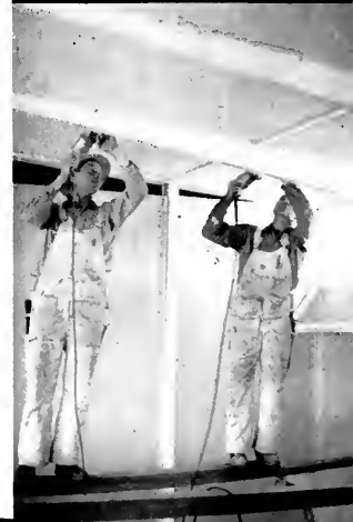
Fastening Roof Panel With Electric Screwdrivers
