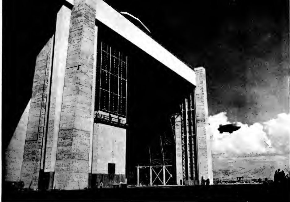
BLIMP HANGAR UNDER CONSTRUCTION FOR U. S. NAVY
