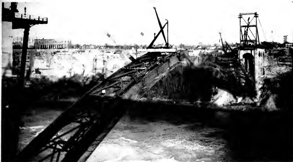
ERECTION SHOWN PROCEEDING FROM BOTH SIDES OF RIVER. INITIAL TIE BACKS HAVE BEEN REMOVED AND ADVANCED FURTHER OUT ON THE SPAN AS ERECTION PROCEEDED
