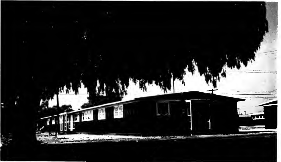
TEMPORARY DORMITORY, WILMINGTON HALL Planned as a community center this development provides cafeteria, recreation, club rooms, library and health services.
