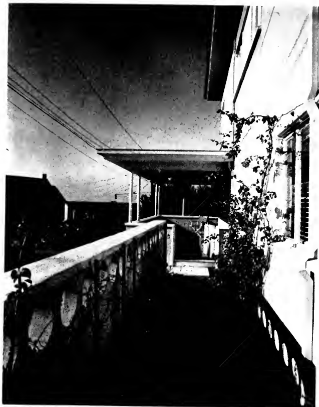
Left: Service walk, showing Concrete Grid Walls.
