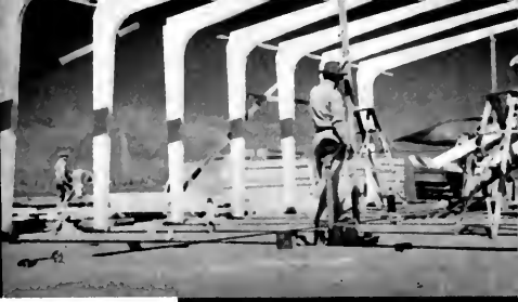
Assembling of Three-Hinged Arches
