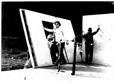
Because every step in the building and erection of this home was planned to the nth degree before a piece of lumber was cut, it goes up as easily as a house of cards. This is one of the houses in a 1000-unit project at Bremerton, Wash., which has been prefabricated in the factory, transported by truck to site, where it is easily erected by workmen in a few hours' time.
