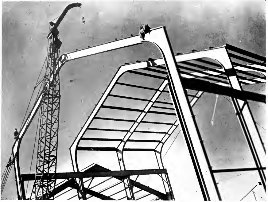
THE AUSTIN COMPANY erects rigid, welded steel framed foundry.
