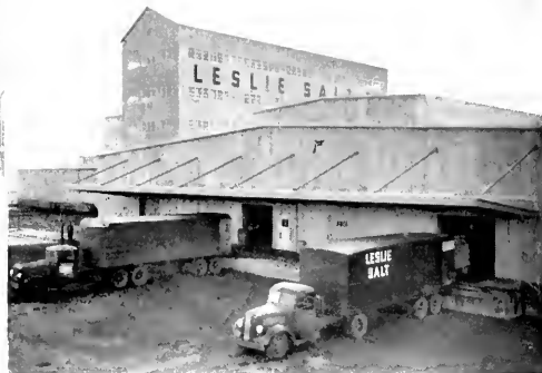
Leslie Salt Company, Newark, California, a recent Corrugated Transite installation by Western Asbestos Co.
