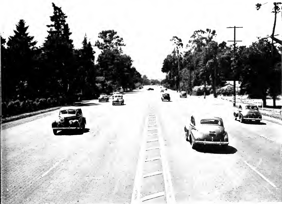
View of widened section of U. S. 101 near Atherton providing a 6-lane divided highway.
