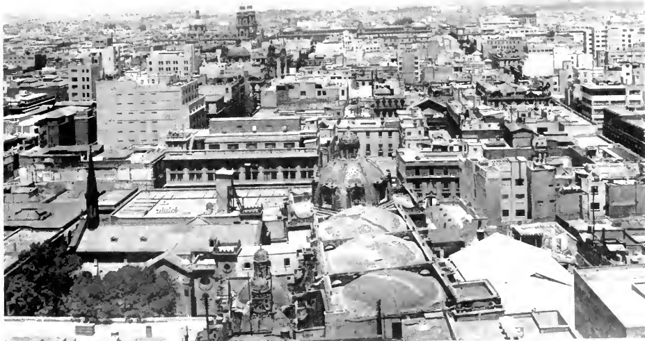
LOOKING EAST from the roof of the Seguros de Mexico building at Avenida San Juan de Letran 9, Mexico City, D. F.
