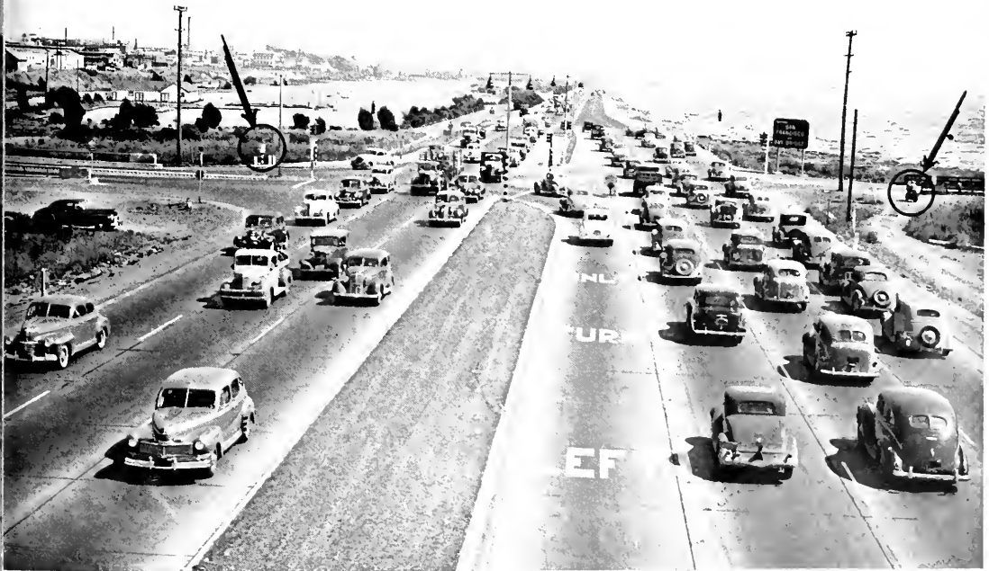
MATIC HIGHWAY CROSSING SIGNAL at intersection of East Shore Highway (left circle) between Oakland and Richmond. More than 45,000 vehicles per day are governed by this electric monitor. Note Highway Patrolman at right (in circle) governing flow of traffic. (Photo California Highways & Public Works.)
