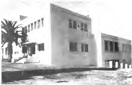
Concrete and hollow tile constructed Girls' School of Maison Carree, Algeria. Eduard Lowe, Architect
