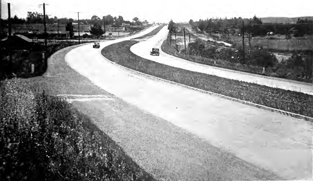
MONTEREY-CASTROVILLE-PRUNEDALE project provides highway as shown looking southerly toward Marina on 4-lane, divided Portland cement concrete pavement. Road to left is Monterey Avenue to Salinas via East Garrison of Fort Ord. (Photo courtesy Calif. Highways & Public Works.)
