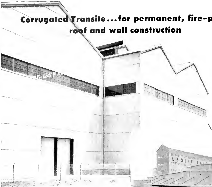
Installation by Western Asbestos Co. of Corrugated Transite for the American Forge Company, Berkeley, California.
