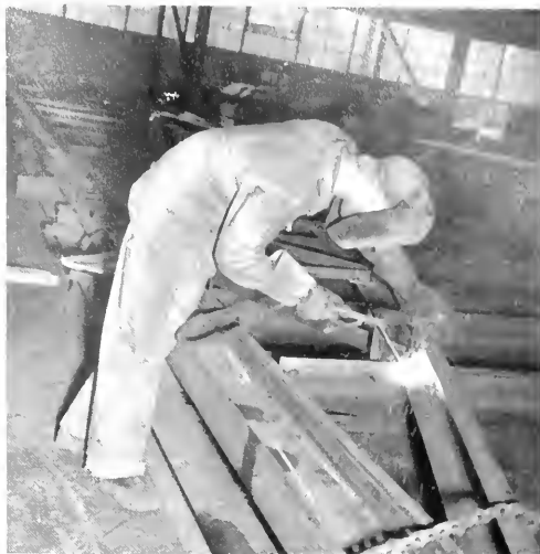
FABRICATION of curved roof truss.
