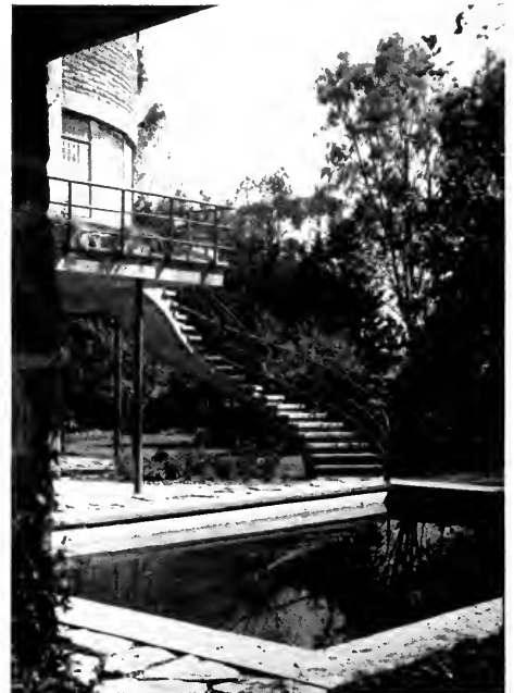
DETAIL of exterior stair from second floor to swimming pool at Dr. Font's home.
