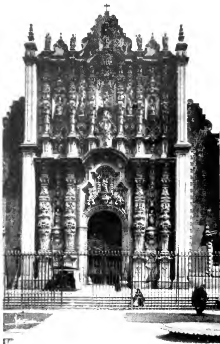
"Sagrario," for the safe keeping of sacred religious objects, in Mexico City, D.F.
