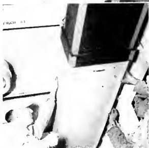
Sewing canvas over Johns-Manville BX1B insulation on a ventilating duct
