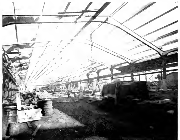
ABOVE: "Three-Form" steel column in welded sawtooth section of industrial plant structure.
