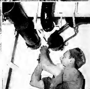
Installing low temperature cork insulation on a refrigeration system
