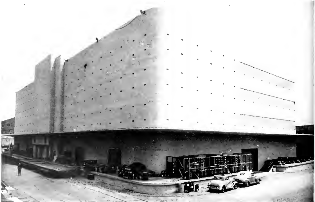
WAREHOUSE OF KAISER COMPANY, Richmond, California
