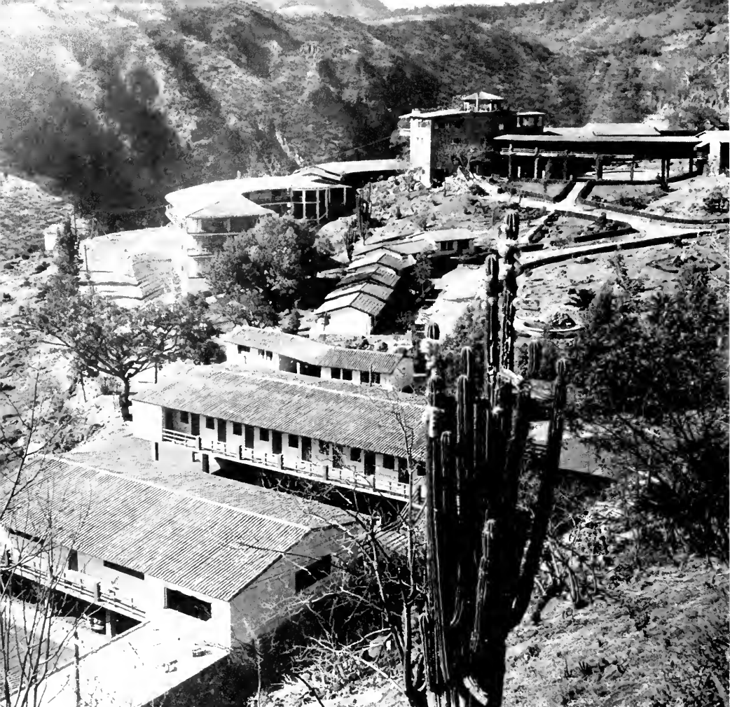
HOTEL Y BALNEARIO in San Jose Purua, Mich., Mexico, looking west with the dining room lookout being shown at the high point. Jorge Rubio, Architecto.
