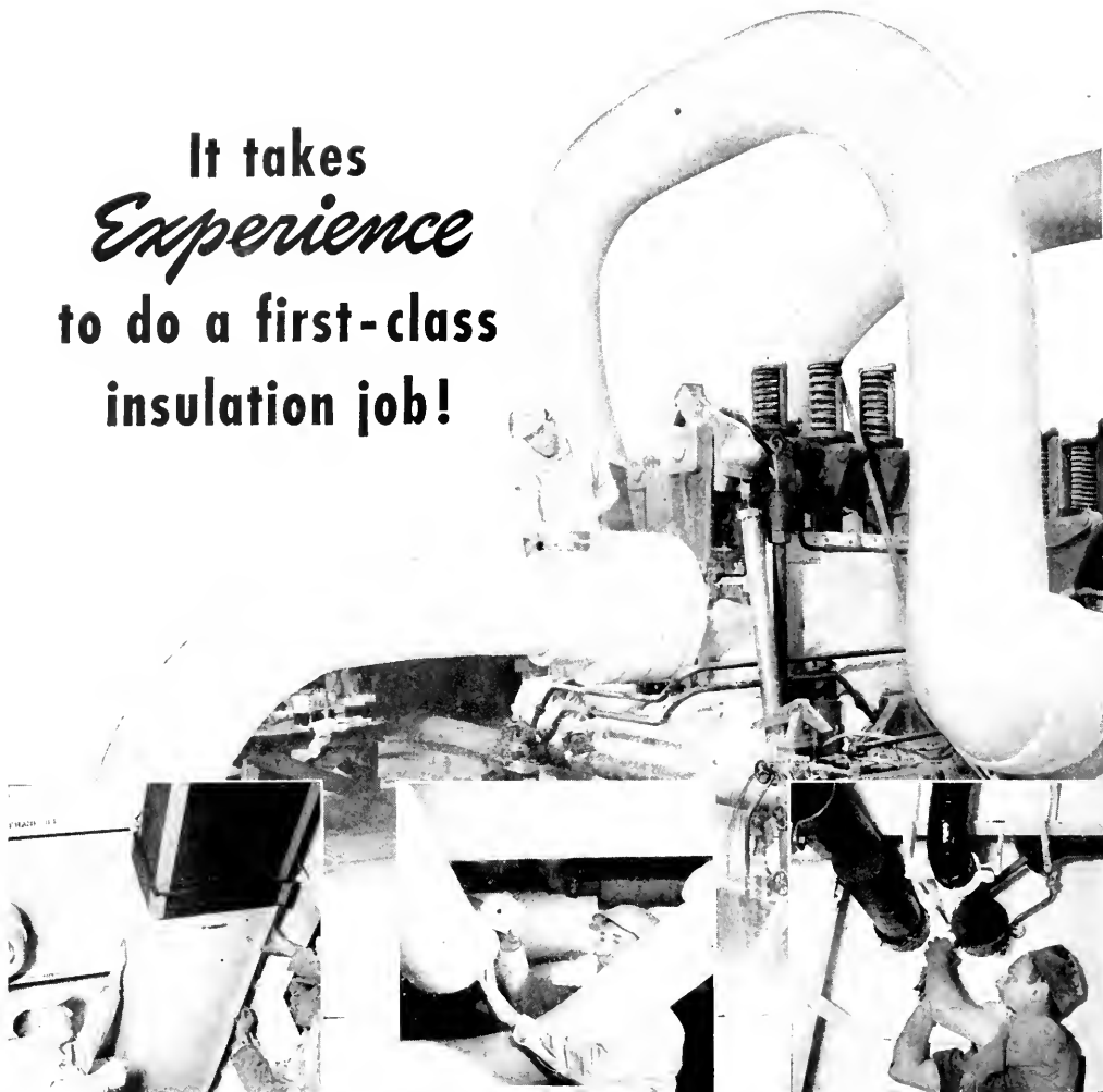
Sewing canvas over Johns-Manville BX1B insulation on a ventilating duct
