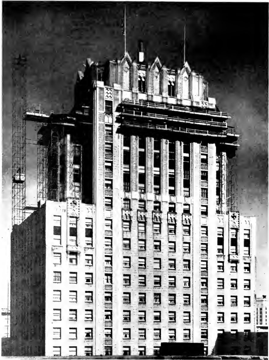
Illustrating use of scaffolding during STARLITE construction
