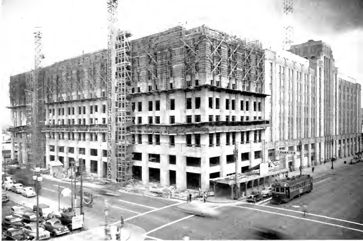
MARKET STREET AT RIGHT—NINTH STREET AT LEFT
