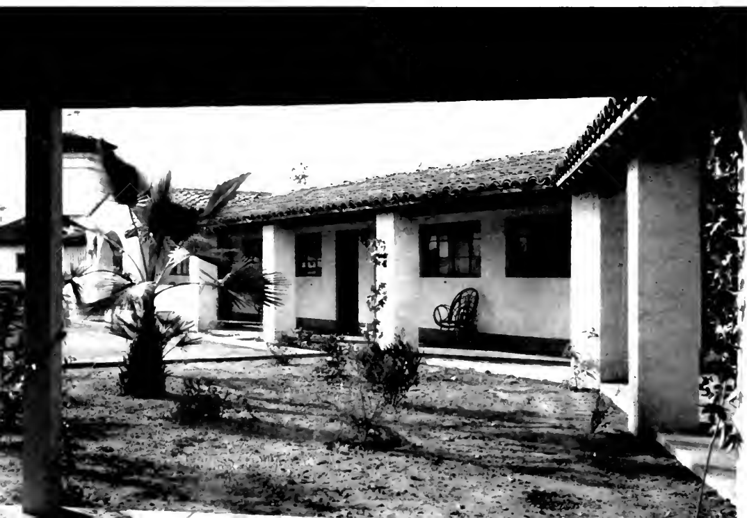
BELOW: Guest room buildings, exposed rafters, concrete block pillars and tile roof add to the pleasure of El Rancho.
