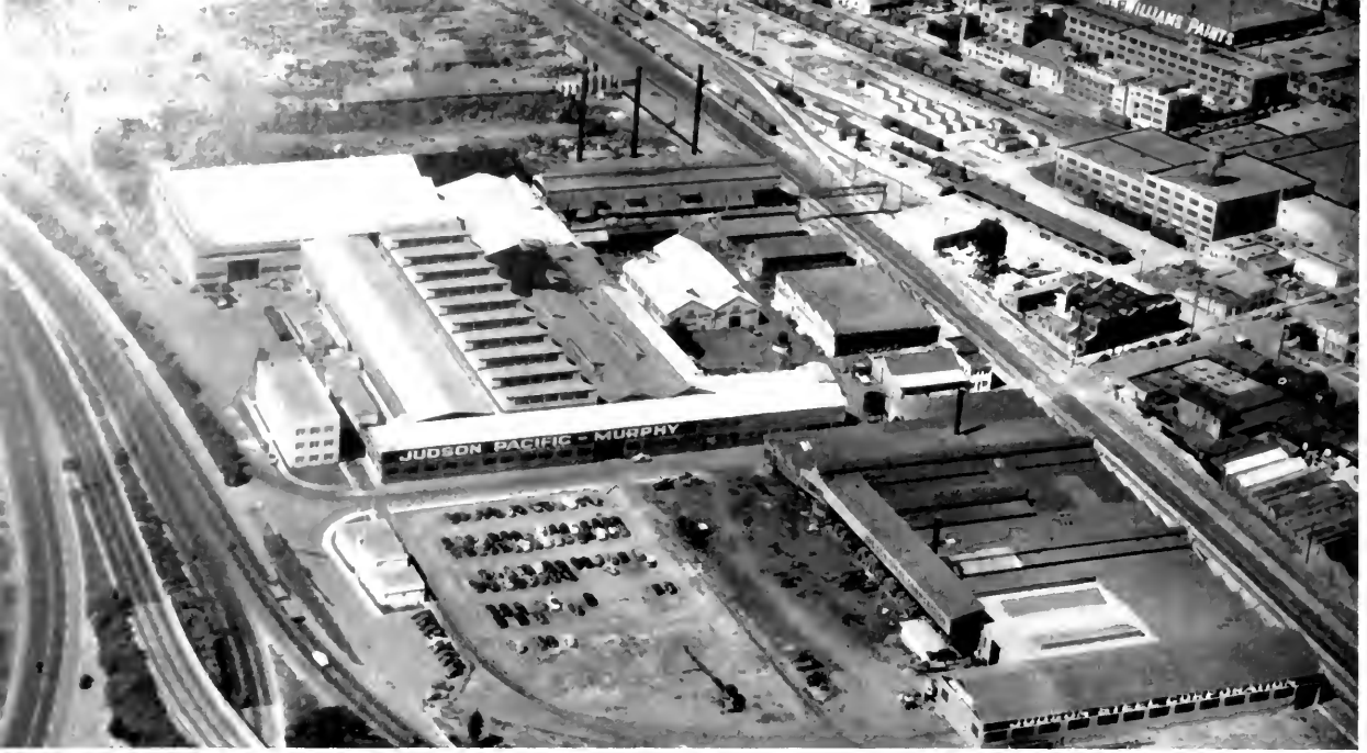
AIR VIEW OF JUDSON PACIFIC-MURPHY CORPORATION STEEL PLANT AT EMERYVILLE
