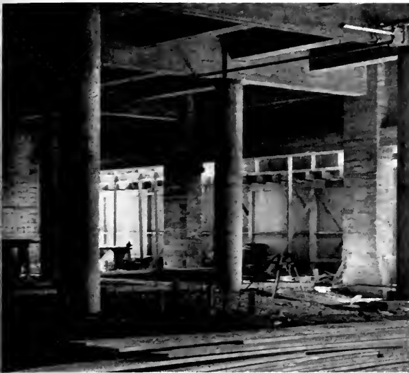
ROUGH INTERIOR: Showing sturdy reinforcing of floors and concrete pillars for upper floor support.
