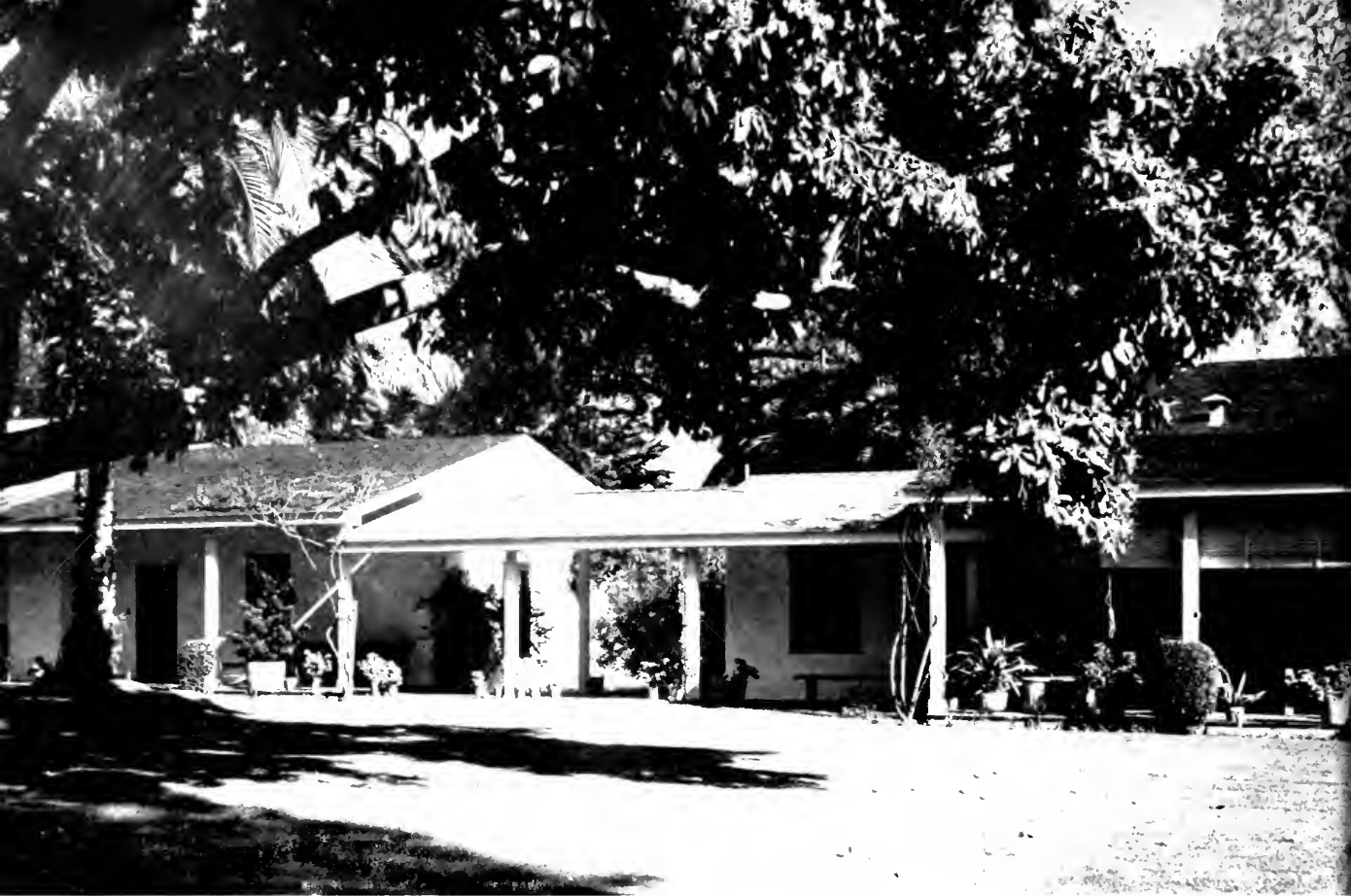
A portion of one of the Rancho Santa Fe buildings
