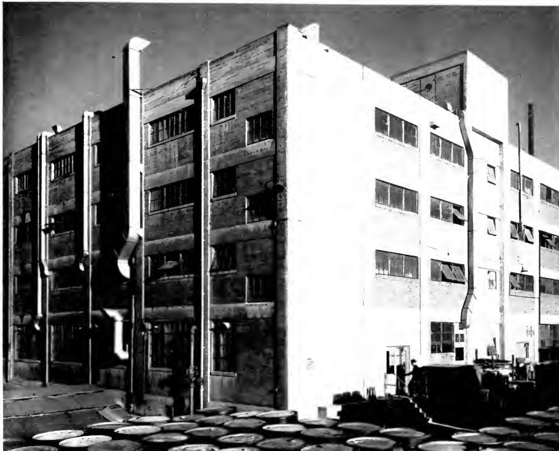
MAIN FOUR-STORY LABORATORY BUILDING
