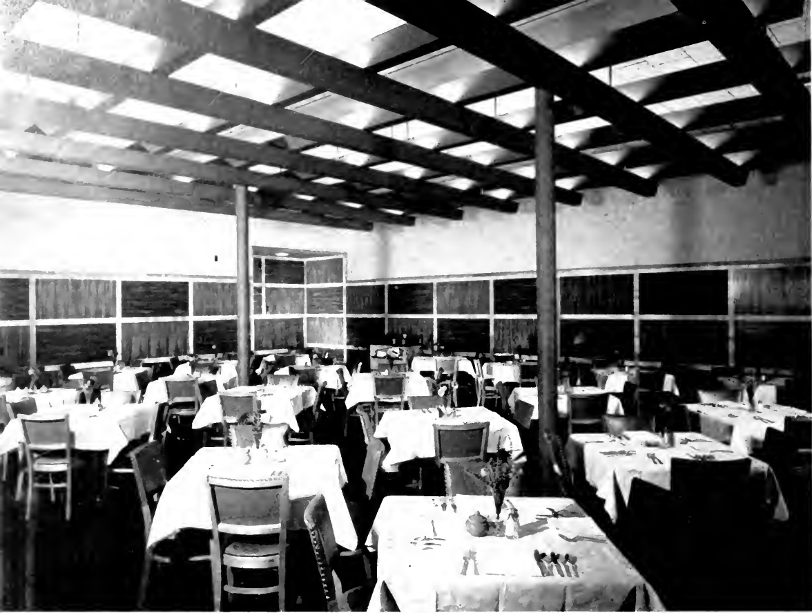
DINING ROOM—Unusual side-wall design and overhead construction
