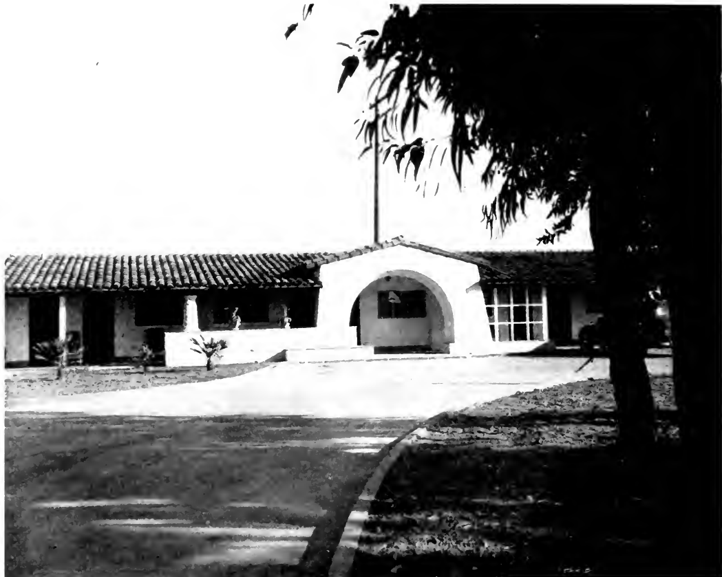
UPPER: Distinctive half circle arch entry to the tile roof porches of the concrete wall guest room buildings.
