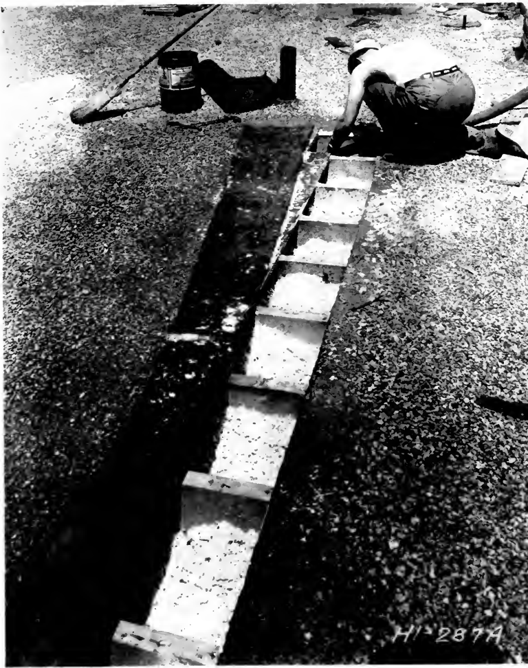
Granular mineral wool insulation being pneumatically applied to a roof. After the space between joists is filled to a depth of four to six inches, the roofing material is replaced and made water-tight.
