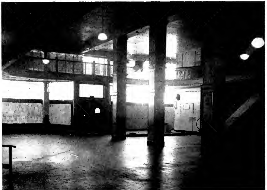
BELOW: Interior of the ground floor prior to remodeling. The problem of large center pillars and mezzanine space with unsightly stairway is clearly shown.
