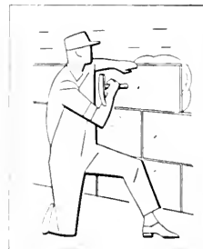
3. Ceramic Veneer is put in place, topped to fill voids.
