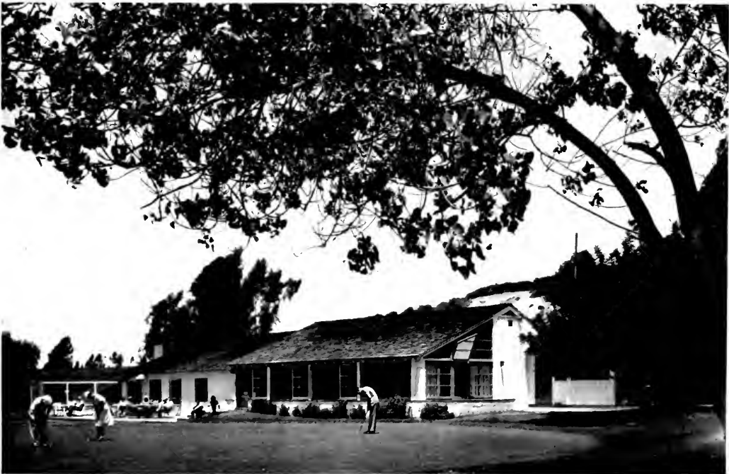
BELOW: Practice putting green and the Rancho Santa Fe golf clubhouse.
