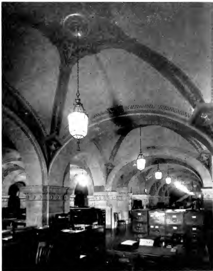
Only scientific air-diffusion could afford proper air-distribution in this room with a vaulted ceiling. Here at the Bank of America, Los Angeles, air enters the room through Anemostats. Lighting fixtures are suspended from each of these air-diffusers.
