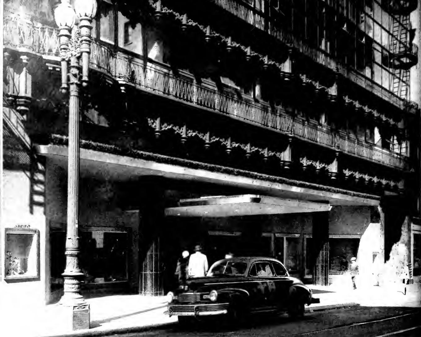
NEW STORE ENTRANCE—Recessed Display Windows
