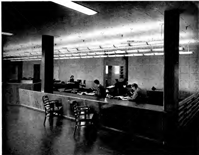
OFFICES are striking examples of uses of various woods. Individual rooms feature Red Cedar, Paneled Redwood planking, Ponderosa Pine planking and Douglas Fir Plywood. Floors are of asphalt tile, ceilings acoustical tile and walls are sheetrock.
