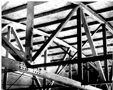
CLOSE-UP view of roof and truss members shows strength of Monochord design. Complete rigidity is had and obstructing pillars are eliminated.
