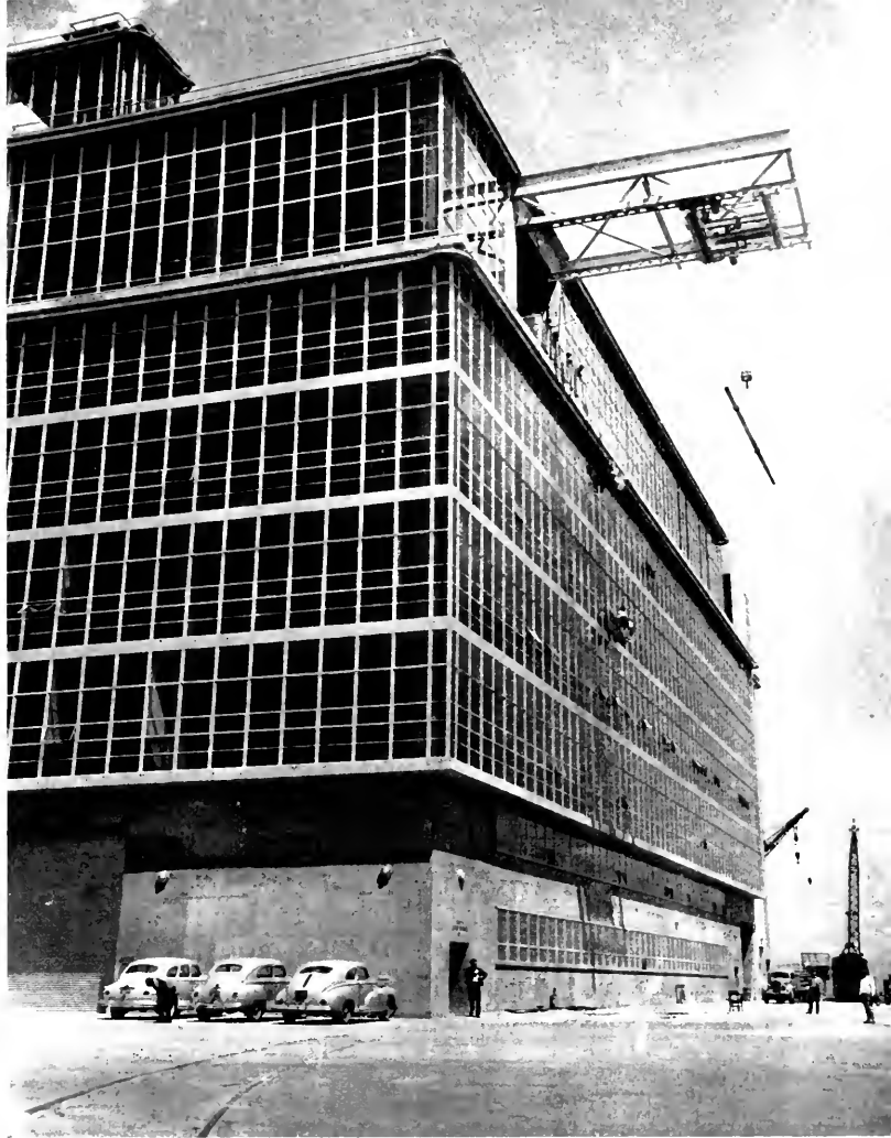
OVERHANGING monorail crane hoisting submarine periscope to sixth floor Optical Shop for calibration and repairs. (Note electric driven bos'n's chairs in use by window washers.
