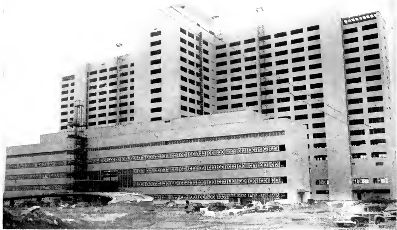
MAIN BUILDING OF THE NEW 1000 BED VETERANS HOSPITAL
