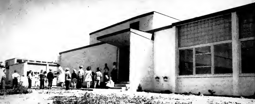
EXTERIOR has exposed concrete block wall painted with oil paint
