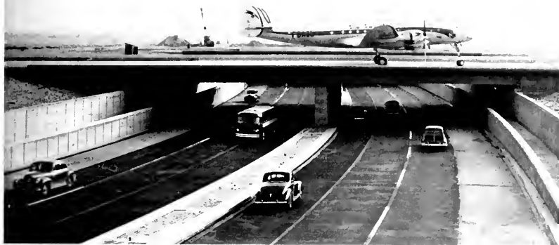
AN Air France Constellation taxis over the world's first roadway underpass built to permit the simultaneous movement of aircraft and surface vehicles at New York's International Airport. The Port of New York Authority Photo.
