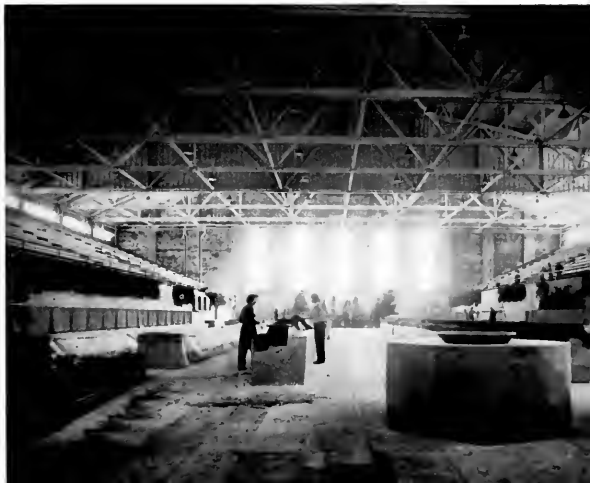
INTERIOR before maple floor is laid. Shows amphitheatre plan with permanent bleacher seats high above floor level.
