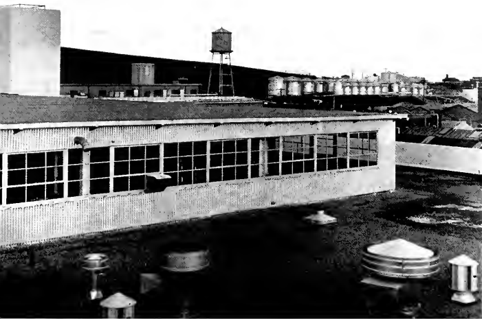
Pent House contains a lunch and recreation room which overlooks the hillside tank farm which supplies the factory's paint and varnish departments.
