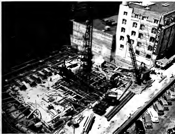
General view of foundation operations showing the driving of steel caissons.
