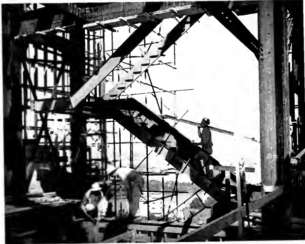
Installation of form work preparatory to pouring concrete on 14th floor.
