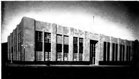
Harold H. Weeks and John W. Gloc, Architects Parker, Steffens & Pearce, General Contractors George W. Reed, Masonry Contractor
