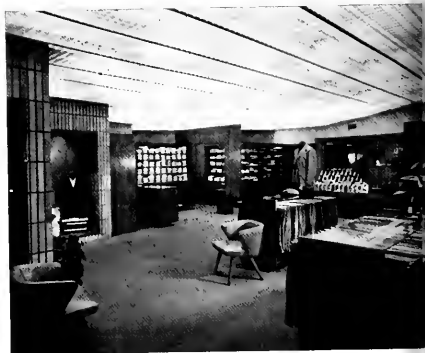
A light intensity of 120 footcandles on the merchandise without glare or shadows was obtained through a metal egg crate ceiling composed of 3-inch by 3-inch cells shielding continuous fluorescent strips on 18-inch centers.
