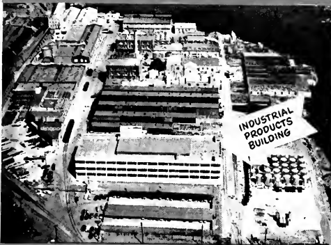
Huge South San Francisco Factory, showing new Industrial Products Building with its own Tank Farm
