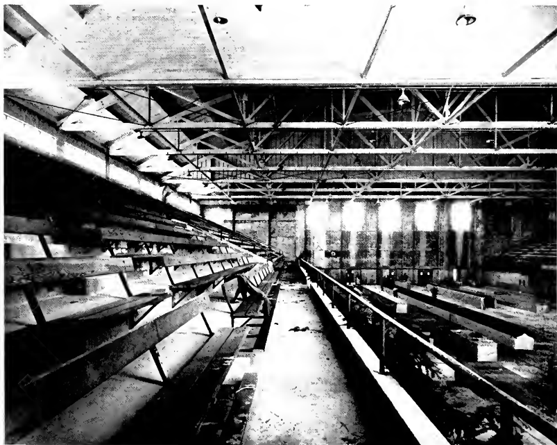
SECTION of permanent bleacher seats with attached backs, looking toward the front of the field house. Two fire walls have been built into the truss section.
