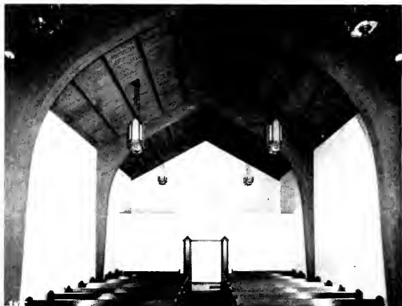
The boomerang arch in the Hollywood Congregational Church with graceful build-up of the elbow by glue lamination technique offers many unusual opportunities in the design by Architects Butler & Butler.
