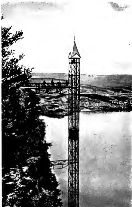
Unique indeed is the open air passenger elevator at Burgenstock which carries people from the high mountain cliffs to the lake shoreline below.
