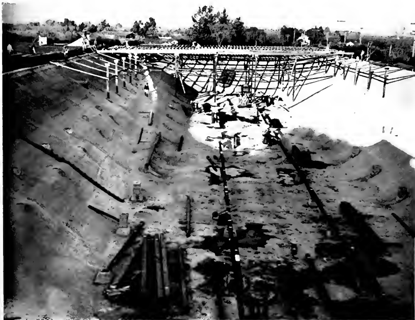
CAMBRIA RESERVOIR, California Water Service Company of San Jose, California, showing a type of work being featured by the Stolte Company along with roads, pipe lines, and other heavy construction.
