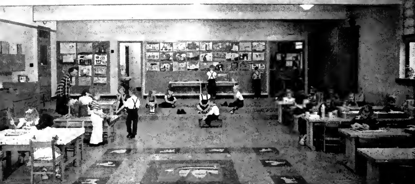
THE Floor of the Kindergarten is asphalt tile over concrete slab. Side wall is pumice block construction covered with acoustic material.
