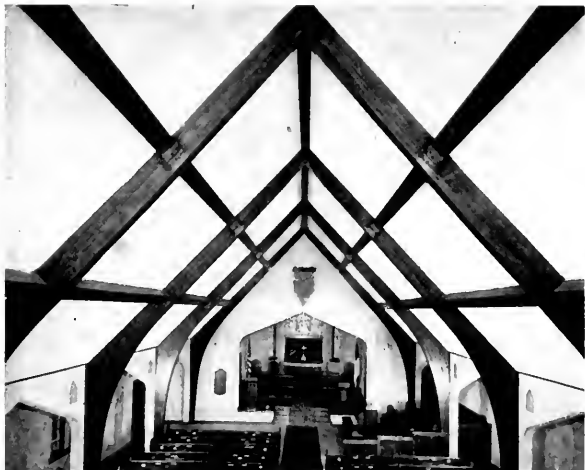
Seattle's St. James Lutheran Church by Architect C. F. Nelson offers still another evidence of individual designing of church interiors with glue laminated arches. Arches form both roof and wall support.
