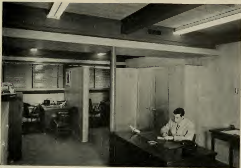
Typical office finished in West Coast hemlock panelling. Roof decking becomes ceiling and timbers of frame exposed to create attractive finish and contrast with the panelling.
