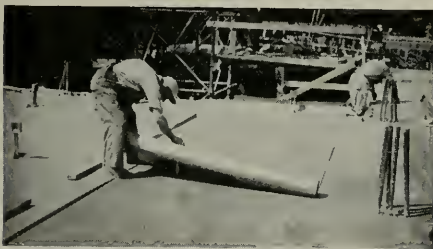
SISALKRAFT at work on 8-story Apartment Hotel, Evanston, Ill.
