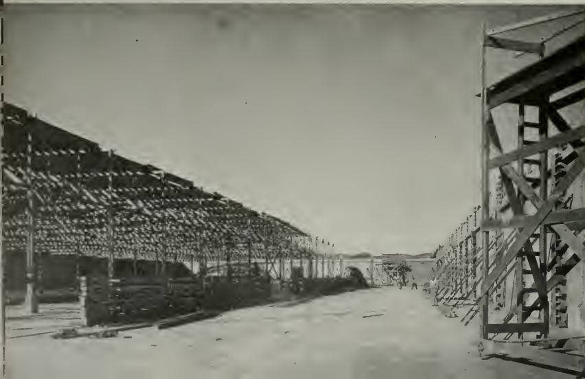
PRE-CAST tilt-up concrete walls are set on solid base
