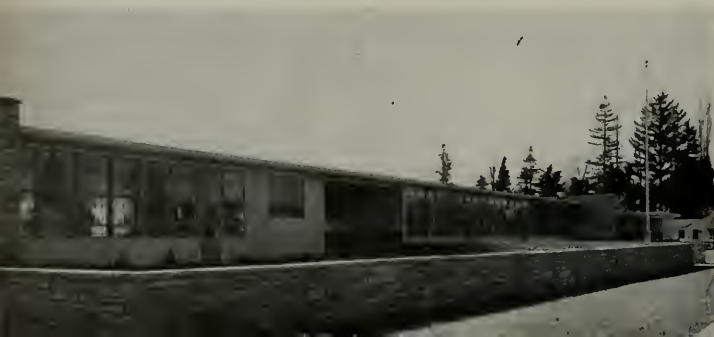
North Elevation Doyle Park School, Santa Rosa, Califor- nia, showing kindergarten wing and stone wall enclou- sure for kindergarten play area.
