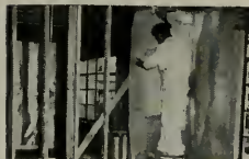
Sisalation as insulation for walls, ceilings and floors
