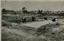
Sisalkraft under and over concrete slabs
