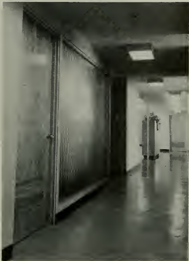
Corrugated glass partitions along interior corridor wall diffuse light and give feeling of spaciousness.
