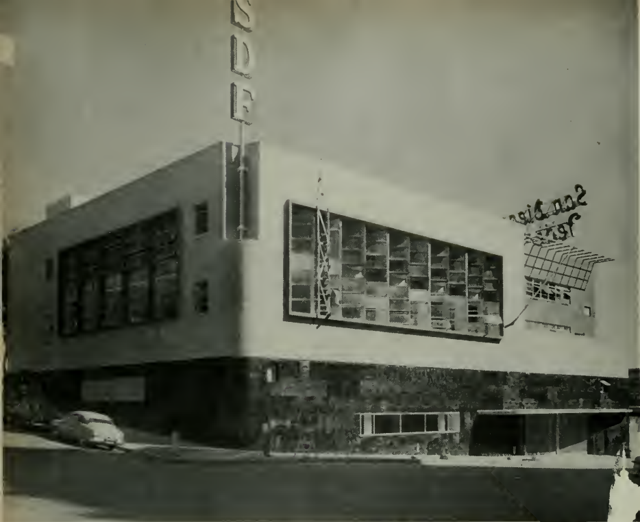
NEW BUILDING VIEWED FROM SIXTH AVENUE AND "A" STREET
