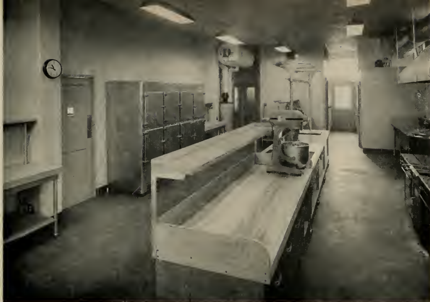
CLEAR AND CERAMIC glazed Structural Units installed in the American Radiator & Standard Sanitary Corp. plant at Torrance, California. Prack & Prack, Architects
