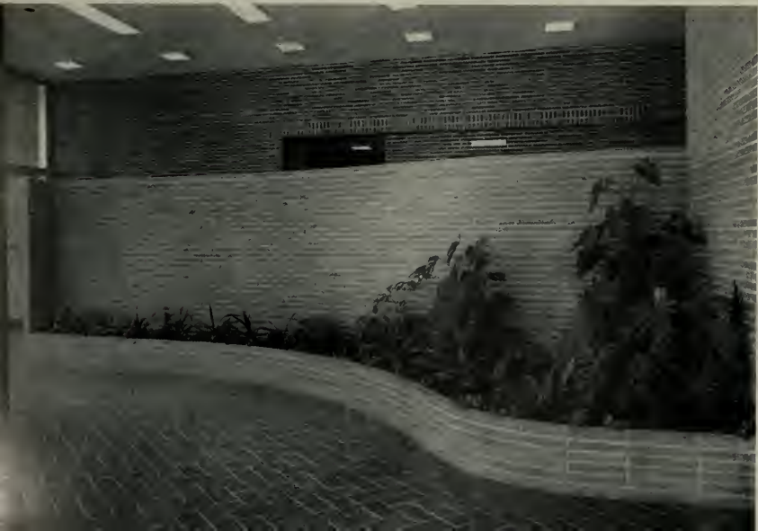
LOBBY ENTRANCE illustrates one of the interesting designs created by skillful masonry and moulded bricks.
