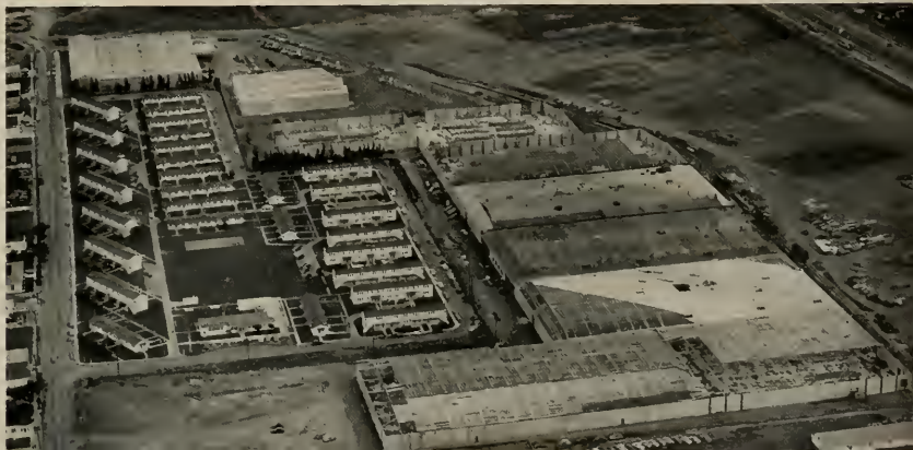
AIR VIEW of site location and one stage of construction
