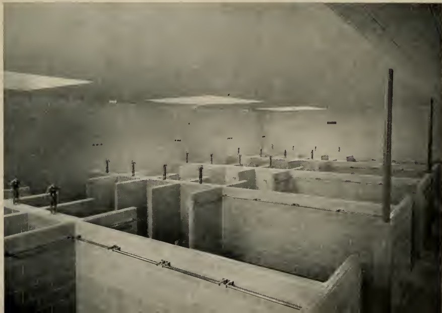
CLEAR glazed Structural Units used in girls' shower and dressing room of South East Junior-Senior High School in San Diego, California. Sam W. Hamill, Architect.
