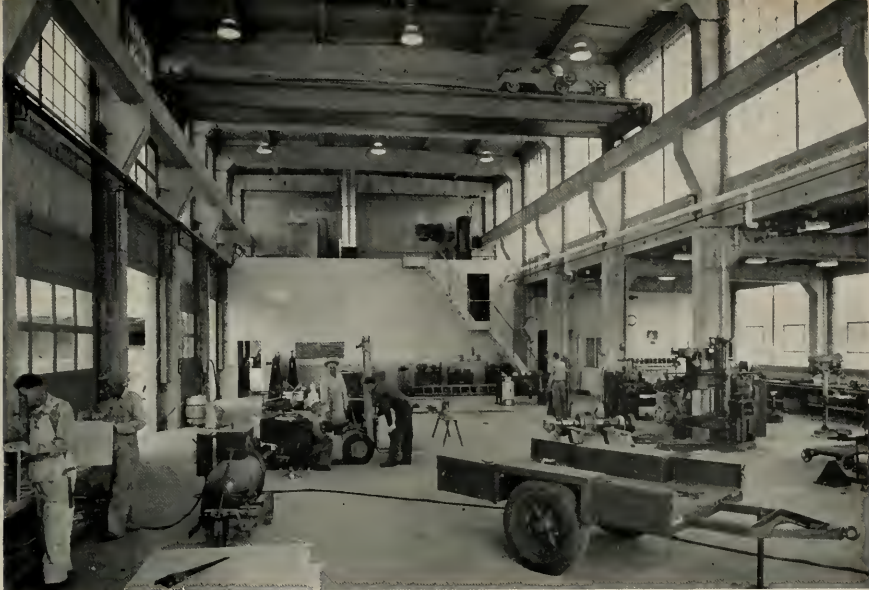
Interior of shop showing rigid frame of concrete skeleton. Concrete framing cast in single unit with overhead beams, columns, horizontal beams and corbels tied together. All work may be done indoors.
