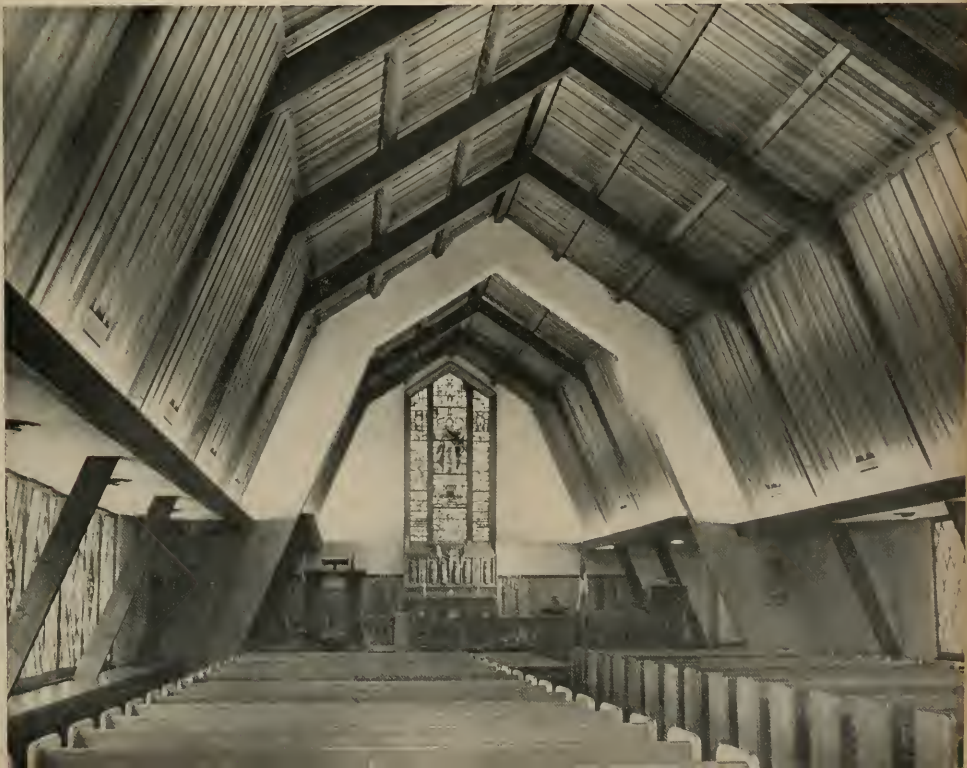
Detail of Nave and Chancel showing exposed waad-arch roof features.
