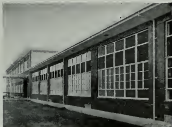
Arvin High School, Bakersfield Ernest L. McCoy, Architect
