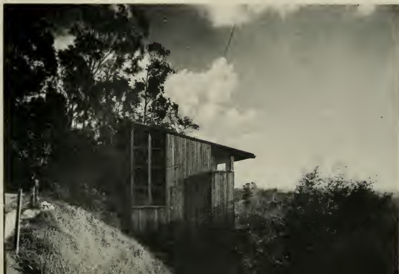
BELOW—House from street level
