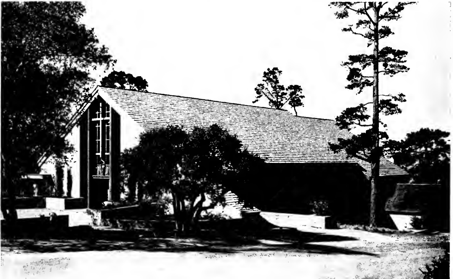
Lower View —Details landscaping arrangement of entrance; long sloping roof, and wings (at right) of lower floor level service rooms.
