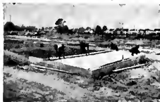
Sisalkraft under and over concrete slabs
