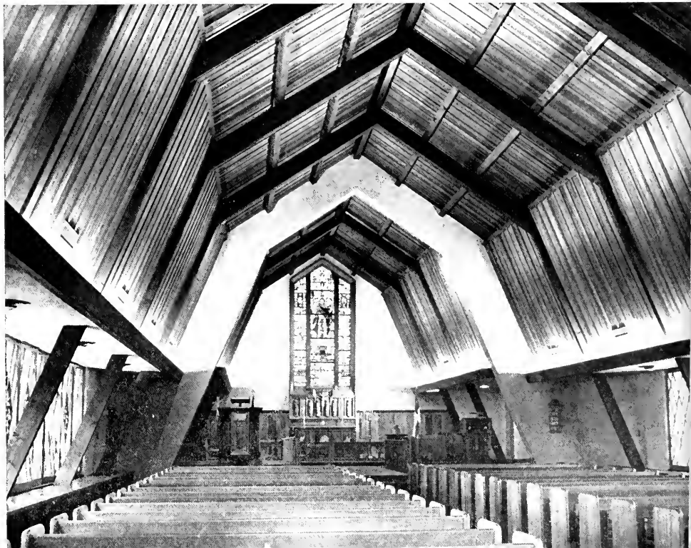
Detail of Nave and Chancel showing exposed wood-arch roof features.
