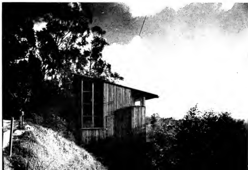
BELOW—House from street level
