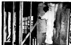
Sisalkraft as insulation for walls, ceilings and floors
