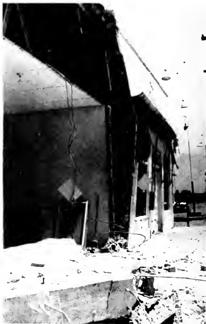
FIG. 2 Walls of this concrete block building in Arvin were not properly anchored to each other.
