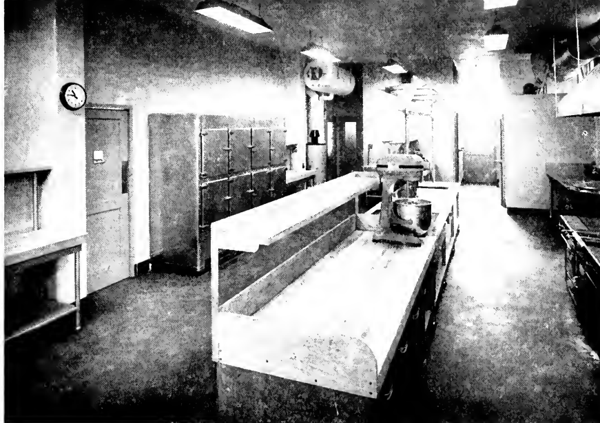
CLEAR AND CERAMIC glazed Structural Units installed in the American Radiator & Standard Sanitary Corp. plant at Torrance, California. Prack & Prack, Architects
