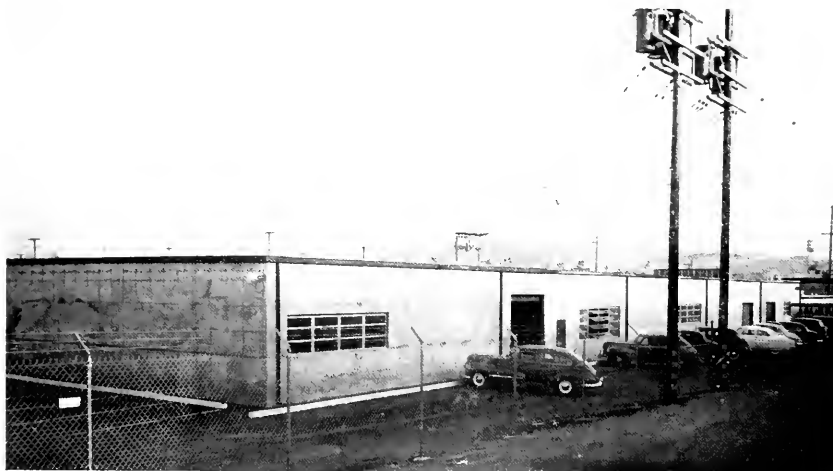
Back and side view of building showing truck income delivery point.
