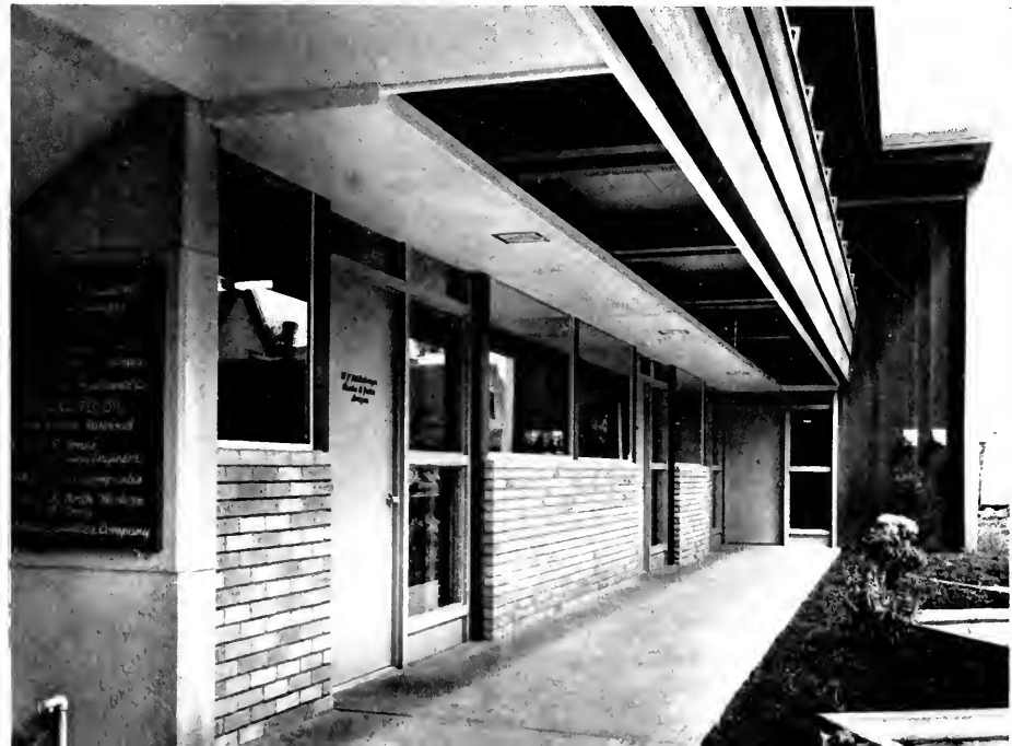
Close-up view of the exterior corridor on ground floor of the Cascade Building with detail of roof section which becomes balcony corridor.
