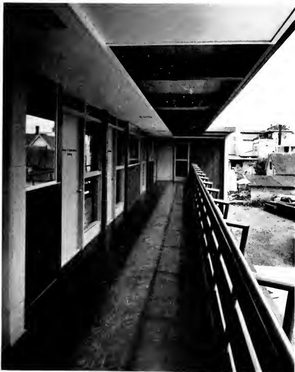
Exterior corridor from balcony level, with overhanging roof to provide ample shelter from winter storms or summer sun.
