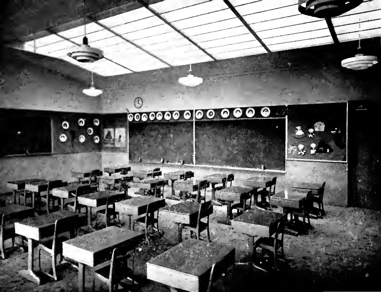
TYPICAL CLASSROOM WITH NEWLY DESIGNED TOP LIGHTING
