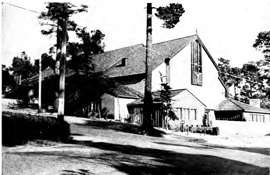
Building viewed from northwest corner, showing sloping site. Wings at right house Music Room, Rector's Office, and Parish Lounge.
