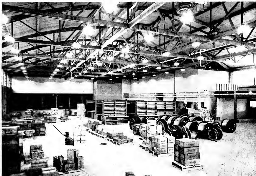
Interior of warehouse with post-free work area of 100x180 feet. A bay of windows around the entire warehouse section provides daylight.
