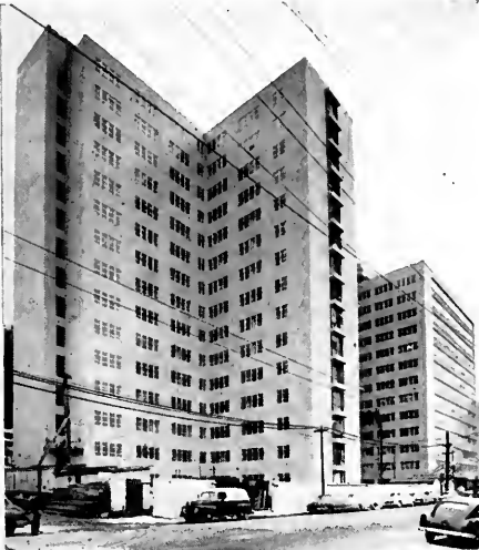
U. C. Medical Center, San Francisco. H. C. Moffett Hospital, Milton Pflueger, Architect and Medical Science Building, Blanchard & Maher, Architects; Huber & Knapik, Engineers.
