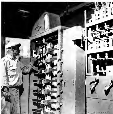
"PUSHBUTTON" CONTROL of materials handling system and batching operations—Joe Mesquite, Kraftile's 30-year man, checking controls.
