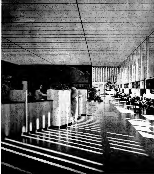
LUMINOUS CEILING illustrated above is implemented with instant-start fluorescent lamps above corrugated plastic.
