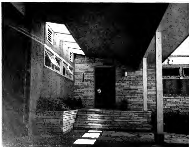
Flagstone steps lead from carport to main entrance door, protected by roof overhang. For privacy from road, windows are high.
