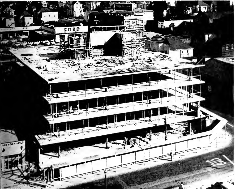
TIOGA BUILDING with floor slabs in permanent position ready for installation of exterior glass walls.
