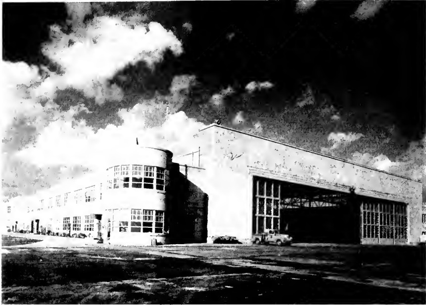
HANGAR and Administration Building, N. S. Naval Reserve Aviation Base, Oakland.
