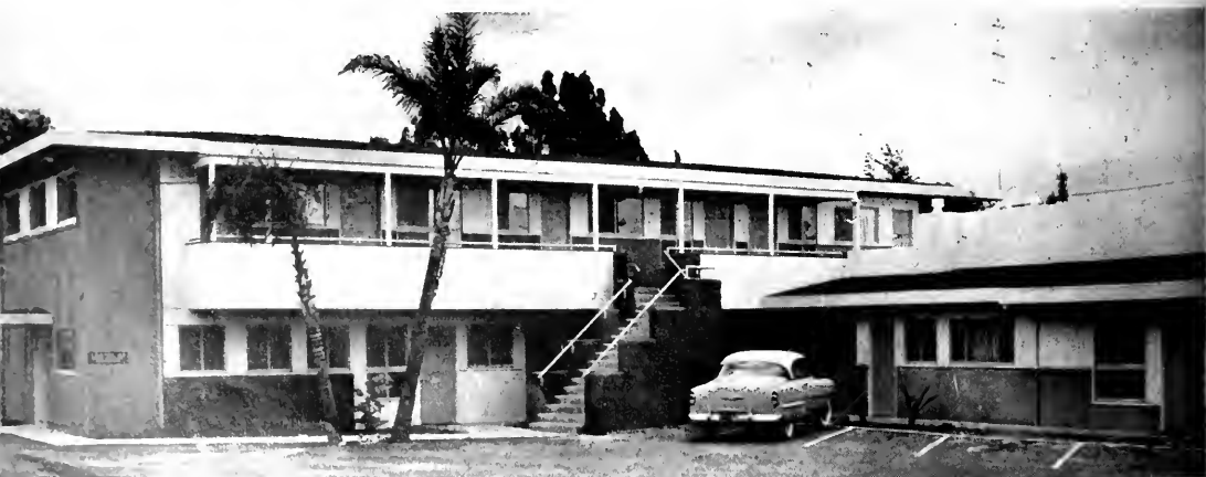
CLOSE-UP view of two story portion of the Grossmont Professional Building, indicating type of architecture and construction.
