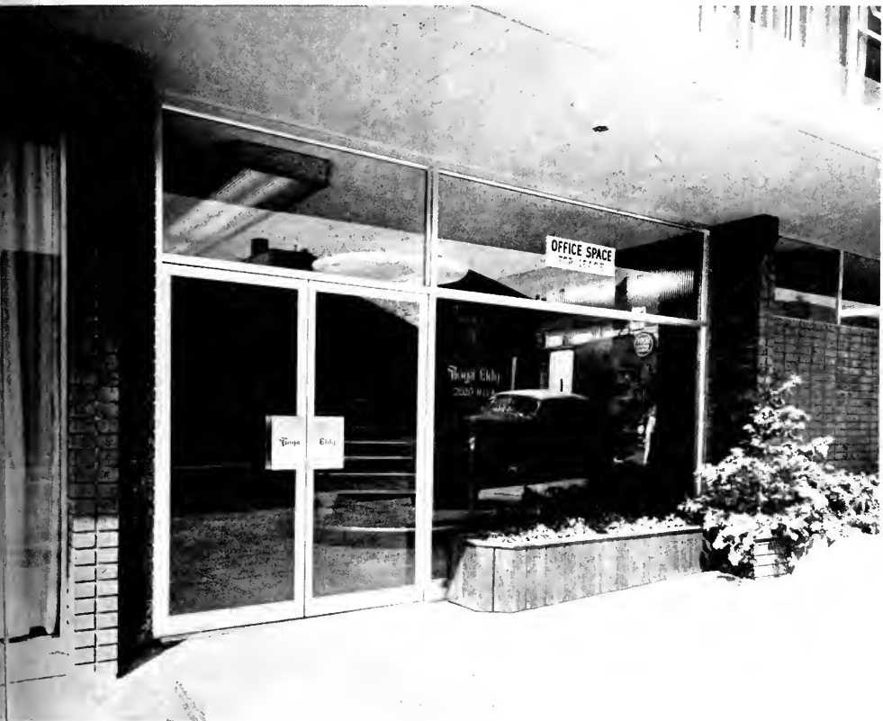
ENTRANCE to the attractive building, showing modern hollow bulbar doors with identification push plates.
