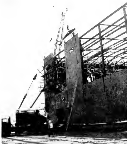
TILT-UP CONCRETE SLAB is being hoisted into second floor position for affixing to steel.
