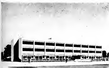
SANTA CLARA COUNTY JAIL AND SHERIFF'S DEPARTMENT FRANK C. TRESEDER, A.I.A., ARCHITECT 100 LAFAYETTE ST. SAN FRANCISCO, CALIF.
