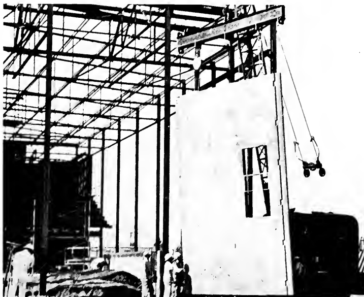
TILT-UP CONCRETE SLAB is being hoisted into second floor position for affixing to steel.
