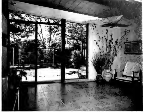
INTERIOR... view looking toward patio and pool, spacious floor to ceiling glass end-wall, exposed wood ceiling, asphalt-tile floor.
