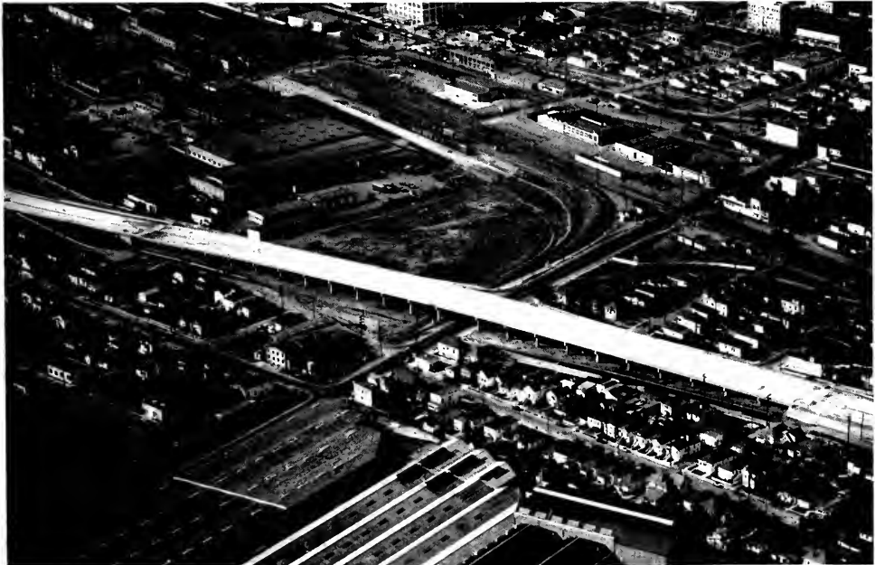
BELOW: Aerial view of Fruitvale (Oakland) Freeway overpass.
