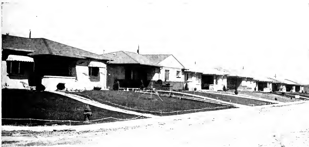
TYPICAL STREET VIEW
