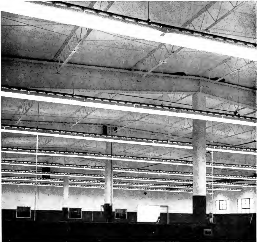
FIG. 1 — LIGHTING FIXTURES in this open-area installation cast an upward light which reduces contrast between ceiling and fixtures and neutralizes any distinct lighting contrast.
