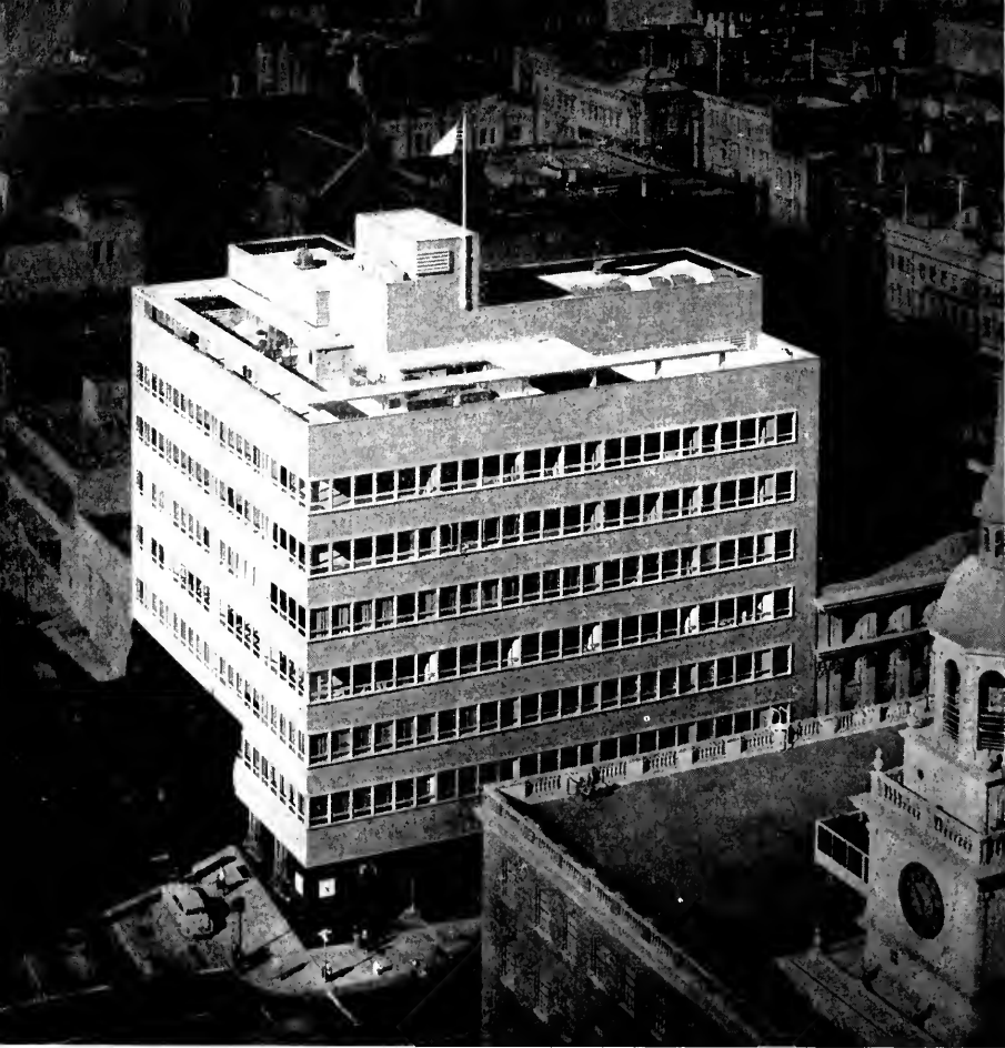
PACIFIC MUTUAL BUILDING, San Francisco LOUBET & GLYNN, Architects
