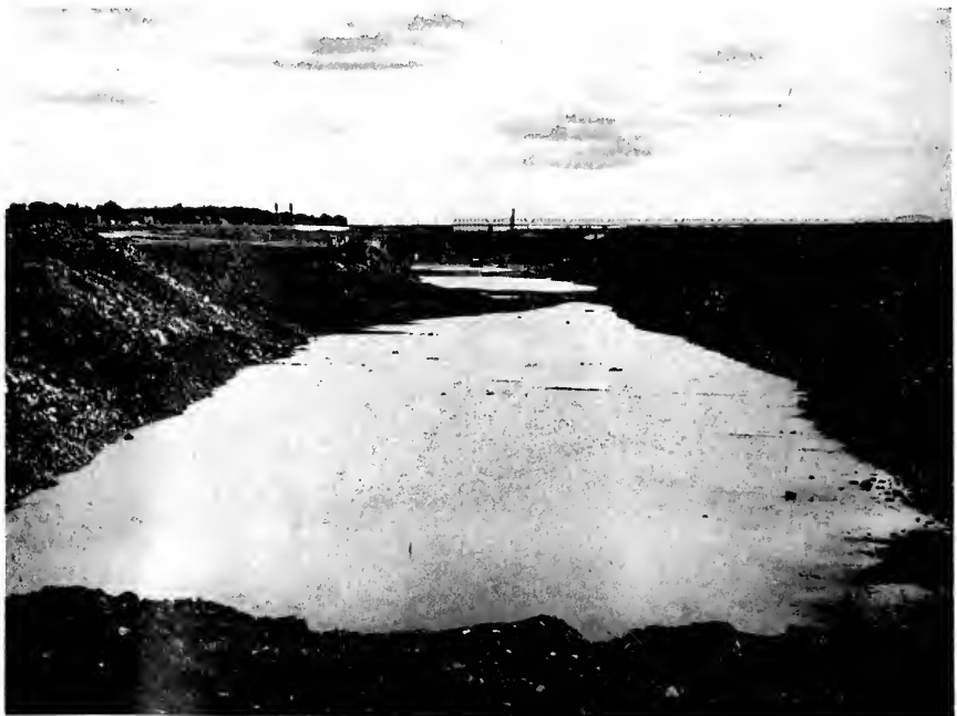
SHIP CHANNEL between Jacques Cartier and Victoria bridges— 3,000,000 cu.yds. of rock excavation in 7,600 ft. of channel.
