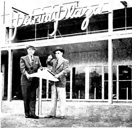
Frank Petrini, market owner, and Sewall Smith (right), architect, discuss construction detail.
