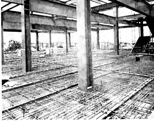
STEEL in place for concrete pouring.
