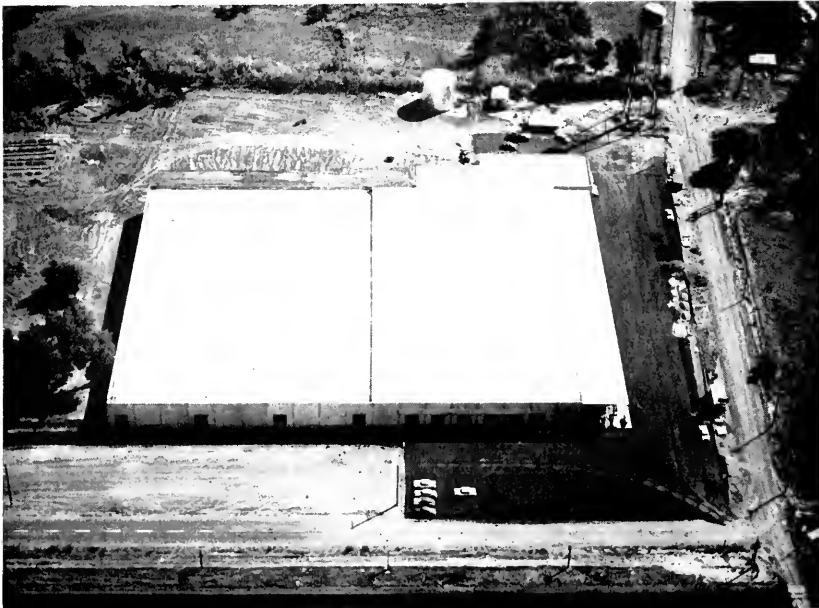
THE BERT McDOWELL office and warehouse, Redding, California
