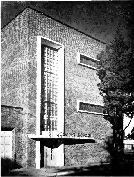
DETAIL of ENTRANCE
