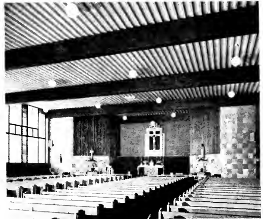
Wide nave is no problem for these laminated beams in this church.
