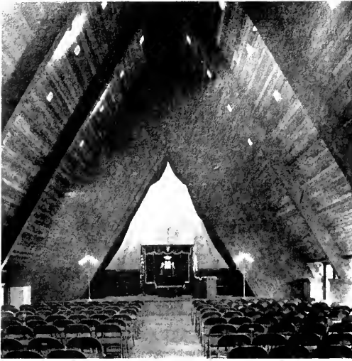
TEMPLE BETH JACOBS CHURCH, Oakland, California, designed by Albert Hunter, Architect. The wedge shaped roof offers beauty and simplicity.
