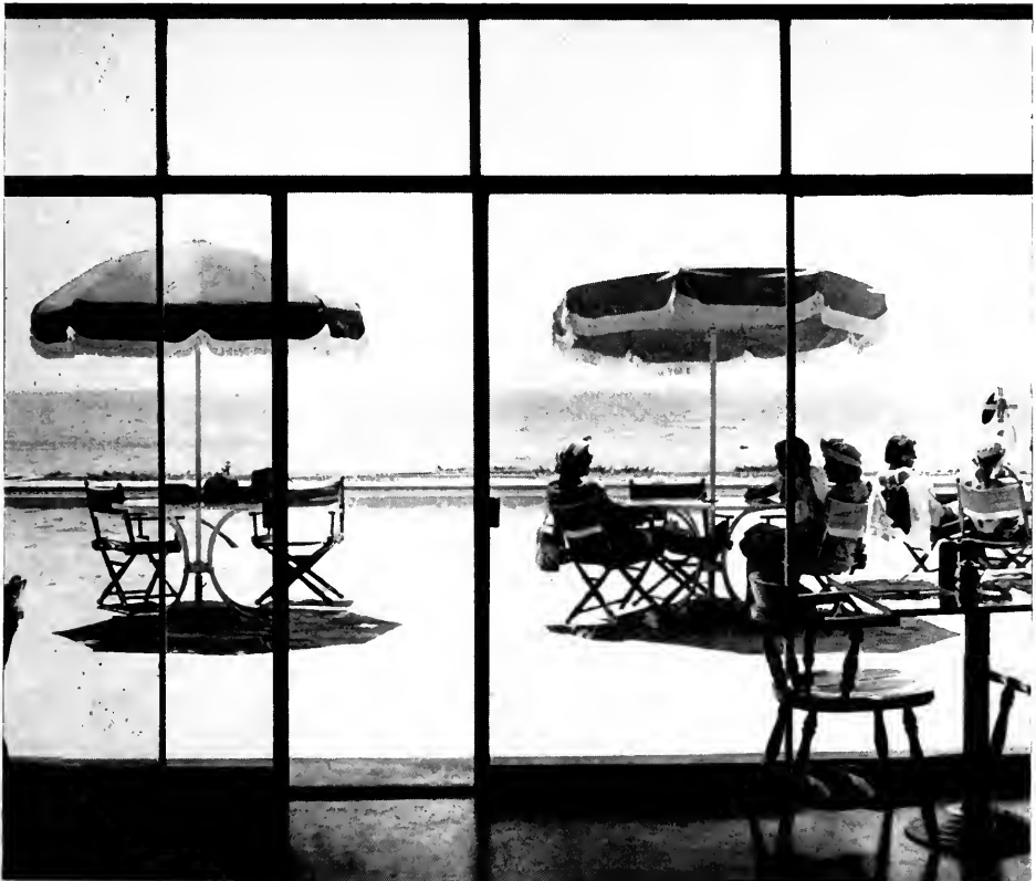
THE PORTUGUESE BEND CLUB utilizes wall of sliding glass doors as only separation between club facilities and the ocean itself. Tight weatherstripping on doors provides protection against ocean breeze during cool days, but preserves view for maximum enjoyment. Kenneth Neptune, Architect, A.I.A.
