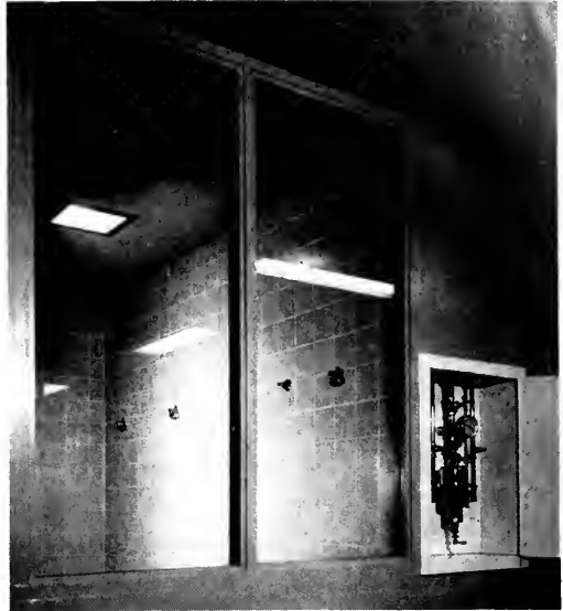
TYPICAL shower room with walls tiled to ceiling . . . oatmeal tile.
