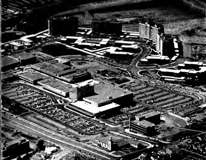
STONESTOWN, San Francisco. Aerial view of large development work.
