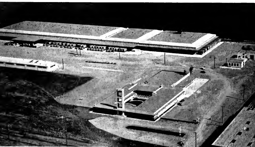
WAREHOUSE AND OFFICES constructed for Lucky Stores, Inc., San Leandro, Calif.
