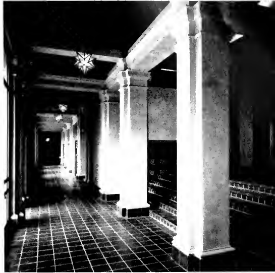
INTERIOR VIEW of the Main Corridor of the Chapel entrance, showing combination use of wood panel ceiling, tile floors and decorative tile wainscoting.
