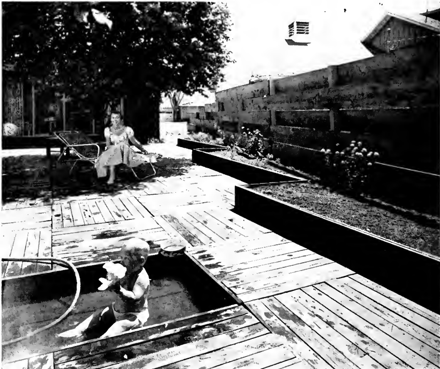
To give the James Luckey family lounging and play room, Architect Louis F. Bronson III decked the entire backyard with Douglas fir and enclosed the area with a distinctive fence.
