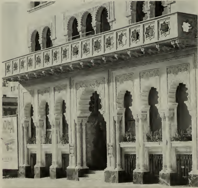
DETAIL, LOWER STORY, ALHAMBRA APARTMENTS J. F. Dunn, Architect
