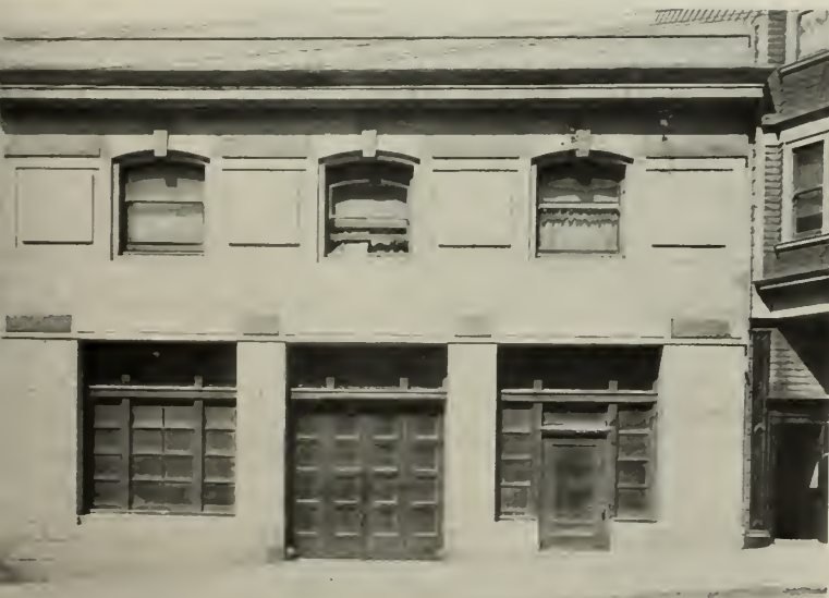
A CLASS C PRIVATE GARAGE WITH CHAUFFEUR'S QUARTERS ABOVE
