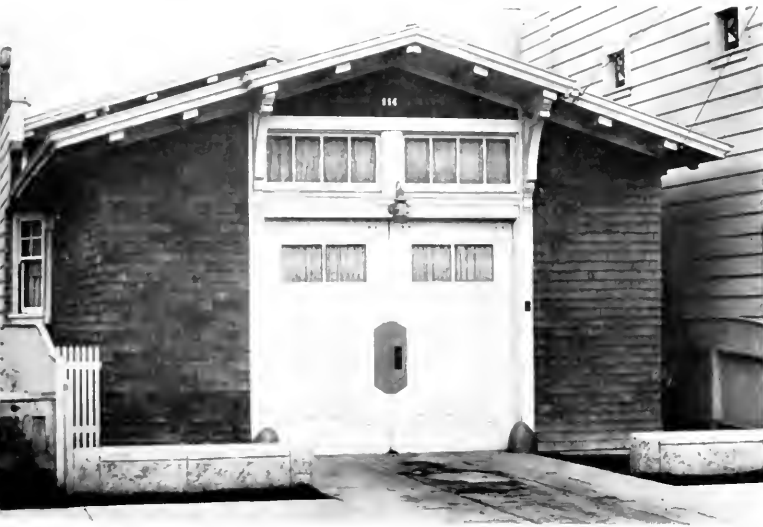
Garage with chauffeur's apartments in rear, for Mr. Frederick Hohwiesner, San Francisco Nathaniel Bleisdell, Architect
