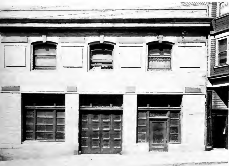
A CLASS C PRIVATE GARAGE WITH CHAUFFEUR'S QUARTERS ABOVE
