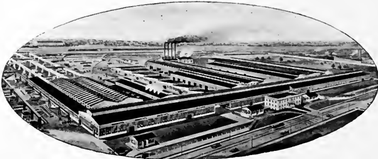
BIRD'S-EYE VIEW OF TRUSSED CONCRETE STEEL COMPANY'S PLANT, YOUNGSTOWN, OHIO
