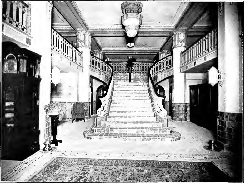
STAIRCASE TO MEZZANINE FLOOR, REAR OF LOBBY, STOWELL HOTEL Frederick Noonan and William Richards, Architect and Engineer Tile Work by Parker Tile & Mantel Co.
