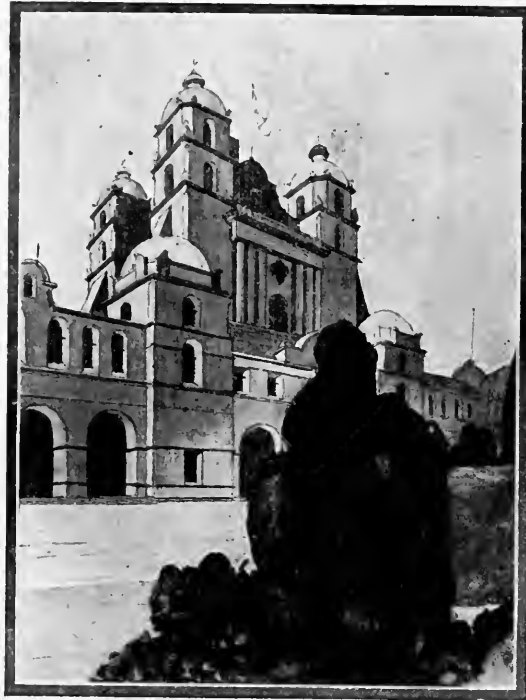
MAIN ENTRANCE TOWER, CALIFORNIA STATE BUILDING
