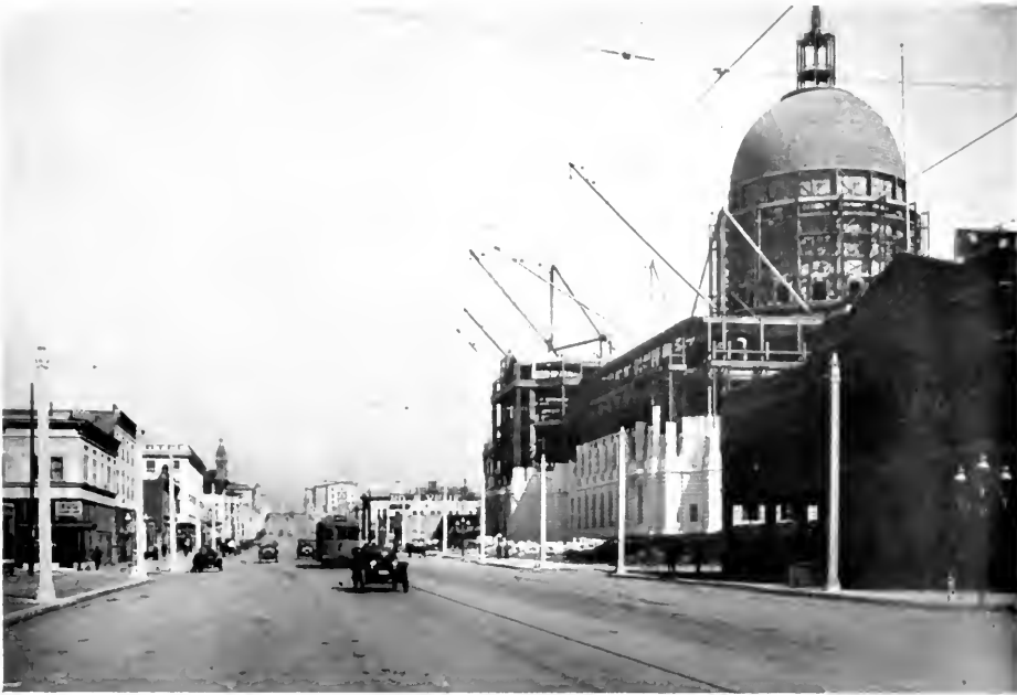
SHOWING CONCRETE POLES OF MUNICIPAL RAILWAY, VAN NESS AVE., SAN FRANCISCO
