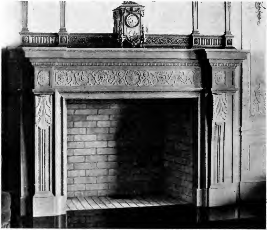
GREY TENNESSEE MARBLE MANTEL IN EHRMANN RESIDENCE, SAN FRANCISCO Designed by Willis Polk & Co., Architects
