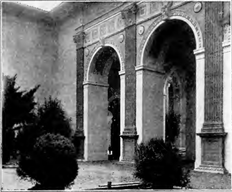
ENTRANCE TO COURT OF FOUR SEASONS Henry Bacon, Architect
