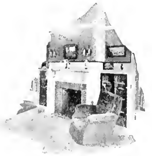
Detail of fireplace in living room. Brick laid in Medusa Waterproofed Stainless White Cement.
