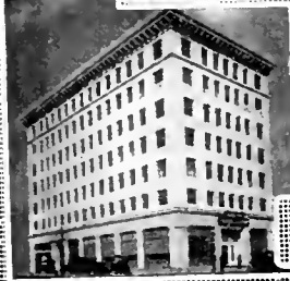
OFFICERS SAVING BLDG. PASADENA, CAL.
