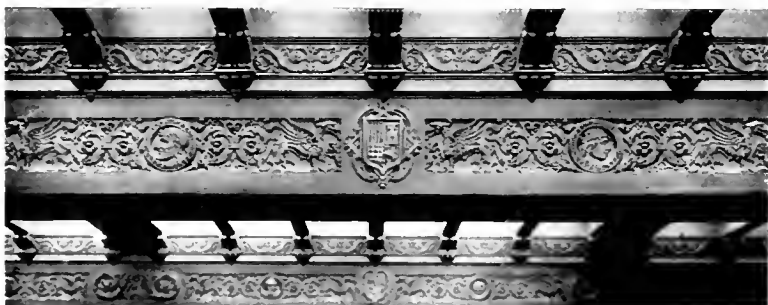
DETAIL OF CEILING IN LOBBY
