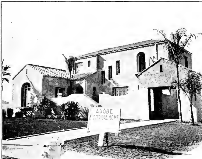
ELECTRICAL HOME, LOS ANGELES
