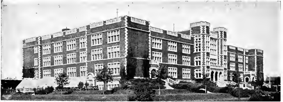
CENTRAL HIGH SCHOOL, MINNEAPOLIS, MINN.
