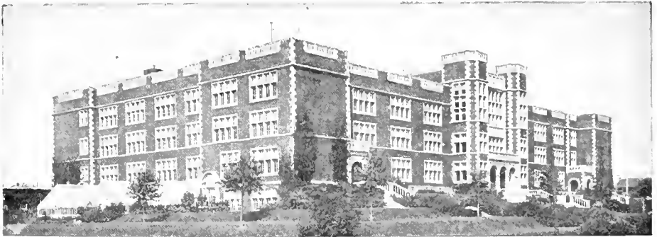
CENTRAL HIGH SCHOOL, MINNEAPOLIS, MINN.
