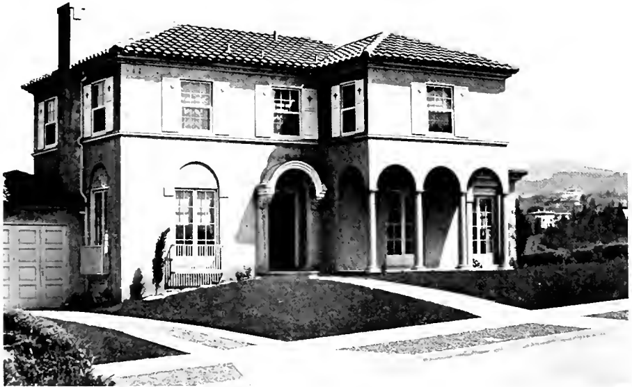
HOUSE FOR MR. A. L. GROSSMAN, OAKLAND (See next page) Will E. Schirmer and Arthur S. Bugbee, Associate Architects
