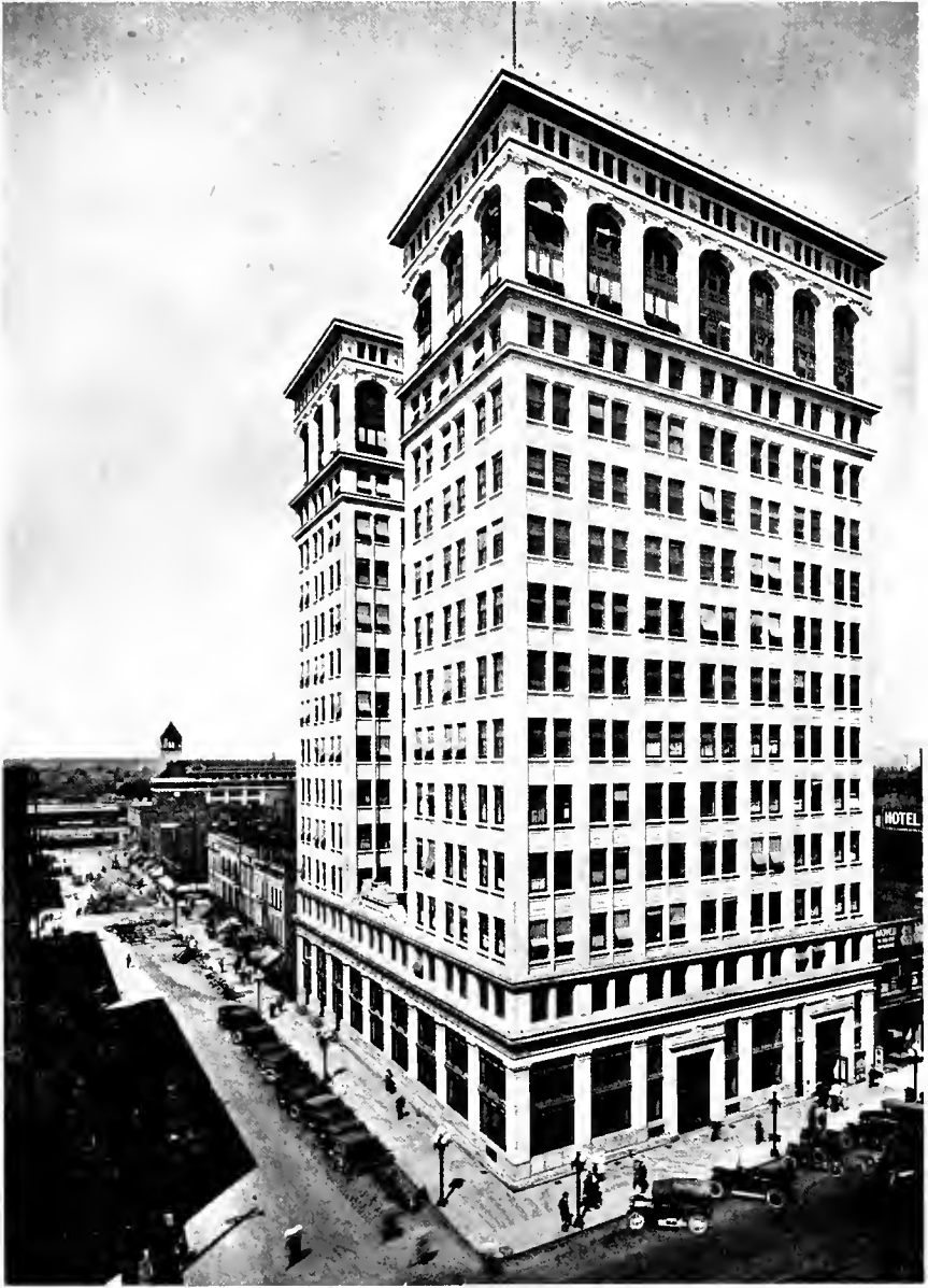
OLD NATIONAL BANK BLDG., SPOKANE, WASH. D. H. BURNHAM & CO., ARCHITECTS
