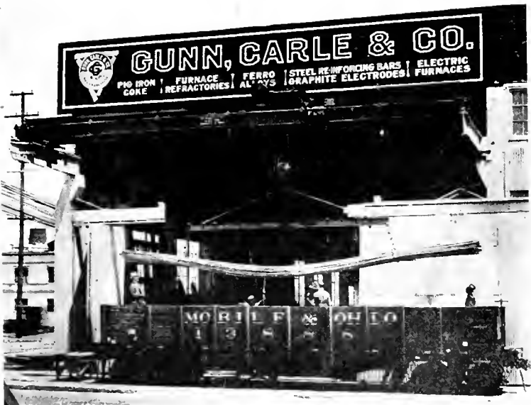
SPUR TRACK, OVERHEAD CRANE AND CAR LOAD Gunn, Carle & Co. Warehouse San Francisco
