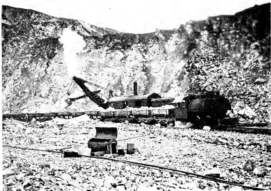
PIEDRA ROCK COMPANY'S PLANT Close-up of quarry face, showing No. 70 Bucyrus steam shovel loading train enroute to crusher.
