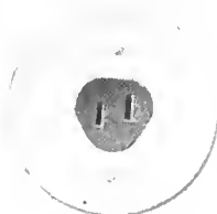
The finished ceiling Elexit
