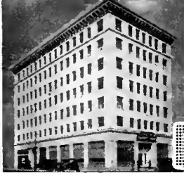
CITIZENS SAVINGS BLDG. PASADENA, CAL.
