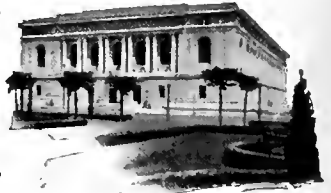
Carnegie Library San Francisco; all sheet metal and iron grills on windows are of Armco Ingot Iron. Geo. W. Kelham, Architect.
