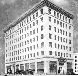
CITIZENS SAVINGS BLDG. PASADENA, CAL.
