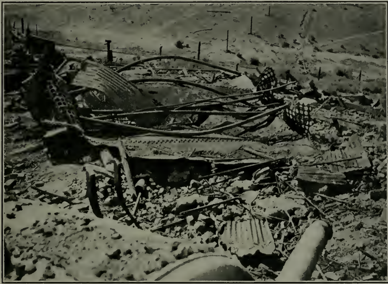
FIG. 2—VIEW OF THE EXPLODED BOILER
