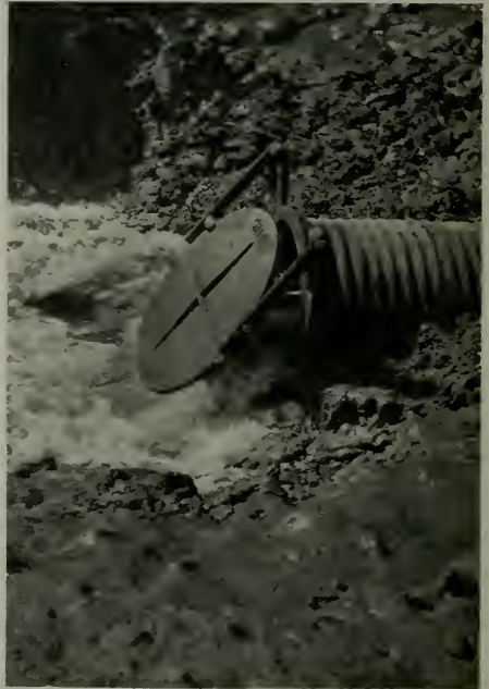
CALCO AUTOMATIC DRAINAGE GATE DRAINING RECLAIMED LAND
