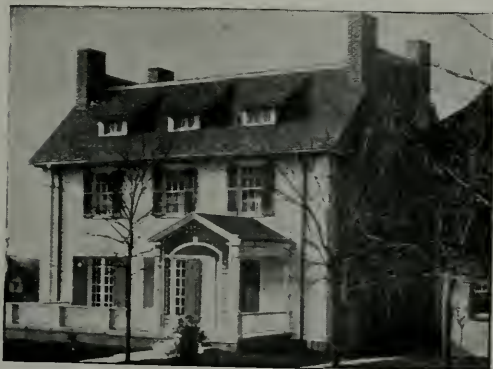
Walls finished with Cabot's Old Virginia White Roof finished with No. 346 Dark Gray Creosote Stain Walter Boschen, Architect, St. Joseph, Mo.
