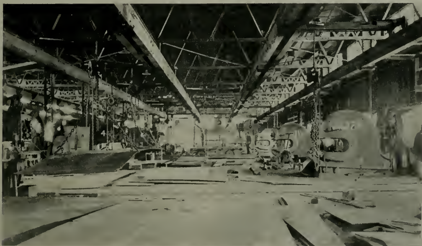
INTERIOR VIEW OF FABRICATING SHOP, UNION CONSTRUCTION COMPANY, OAKLAND
