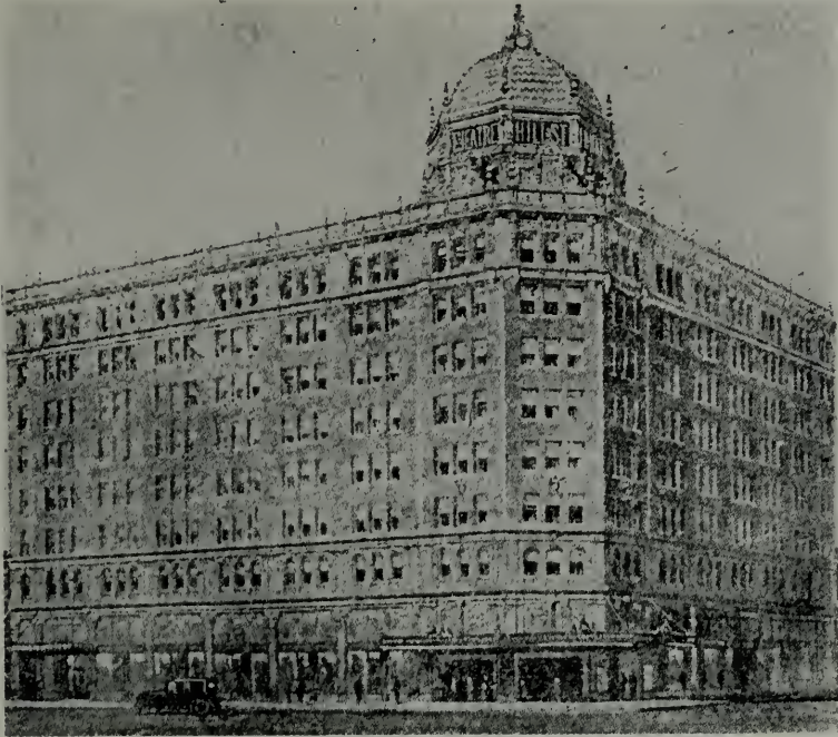
Los Angeles Junior Orpheum Theater, now under construction at Eighth and Hill Streets, Los Angeles, Macdonald & Kahn, General Contractors, G. Albert Lansburgh, Architect
