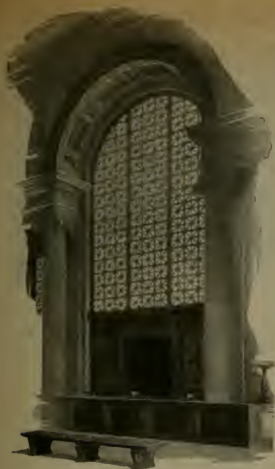
Detail of Carnegie Library, San Francisco, with Armco Ingot Iron window grill.
