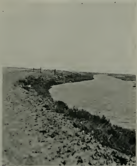
DRAINAGE DITCH INSIDE THE LEVEE, OLIVER SALT WORKS
