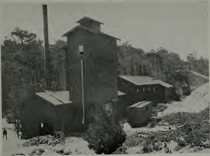
PLANT AT LAKE MAJELLA
