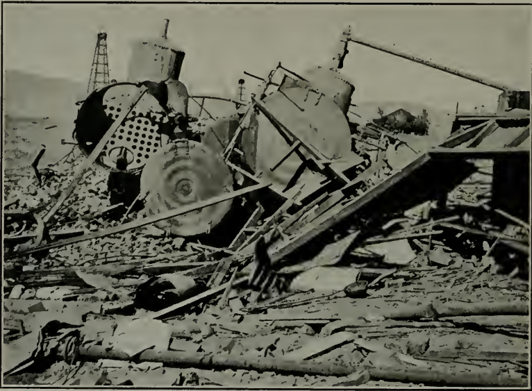
FIG. 1—VIEW OF NUMBER 2 AND NUMBER 3 BOILERS
