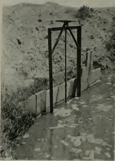
24-INCH CAST IRON SLIDE GATE, OLIVER SALT WORKS
