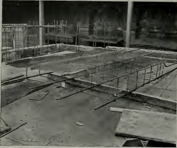
EXPANDED METAL LATH FASTENED TO REIN- FORCING STEEL READY FOR PLACING.
