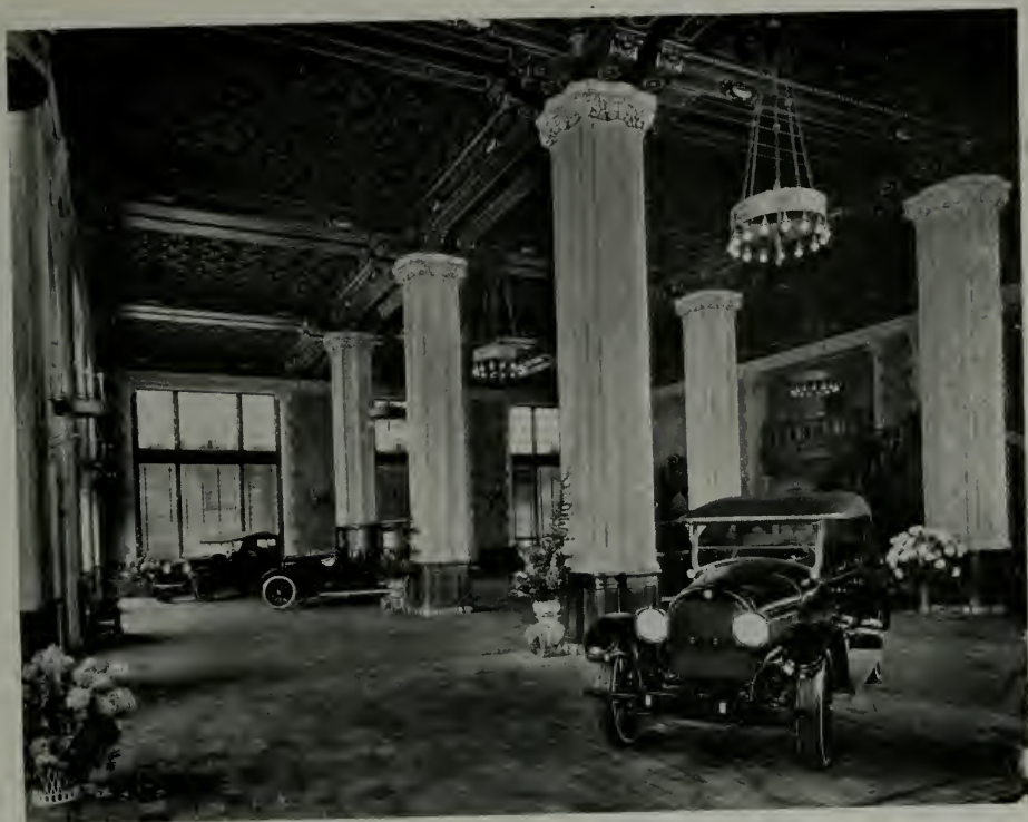
SHOW ROOM, DON LEE BUILDING, SAN FRANCISCO Weeks & Day, Architects
