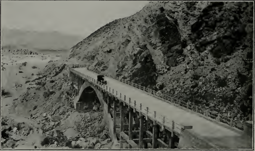
BRIDGE ON CALIFORNIA STATE HIGHWAY, IMPERIAL COUNTY, OVER MYERS CREEK
