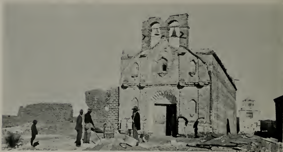
FACADE, SAN ANTONIO DE OQUITOA
