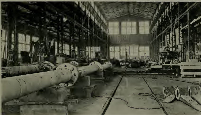
INTERIOR VIEW OF MACHINE SHOP, UNION CONSTRUCTION COMPANY, OAKLAND
