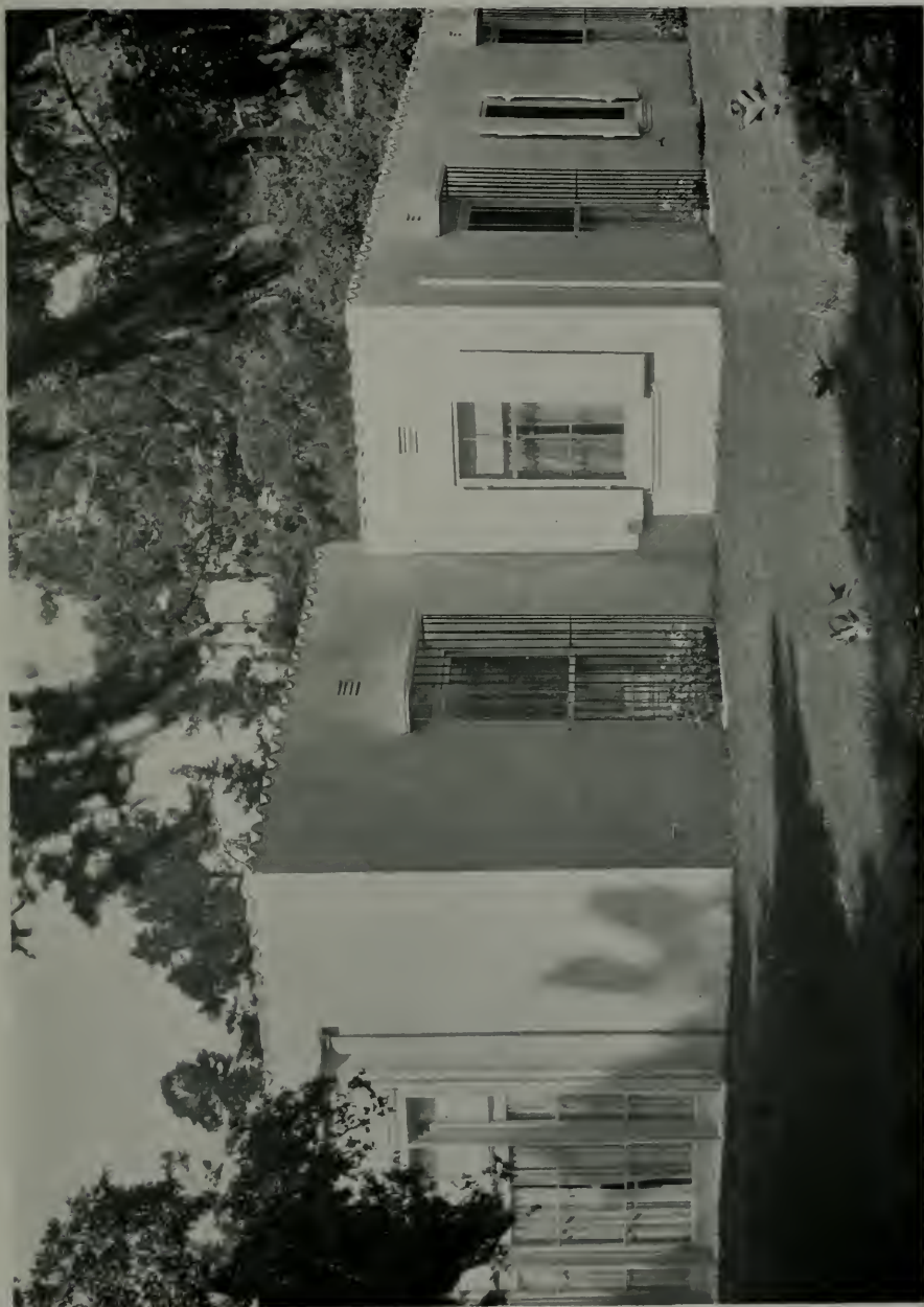
HOUSE FOR MR. JOHN S. CRAVENS, PEBBLE BEACH, CAL. LEWIS P. HOBART, ARCHITECT
