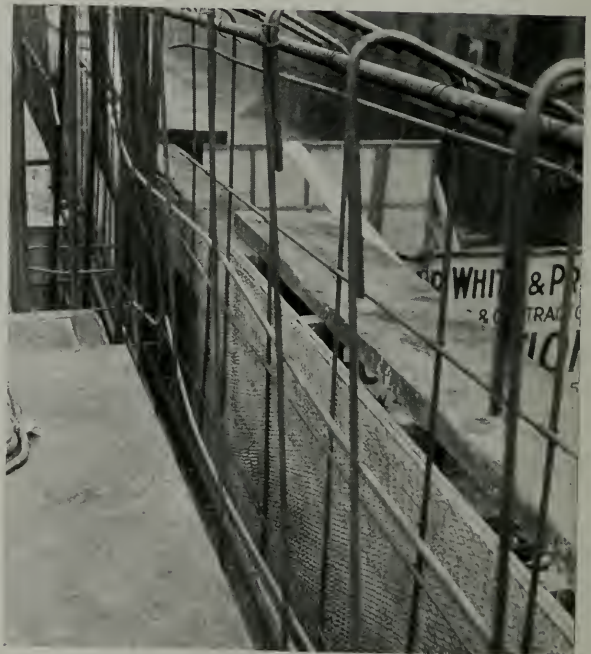
EXPANDED METAL LATH USED AS "FORM" FOR SPECIAL SUR- FACING CONCRETE.
