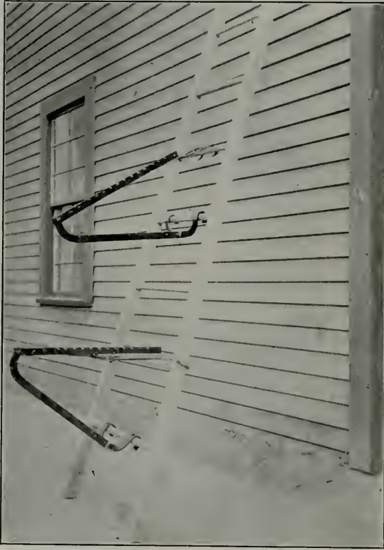
FIG. 1—CHICAGO AND LOS ANGELES LADDER BRACKETS
