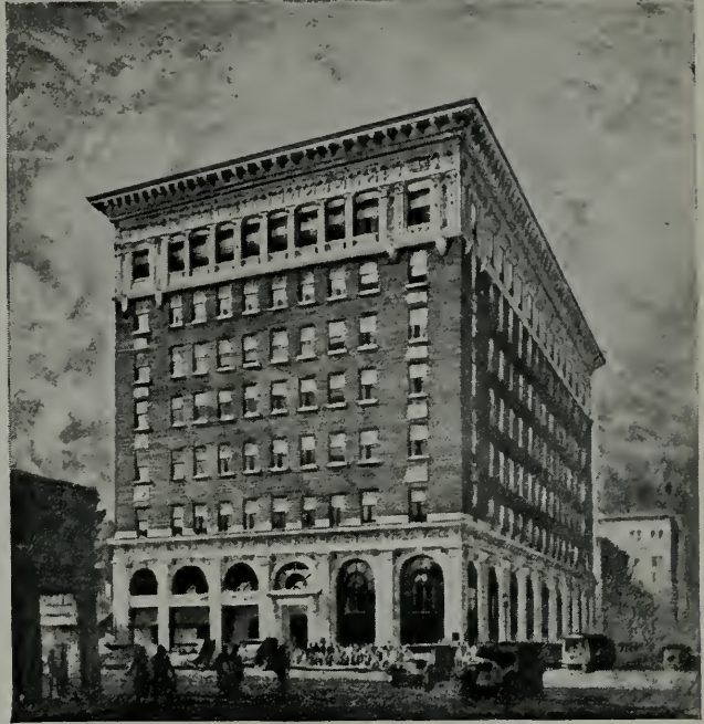
Copyright 1921 by National Terra Cotta Society Drawing by Hugh Ferriss TWO REPUBLICS LIFE INSURANCE BUILDING EL PASO, TEXAS Ivory Matt glazed Terra Cotta TROST AND TROST, Architects
