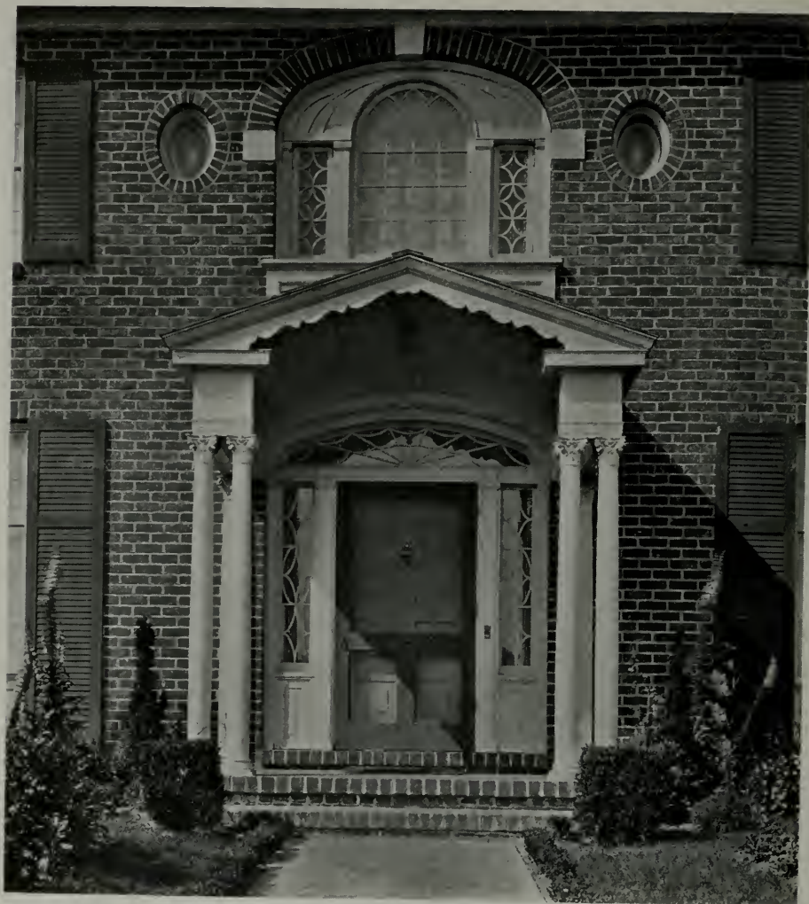
ENTRANCE, HOUSE FOR MR. FRANK KALES, ALAMEDA, CAL. Sidney B. & Noble Newsom, Architects
