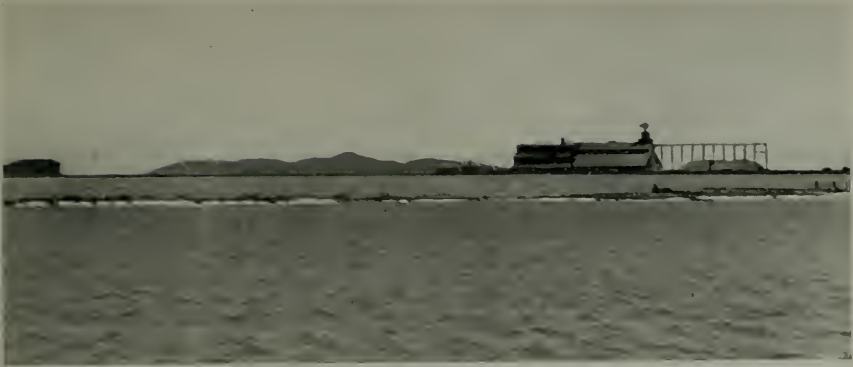
GENERAL VIEW OF OLIVER SALT POND (Note the salt line on the small dykes)
