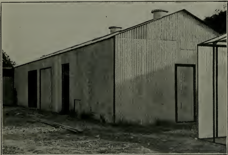
WAREHOUSE, SAN JOSE, STEEL FRAME AND CORRUGATED IRON SIDES
