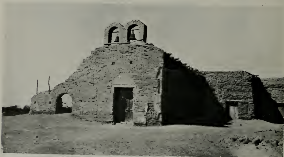
FACADE, SAN FRANCISCO DE ATIL
