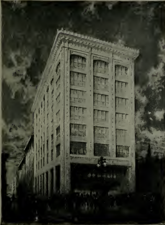
Copyright, 1921, by National Terra Cotta Society Drawing by Hugh Ferriss Sales and Service Building PACKARD MOTOR CAR CO. OF PHILADELPHIA Cream matt glazed Terra Cotta ALBERT KAHN, Architect
