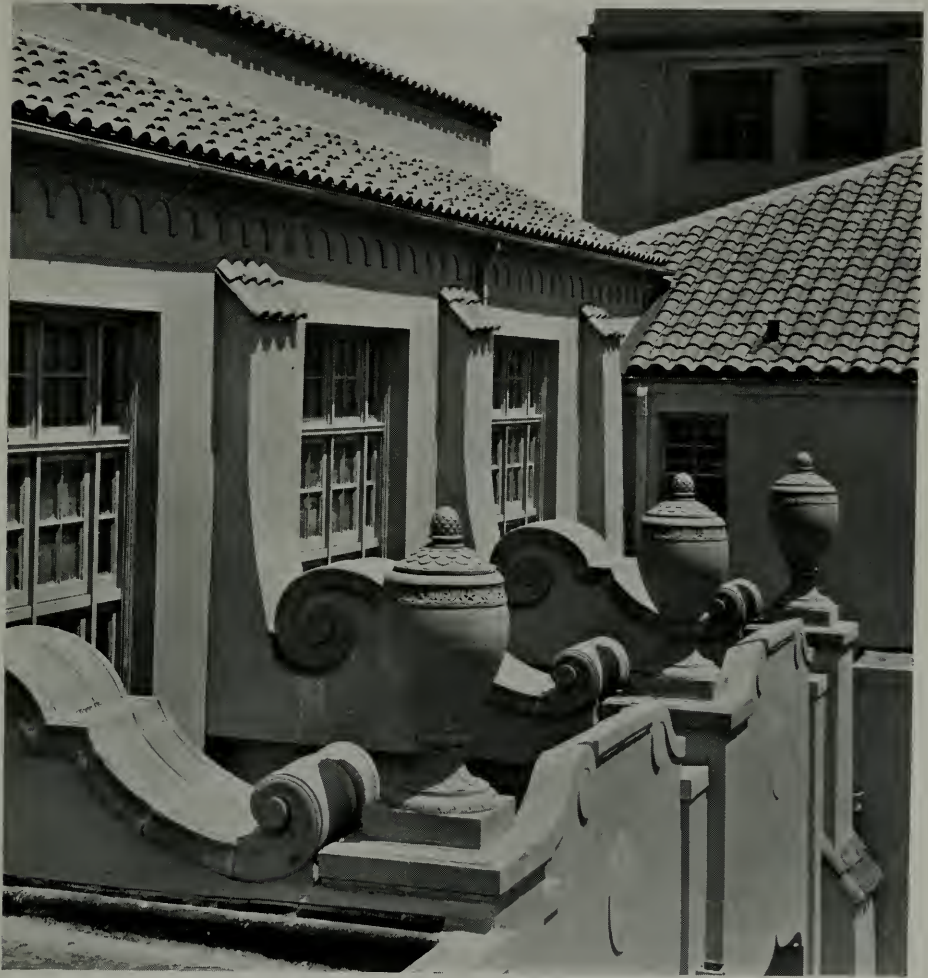
AUDITORIUM CLERESTORY, SALINAS UNION HIGH SCHOOL, SALINAS, CAL. Ralph Wyckoff, Architect
