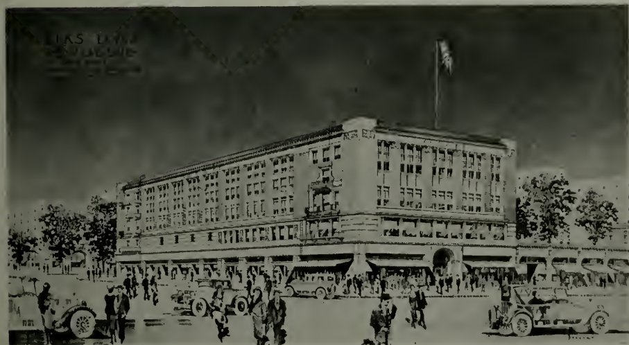
ELKS LODGE BUILDING, SANTA MONICA, CALIFORNIA
