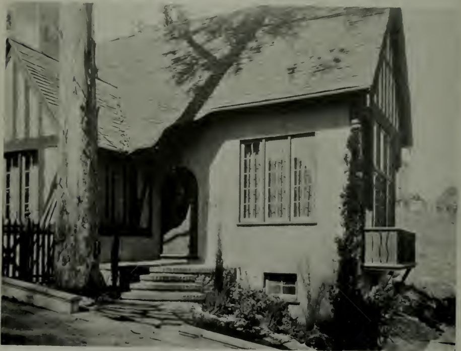
HOUSE OF W. R. DAVENPORT, SAN FRANCISCO Masten and Hurd, Architects
