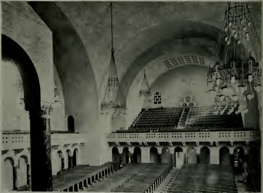
INTERIOR, CONGREGATION EMANU-EL TEMPLE, SAN FRANCISCO S. Schnaittacher and Bakewell & Brown, Architects
