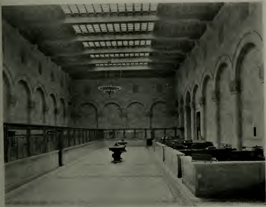
MAIN BANKING ROOM, CENTRAL BANK, OAKLAND George William Kelham, Architect
