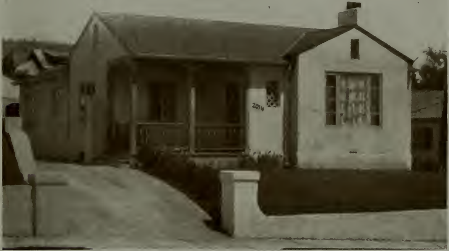
HOUSE OF MR. R. M. CULLER, SANTA BARBARA, CALIFORNIA Soule, Murphy & Hastings, Architects
