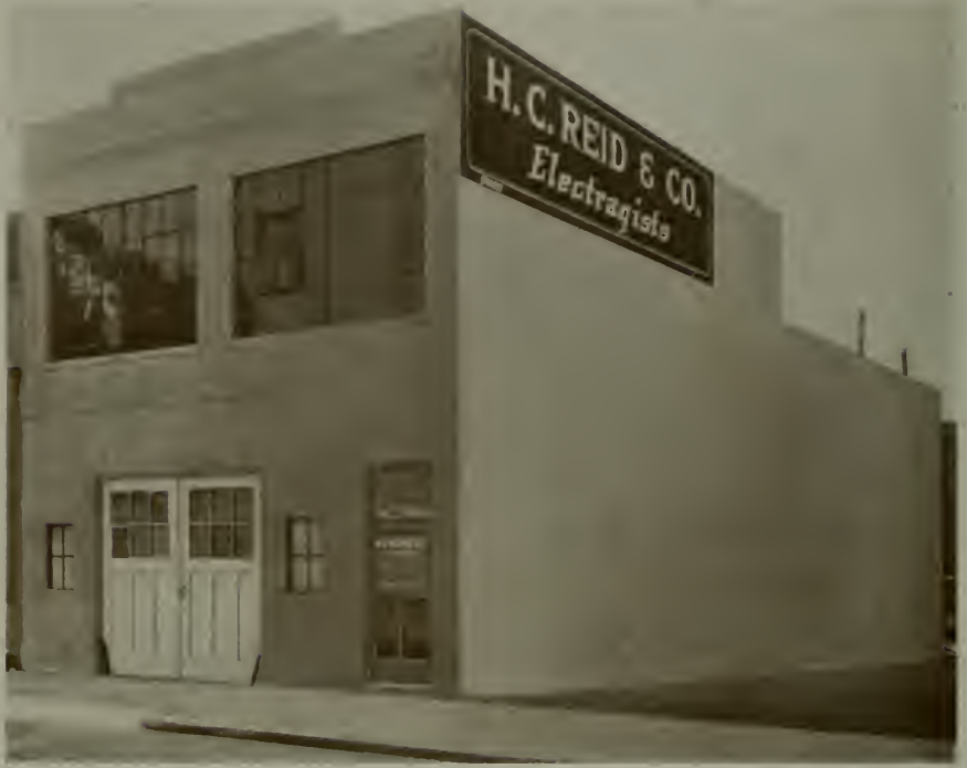
NEW HOME OF H. C. REID & CO., SAN FRANCISCO Earl Markwart, Engineer
