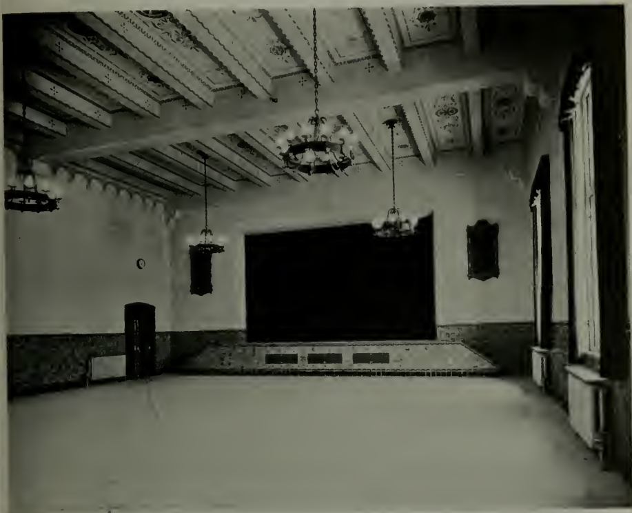
AUDITORIUM, DUDLEY STONE SCHOOL, SAN FRANCISCO John Reid, Jr., Architect
