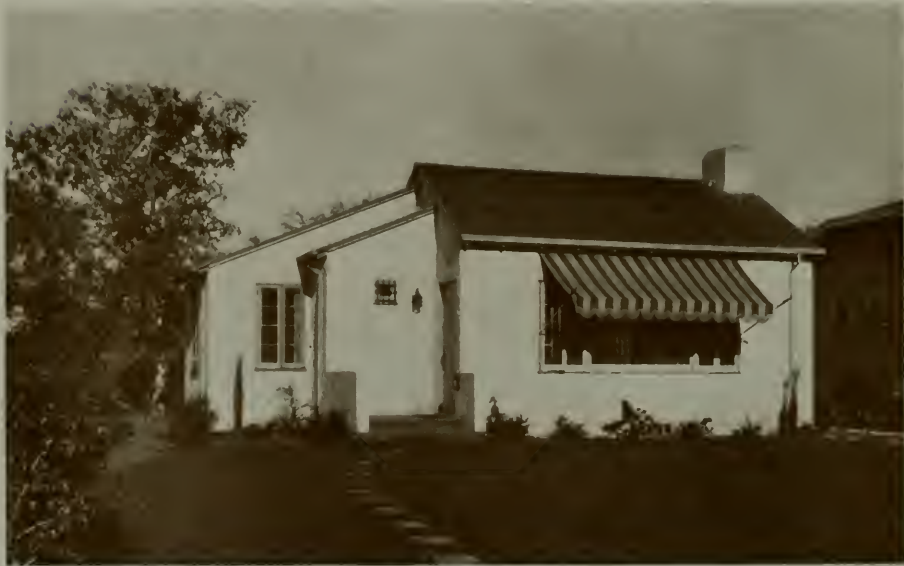
SMALL HOUSE, SANTA BARBARA E. Keith Lockard, Architect
