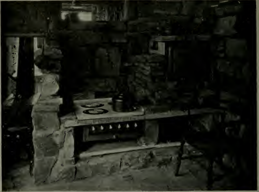
KITCHEN, HOUSE OF J. M. MENDEL, MONTEREY Frederick H. Reimers, Architect
