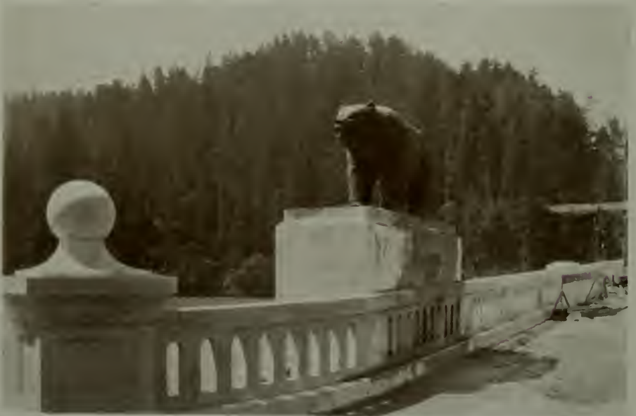
PYLONS SURMOUNTED BY GRIZZLY BEARS, KLAMATH RIVER BRIDGE
