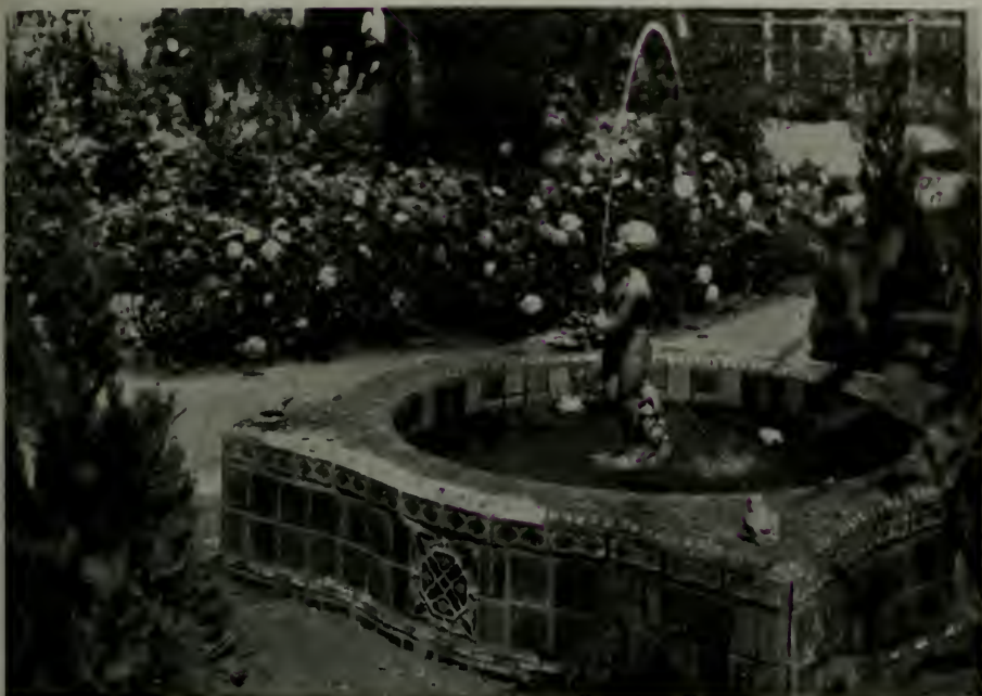
FOUNTAIN, RESIDENCE OF W. O. HORABIN, PALO ALTO Birge M. Clark, Architect
