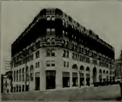
UNION AUTO EXCHANGE BUILDING LOS ANGELES, CALIF.
