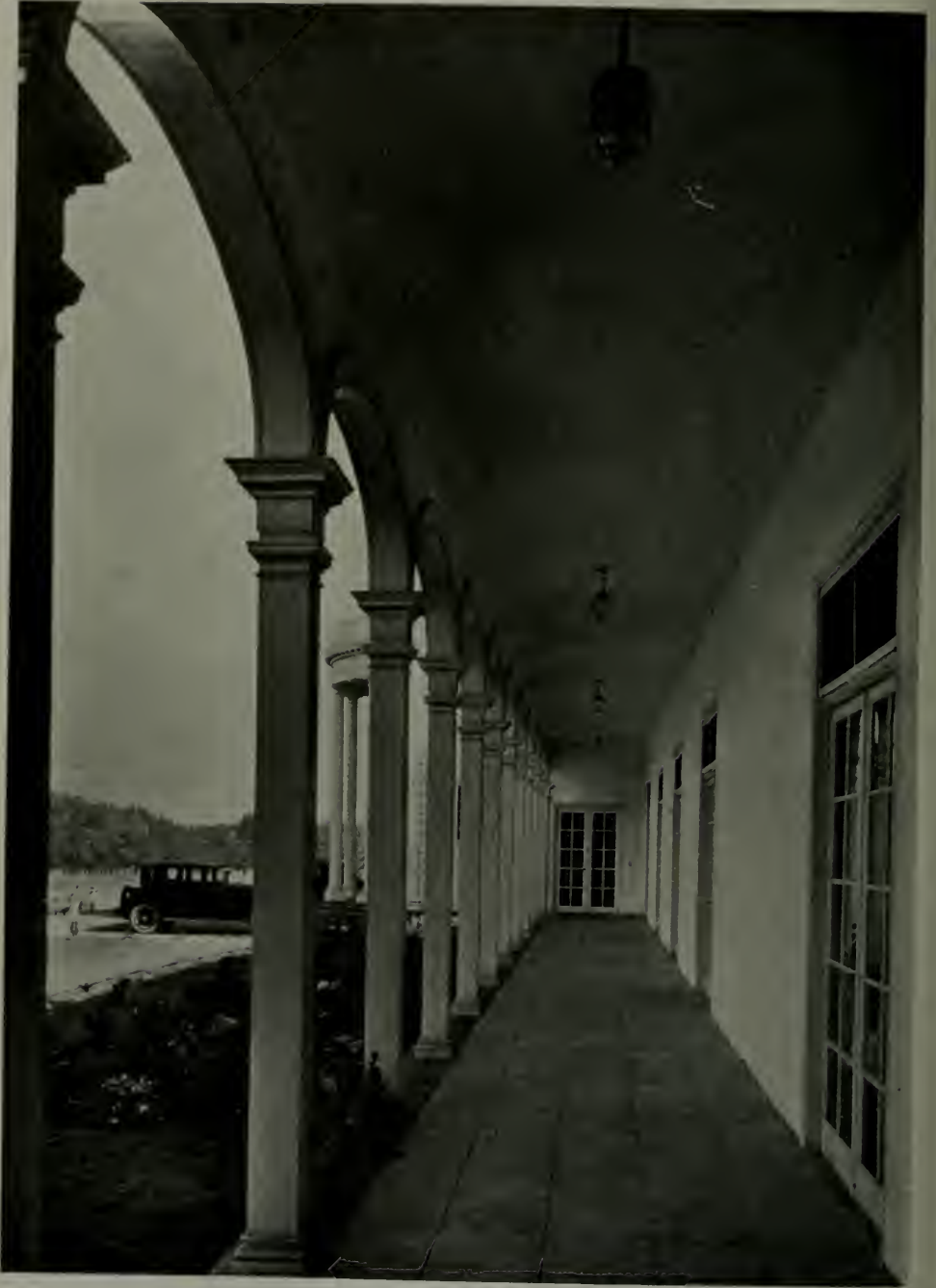
PORCH, CALIFORNIA GOLF CLUB, SAN MATEO COUNTY WILLIS POLK AND COMPANY, ARCHITECTS
