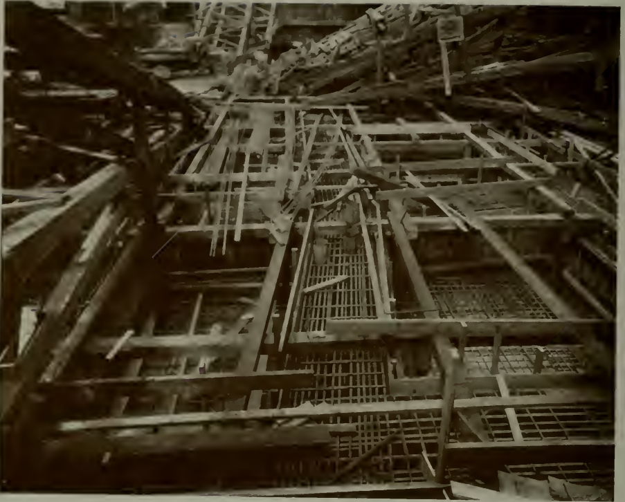
FIG. I - FOOTINGS, NORTH SIDE HUNTER-DULIN BUILDING, SAN FRANCISCO
