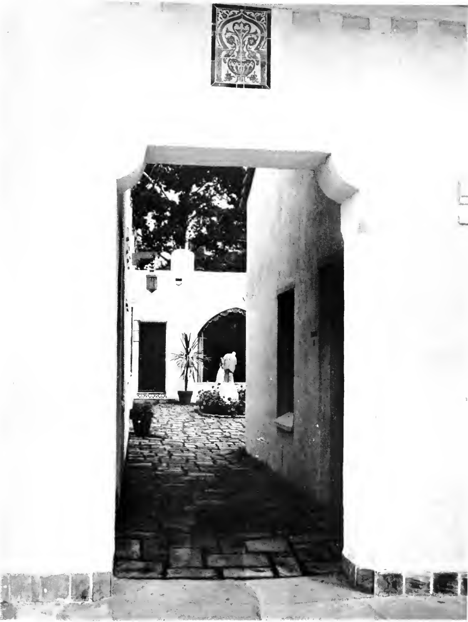
SHOPPE BUILDING FOR L. C. MERRELL, CARMEL, CALIFORNIA BLAINE AND OLSON, ARCHITECTS
