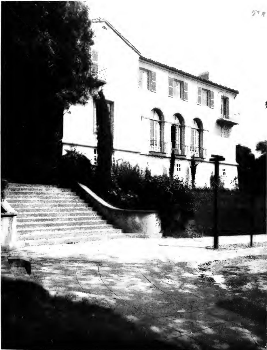
ALPHA PHI FRATERNITY HOUSE, BERKELEY, CALIFORNIA W. ALFRED H. RATCLIFF, JR., ARCHITECT
