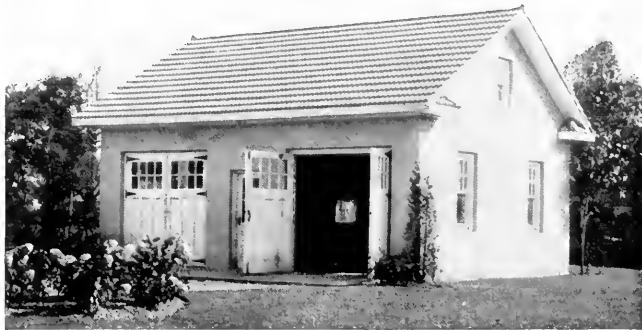
DOUBLE GARAGE OF CONCRETE BLOCKS AND ROOFING TILE
