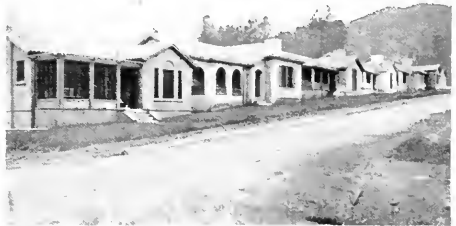
MOCCASIN POWER PLANT OPERATORS' COTTAGES Constructed of Concrete and Tile, Electrically Heated and Lighted
