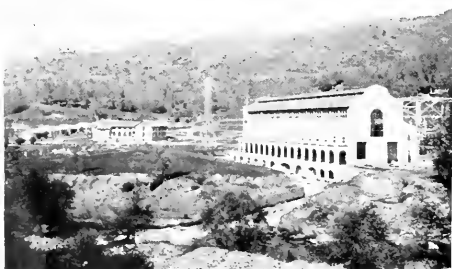
MOCCASIN POWER HOUSE, CLUB HOUSE AND COTTAGES
