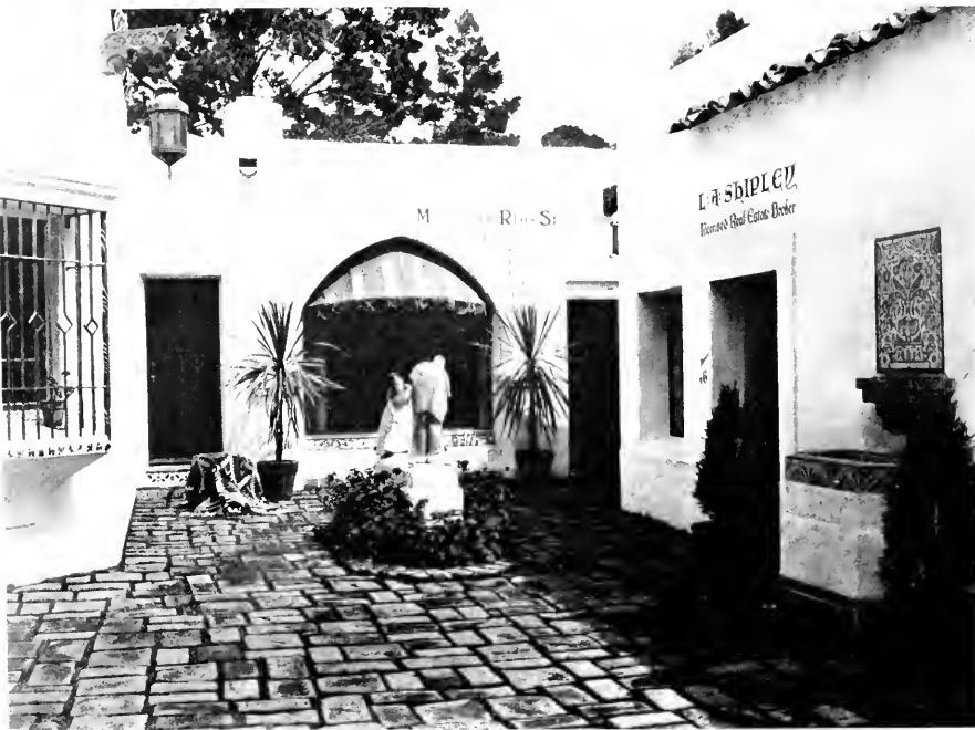
SHOPPE BUILDING FOR L. C. MERRELL, CARMEL, CALIFORNIA Blaine and Olson, Architects
