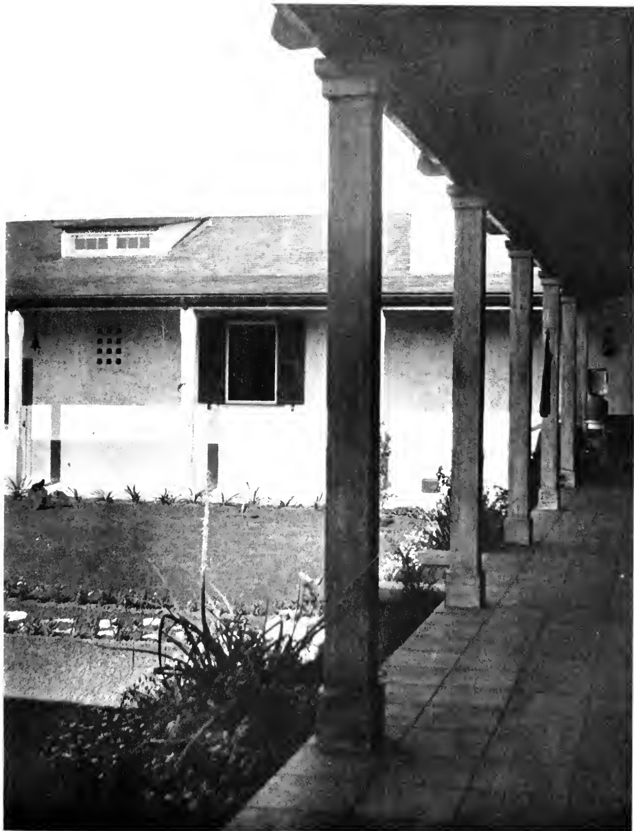
RANCH HOUSE FOR Y. R. DEL VALLE. "THE RIVIERA," CALIFORNIA JOHN BYERS, ARCHITECT
