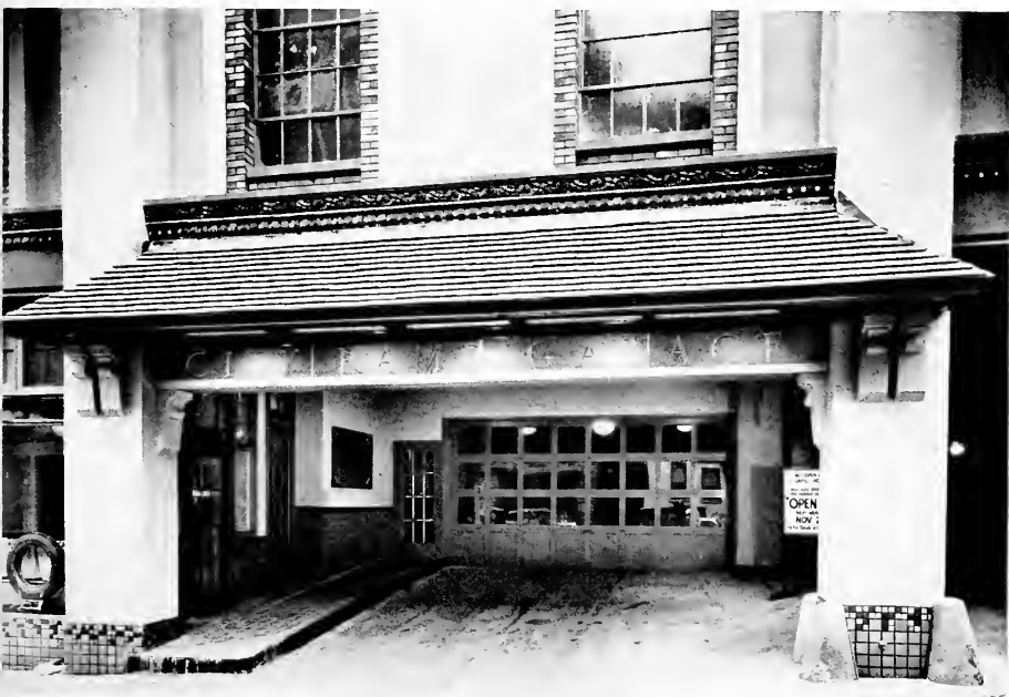
CITY RAMP GARAGE, SPOKANE, WASHINGTON Whitehouse & Price, Architects
