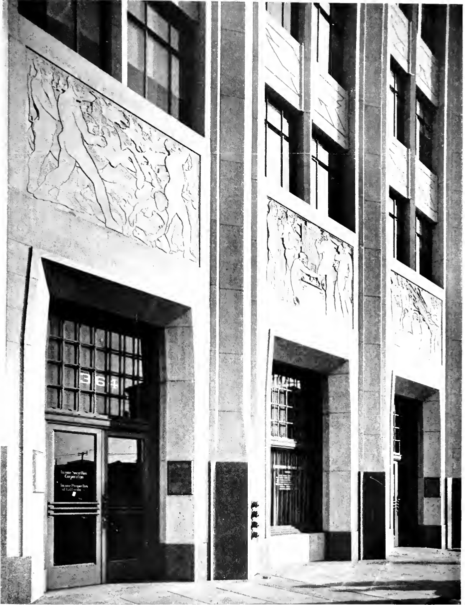
DETAIL OF LOWER STORIES, INCOME SECURITIES BUILDING, OAKLAND FREDERICK H. REIMERS, ARCHITECT
