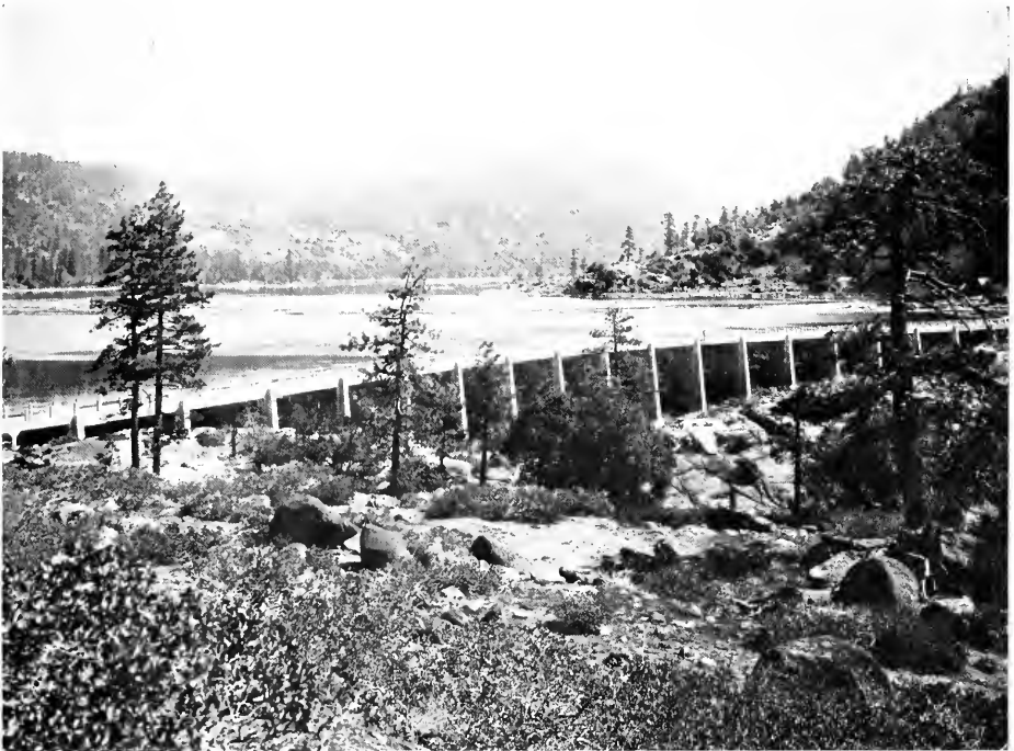
LAKE ELEANOR DAM, HETCH HETCHY PROJECT The buttressed arches are 1,260 feet long and 70 feet high
