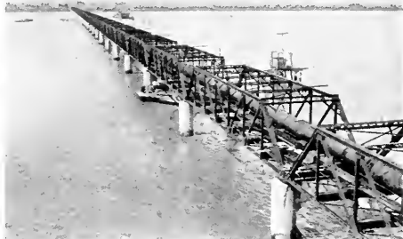
DUMBARTON PIPE BRIDGE, HETCH HETCHY AQUEDUCT
