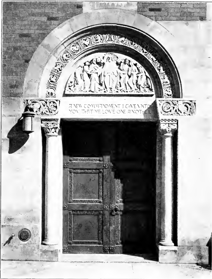
Detail side entrance, St. Bartholomew Community House, New York City. B. G. Goodhue Associates, Architects. Variegated Indiana Limestone base and trim
