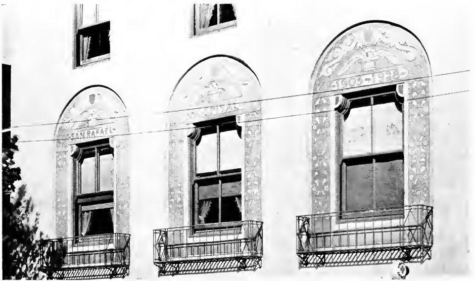
SAN RAFAEL HOSPITAL, SAN RAFAEL, CALIFORNIA Note Window Decorations in Sgraffiti
