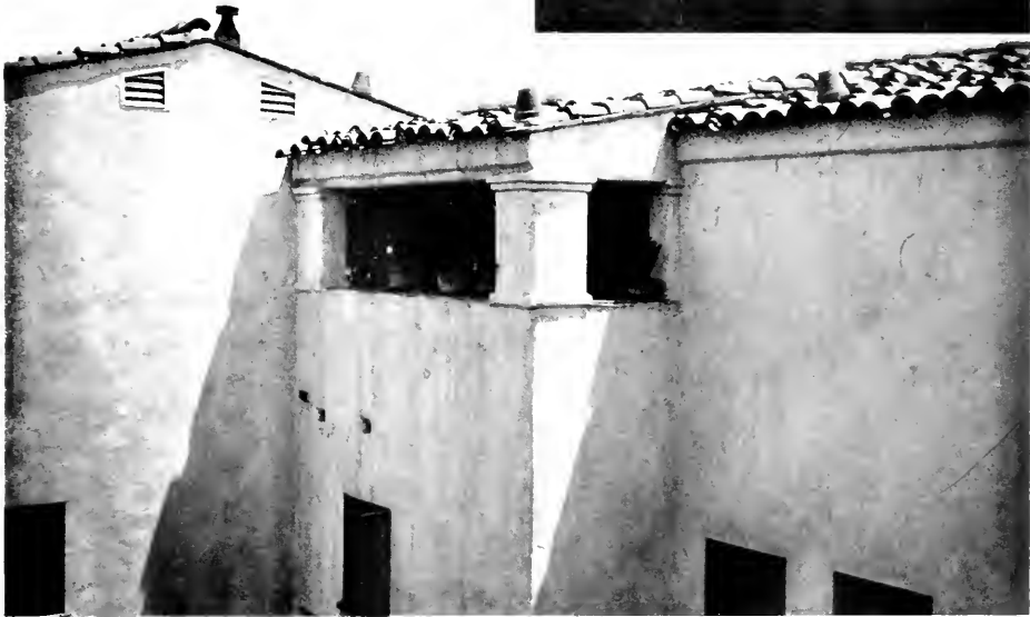
LOGGIA, HOUSE FOR DEAN B. GREGG, LOS ANGELES, CALIFORNIA
