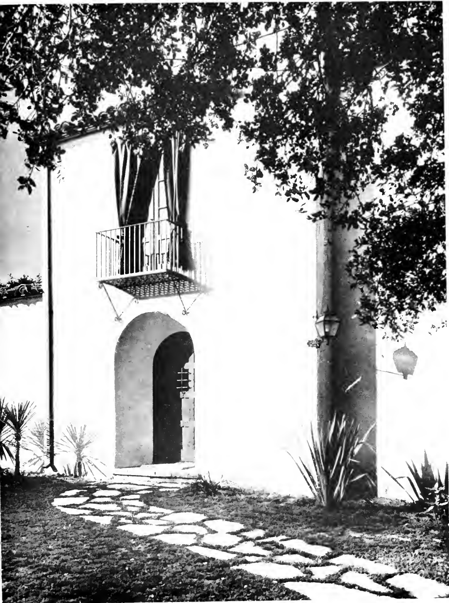
HOUSE FOR MR. W. G. GILSON, HILLSBOROUGH OAKS DODGE A. RIEDY, ARCHITECT
