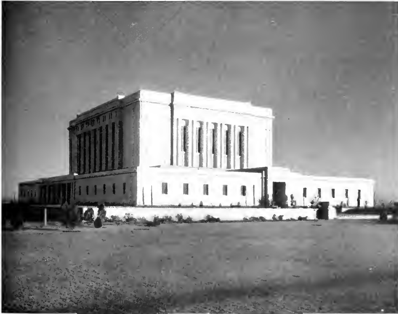
CHURCH OF JESUS CHRIST OF LATTER-DAY SAINTS, MESA, ARIZONA YOUNG & HANSEN, ARCHITECTS
