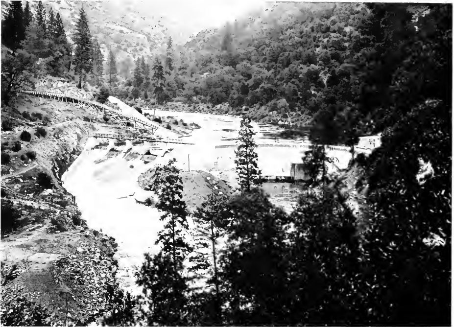
EARLY INTAKE DIVERSION DAM ON TUOLUMNE RIVER
