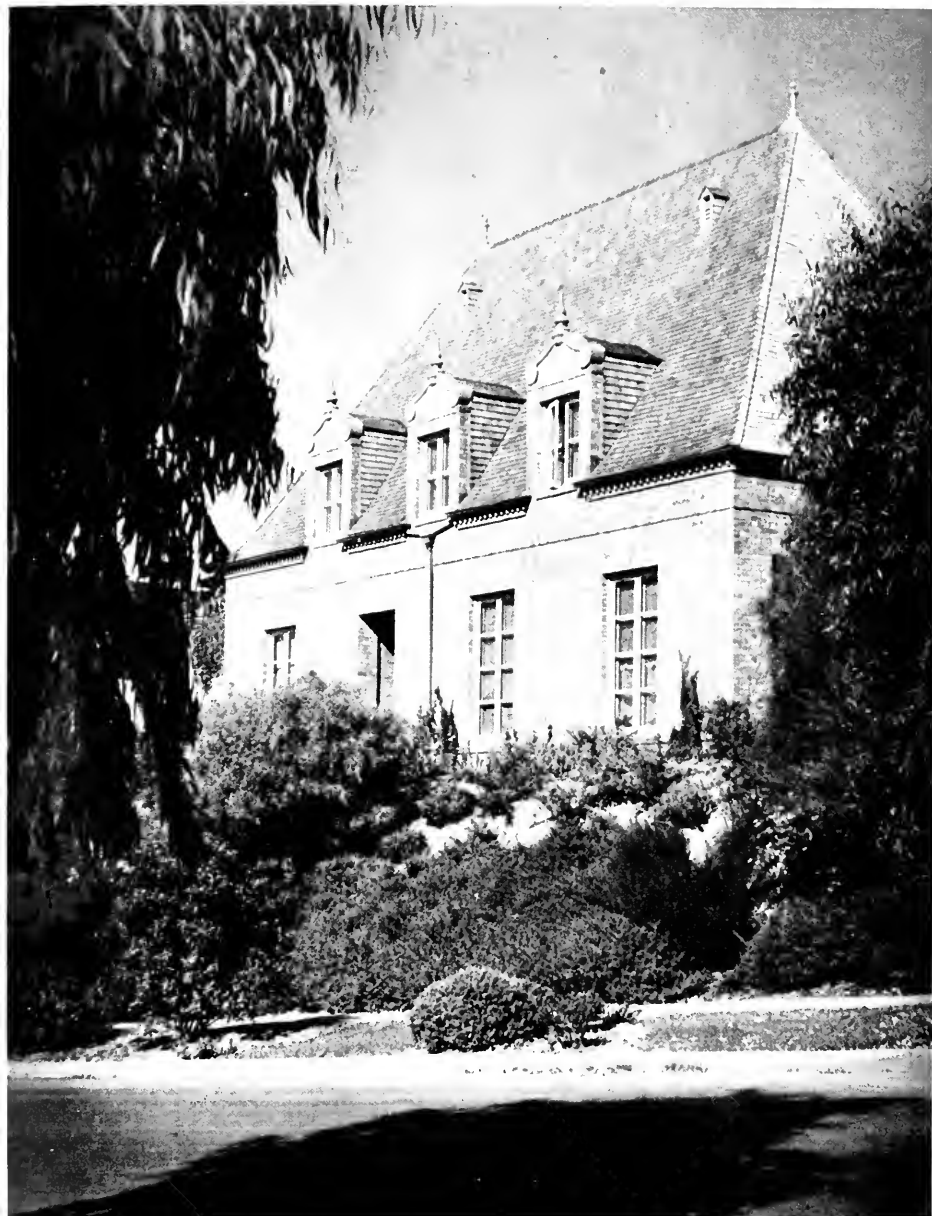
HOUSE FOR MR. A. MEYERS, ST. FRANCIS WOOD, SAN FRANCISCO WILLIAM L. GARREN, ARCHITECT
