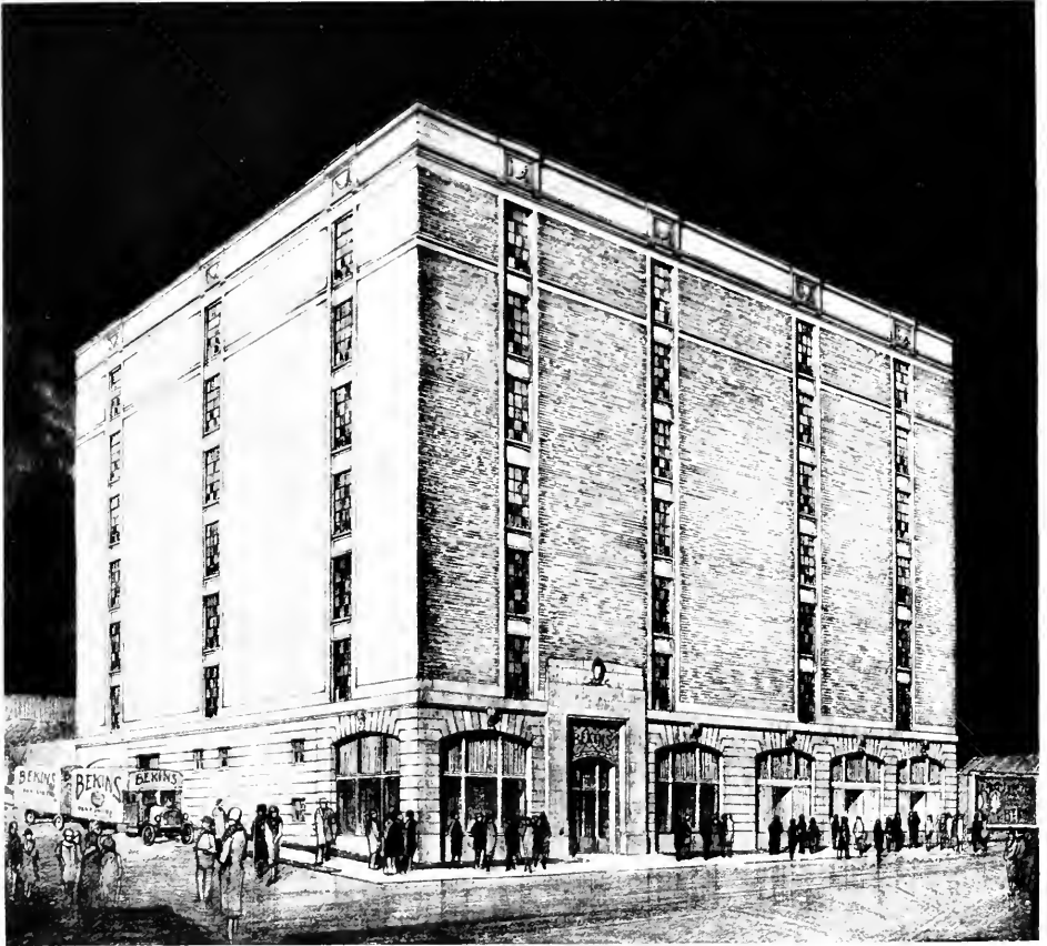
ADDITIONS TO BEKIN'S STORAGE WAREHOUSE, SAN FRANCISCO
