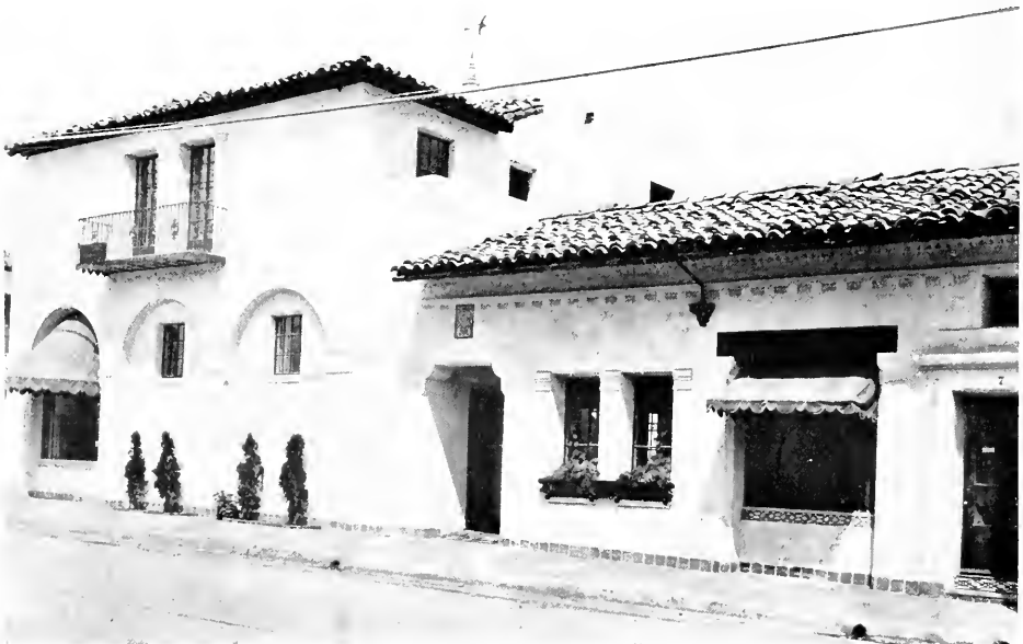
SHOPPE BUILDING FOR L. C. MERRELL, CARMEL, CALIFORNIA Blaine and Olson, Architects
