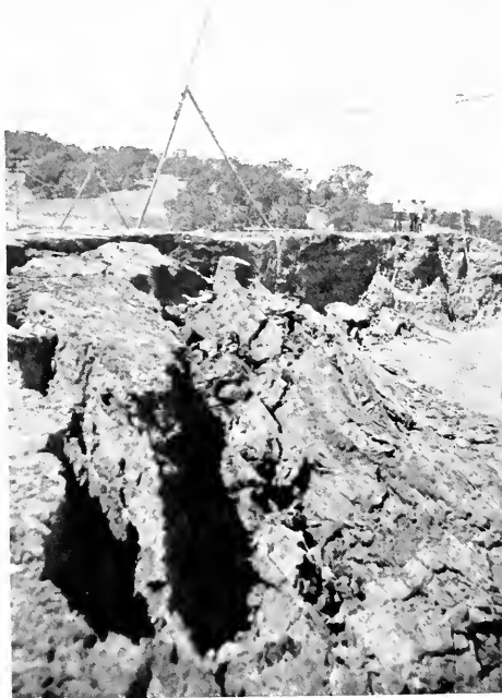
NORTH END OF BREAK NEAR CREST, LAFAYETTE DAM
