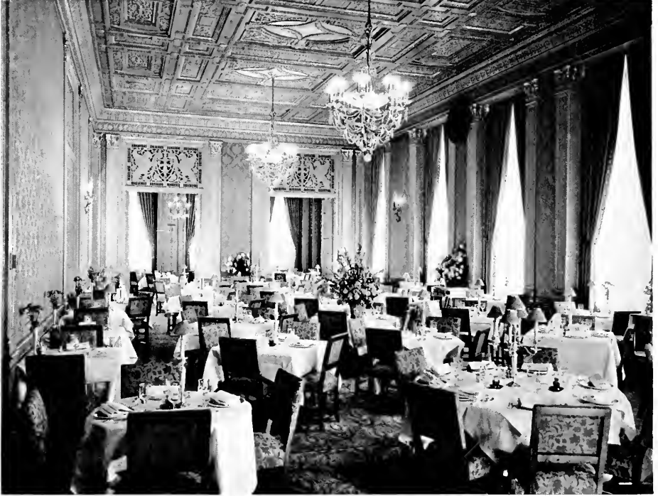
MAIN DINING ROOM, SIR FRANCIS DRAKE HOTEL, SAN FRANCISCO Weeks & Day, Architects and Engineers
