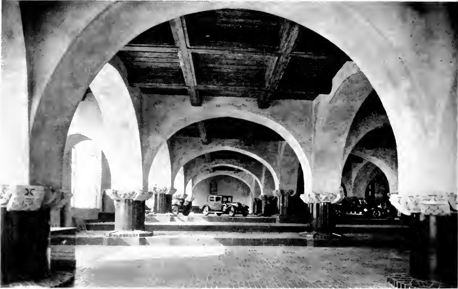
EARLE C. ANTHONY BUILDING, OAKLAND, CALIFORNIA Bernard R. Maybeck, Powers & Ahnden, Associated Architects
