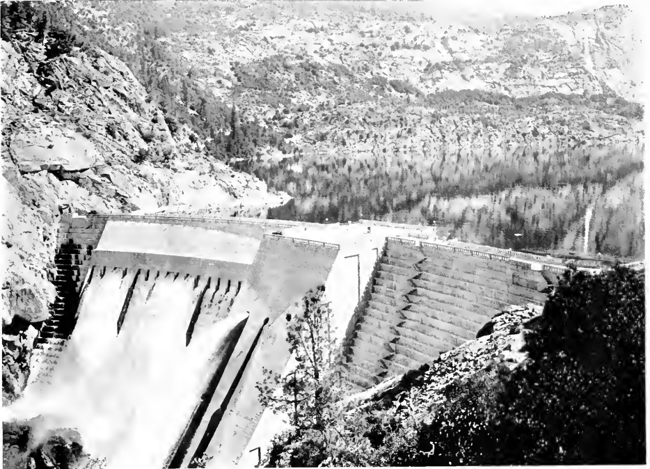
O'SHAUGHNESSY DAM AT HETCH HETCHY
