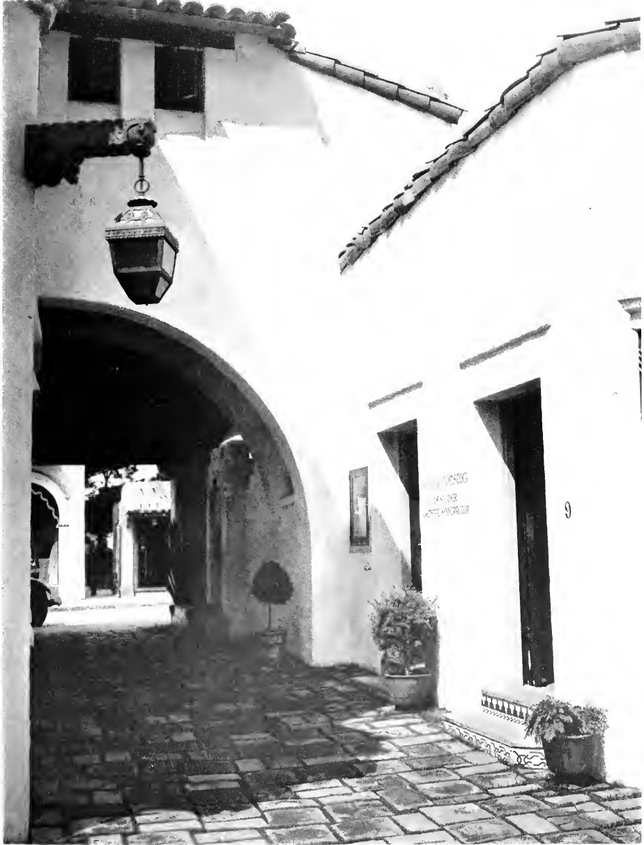
SHOPPE BUILDING FOR L. C. MERRELL, CARMEL, CALIFORNIA BLAINE AND OLSON, ARCHITECTS
