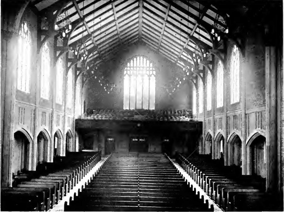
LOOKING TOWARD ENTRANCE, FIRST M. E. CHURCH, BERKELEY George Rushforth, Architect
