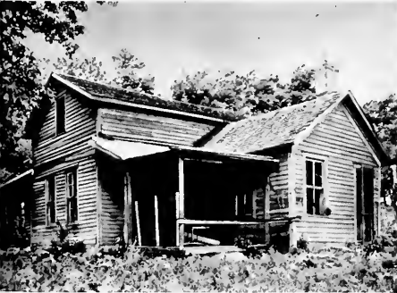
DILAPIDATED FARM HOUSE BEFORE ARCHITECTURAL TREATMENT
