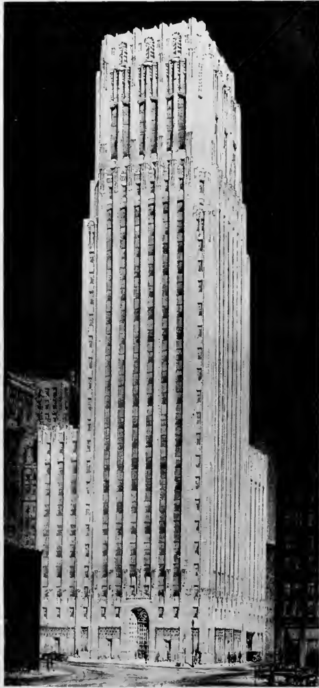
SHELL OIL BUILDING, SAN FRANCISCO GEORGE W. KELHAM, ARCHITECT
