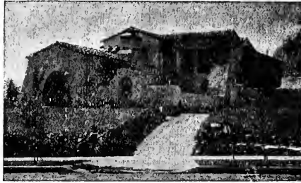
10415 Lynbrook Drive, Westwood. National Thrift Co., Gen. Contractor & Builder. Irving Black, Architect. C. W. Darling, Plastering Contractor.
