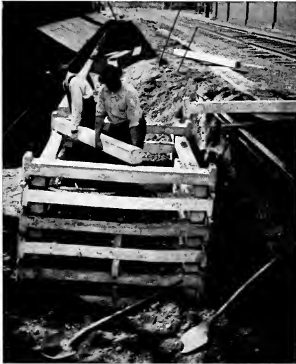
NO TOOLS REQUIRED BY THESE WORKMEN IN CRIB CONSTRUCTION
