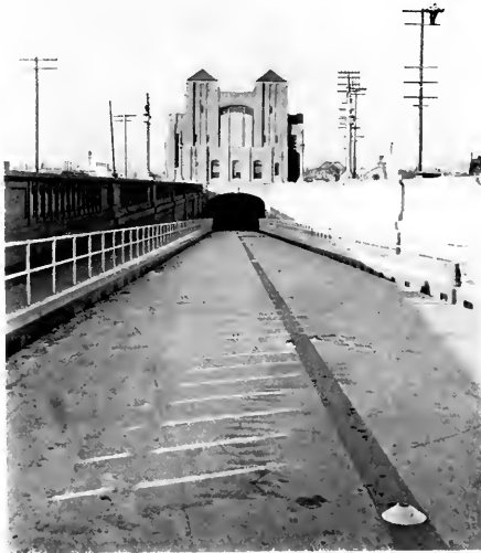
ALAMEDA APPROACH TO TUBE AND VENTILATION EQUIPMENT BUILDING AT PORTAL
