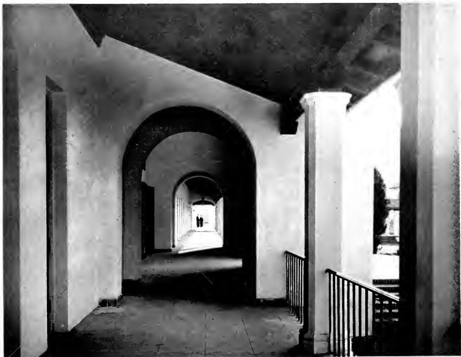
ARCADE, ST. MARY'S COLLEGE, CALIFORNIA John J. Donovan, Architect
