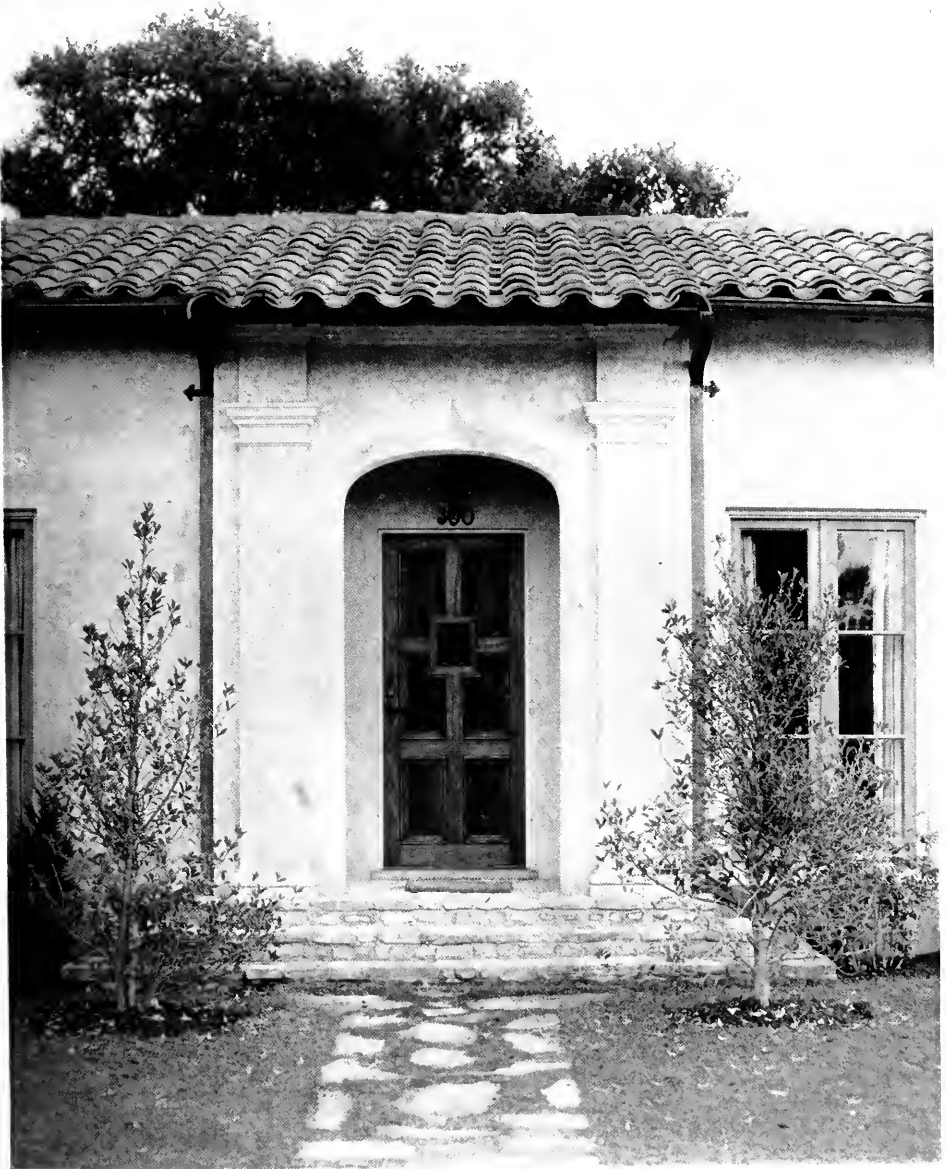
DETAIL, HOUSE OF MRS. F. W. HUNT, PALO ALTO, CALIFORNIA JOHN K. BRANNER, ARCHITECT
