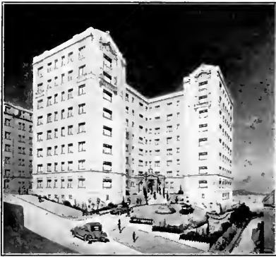
TOWNHOUSE APARTMENTS, LOS ANGELES Weir Electric Heaters Used Throughout
