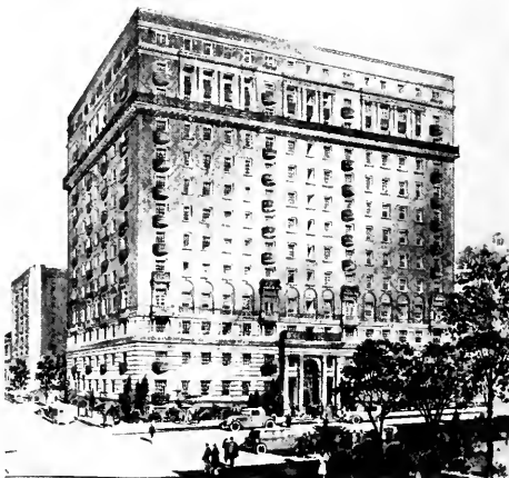
TOWNHOUSE APARTMENTS, LOS ANGELES
