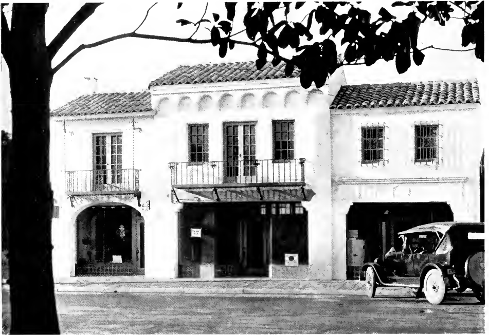
WAVERLY STREET SHOP BUILDING, PALO ALTO Birge N. Clark, Architect
