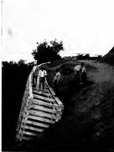
PICTURE SHOWS GENERAL CONSTRUCTION VIEW BEING BACK-FILLED
