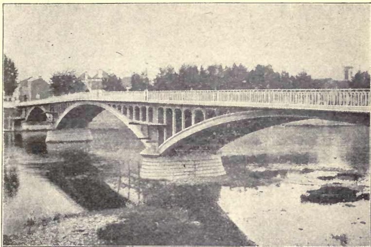
Fig. 151.—Bridge at Chatellerault, 26 feet by 450 feet long, central arch of 450 ft. span, side arches 135 ft. span, rise 1-10 of the span.
