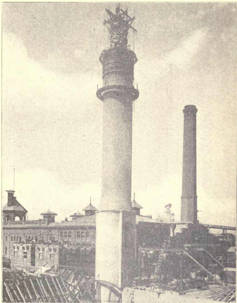
Fig. 132.—Reinforced Concrete Chimney, in course of erection, Los Angeles.
