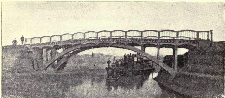
Fig. 158.—Arched Bridge of 60 ft. span. Ribs support by means of spandrel columns, the reinforced concrete roadway; railings consist of reinforced concrete posts and arches.
