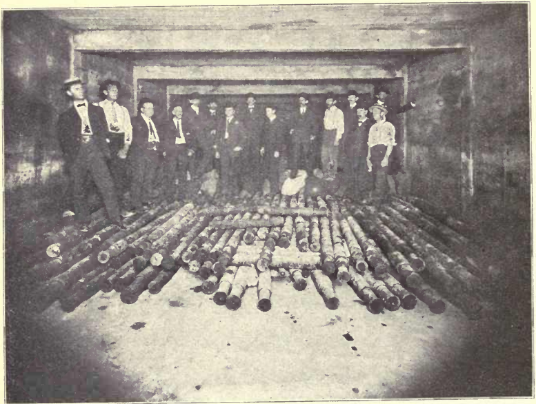
Fig. 18.—Test of Girders and Floor. Champion Ice Co.'s Cold Storage House, Covington, Ky. Load, 150,000 pounds; 600 pounds per square foot.
