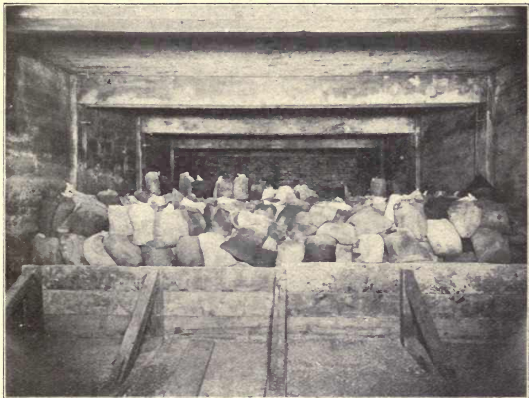
Fig. 17.—Test of Girders and Floor. Champion Ice Co.'s Cold Storage House, Covington, Ky. Load, 150,000 pounds; 400 pounds per square foot.
