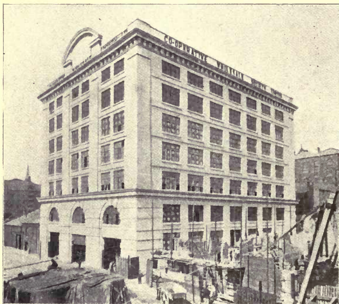
Fig. 53.—Ware-house, New Castle-on-Tyne, with Floor Loads of 800 pounds per square foot.
