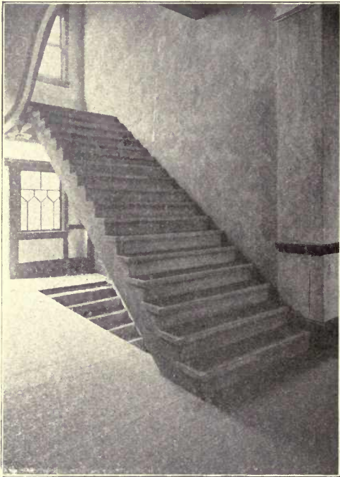
Fig. 71.—Staircase, Salvation Army Building, Cleveland, O.
