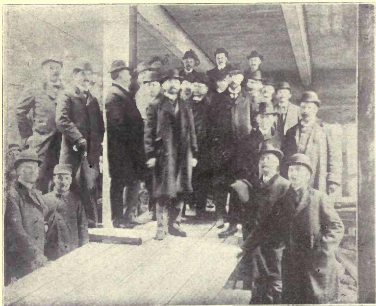
Fig. 7.—Test of Girder, Salvation Army Building, Cleveland, O.
