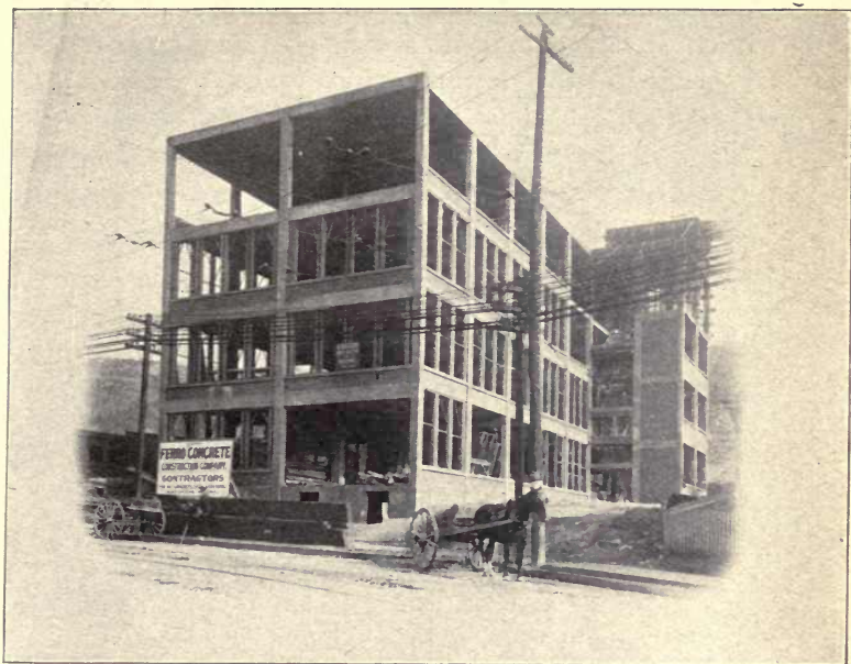
Fig. 76.—MacDonald & Kiley's Shoe Factory, Cincinnati, O. Reinforced concrete skeleton construction. 8 inch brick fillings.
