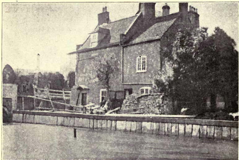
Fig. 57—Sheet Piles, retaining bank 6
