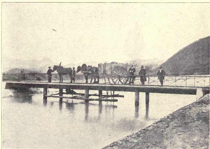
Fig. 148.—Continuous Girder, Bridge on Concrete Pier Foundation.
