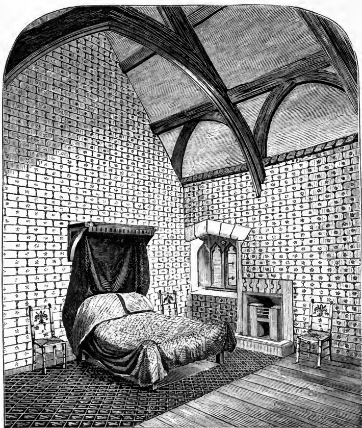
Upper Room in one of the Vicars' Houses in the Close, c. 1360.
