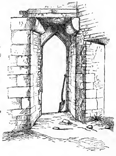
Doorway in a Vicar's House, A.D. 1360.
