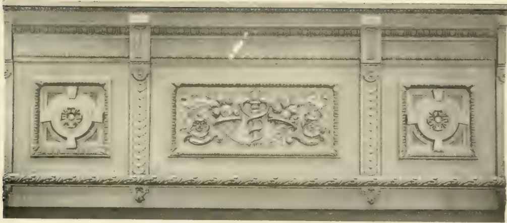
Cast Iron Window Spandril
