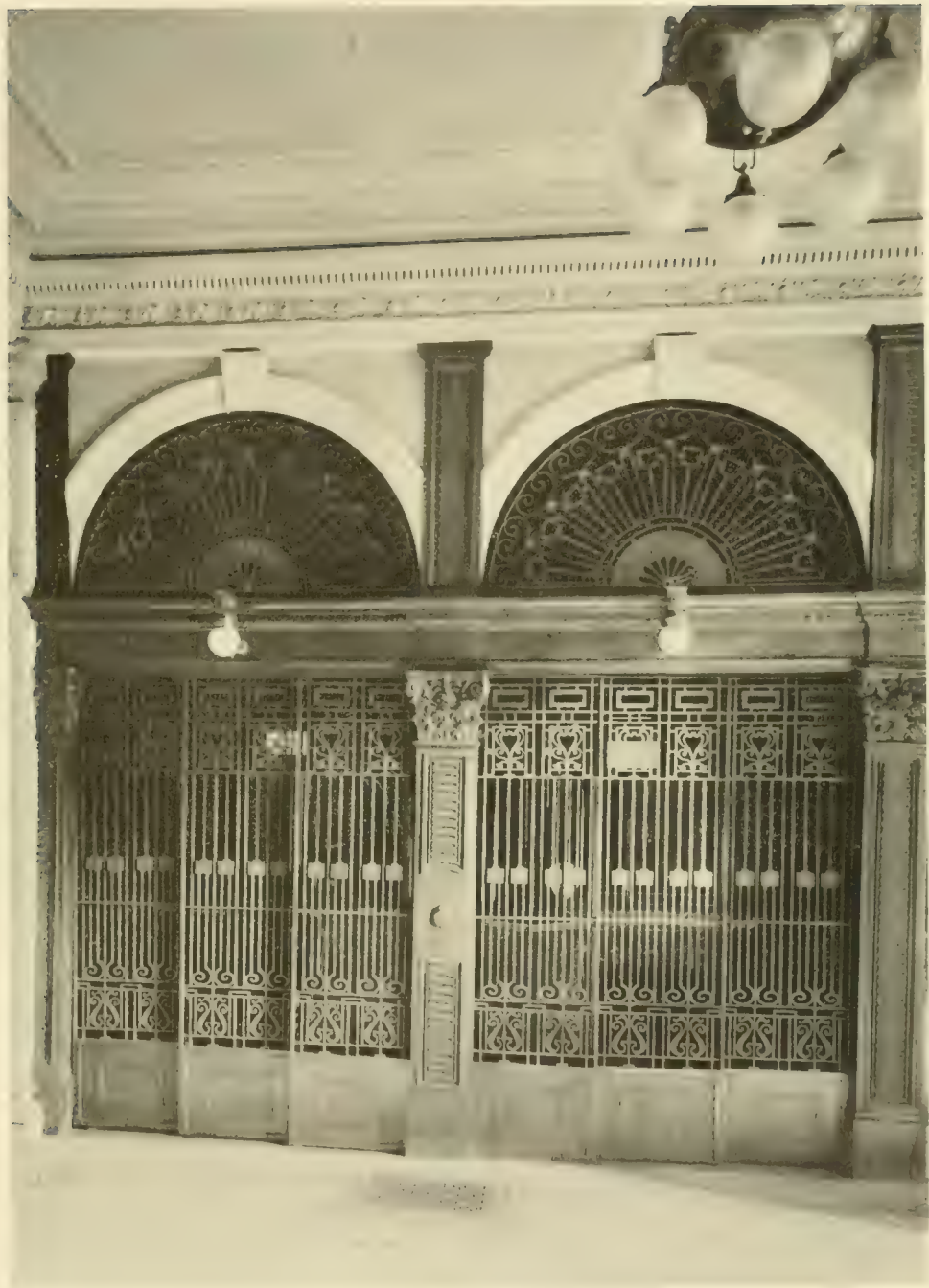
Cast and Wrought Iron Elevator Enclosures
