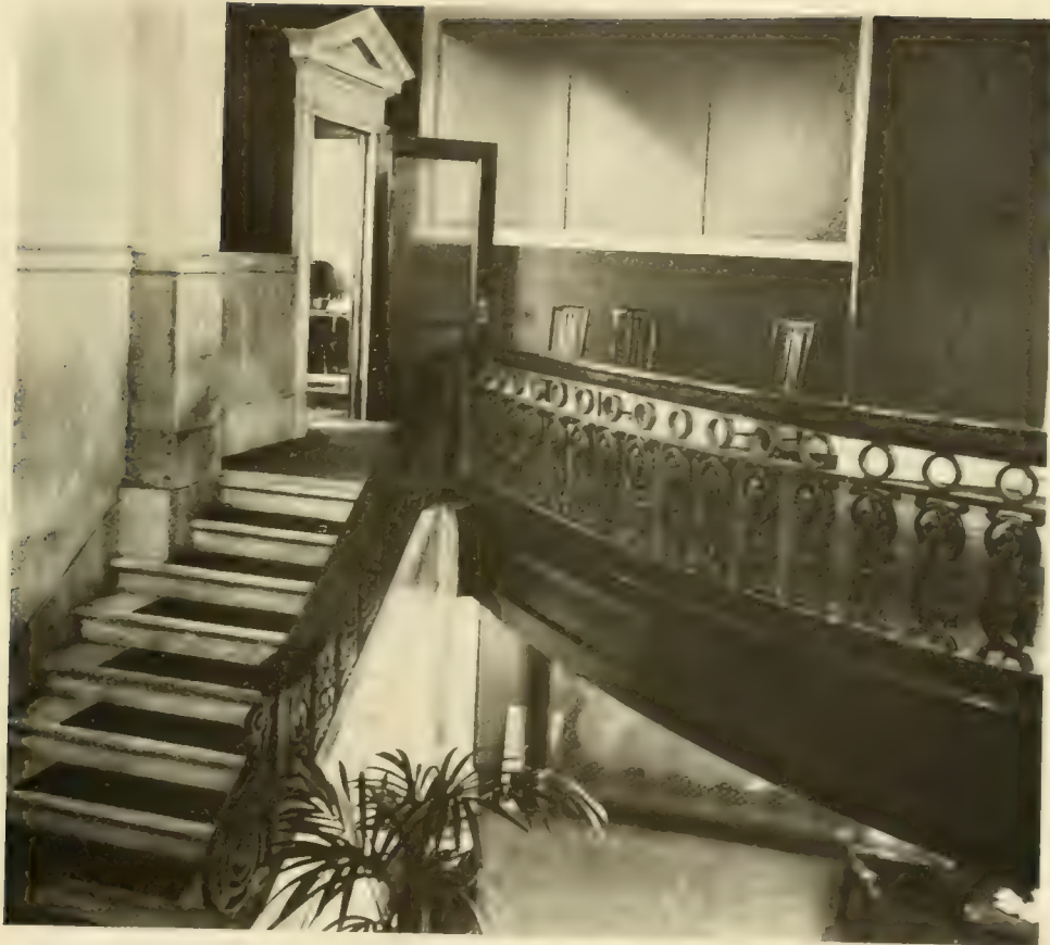
Cast Iron Railing and Stairs
