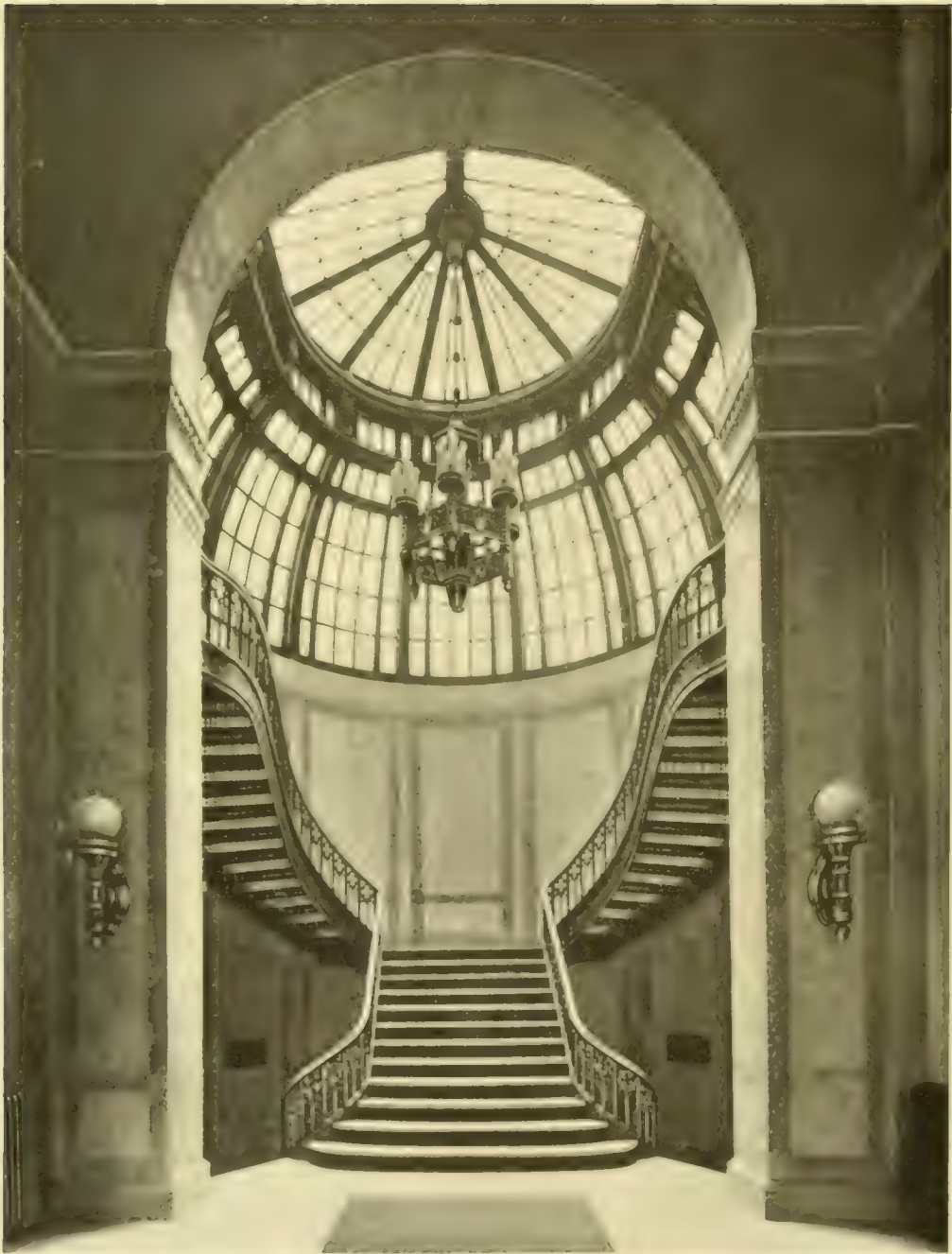
Cast Iron Stairs and Dome
