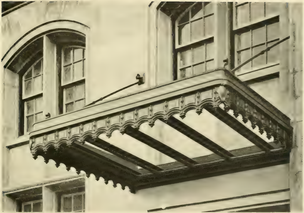
Cast Iron Marquise
