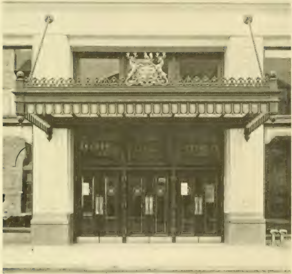
Cast Iron Marquise and Entrance
