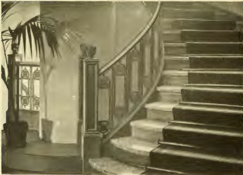
Cast Iron Stair Railing
