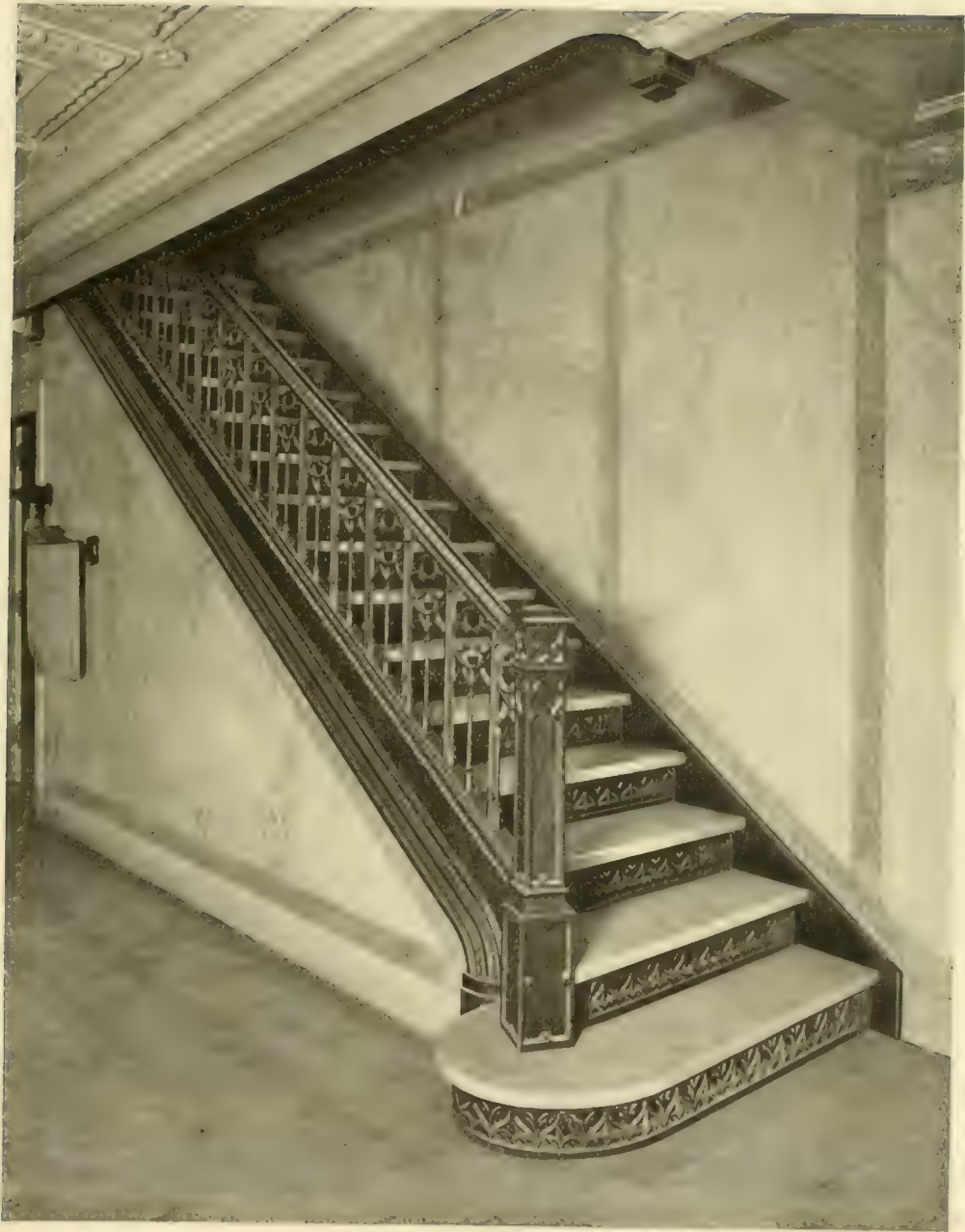
Cast Iron Stairs
