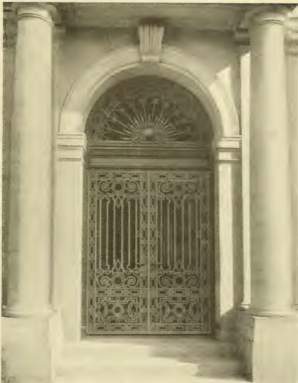
Cast and Wrought Iron Entrance
