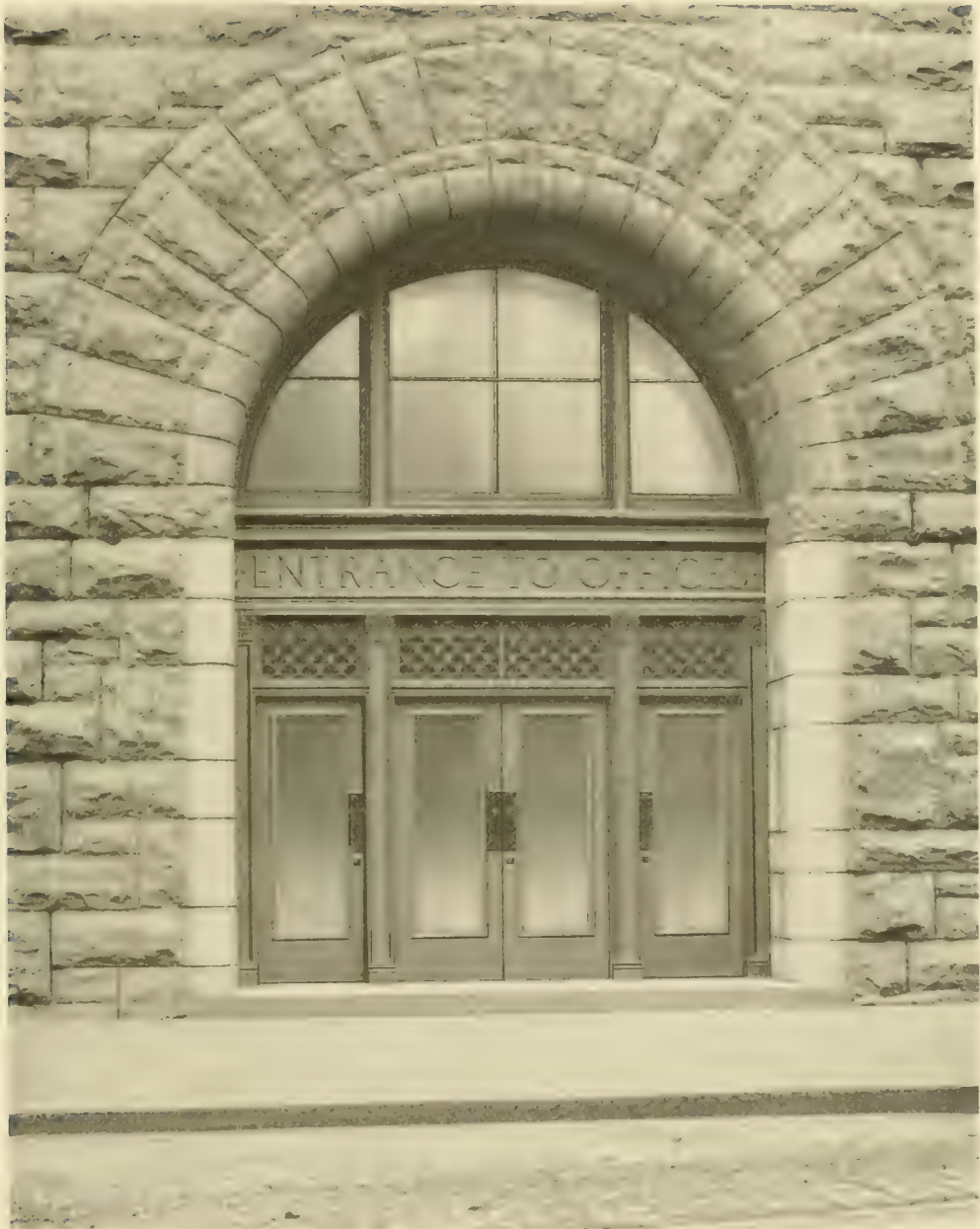
Cast Iron Office Entrance (Hollow Steel Doors)
