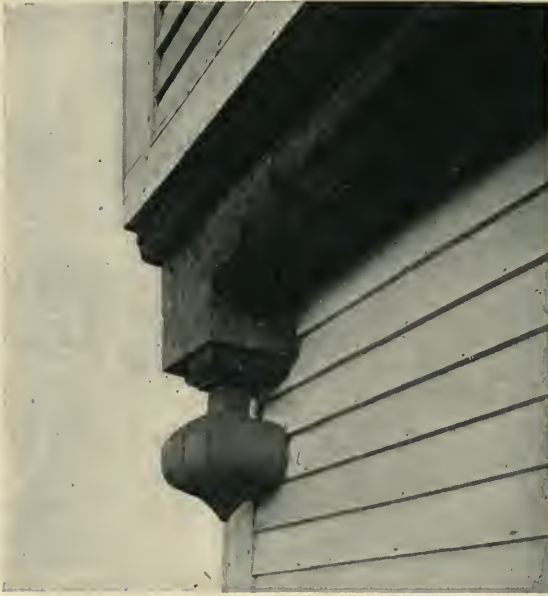
DETAIL OF OLD BROWN HOUSE, HAMILTON, MASSACHUSETTS
