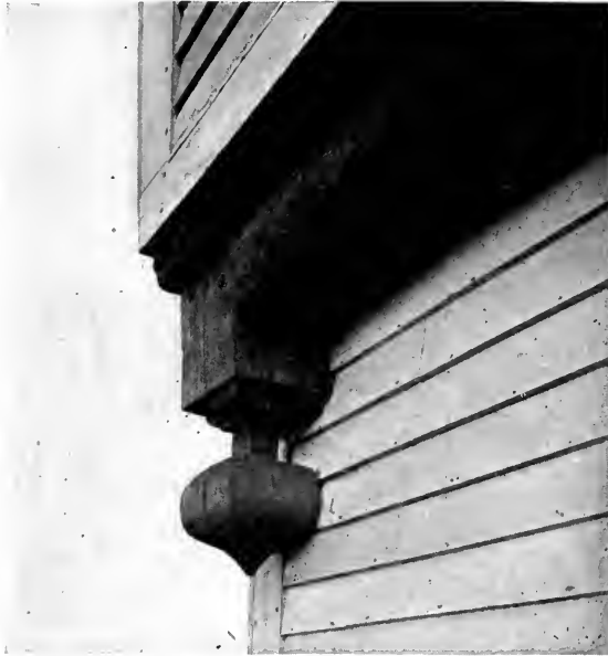
DETAIL OF OLD BROWN HOUSE, HAMILTON, MASSACHUSETTS
