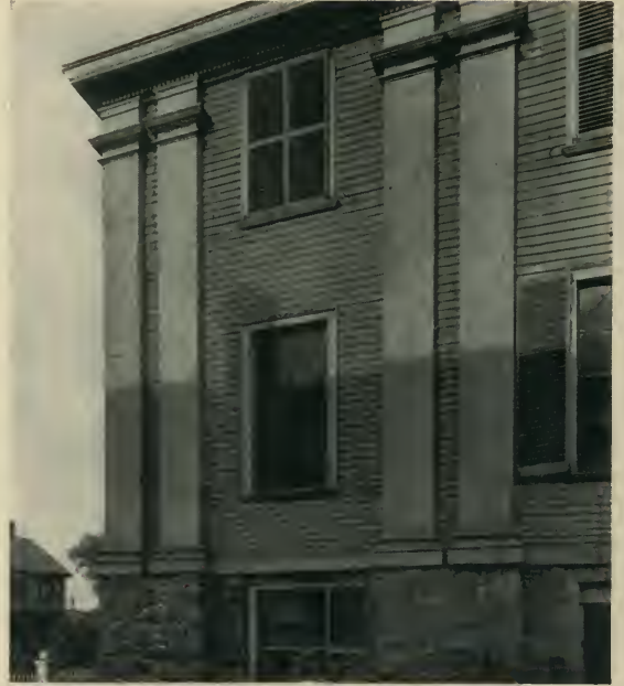
Pilaster and Cornice Detail
