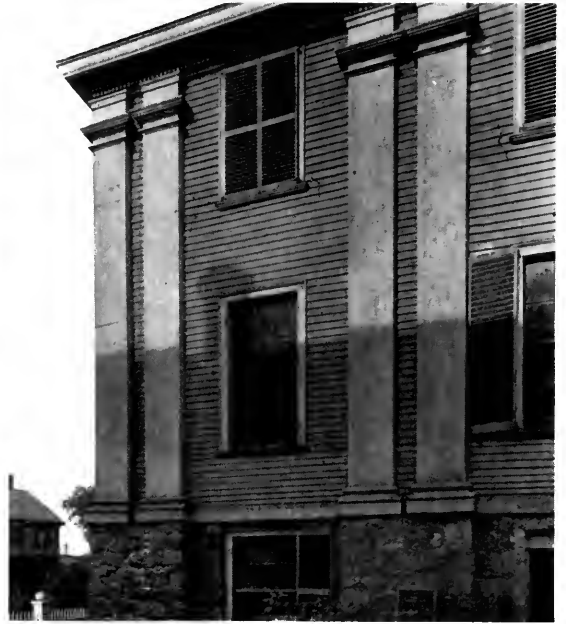
Pilaster and Cornice Detail
