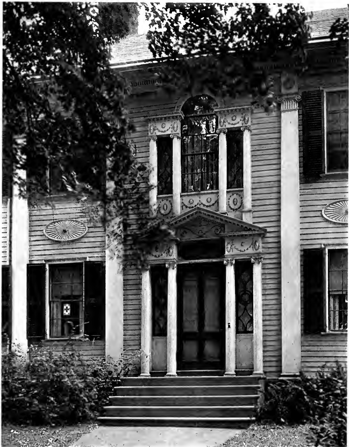
THE FULLERTON HOUSE, WINDSOR, VERMONT. Entrance Detail.
