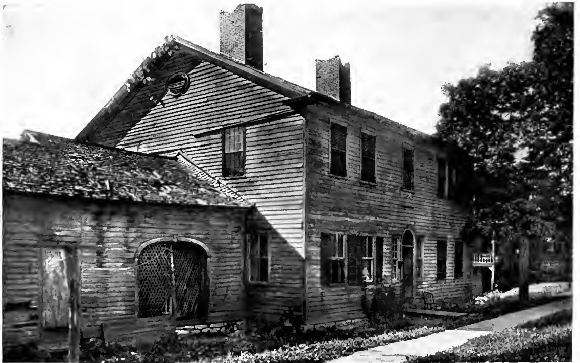
HOUSE AT MIDDLEBURY, VERMONT.
