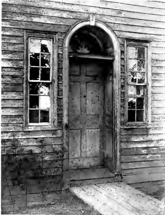
HOUSE AT MIDDLEBURY, VERMONT.
