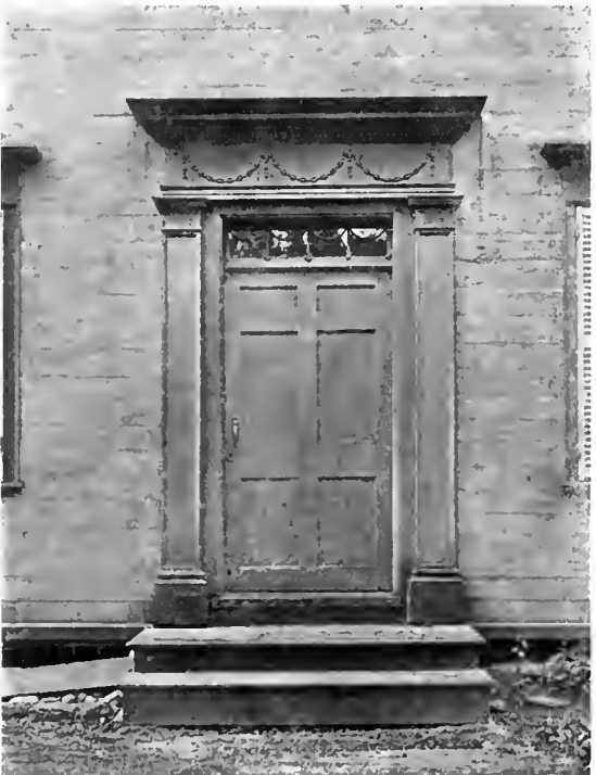
THE JOHONNOT HOUSE, WINDSOR, VERMONT.
