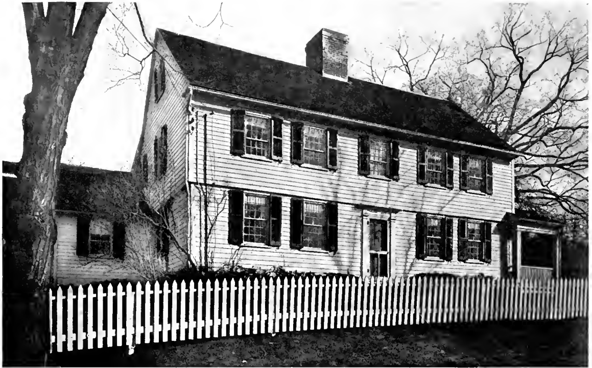
HOUSE AT HILLSTEAD, FARMINGTON, CONNECTICUT. Excellent but rather sophisticated example of type of house which embraces elements of design from several periods, all probably earlier than itself.
