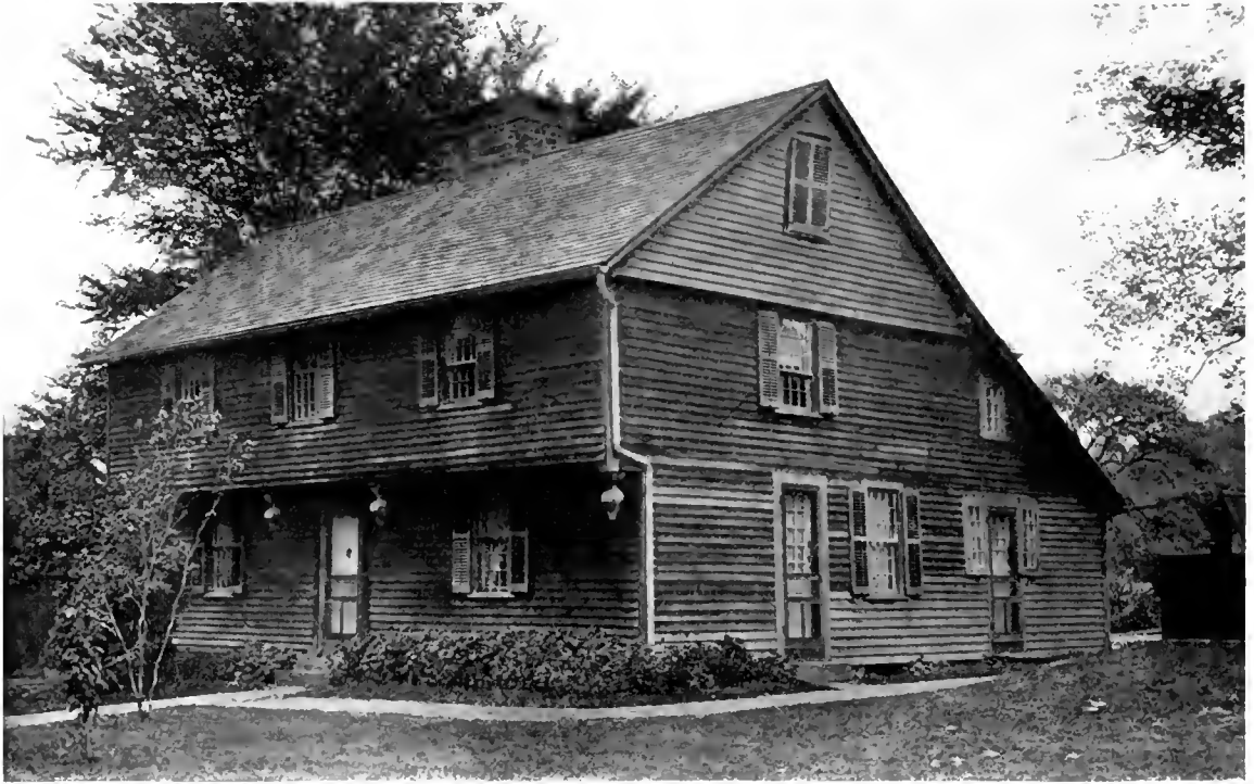
THE WHITMAN HOUSE, FARMINGTON, CONNECTICUT. Noteworthy as an example of the overhang construction with original drops and stone chimney.
