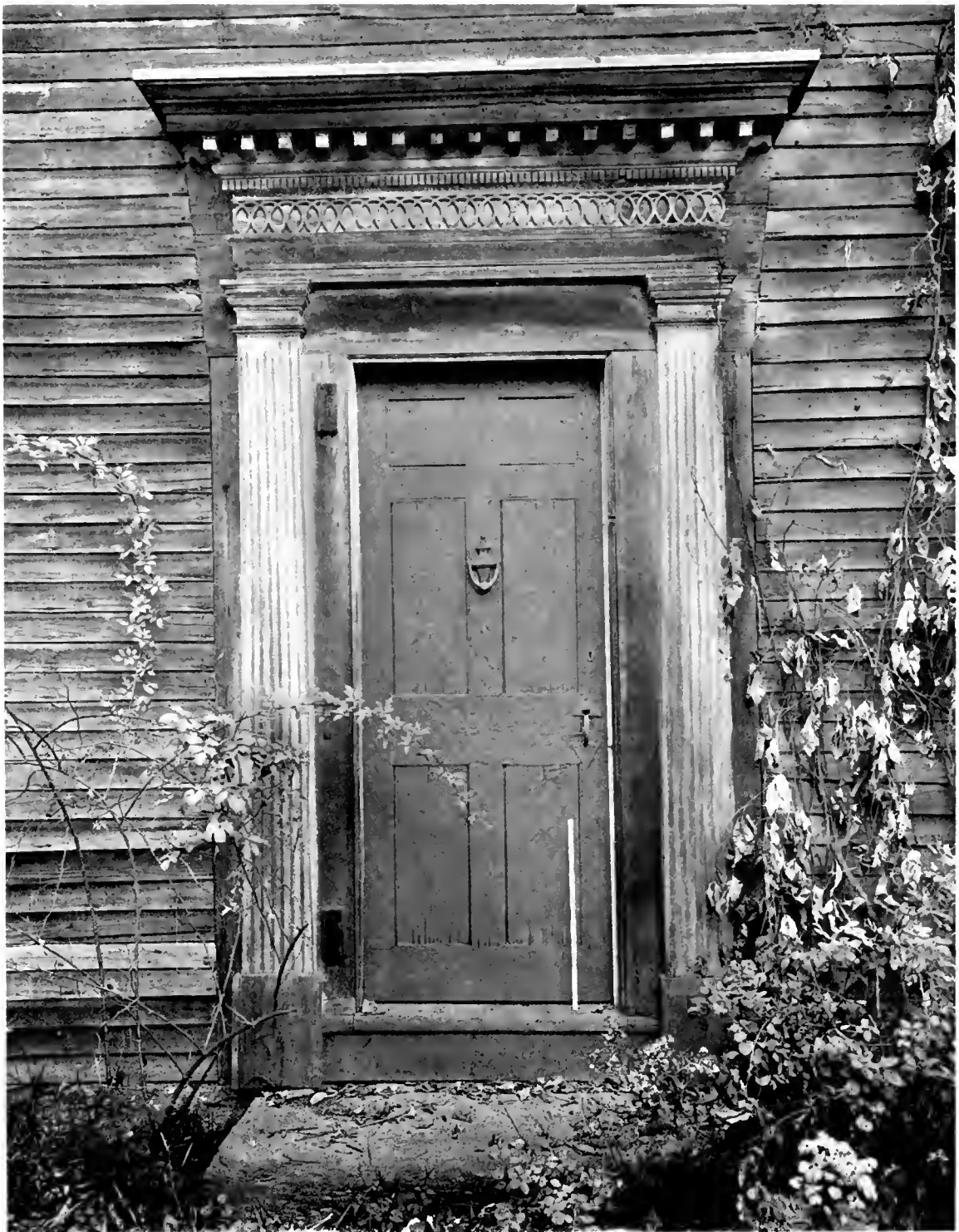
THE FRARY HOUSE, DEERFIELD, MASSACHUSETTS. Detail of Side Entrance Doorway.
