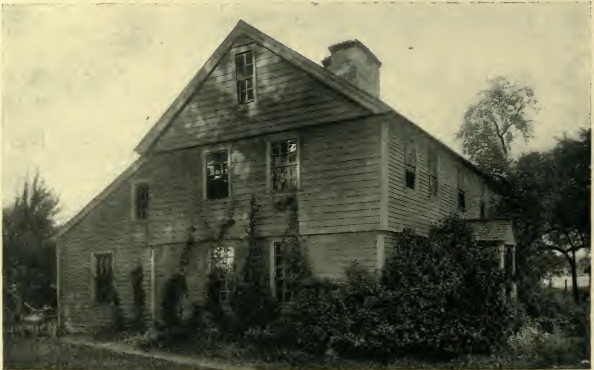
THE WALKER HOUSE, STRATFORD, CONNECTICUT. Built circa 1670.
