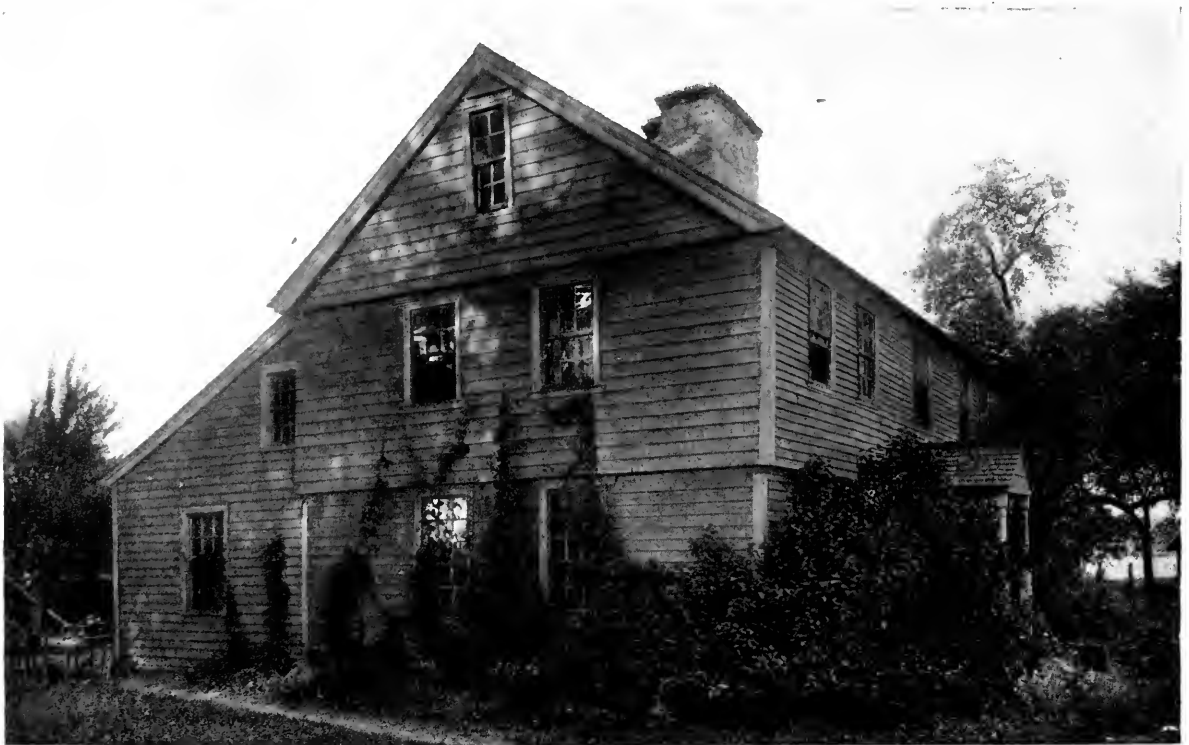
THE WALKER HOUSE, STRATFORD, CONNECTICUT. Built circa 1670.
