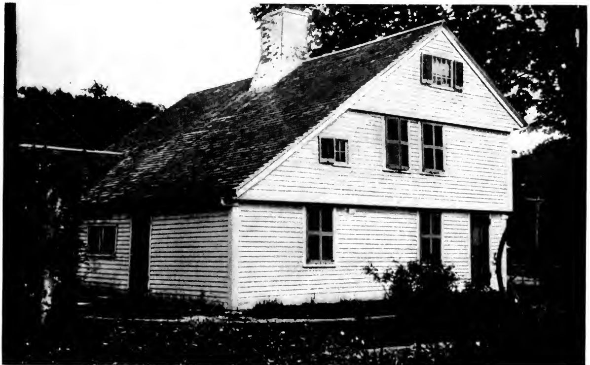
THE HOLLISTER HOUSE, SOUTH GLASTONBURY, CONNECTICUT. Built circa 1675.
