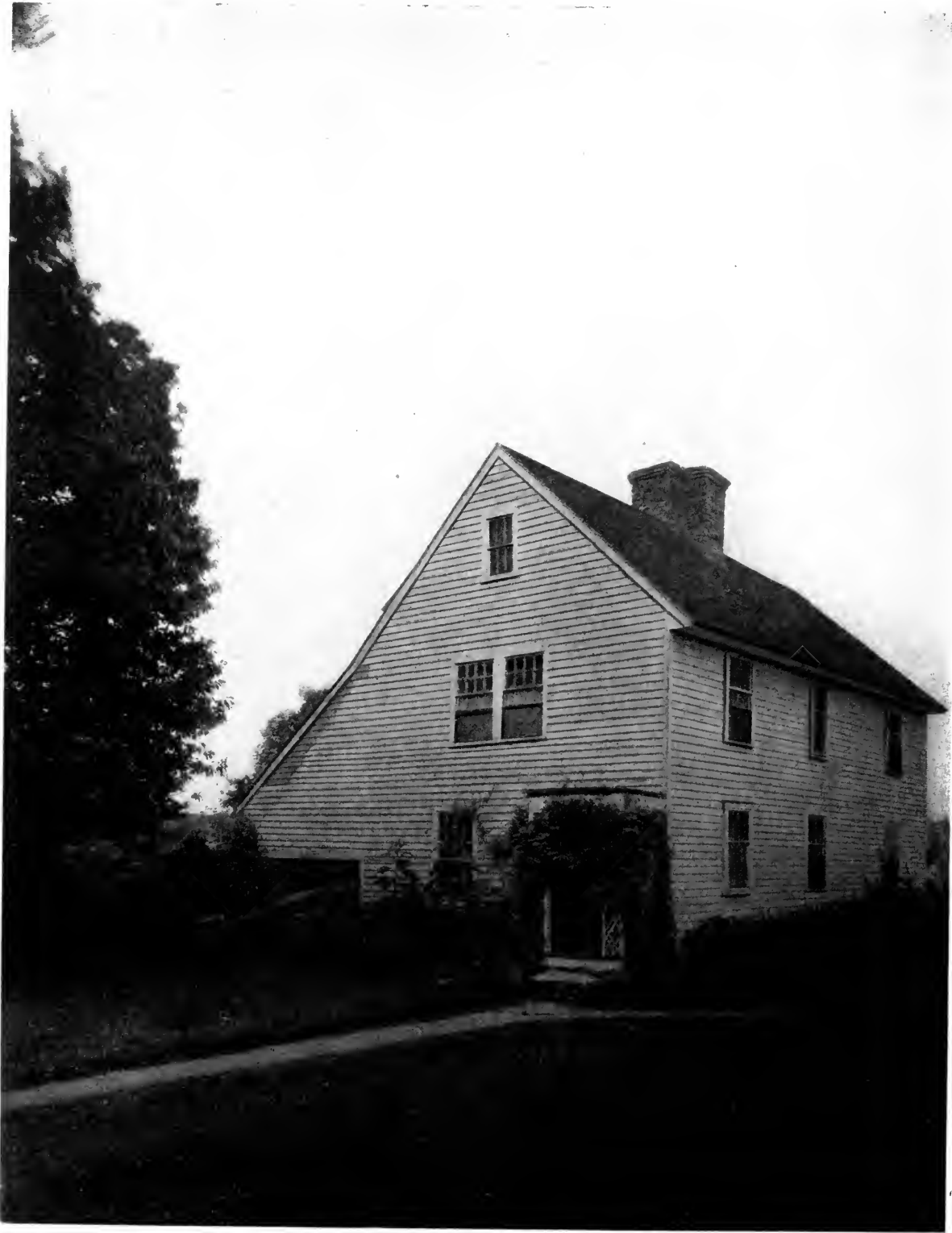
THE ACADIAN HOUSE, GUILFORD, CONNECTICUT.
