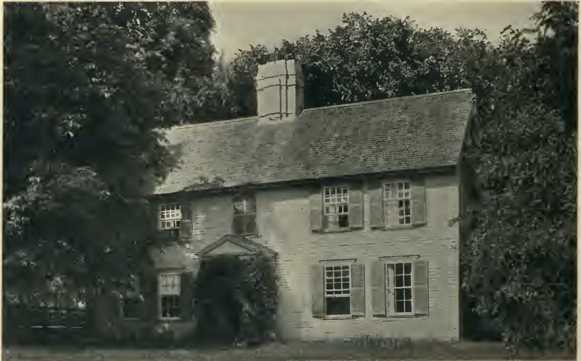
"GOVERNOR BRADSTREET HOUSE," NORTH ANDOVER, MASSACHUSETTS.
