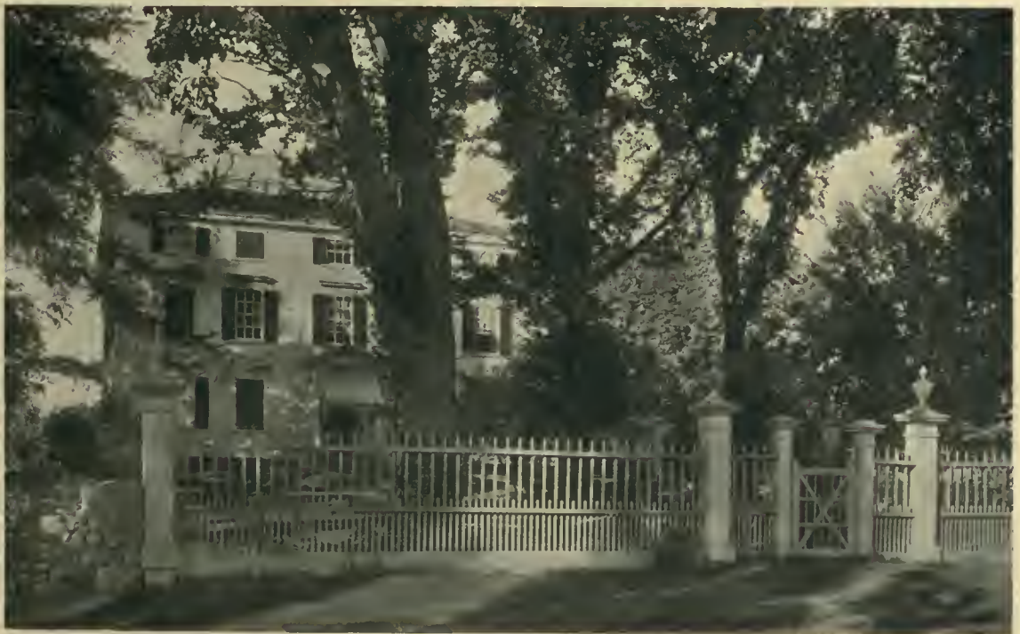
THE KITTREDGE HOUSE, NORTH ANDOVER, MASSACHUSETTS.
