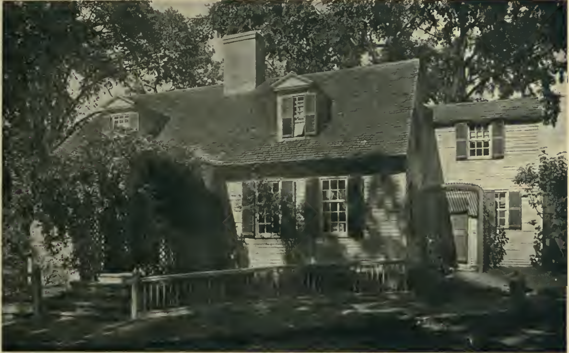
OLD HOUSE AT ANDOVER, MASSACHUSETTS
