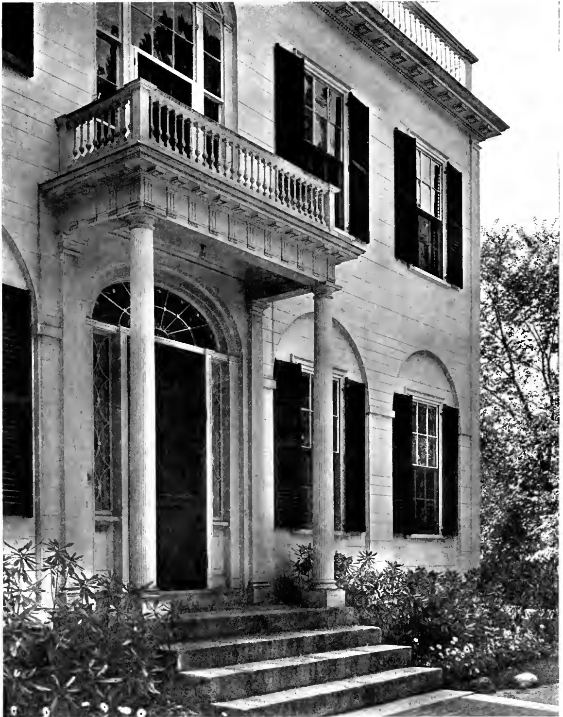
THE PHELPS HOUSE, ANDOVER HILL, MASSACHUSETTS. 1809-1812. Detail of Doorway and Entrance Porch.
