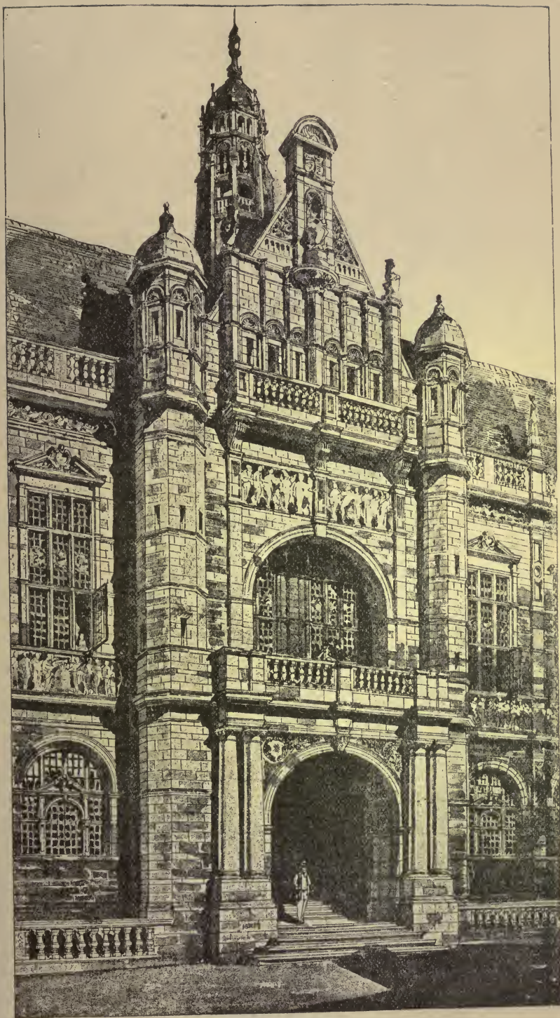
ENTRANCE, SHEFFIELD MUNICIPAL BUILDING,
