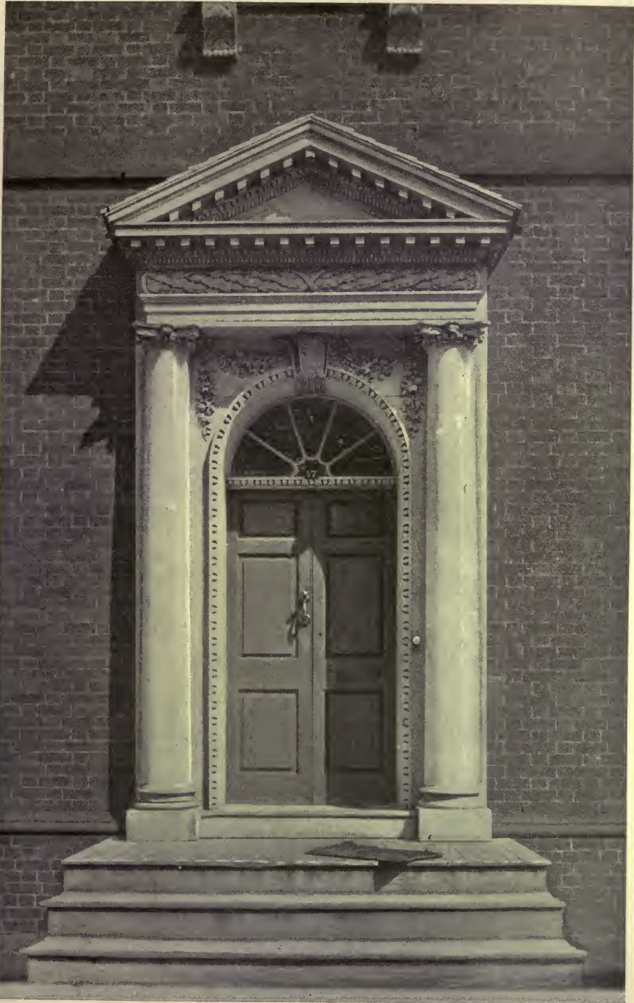
DOORWAY OF HARWOOD HOUSE.
