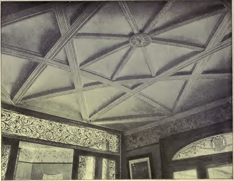
CEILING UNDER N. POULSEN'S FLOOR CONSTRUCTION.
