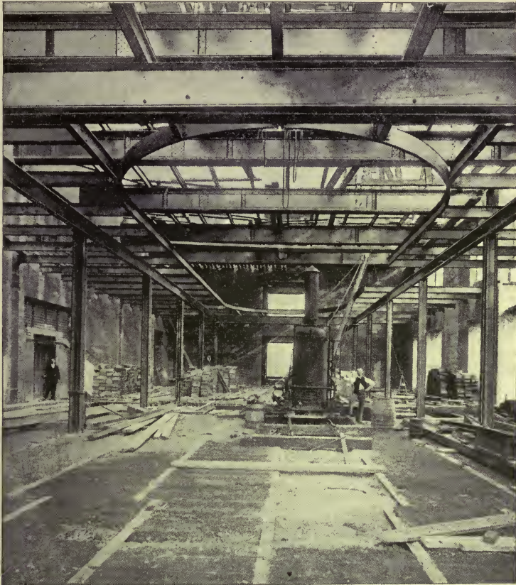
Riveted girder and hoisting engine, new wing, American Museum of Natural History.
