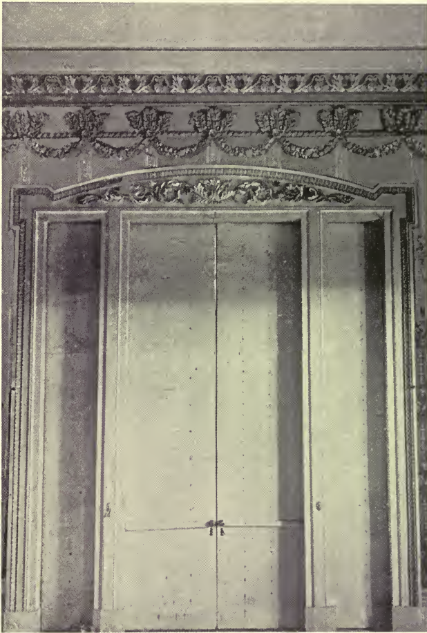
WINDOW IN LIBRARY OF VAN RENSSELAER MANOR HOUSE.
