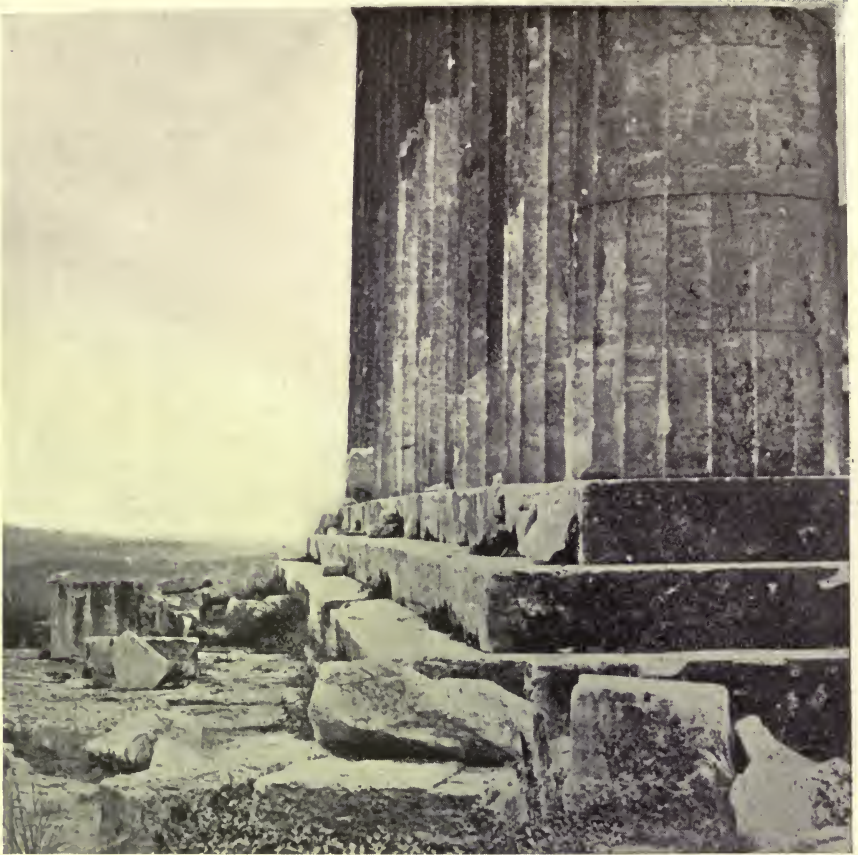
Illustration showing the curves of the Stylobate of the Parthenon. (From a photograph)
