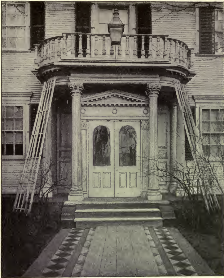
GOVERNOR LANGDON'S HOUSE, PORTSMOUTH, N. H.
