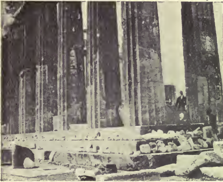
Illustration showing the curves of the Stylobate of the Parthenon. (From a photograph.)
