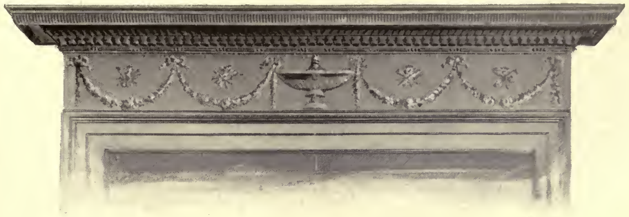
Entablature of a door in No. 25 Pearl Street, Albany.
