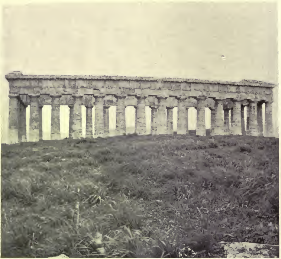
Greek temple at Egesta, Sicily. From a photograph showing the curves of the entablature.
