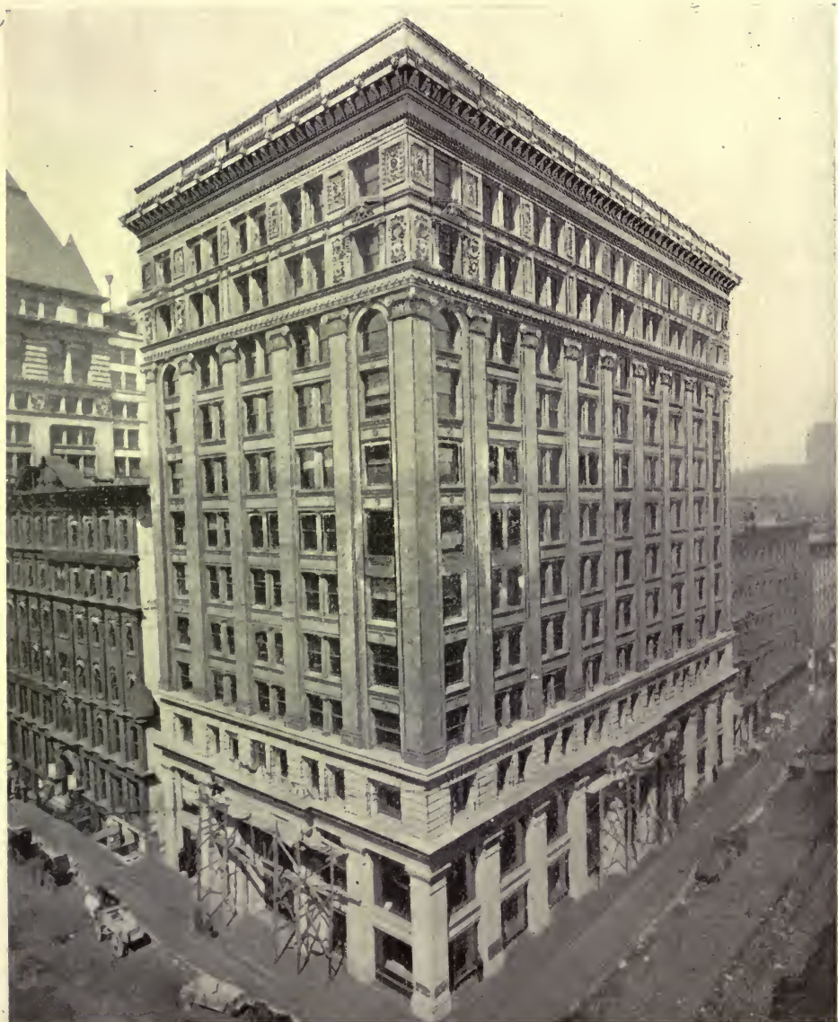
NEW YORK LIFE INSURANCE COMPANY'S BUILDING.
