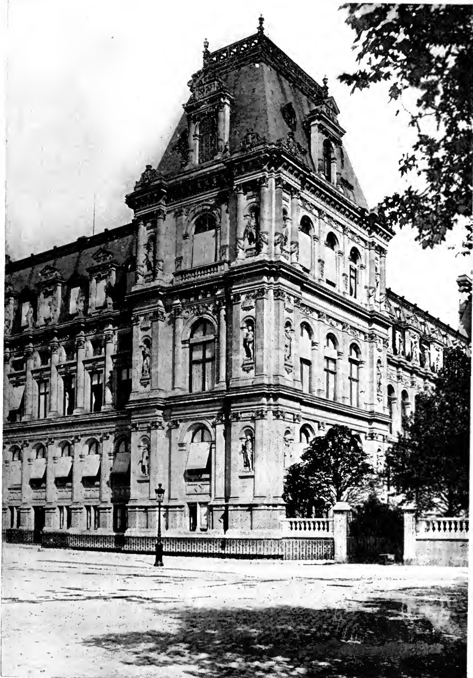
PAVILION ON THE QUAY CITY HALL, PARIS.
