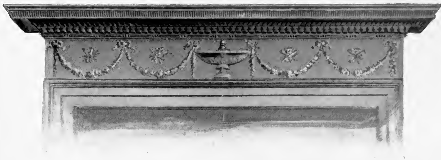
Entablature of a door in No. 25 Pearl Street, Albany.
