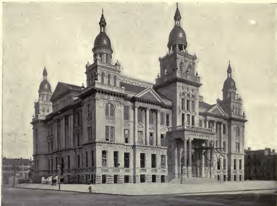
THE NEW CITY HALL, JERSEY CITY.
