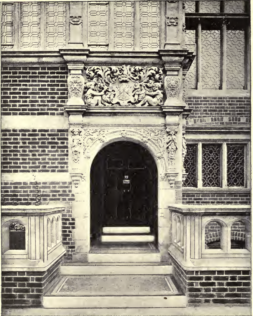
ENTRANCE, HARRINGTON GARDENS.
