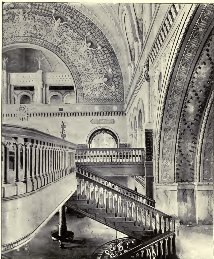
GRAND STAIRCASE, BETWEEN THE WAITING-ROOM AND THE GRAND HALL—UNION STATION.
