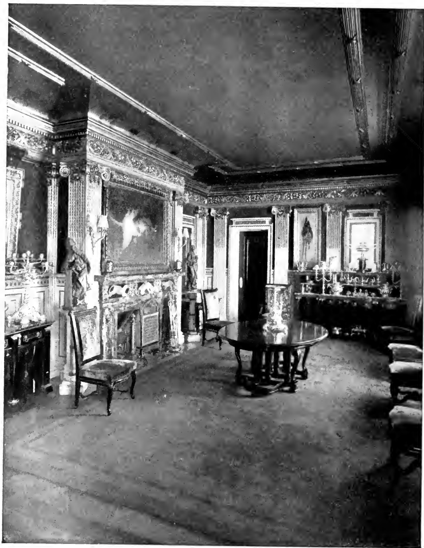
DINING-ROOM, GEORGIAN COURT.
