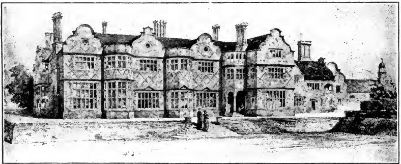
81. The same. The projection of one gable does not prevent its grouping with the others. There is also a group of three bays between the gables.
