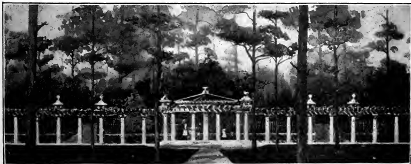
Pergola in Grounds of Georgian Court.
