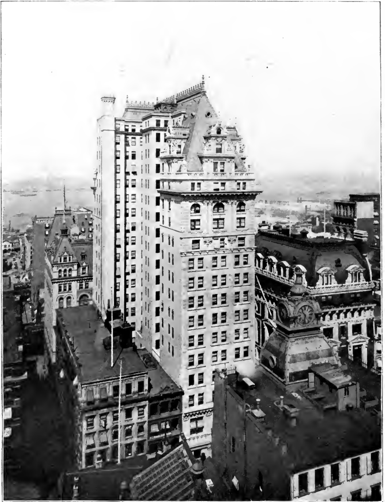
THE WASHINGTON LIFE BUILDING. (From the East.)
