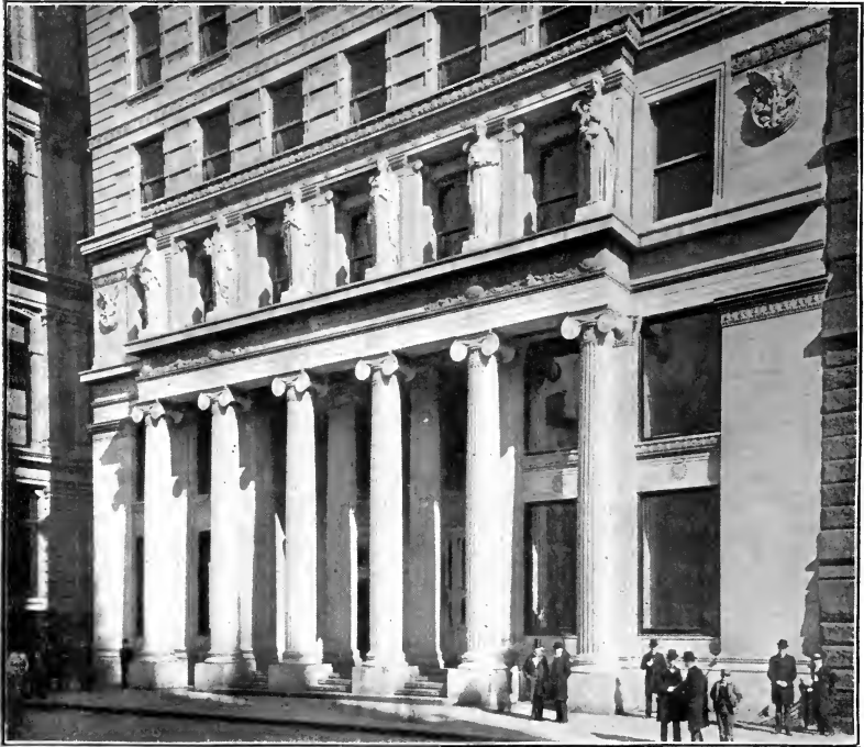
FIG. 3.—ENTRANCE TO AMERICAN SURETY BUILDING.
