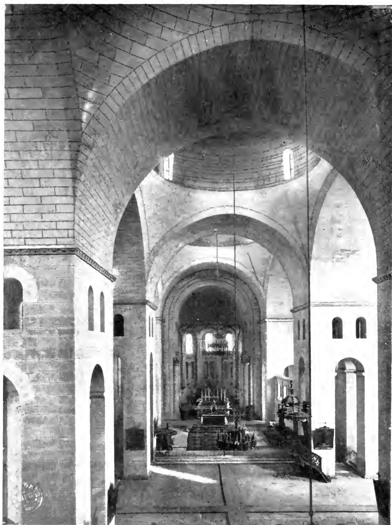
S. FRONT, PÉRIGUEUX. (View of Interior, from the West.)
