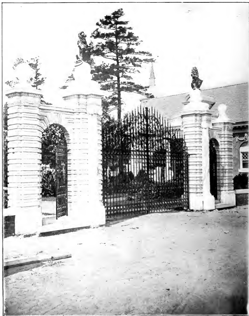
THE ENTRANCE GATES TO GEORGIAN COURT.
