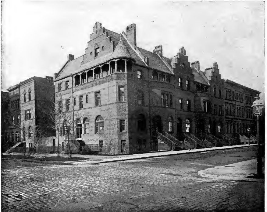
SOUTHWEST CORNER OF WEST END AVENUE AND 83D STREET.
