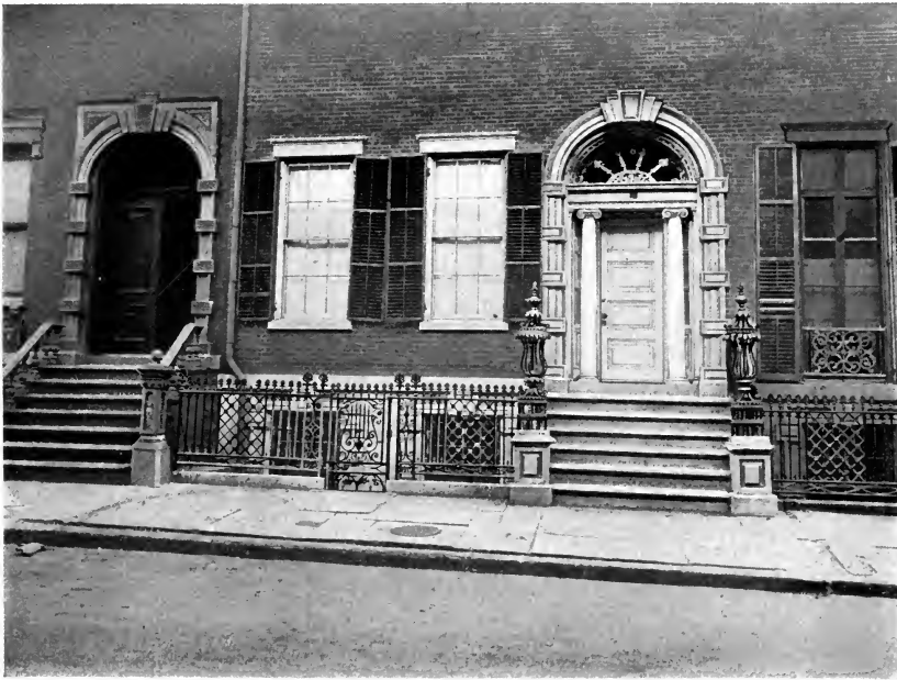
NOS. 27 AND 29 EAST 4TH STREET.
