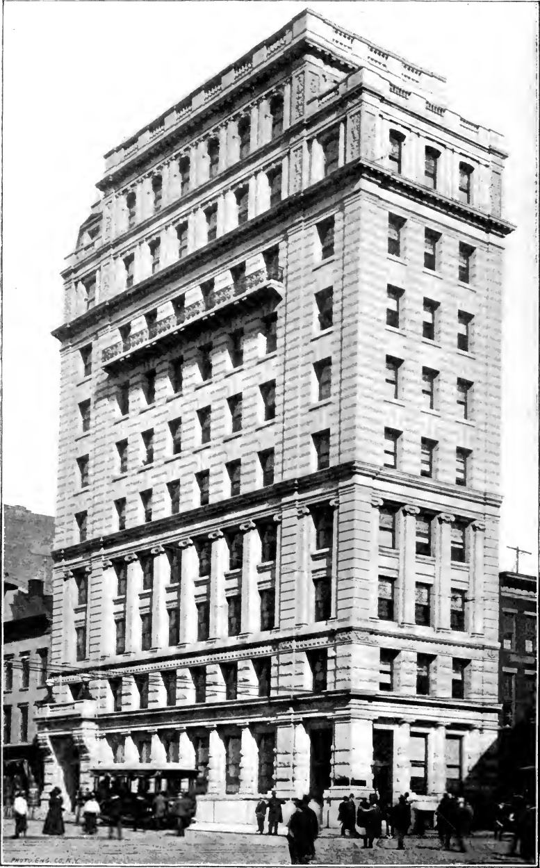
MECHANICS' BANK BUILDING. Fulton and Montague Streets, Brooklyn.
