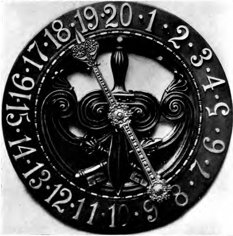
FIG. 4.—ELEVATOR INDICATOR, AMERICAN SURETY BUILDING.
