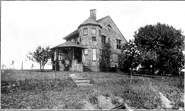
228. Small country house, a single mass, with one subordinate mass and one appendage.
