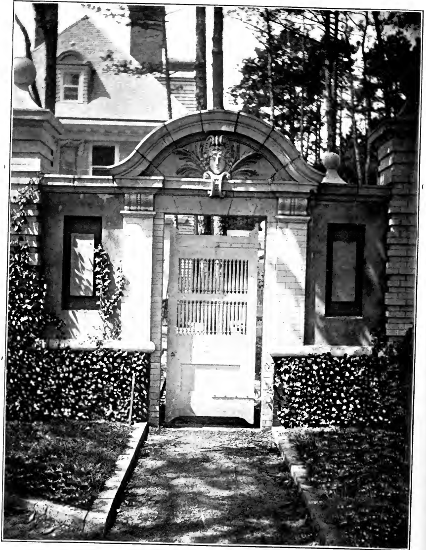
SERVANTS' ENTRANCE, GEORGIAN COURT.
