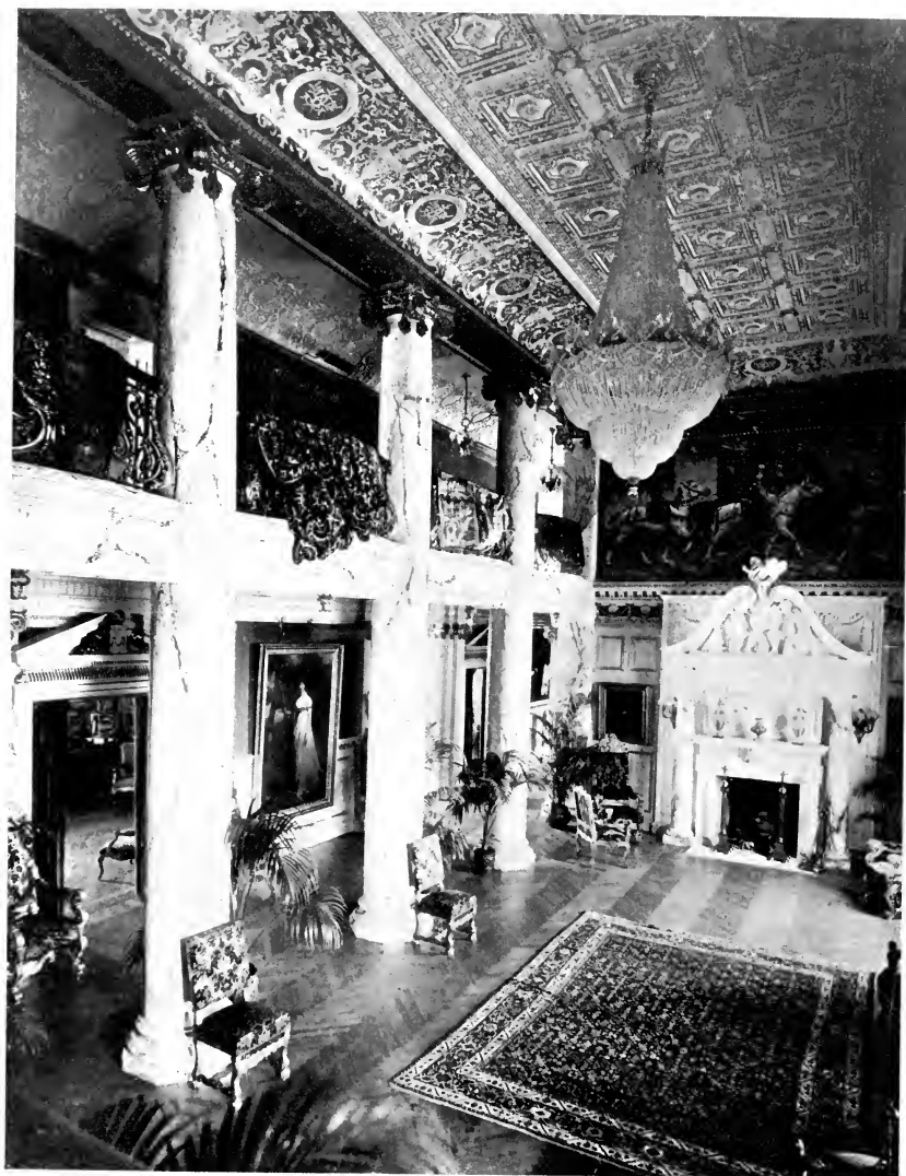
THE GREAT HALL OF GEORGIAN COURT, LOOKING WEST.
