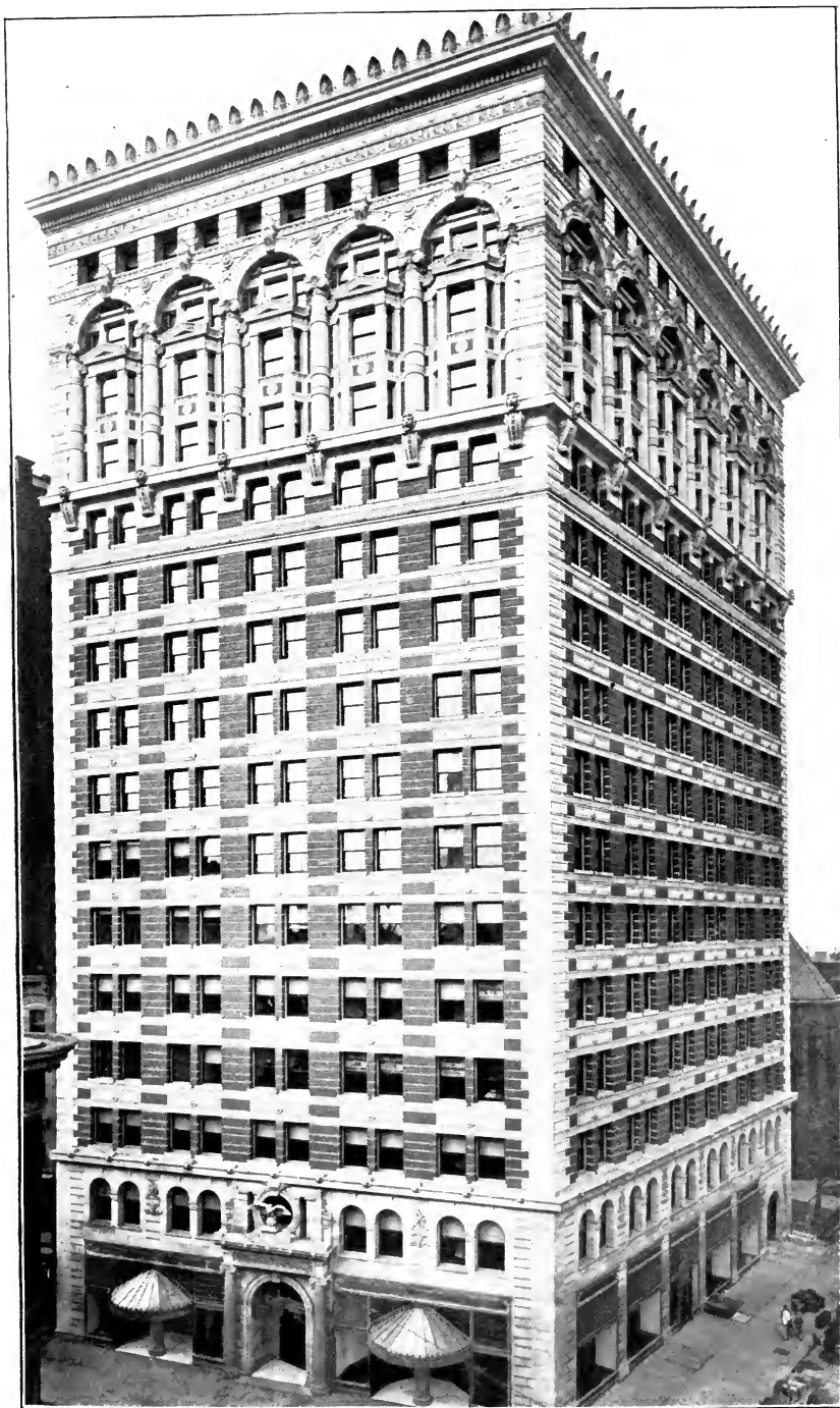
FIG. 5.—ST. JAMES' BUILDING. S. W. Corner Broadway and 26th St., New York City. Bruce Price, Architect.
