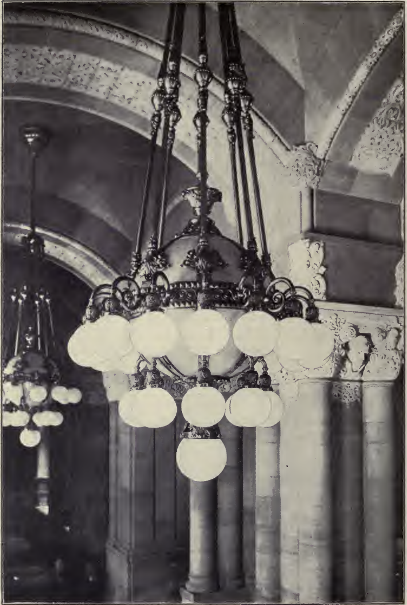
INTERIOR ELECTRIC LIGHT FIXTURES. CAPITOL, ALBANY, N. Y.
