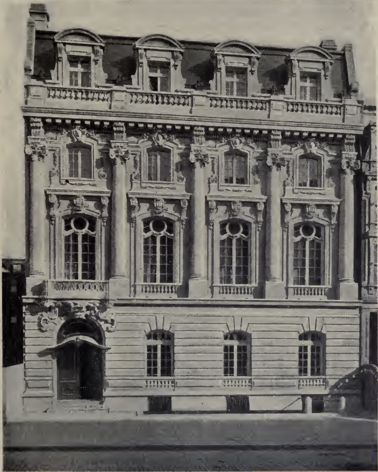
RESIDENCE OF HENRY T. SLOANE (Of Indiana Limestone),
