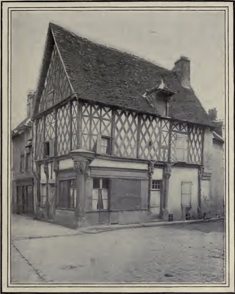
FIG. 16.—WOODEN HOUSE, LEVROUX (INDRE).
