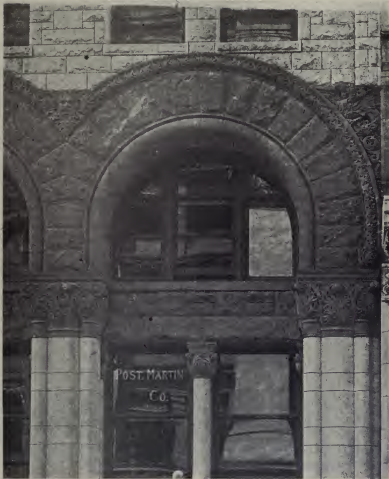
45 and 47 Wall Street.
