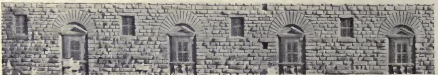
Fig. 6. Part of basement of Pitti Palace, Florence. The blocks though classed as rock-faced are not left entirely as the stone first broke away, but have been worked to a somewhat rounded form. Those of the retaining walls below are much bolder.
