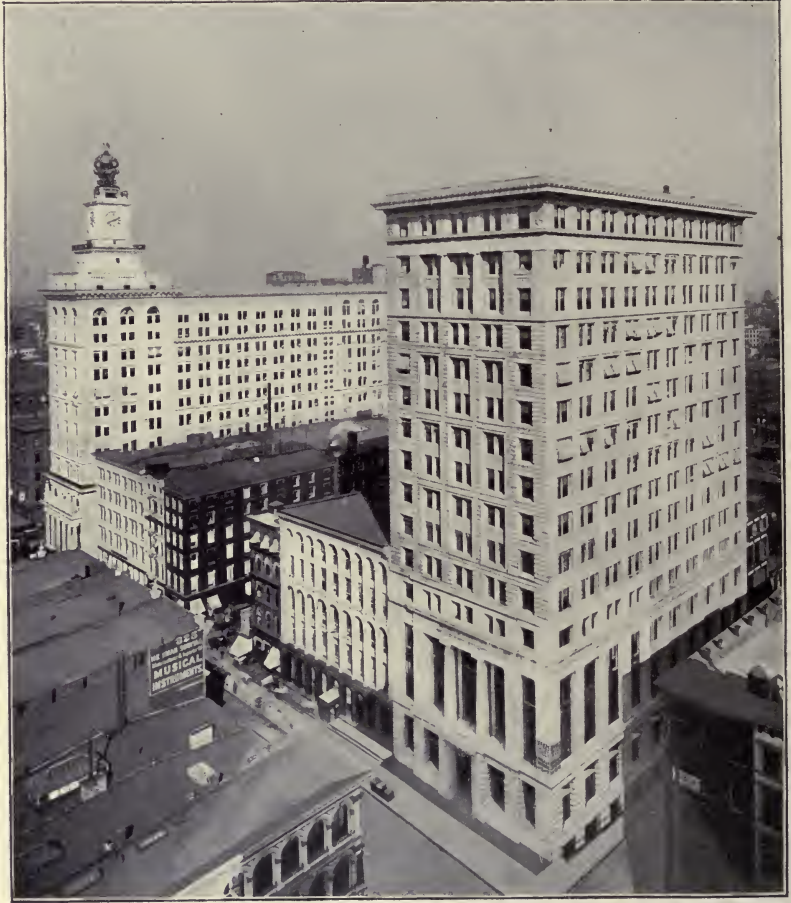
CENTRAL NATIONAL BANK BUILDING, Pearl Street and Broadway, New York City.
