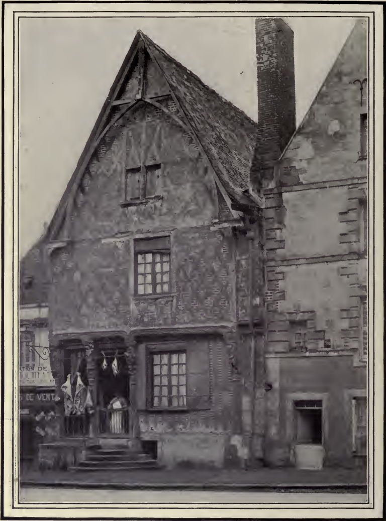
FIG. 15.—WOODEN HOUSE, LUYES (INDRE-ET-LOIRE).
