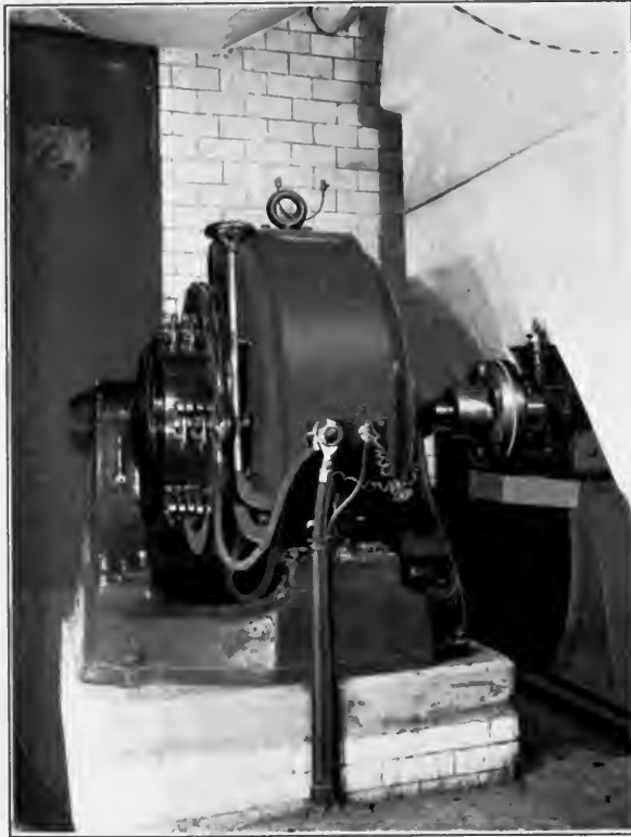
C & C ELECTRIC MOTOR INSTALLED IN HOTEL ST. REGIS.
