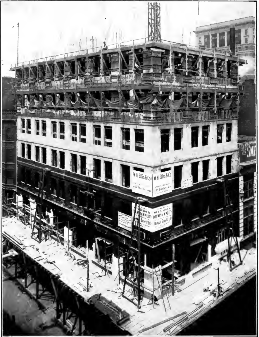
THE INGALLS BUILDING. Showing Method of Construction.
