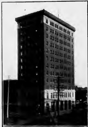
July 1.—External construction finished.
