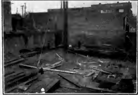
Dec. 15, 1902.—Excavation complete and column bases set.
