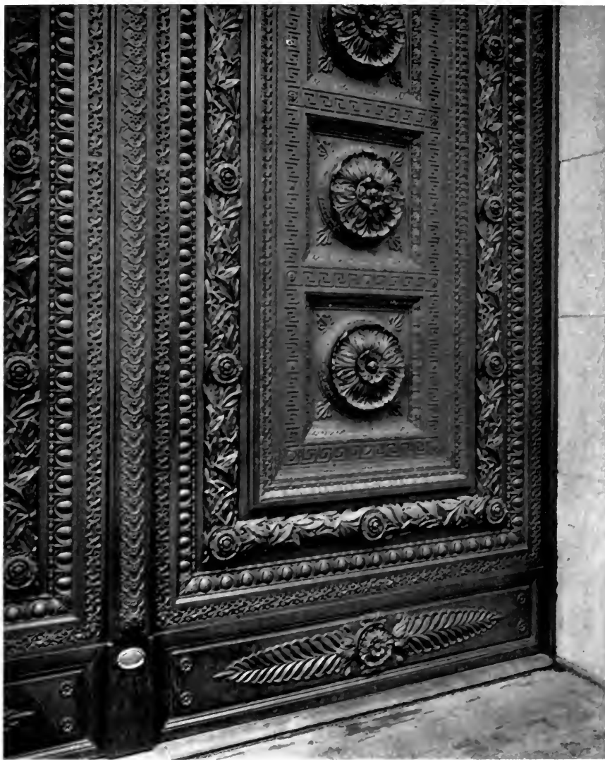
DETAIL OF THE MAIN DOOR.
