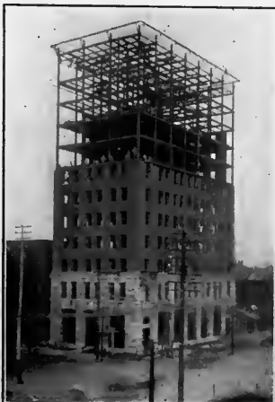
March 13.—Brickwork seven stories high.
