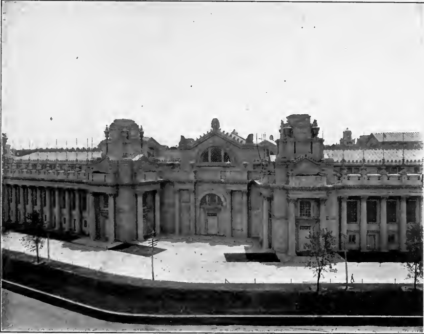
PROJECTING ANGLE OF THE ELECTRICITY BUILDING.
