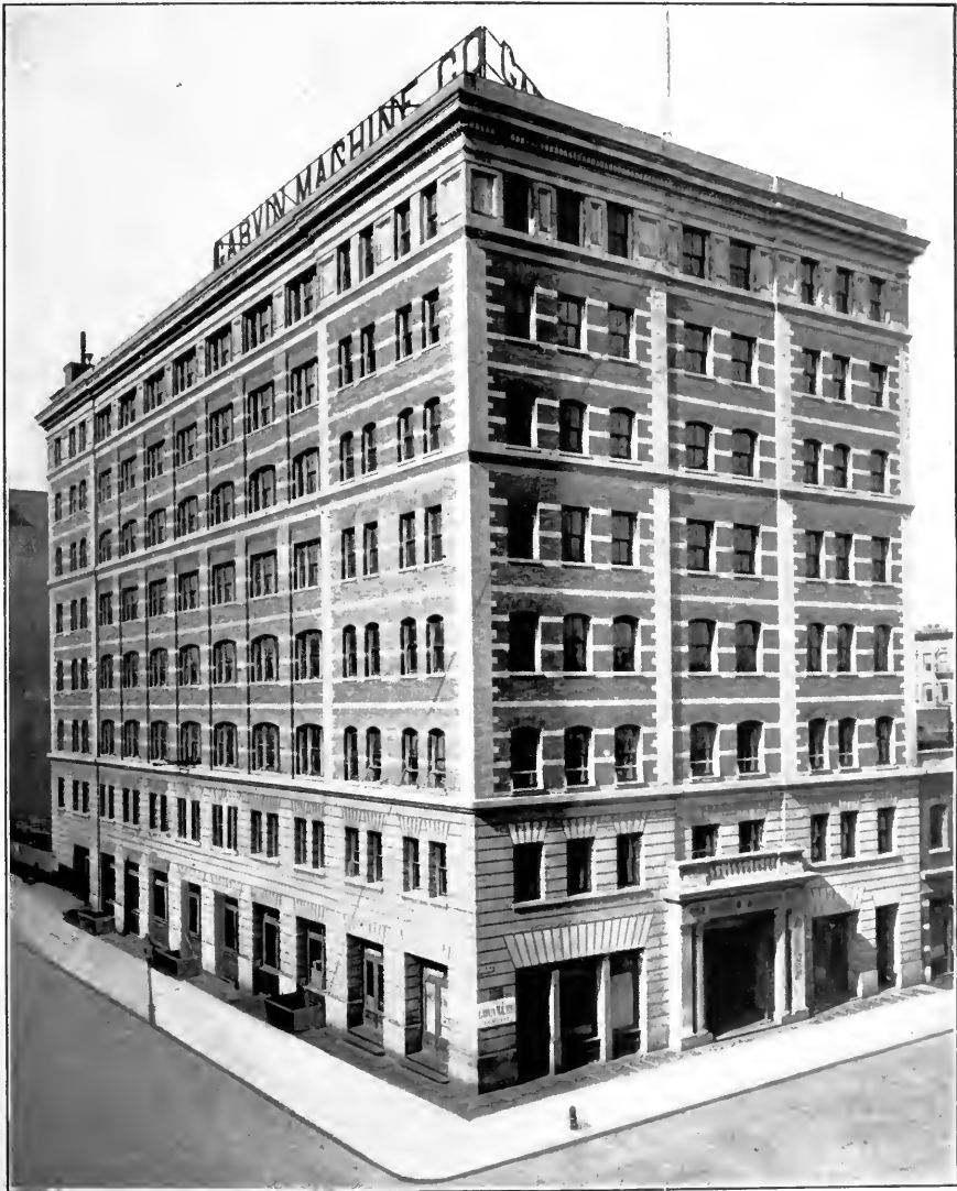
FIG. 8.—BUILDING OF THE GARVIN MACHINE CO.
