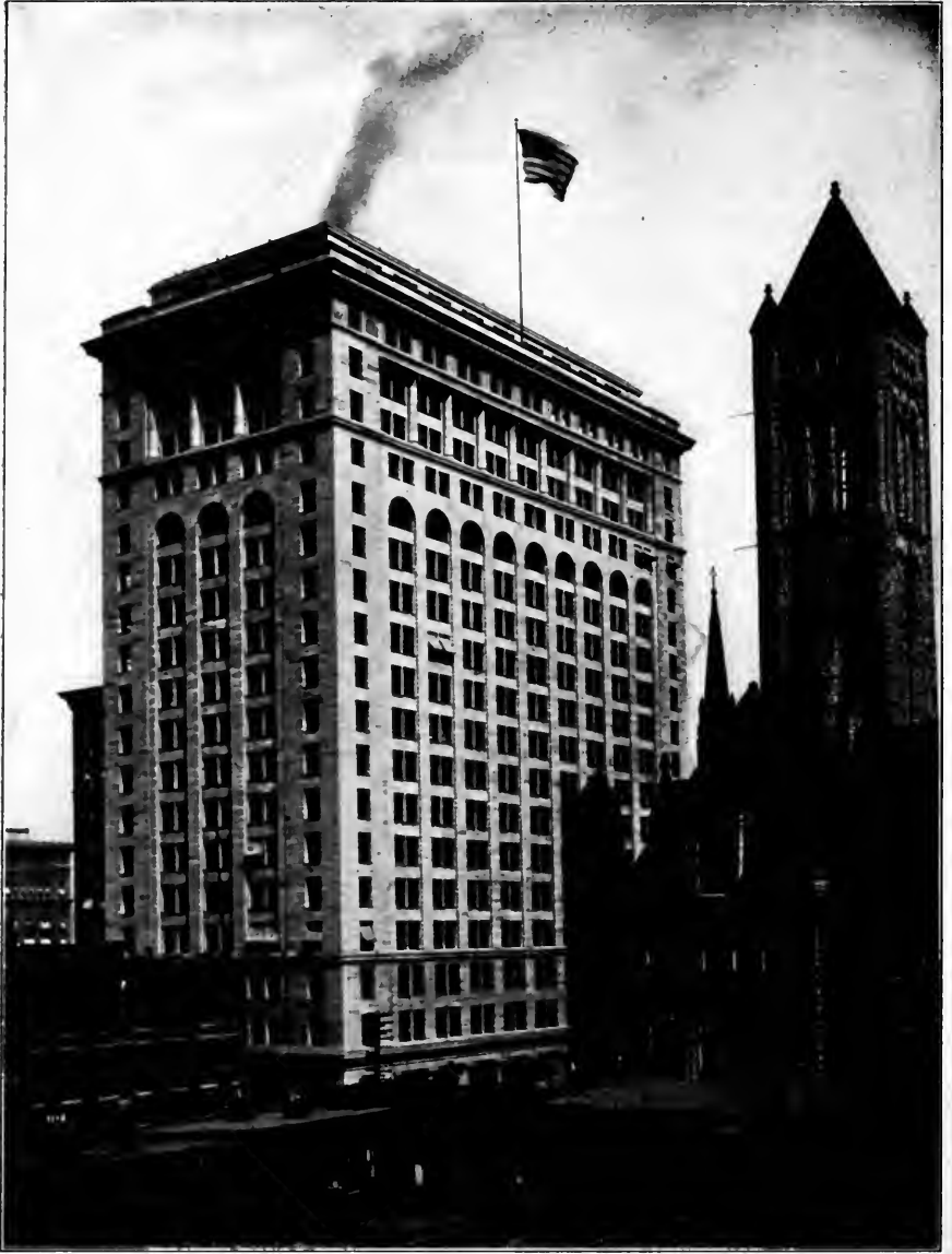
THE FRICK BUILDING.
