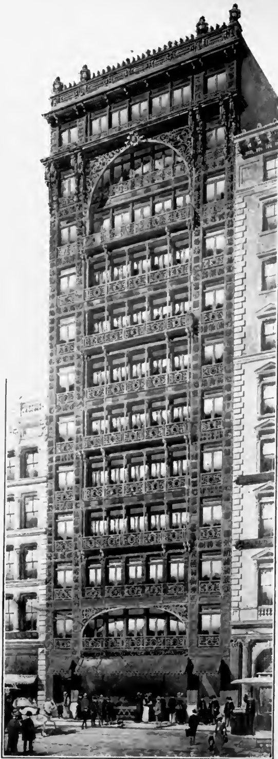
THE SINGER BUILDING AS COMPLETED.
