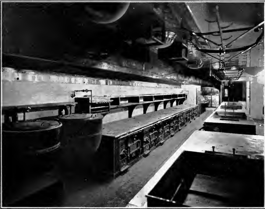
THE HOTEL ST. REGIS. (The Kitchen.)
