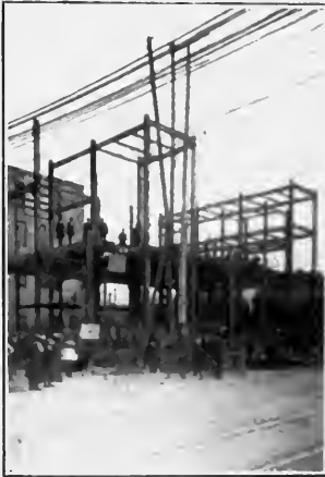
Jan. 2, 1903.—Foundations complete and steelwork carried above first floor.
