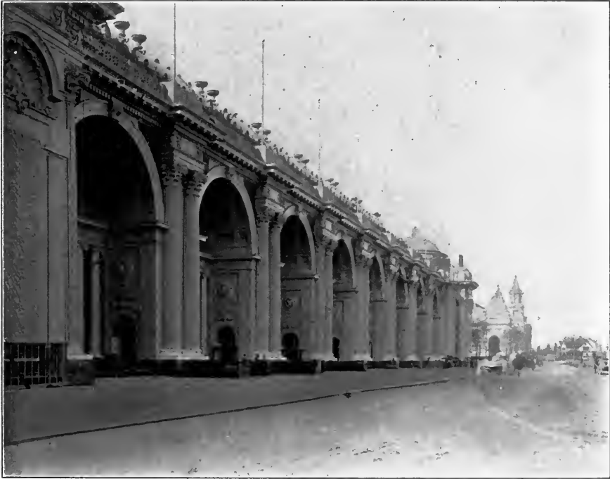
NORTH FAÇADE OF THE PALACE OF MANUFACTURES.
