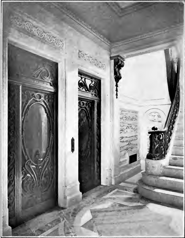
BRONZE-FINISHED IRON STAIR RAILING AND ELEVATOR ENCLOSURES.
