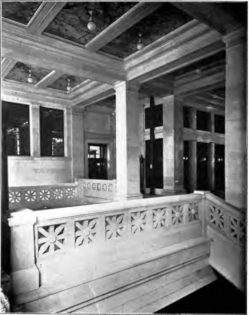
STAIRS AND HALL—FRICK BUILDING.
