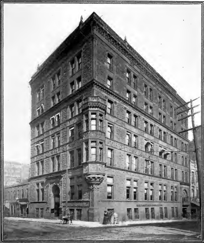
NEW ENGLAND LIFE BUILDING.
