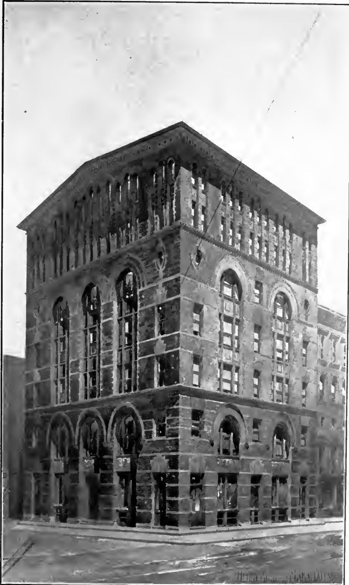
FIG. 7.—THE TARRANT BUILDING.
