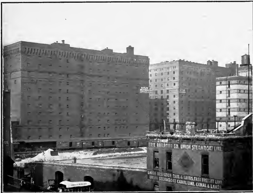
FIG. 17. THE BUTLER BROS.' WAREHOUSES.
