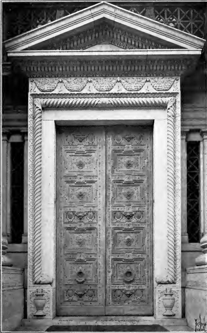
BRONZE DOORS OF KNICKERBOCKER TRUST CO.'S BUILDING.
