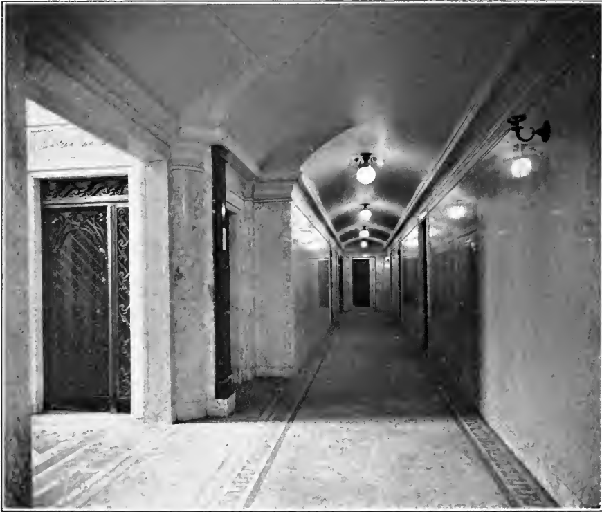
TYPICAL CORRIDOR IN HOTEL ST. REGIS. (Marble furnished by John H. Shipway & Bro.)
