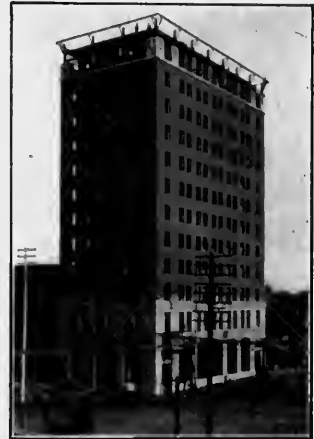
April 1.—Brickwork to lower tier of cornice.
