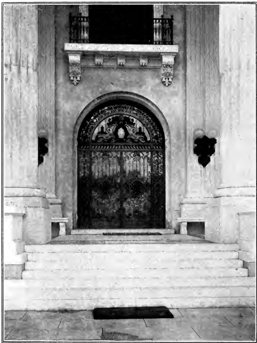
ENTRANCE DOOR OF "WHITEHALL."
