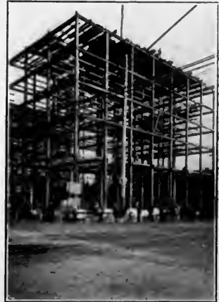
Jan. 15.—Granite water-table set and six tiers of beams in place.
