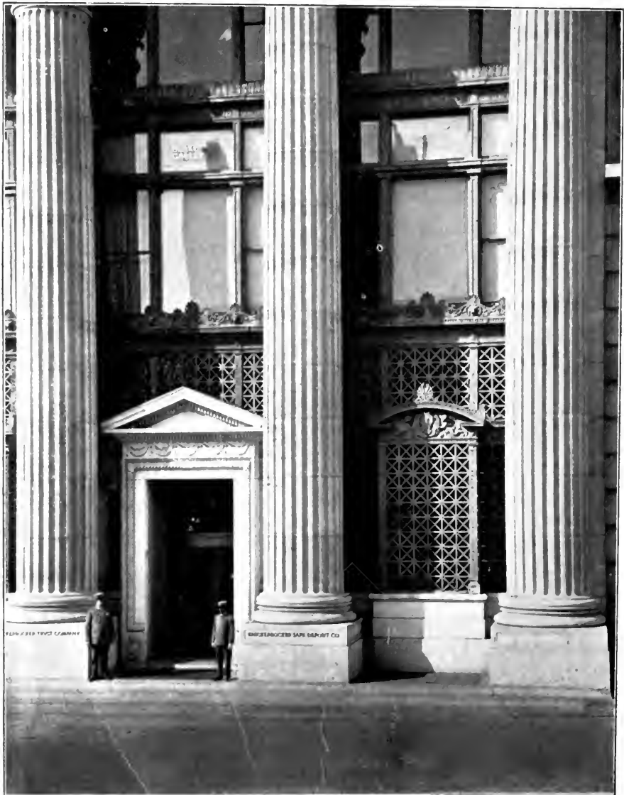
THE BUILDING OF THE KNICKERBOCKER TRUST CO.—DETAIL OF THE EXTERIOR. 34th Street and Fifth Avenue, New York City. McKim, Mead & White, Architects.
