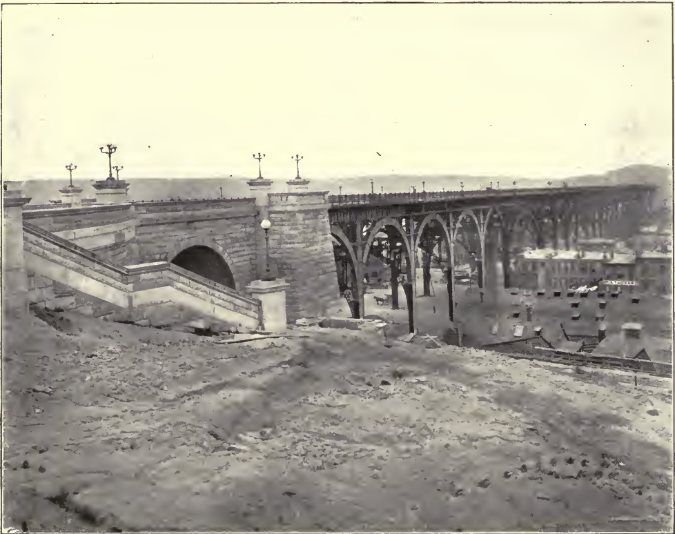
FIG. 8. THE MANHATTAN VALLEY VIADUCT.
