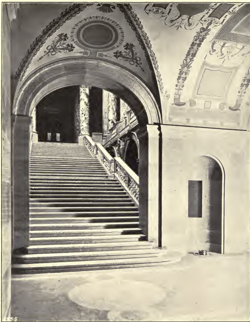
EAST END OF THE GRAND STAIRWAY.
