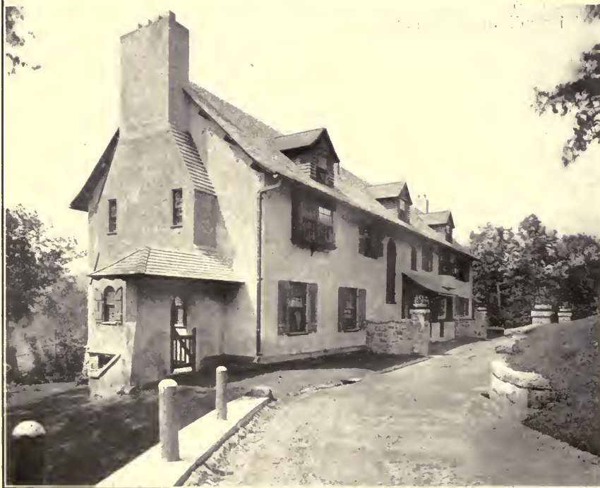
THE HOUSE OF MR. T. HARLESTON DEACON.
