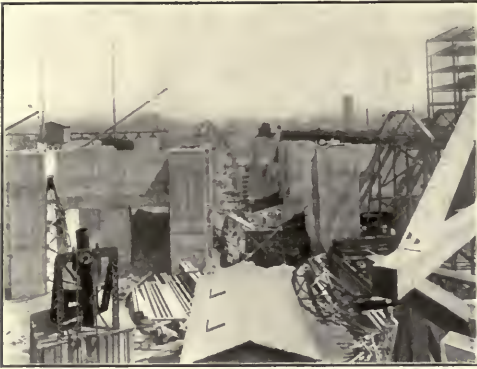
THE STATION IN THE COURSE OF CONSTRUCTION.
