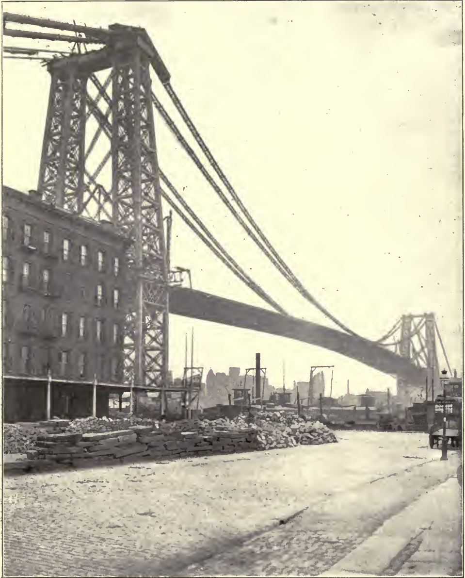
FIG. 1. THE WILLIAMSBURGH BRIDGE. Before the Building of the Stiffening Truss.
