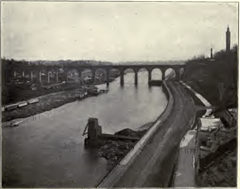
FIG. 7. "HIGH" BRIDGE OVER THE HARLEM RIVER.
