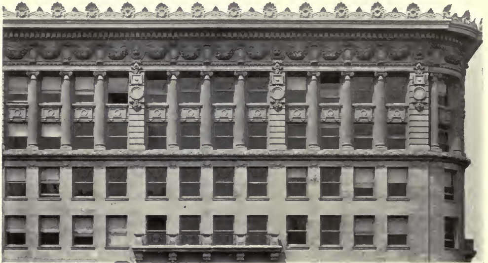
DETAIL SHOWING TORUS, COLUMNS, PILASTERS, FACIA AND FRIEZE OF TERRA-COTTA. BUILDING NORTH-WEST CORNER OF FIFTH AVENUE AND THIRTY-SECOND STREET, NEW YORK CITY.
