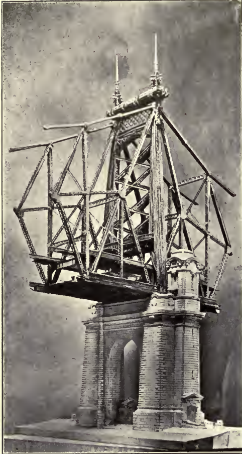
FIG. 20. PIER AND TOWER OF THE BLACKWELL'S ISLAND BRIDGE.
