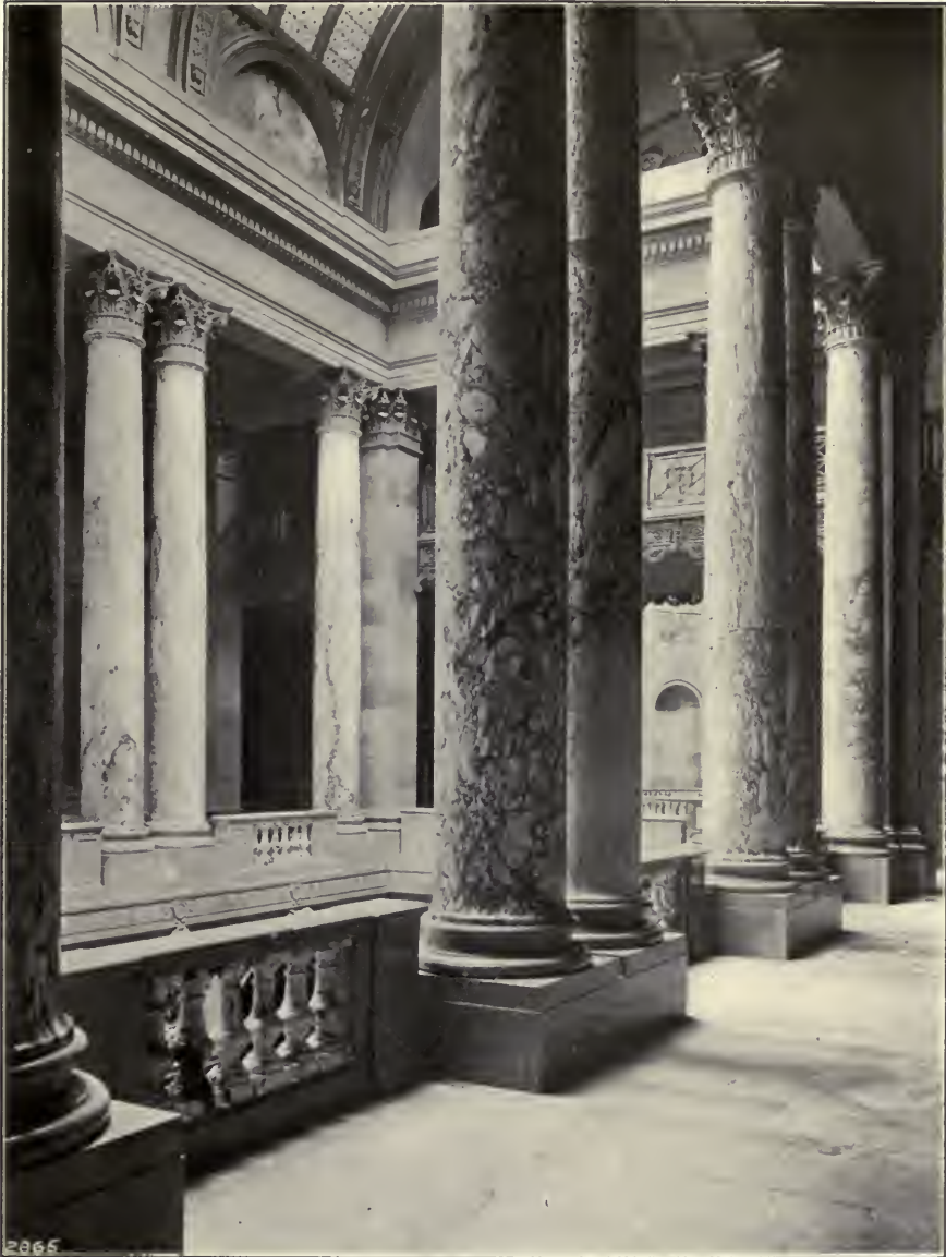
EAST END OF THE CORRIDOR ON THE SECOND FLOOR.
