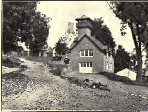
BUILDING FOR HOOK AND LADDER CO. Wyoming, N. Y. Pond & Pond, Architects.
