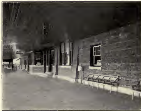
THE STATION OF C. & N. W. R. R. Madison, Wis. Frost & Granger, Architects.
