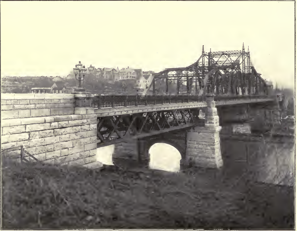
FIG. 15. SHIP CANAL BRIDGE OVER THE HARLEM RIVER.
