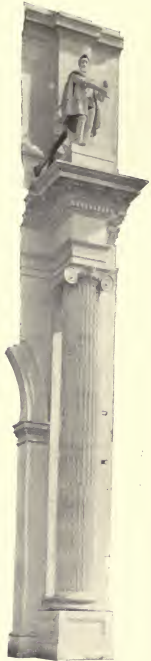
FIG. 12. A COLUMN OF THE MAIN ENTRANCE. D. H. Burnham & Co., Architects.
