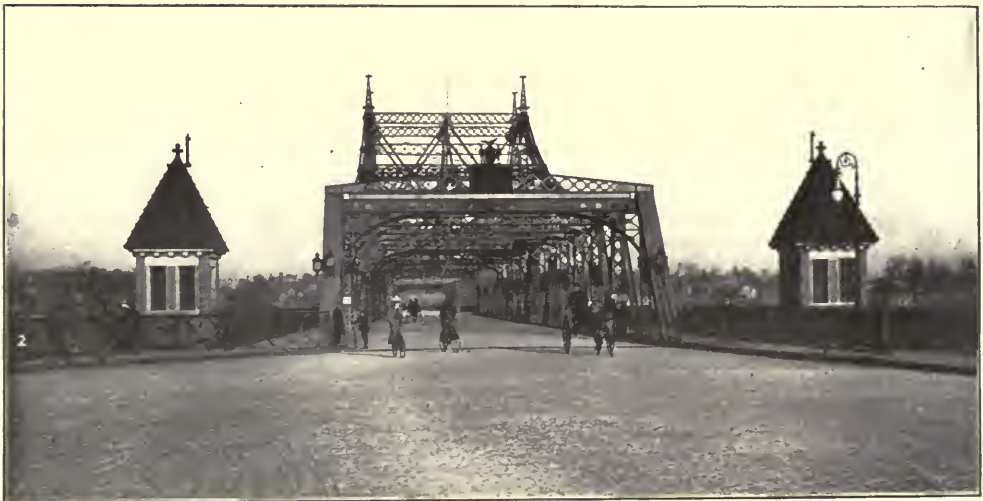
FIG. 13. ROADWAY OF THE CENTRAL BRIDGE.
