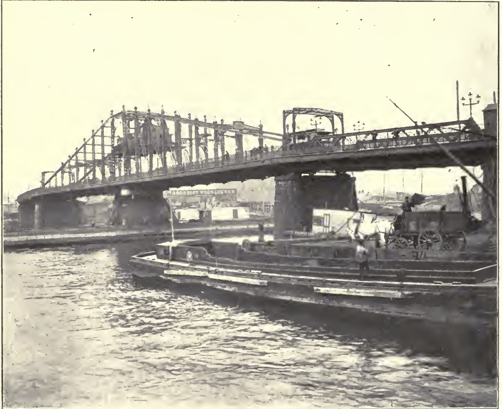
FIG. 3. THE BRIDGE AT MADISON AVE.
