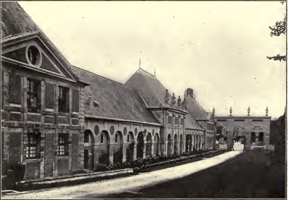
FIG. 11. OUTBUILDINGS TO THE RIGHT OF THE ENTRANCE TO THE CHATEAU.
