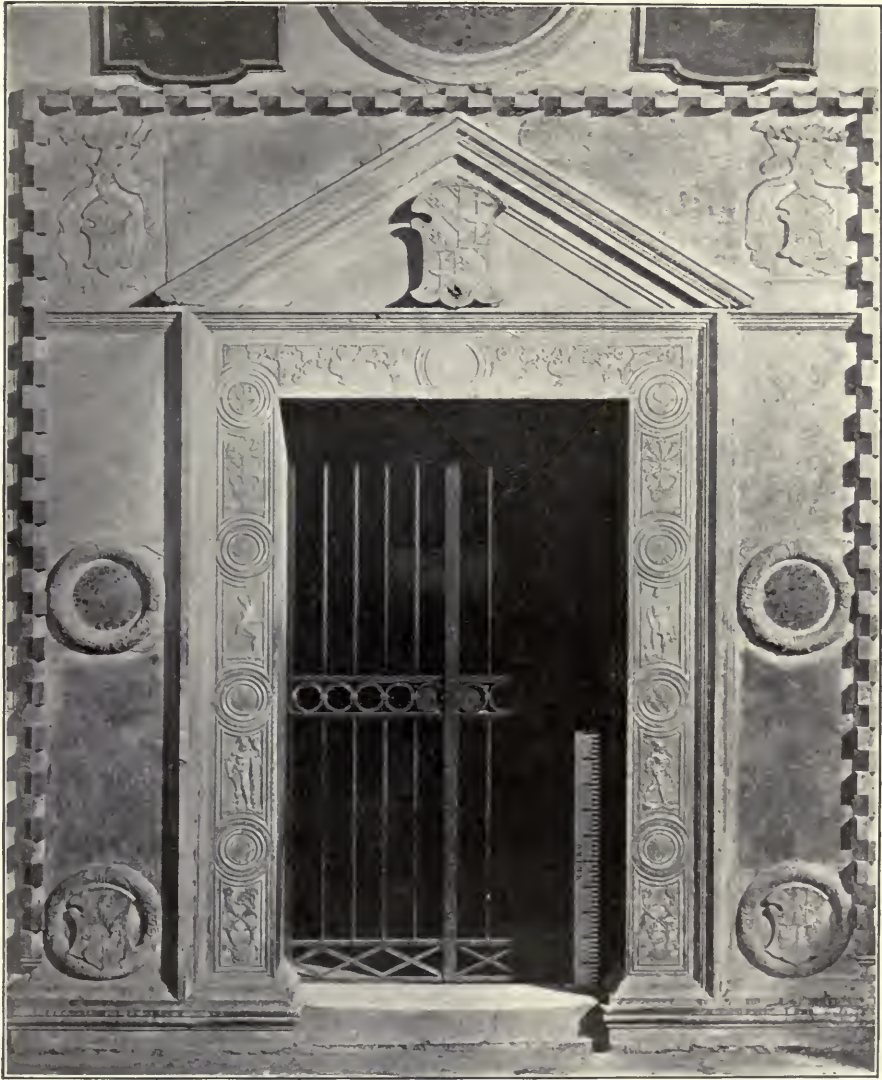
FIG. 9.—AN INTERIOR DOORWAY.
