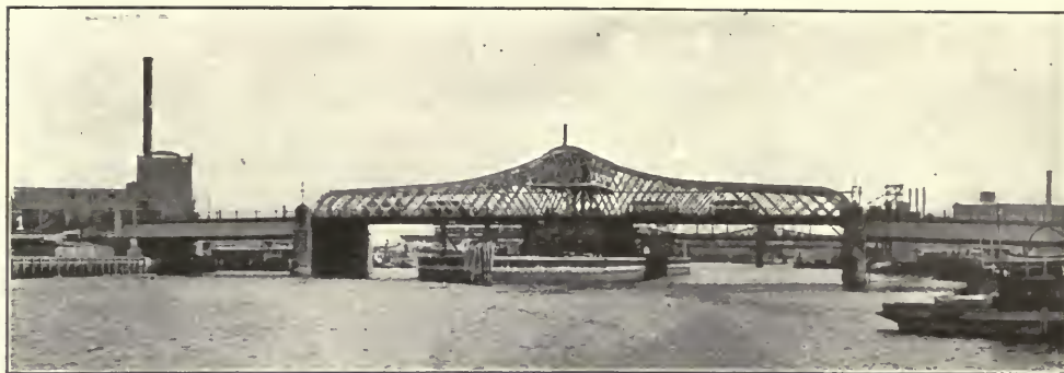
FIG. 4. THE THIRD AVE. BRIDGE.
