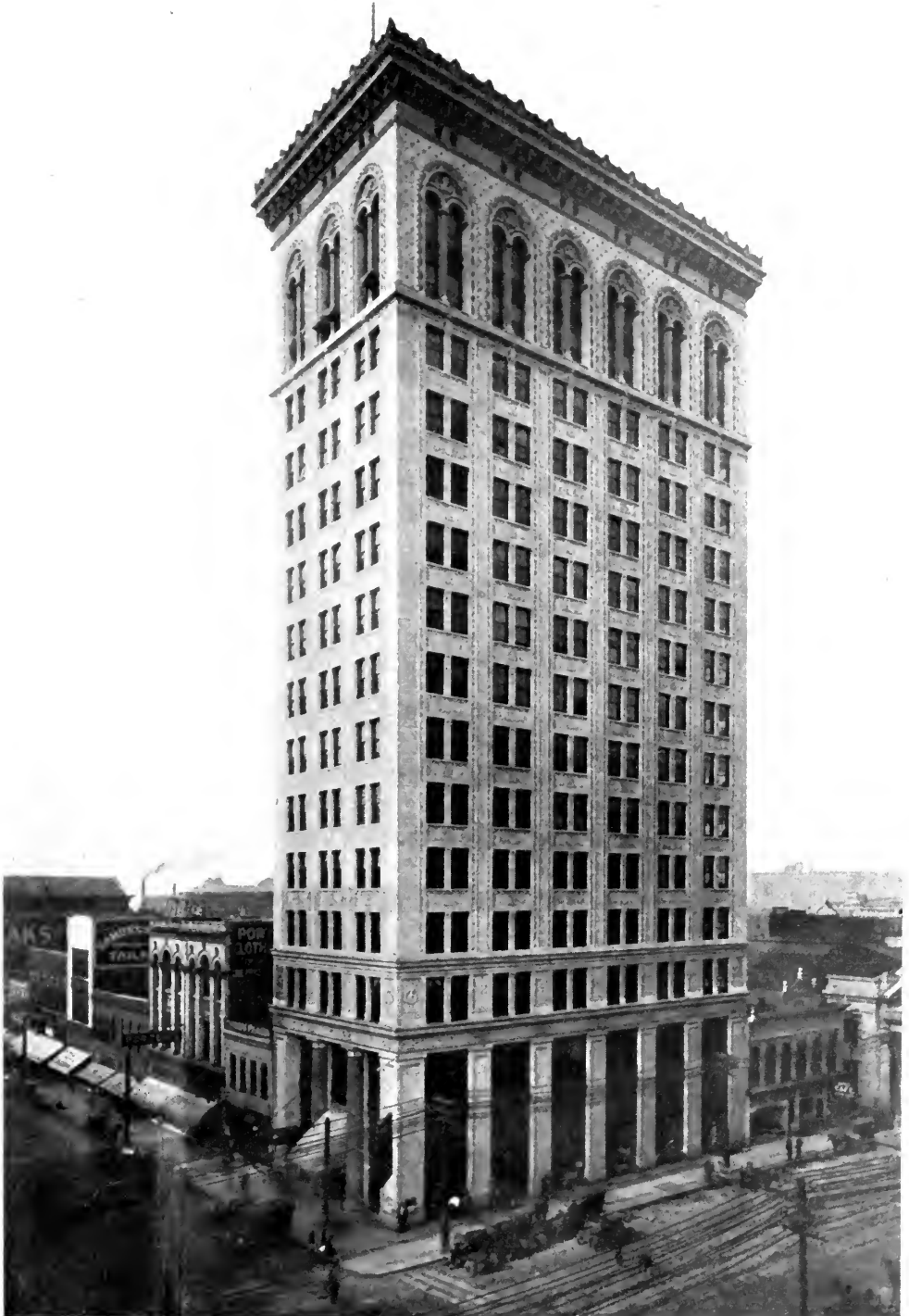
THE EMPIRE BUILDING, BIRMINGHAM, ALA. J. E. R. Carpenter, } Assoc. Archts. Walter D. Blair, } Warren & Welton, }
