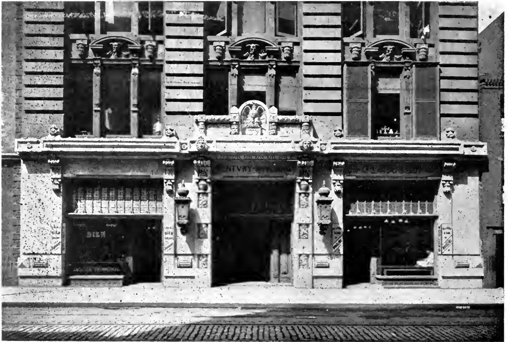
DETAIL OF LOWER STORIES OF THE TWELVE-STORY REINFORCED CONCRETE "CENTURY BUILDING."
