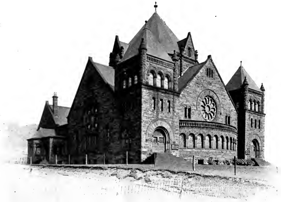
FIRST UNITED PRESBYTERIAN CHURCH. Thomas Boyd, Architect.
