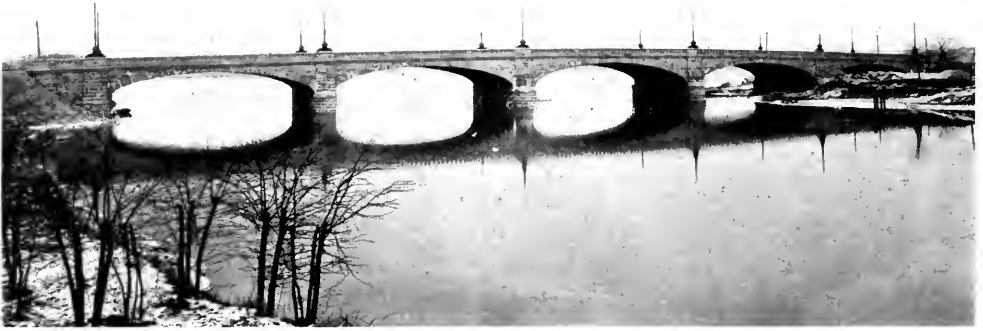
FIG. 1. BRIDGE OVER WHITE RIVER, MORRIS, INDIANAPOLIS.
