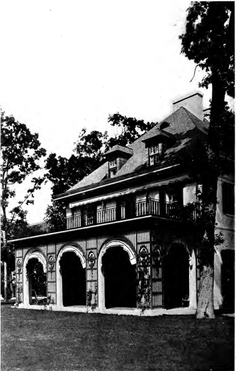
PORCH DETAIL. A HOUSE AT MOUNT KISCO, N. Y. DELANO AND ALDRICH, ARCHITECTS.
