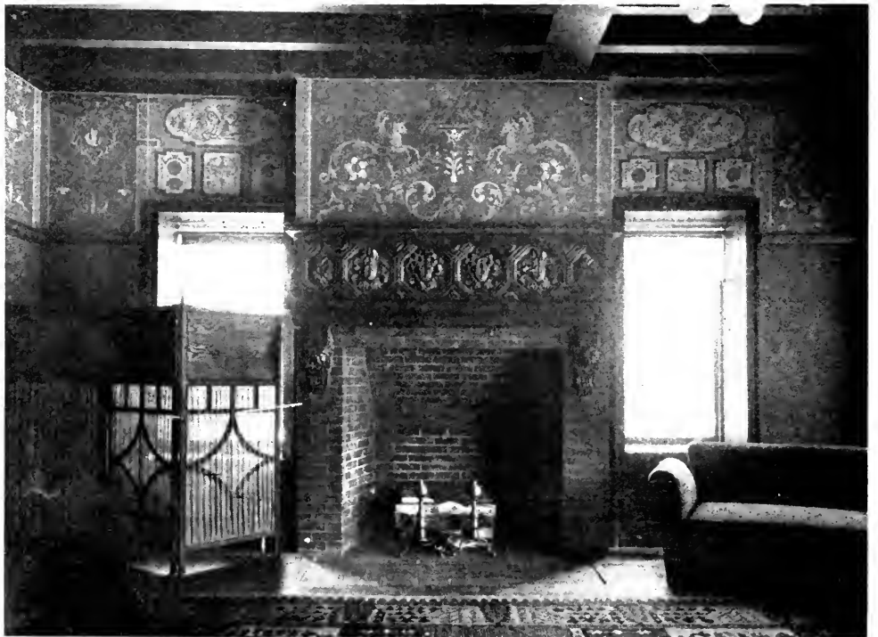
Mantel in Owner's Room.
