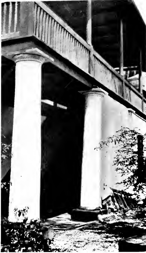
DETAIL OF COLONNADE HOUSE ON BAYOU ST. JOHN.
