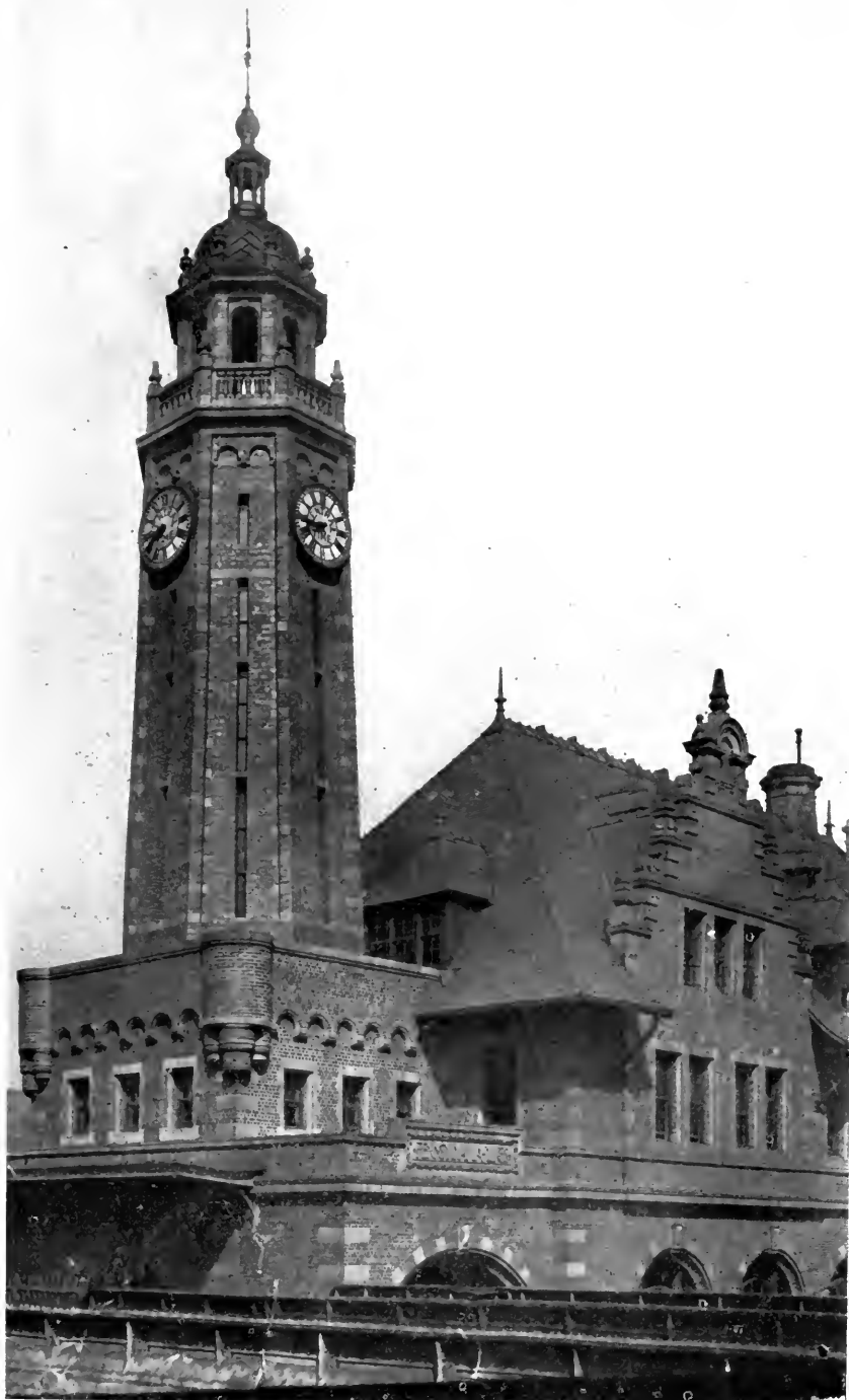
FORT WAYNE STATION, ALLEGHENY. Price and McLanahan, Architects.
