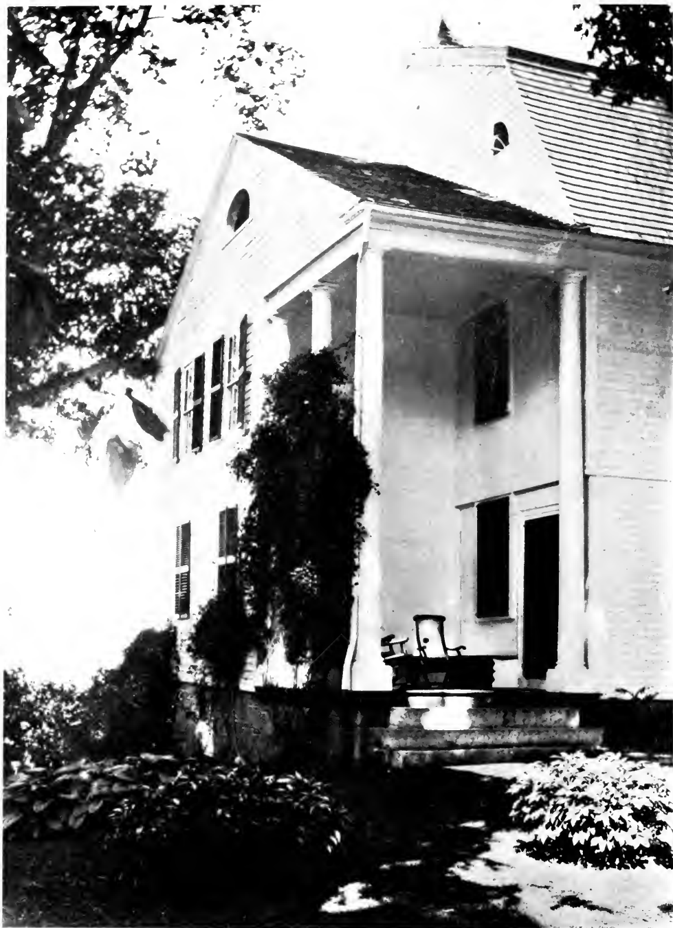
An unexcelled end treatment of a house and incidently of a doorway. It is in Litchfield and tradition has it that its owner, before building it, had visited Mt. Vernon. Vignola has been absolutely disregarded in proportioning the columns and the resulting delicacy is peculiarly appropriate to wood. The other end of the house has the same motif.
