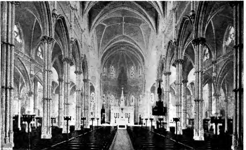
Interior (Showing Fine Aisles). SAINT PAUL'S (R. C.) CATHEDRAL. Egan & Prindeville, Architects.
