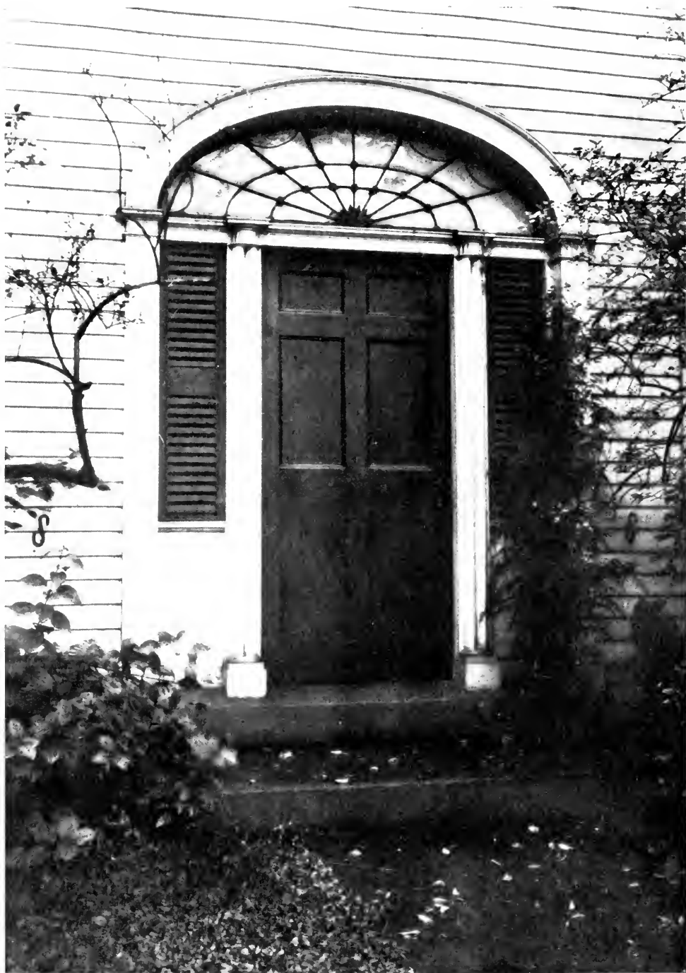
An unpretentious flat doorway on a Deerfield house. Its lines throughout, even to the leaded glass of the fan, are most pleasing; but its distinguishing feature is the engaged double colonnette each side of the door, with its two members egg-shaped, not round.
