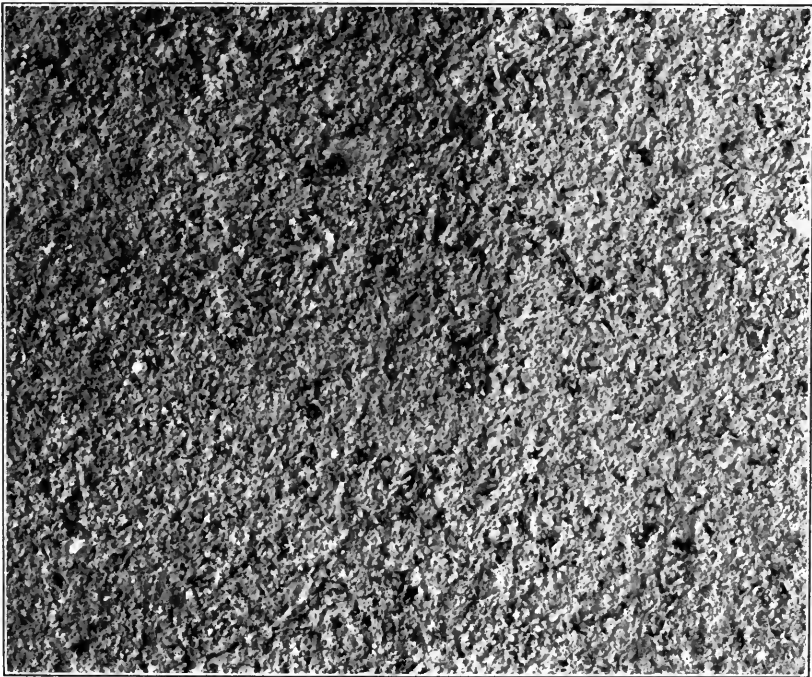
FIG. 8. SAND BLAST TREATMENT OF CONCRETE SURFACE.
