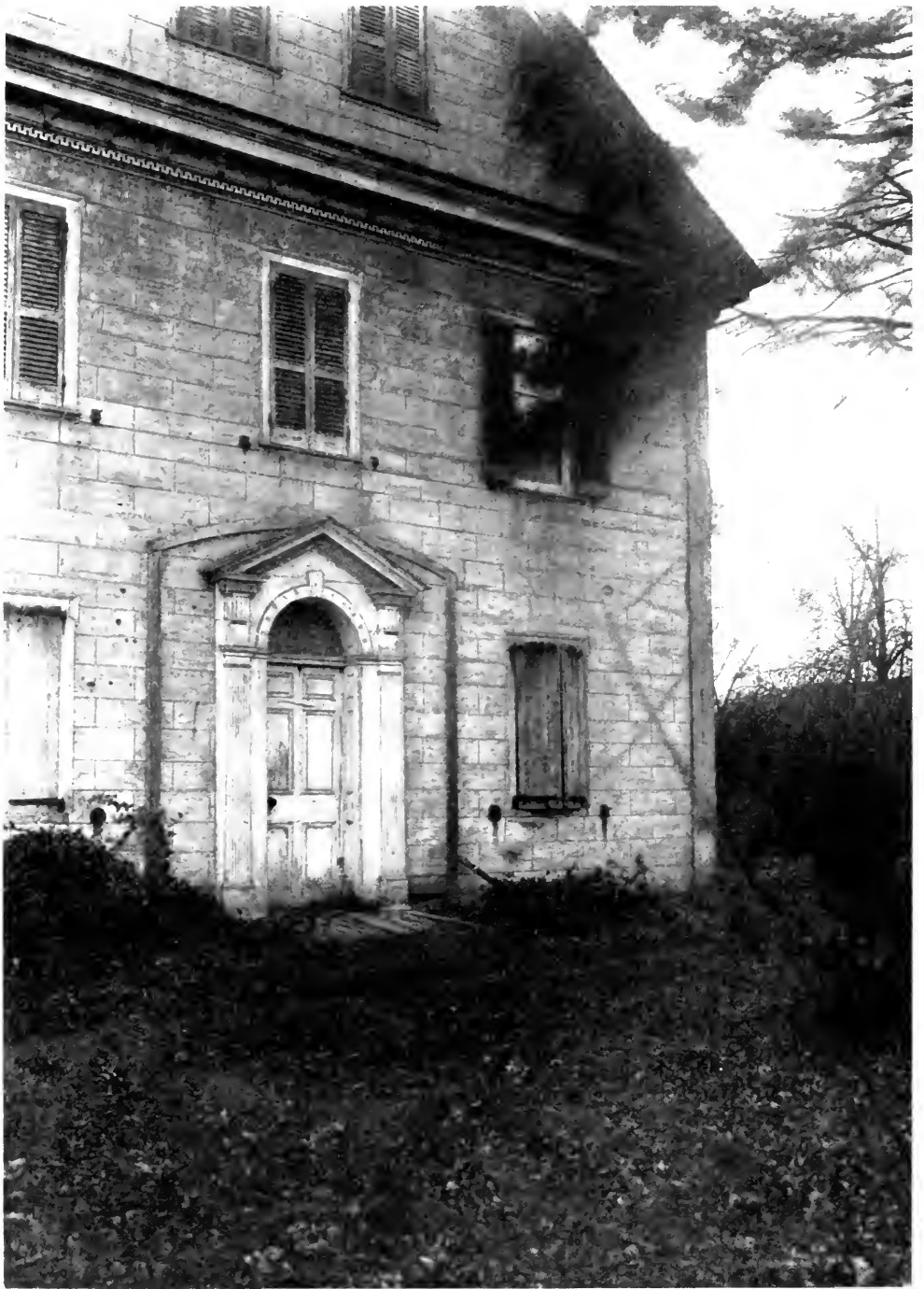
DOORWAY OF A WOODEN HOUSE NEAR DOUGLASVILLE, PA., ALMOST FALLEN TO DECAY—THE WOODEN WALLS WERE BUILT IN THE MANNER OF CUT-STONE WORK—THE REMAINS OF AN ARBOR ARE STILL SEEN AROUND DOORWAY.
