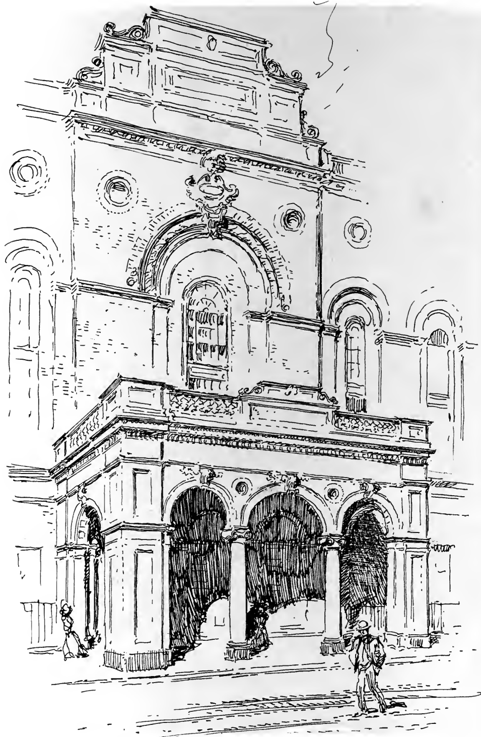
PORTE-COCHERE—MADISON SQUARE GARDEN. Fourth Avenue Façade. New York City
