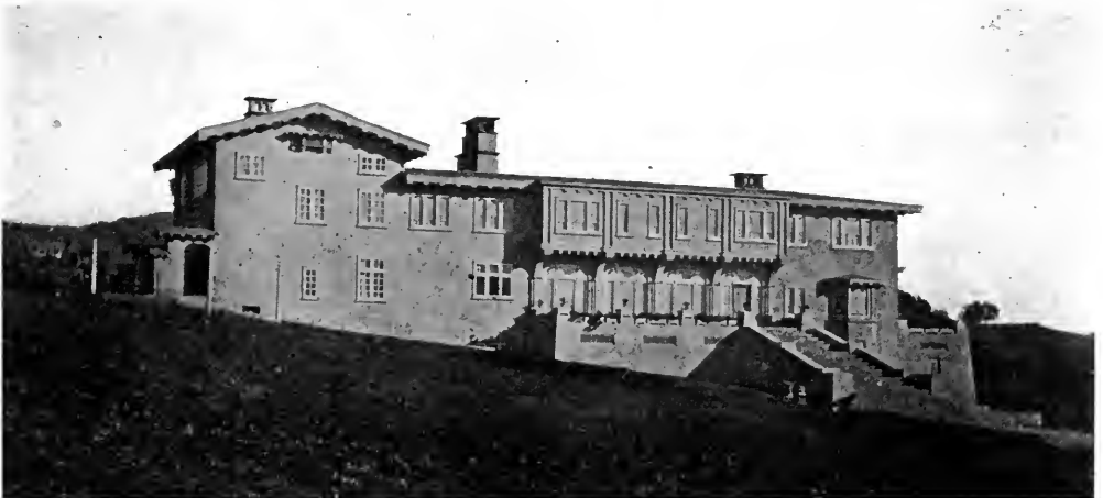
RESIDENCE AT PIEDMONT, CALIFORNIA.
