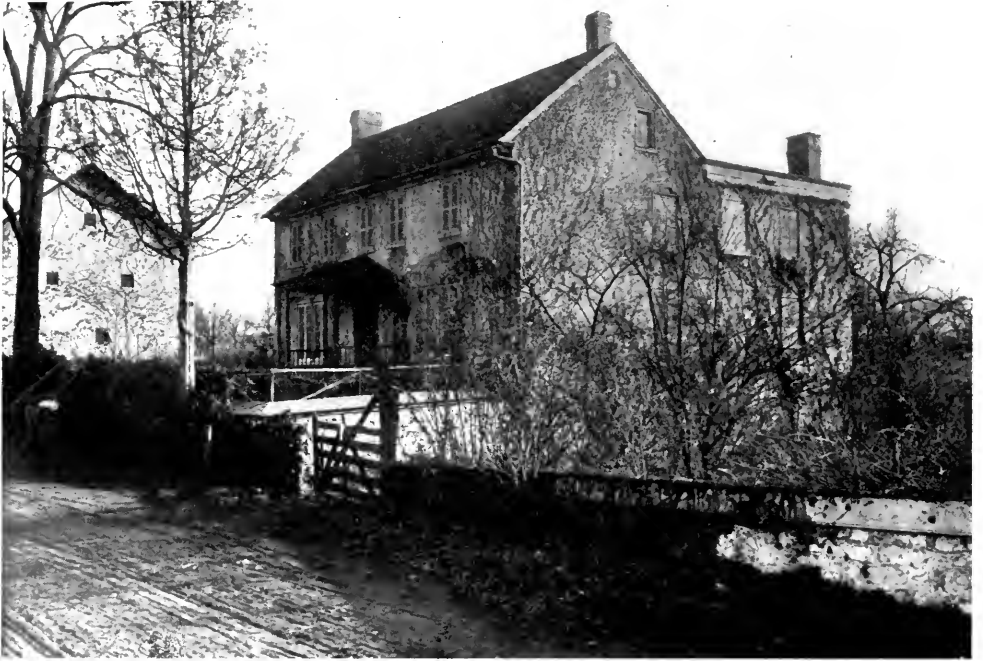
A STUCCO COVERED STONE HOUSE IN CHESTER COUNTY, PA—THE MARBLE SLAB IN THE GABLE END BEARS THE DATE 1810.
