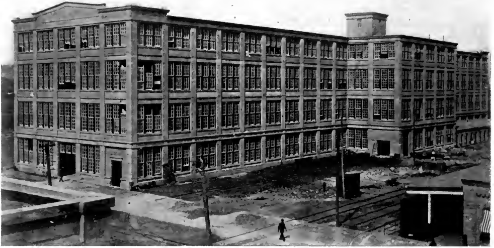
FIG. 4. A REINFORCED CONCRETE FACTORY BUILDING.
