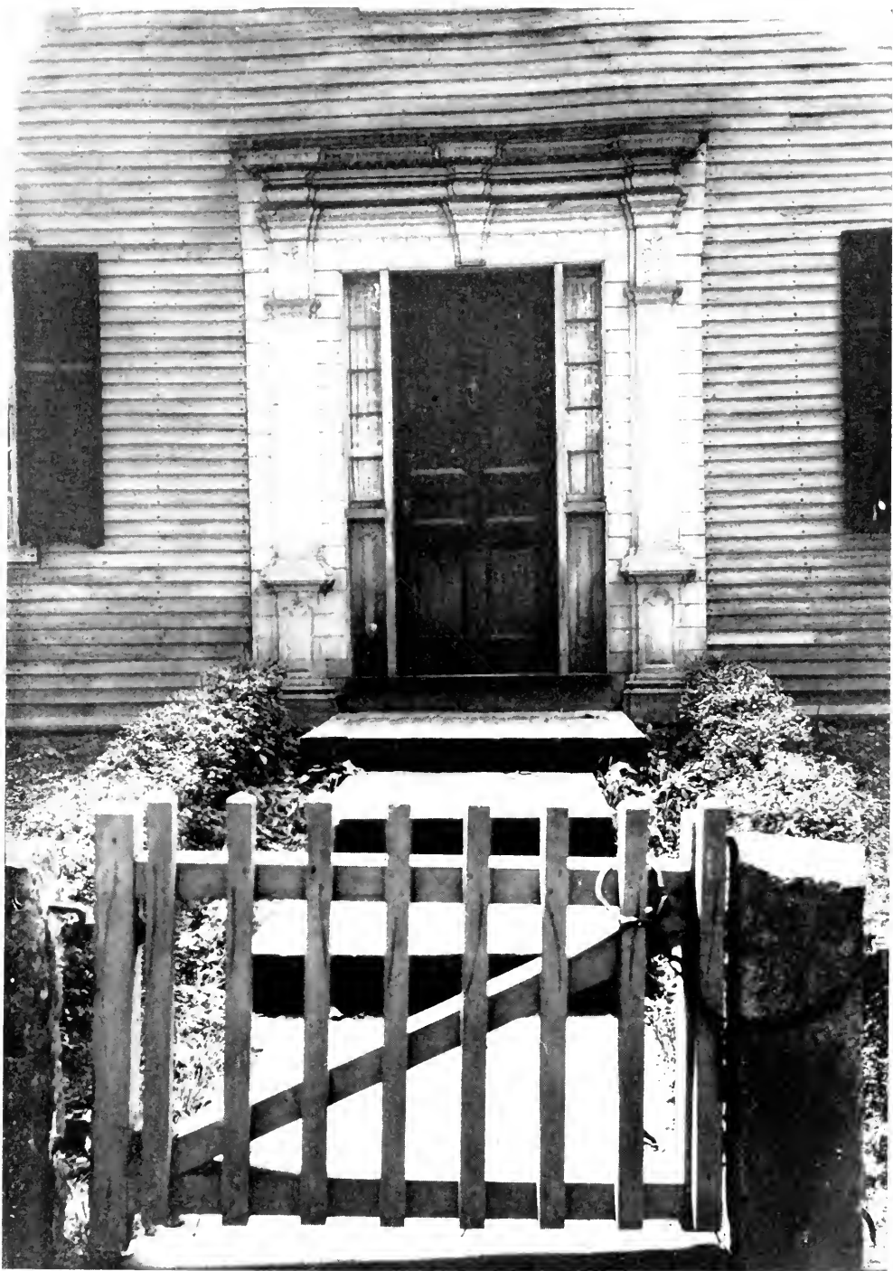
A Deerfield example that is a literal copy in wood of a Georgian stone doorway. Made before Colonial Woodworkers had learned the more graceful and more delicate possibilities of their material; in fact it is early enough to still show a trace of Gothic feeling in the lower panels. It is interpreted with as much naivety and innocence of classic proportions as was its prototype interpreted from the Italian Renaissance. Although of the same date as the house, the door was not built in situ but was ordered separately from some skilled workman and set up intact in the opening left for it.
