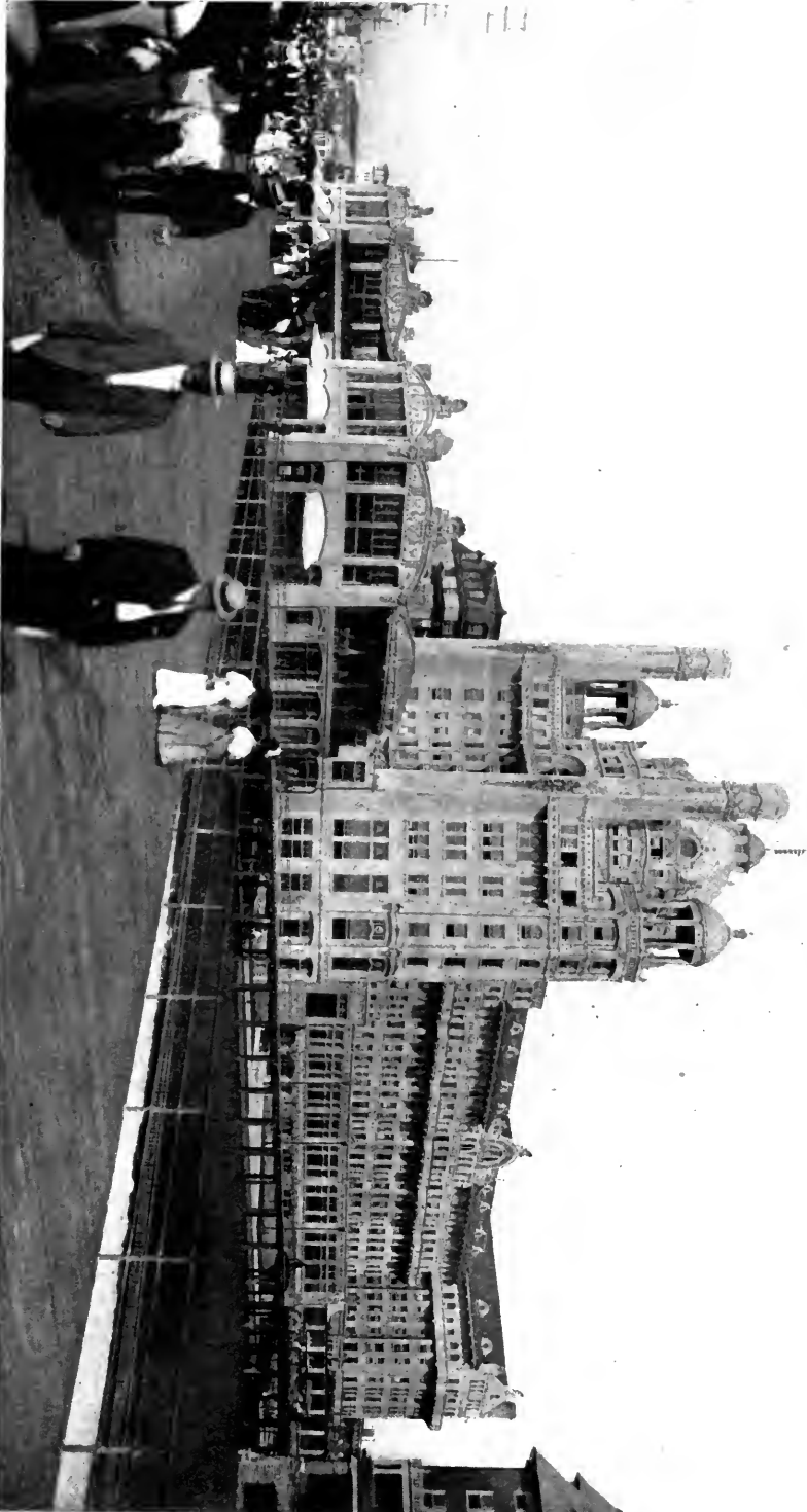
FIG. 12 — THE MARLBOROUGH-BLENHEIM HOTEL, ATLANTIC CITY, N. J.—CONCRETE DECORATED WITH INLAID COLOURED TILES
