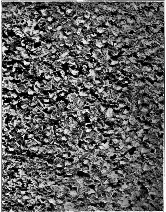
FIG. 10. SURFACE FINISHED BY PNEUMATIC HAMMER.
