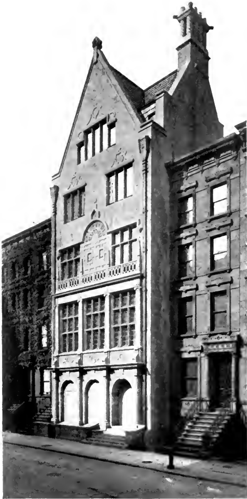
FIG. 6.—NO. 57 EAST 55TH STREET. Taylor & Levy, Architects.
