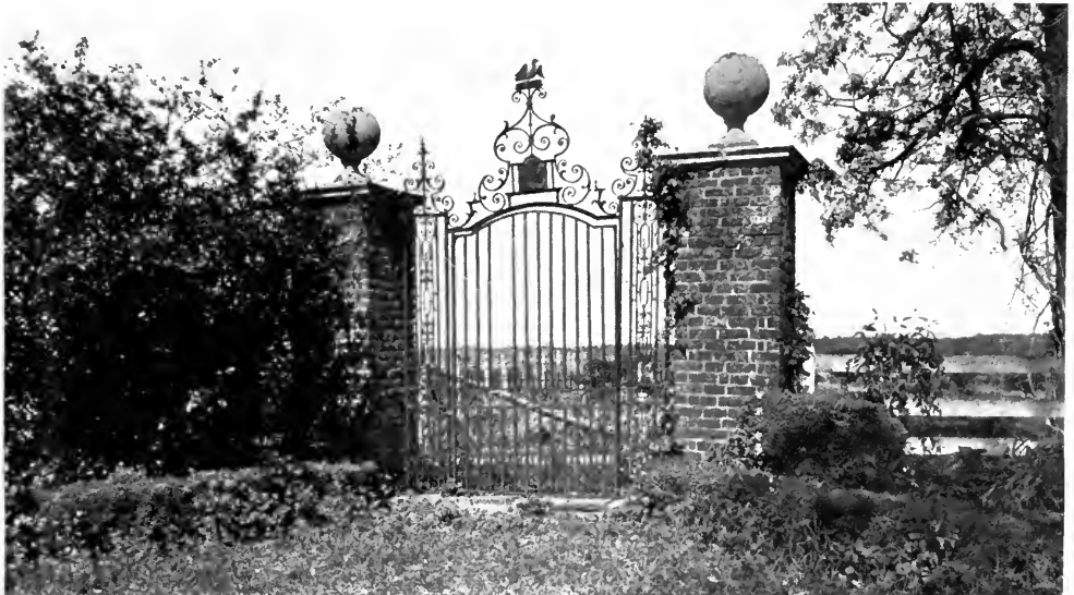
EAST GATE—"WESTOVER," VIRGINIA.
