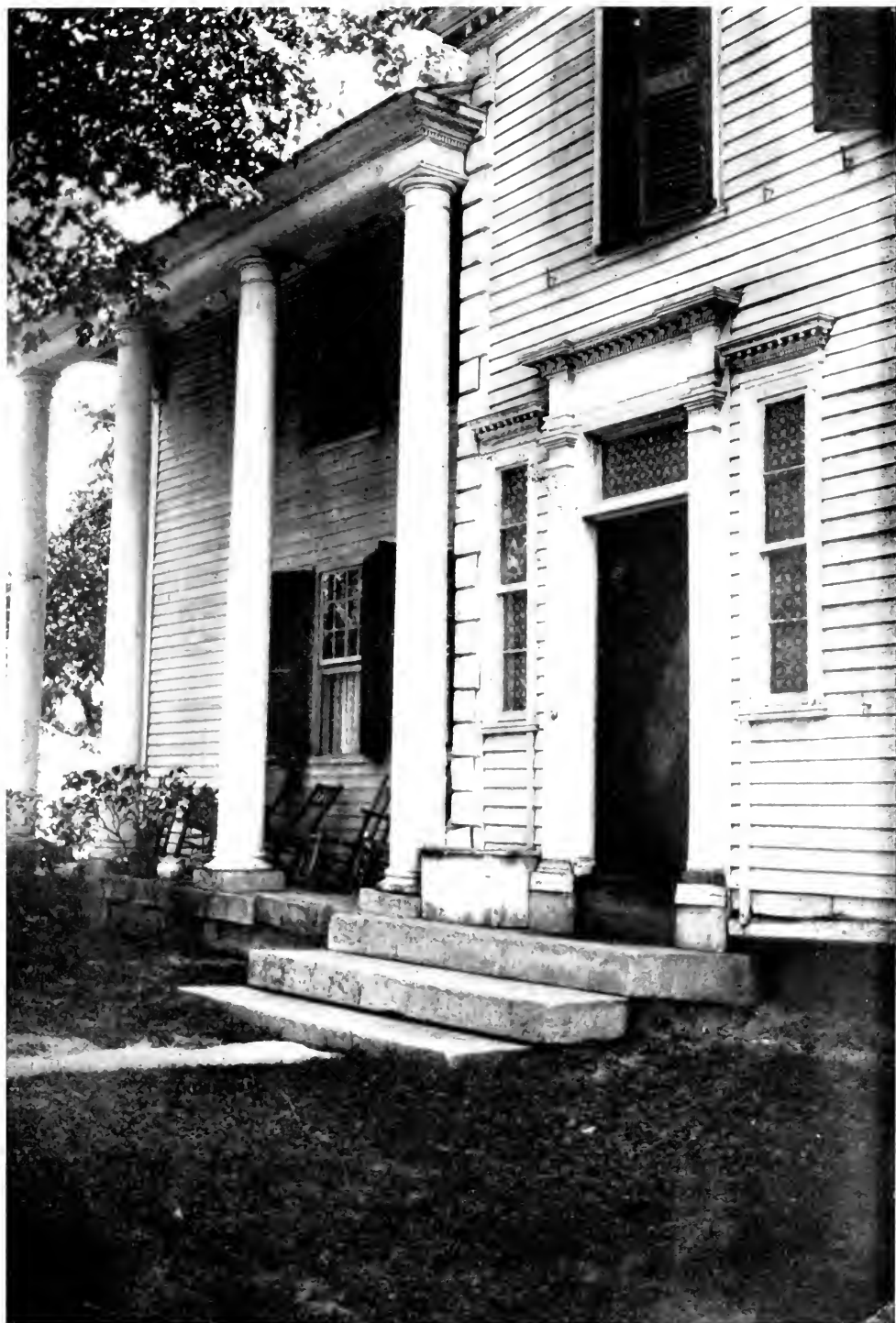
A doorway whose every detail is admirable; yet whose most salient appeal is the perfect relationship it maintains with the columnar portico beyond. This fine old Litchfield house, built in 1792, is unfortunately being allowed to fall into ruin.
