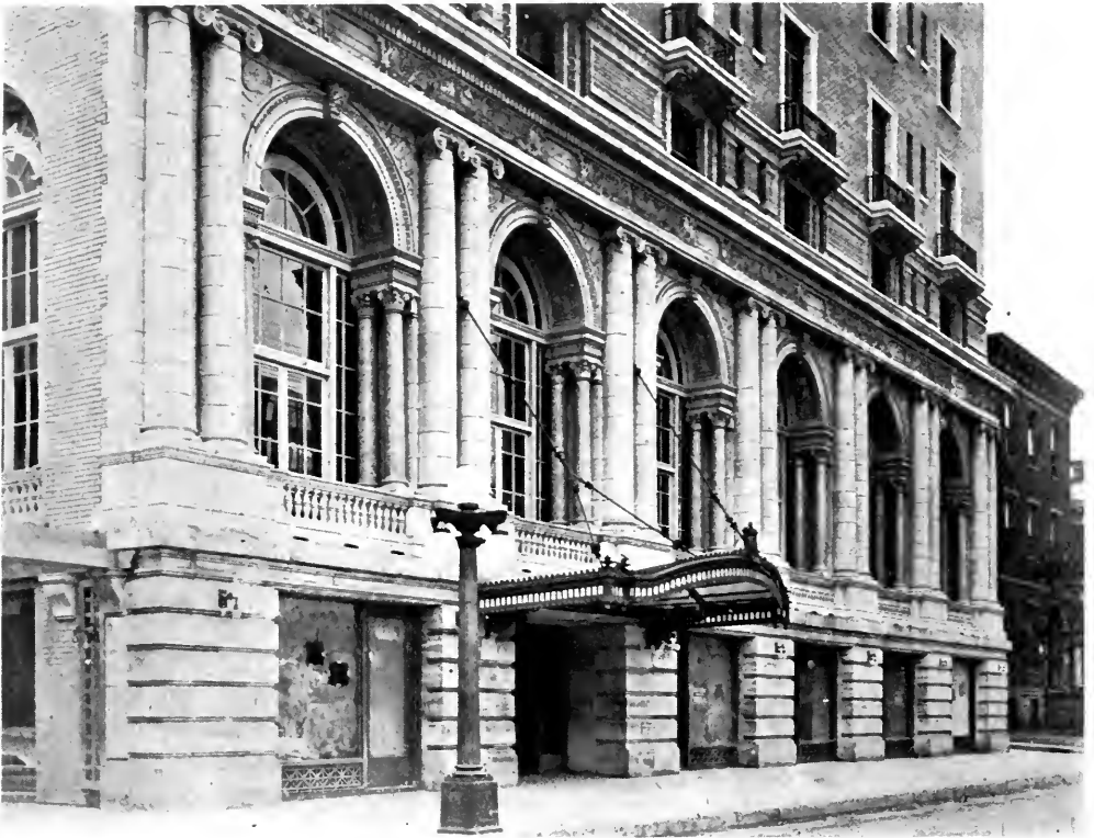
LOWER STORY DETAIL—THE HERMITAGE HOTEL.
