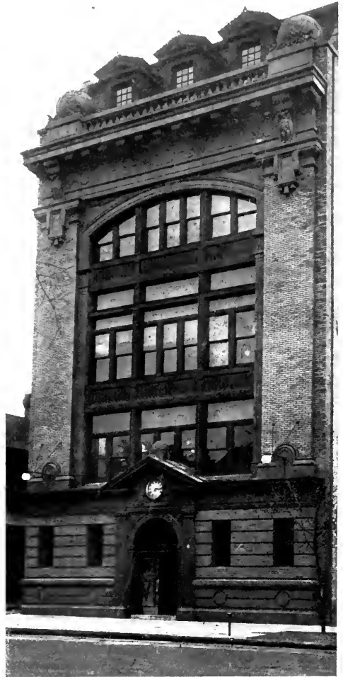
THE AGE HERALD NEWSPAPER BUILDING. Birmingham, Ala. Wm. C. Weston, Architect.
