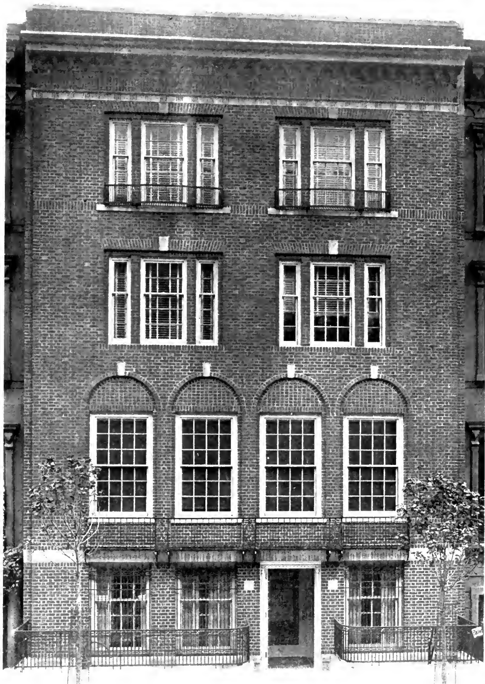
FIG. 12.—NO. 121 EAST 62D STREET, N. Y. CITY. Grosvenor Atterbury, Architect.
