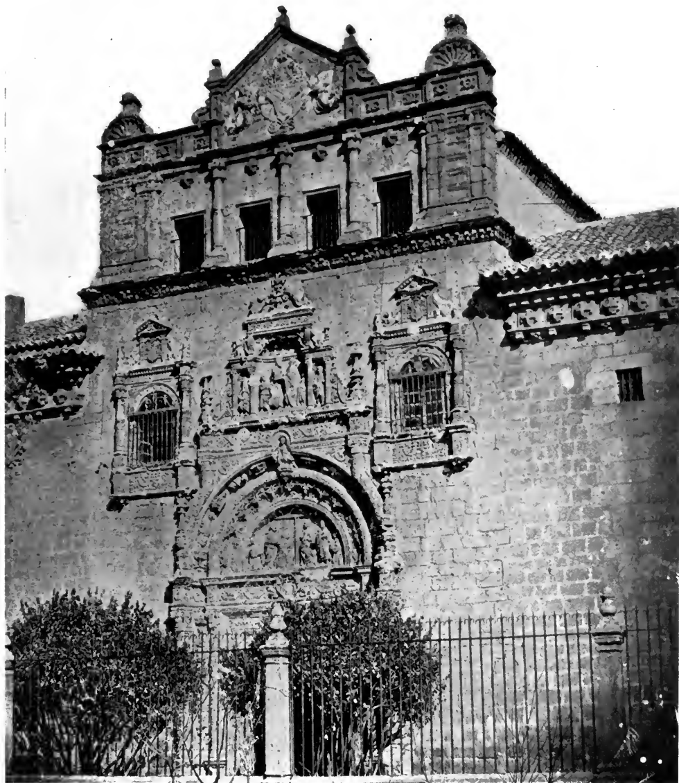
PORTAL OF CARDINAL MENDOZA'S HOSPITAL OF THE HOLY CROSS.
