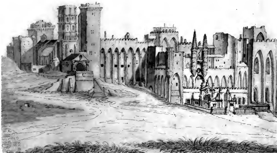
AN EIGHTEENTH CENTURY DRAWING IN THE MUSÉE CALVET AT AVIGNON, SHOWING THE TWO TURRETS OVER ENTRANCE AND THE RAVELIN BUILT BY THE PAPAL LEGATE COLONNA—ARCHITECTURAL FEATURES WHICH NO LONGER EXIST.
