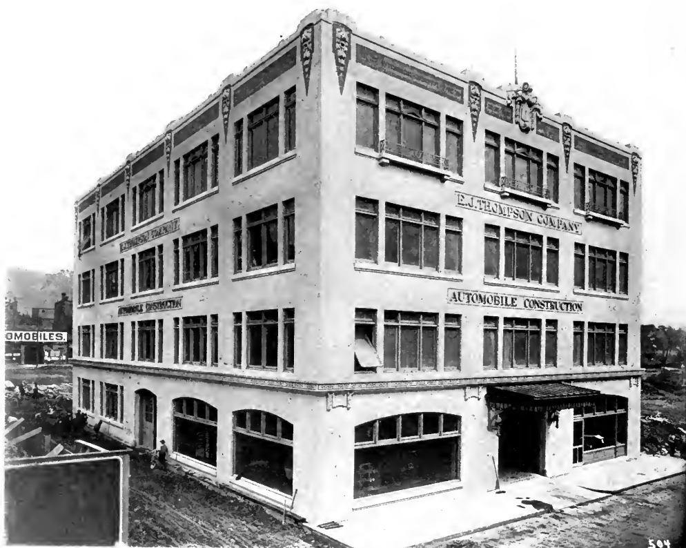
REINFORCED CONCRETE GARAGE, Rutan & Russell, Architects.
