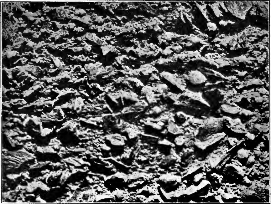
FIG. 11. TRAP ROCK AGGREGATE WITH BRUSH OR SCRUBBED WORK TREATMENT.
