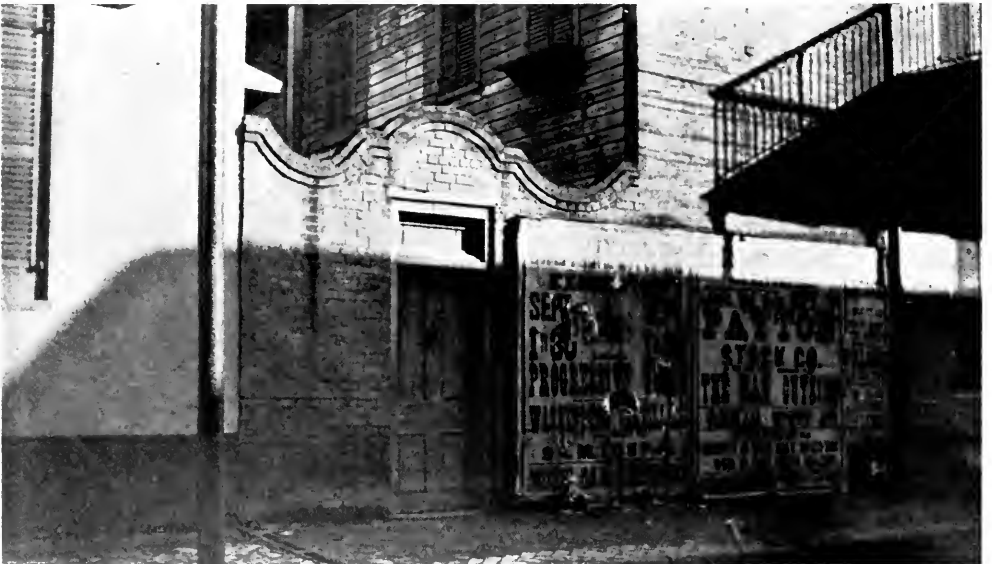
A COURTYARD ENTRANCE.
