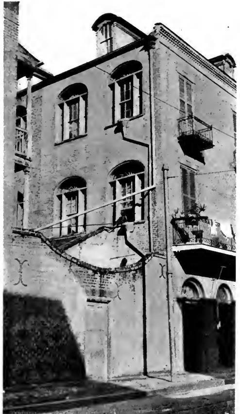
A COURTYARD ENTRANCE.
