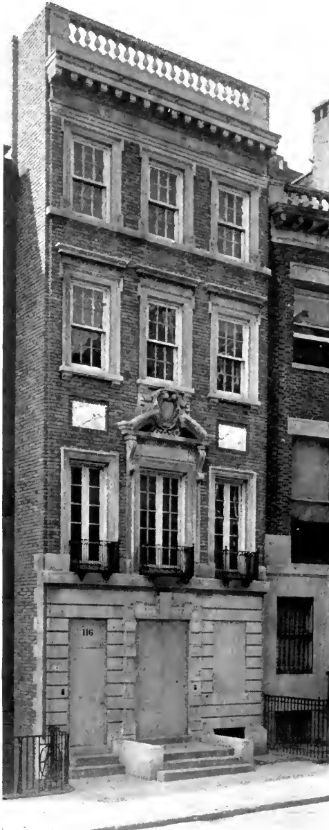
FIG. 5.—NO. 116 EAST 78TH STREET. Rouse & Goldstone, Architects.
