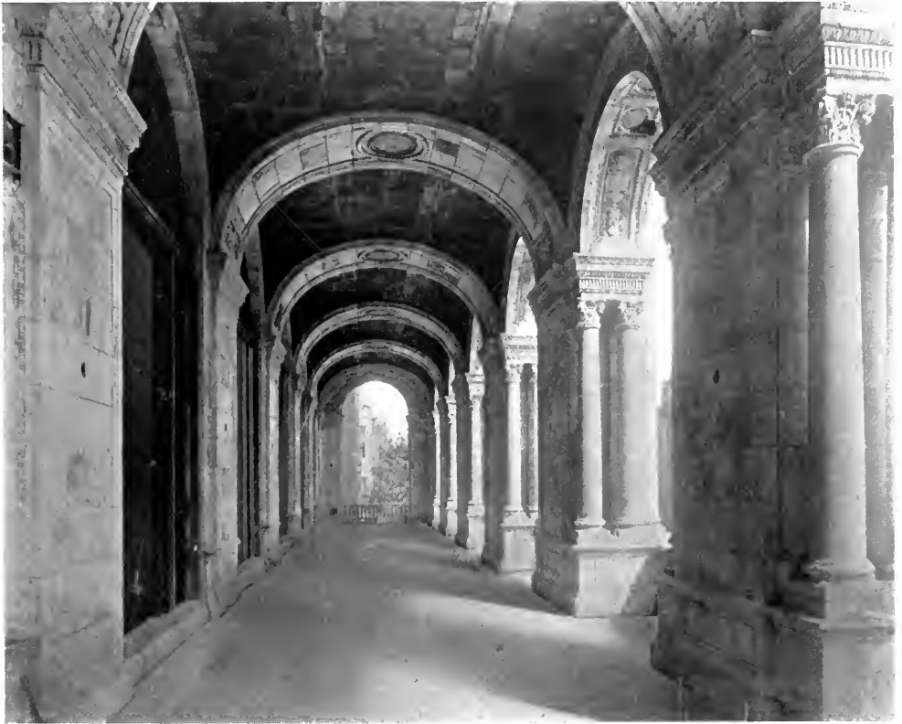
LOGGIA DETAIL—THE HERMITAGE HOTEL.
