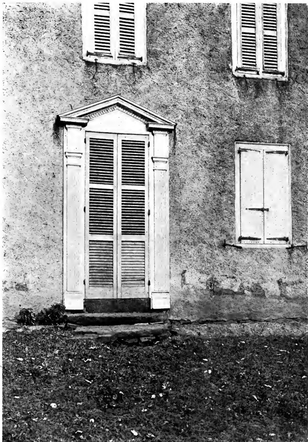
DOORWAY DETAIL OF THE STUCCO-COVERED STONE HOUSE NEAR GLASGOW—WOOD STEPS OR AN ENTRANCE PORCH PROBABLY WERE INCORPORATED IN THE DESIGN BUT HAVE GIVEN PLACE TO THE ROUGH STONE STEPS.
