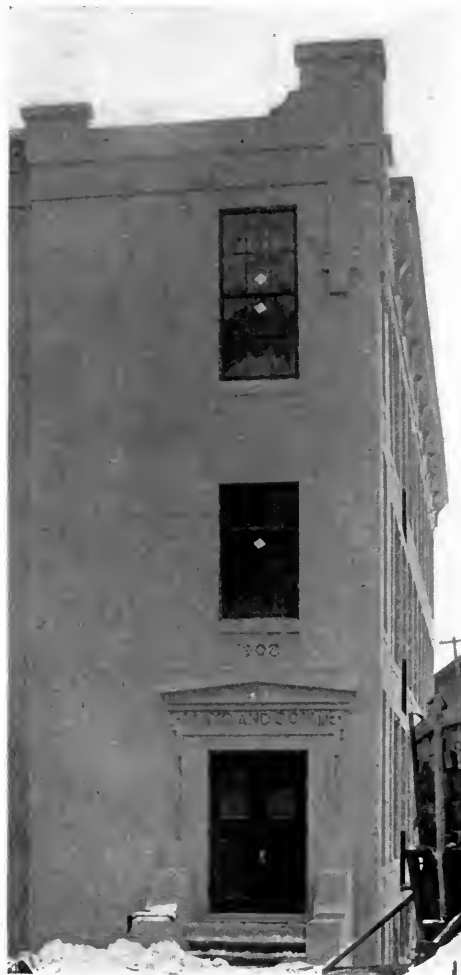
FIG. 6. SKILFUL TREATMENT OF A CONCRETE CORNICE.
