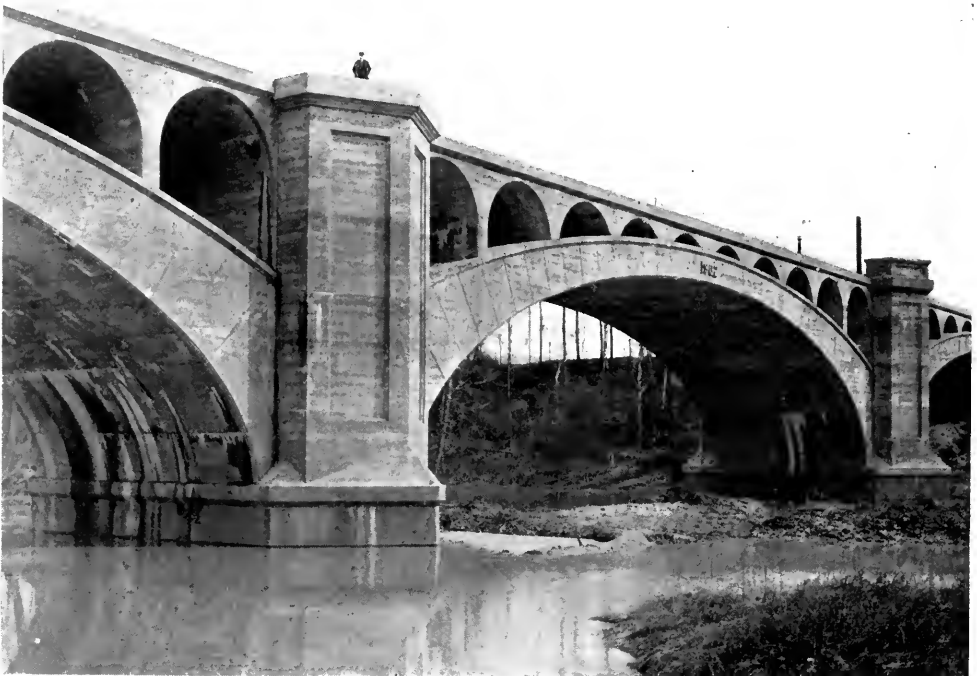
FIG. 2. I. C. R. R. BRIDGE OVER BIG MUDDY RIVER, CARBONDALE, ILLS.
