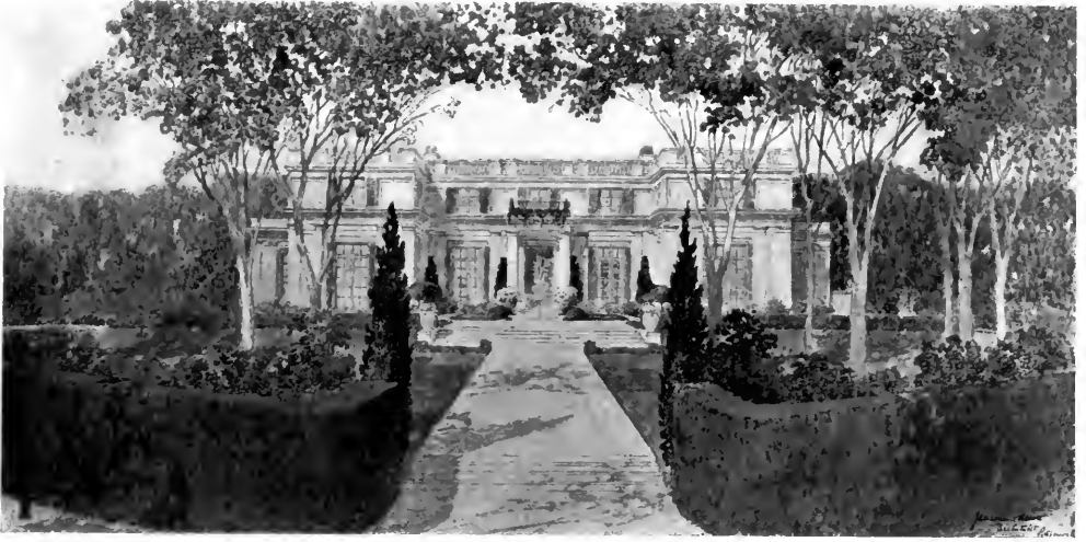
RESIDENCE OF J. L. KENDALL, ESQ., WOODLAND ROAD. Janssen & Abbott, Architects.
