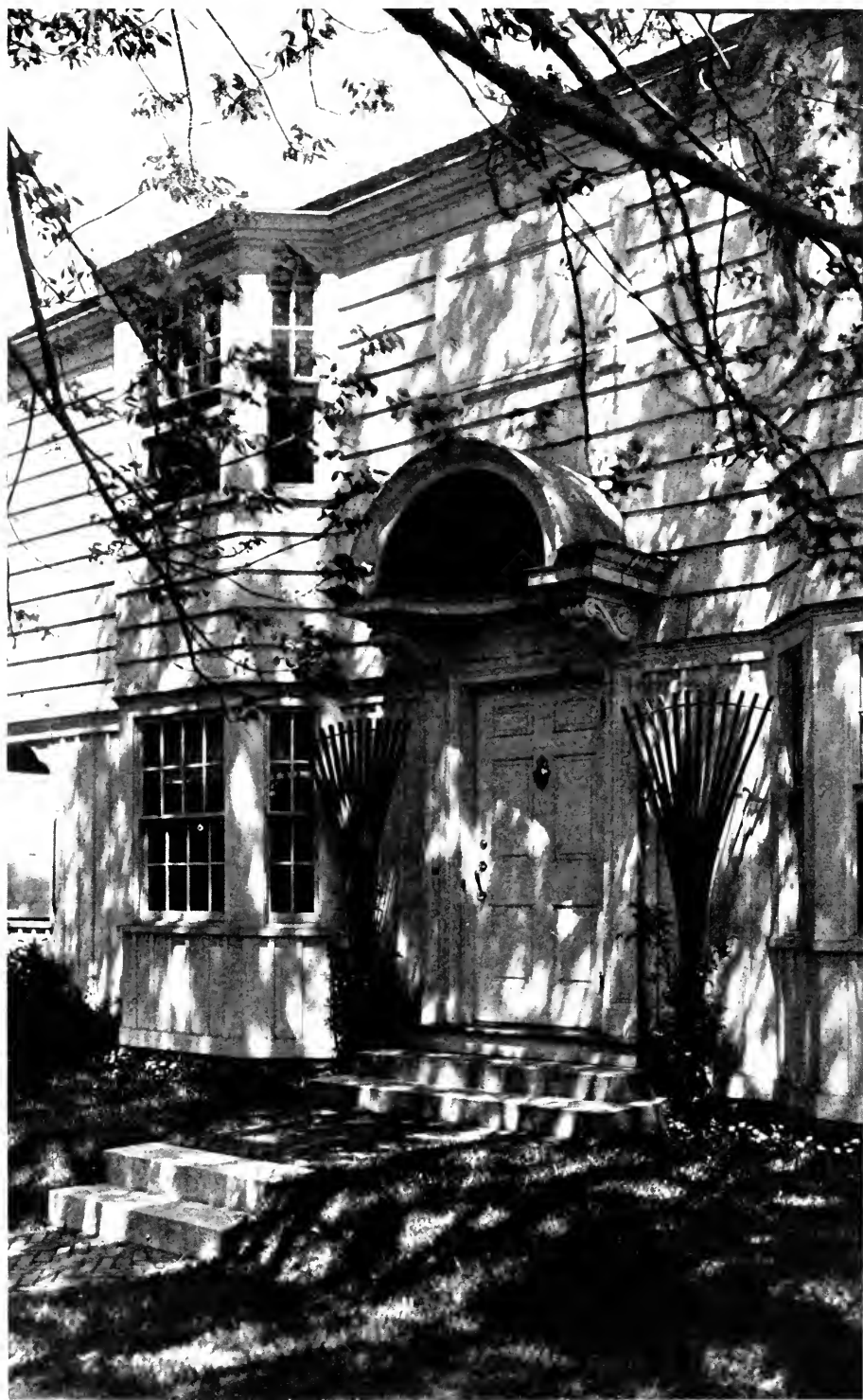
ENTRANCE DOOR—A COUNTRY COTTAGE. PARKER MORSE HOOPER, ARCHITECT.
