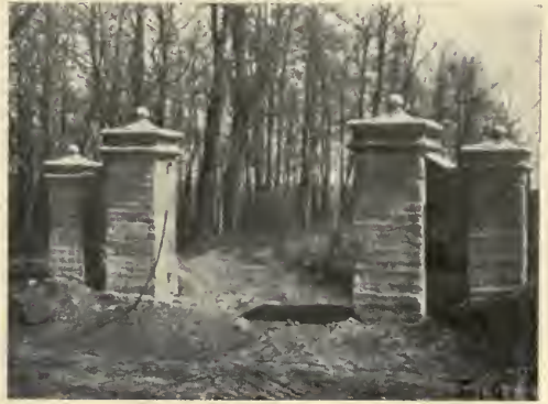
FIG. 8—CONCRETE USED FOR ENTRANCE, ROUGH FINISH.
