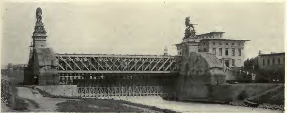
DAM AND GATES AT NUNDORF.
