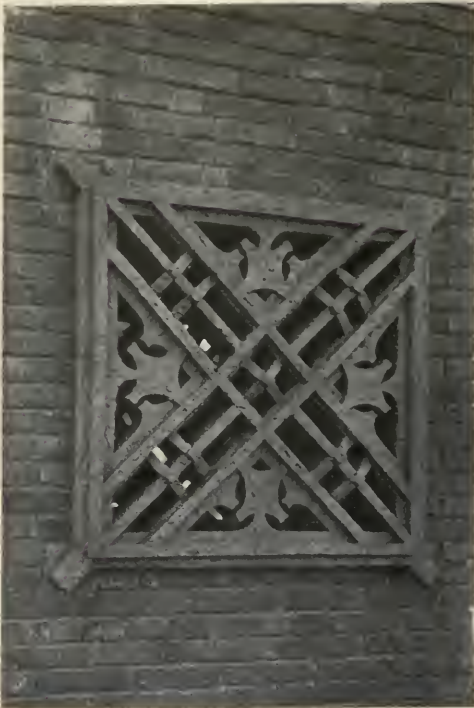
DETAIL OF CHIMNEY TOP—THE PEOPLE'S SAVINGS BANK. Louis H. Sullivan, Architect.
