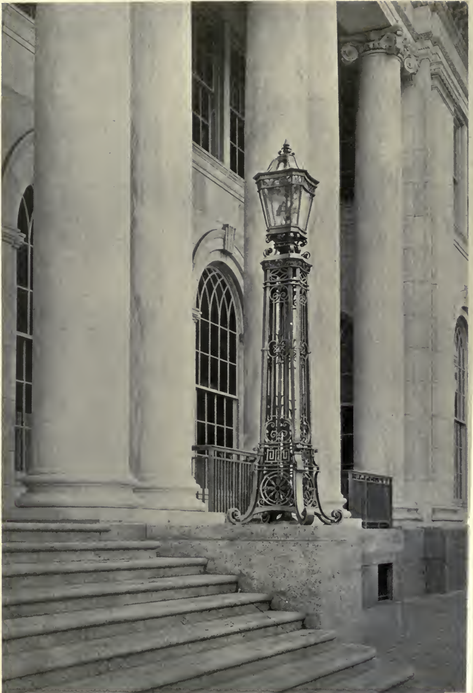
DETAIL OF MARBLE COLONNADE—THE HOME OF THE CURTIS PUBLISHING COMPANY, PHILADELPHIA, PA. EDGAR V. SEELER, ARCHITECT.
