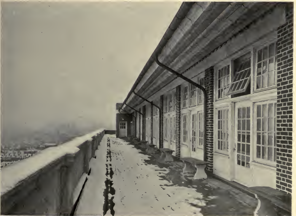
Terrace Outside Recreation Room.
