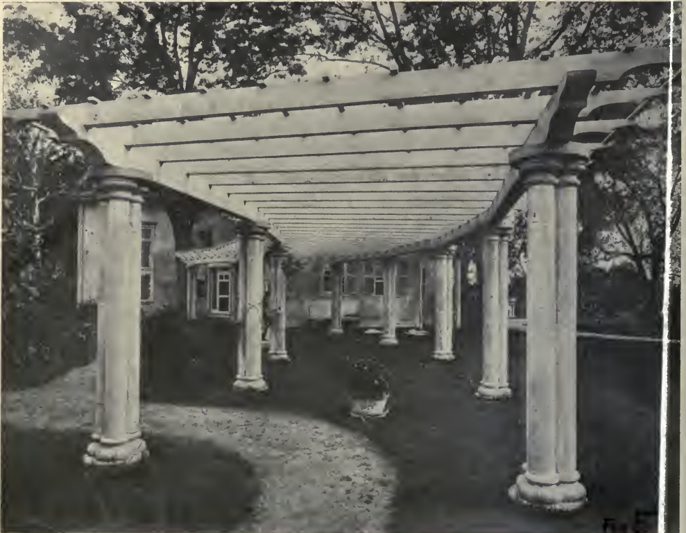
FIG. 5—GROUPED COLUMNS FOR THE PERGOLA.
