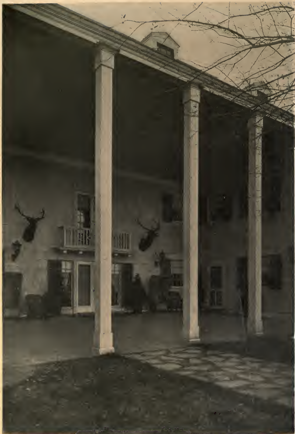
ENTRANCE DETAIL—COUNTRY SEAT OF ROBERT J. COLLIER, ESQ., WICKATUNK, N. J. JOHN RUSSELL POPE, ARCHITECT.
