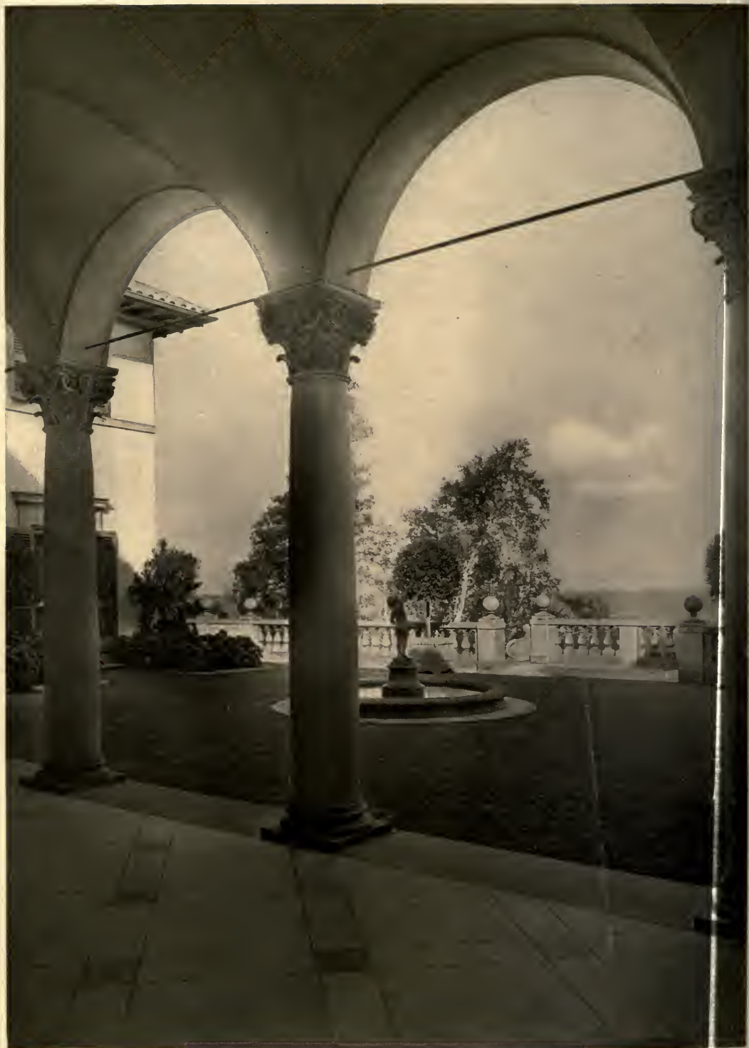
"THE LOGGIA"—HOUSE OF HAROLD F. McCORMICK, Esq. LAKE FOREST, ILL., CHAS. A. PLATT, ARCHITECT
