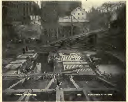
COFFERDAM AND FOUNDATION GRILLAGES.
