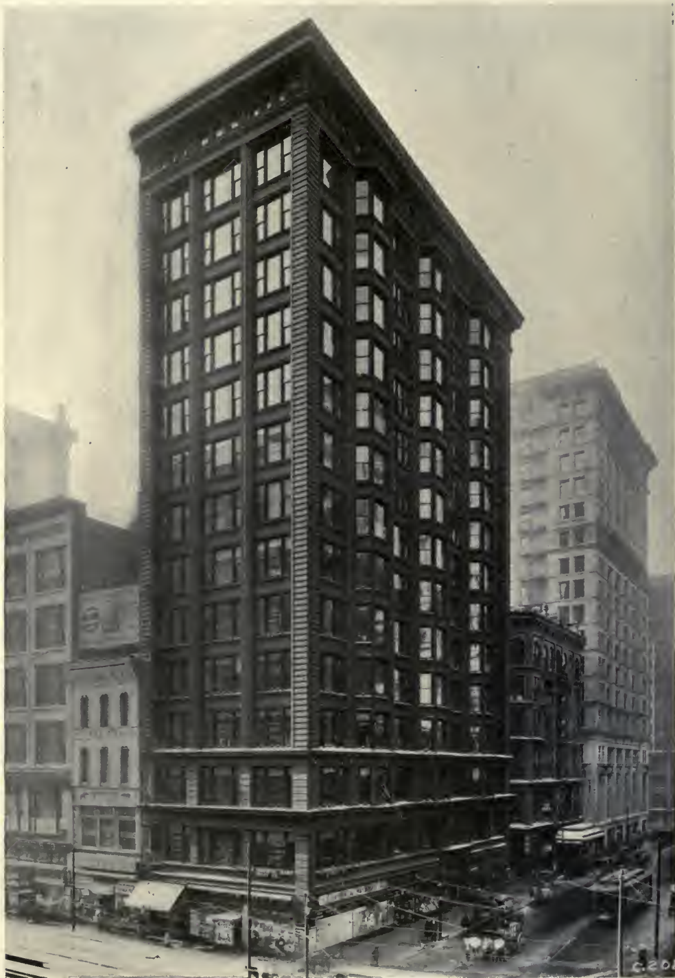
CHICAGO SAVINGS BANK BUILDING. HOLABIRD & ROCHE, ARCHITECTS.
