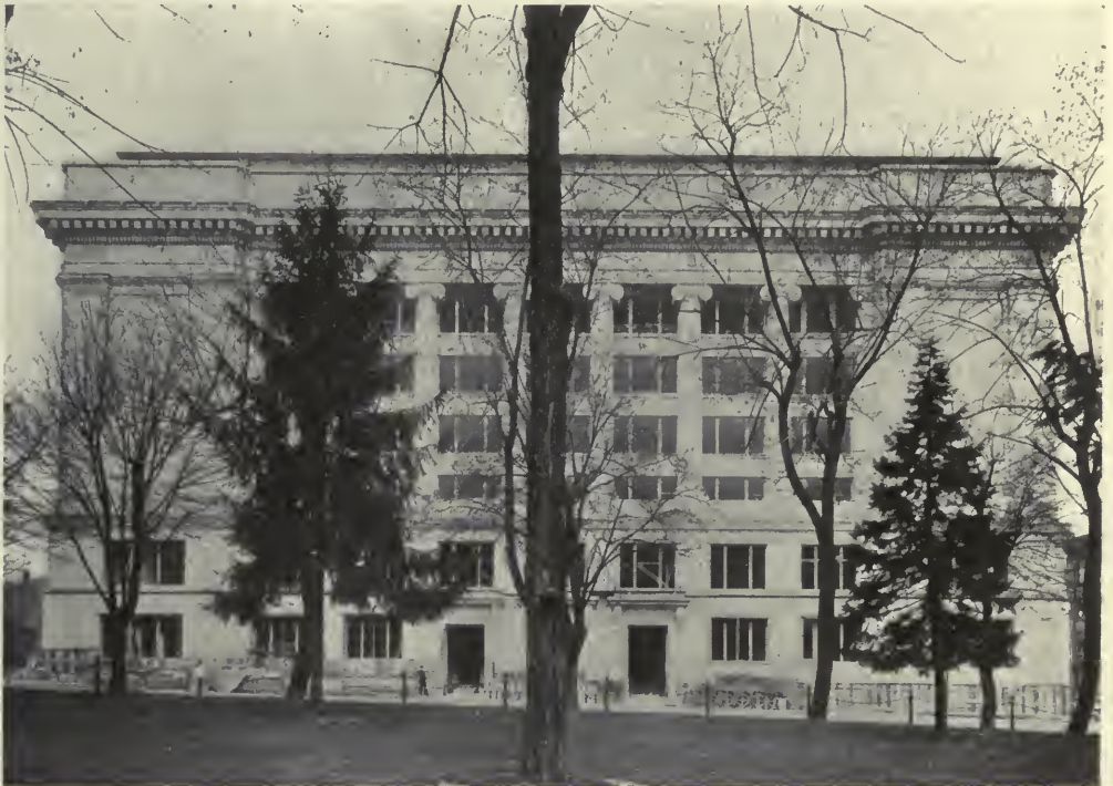
NEW COUNTY COURT HOUSE, PORTLAND, OREGON. Whidden & Lewis, Architects.
