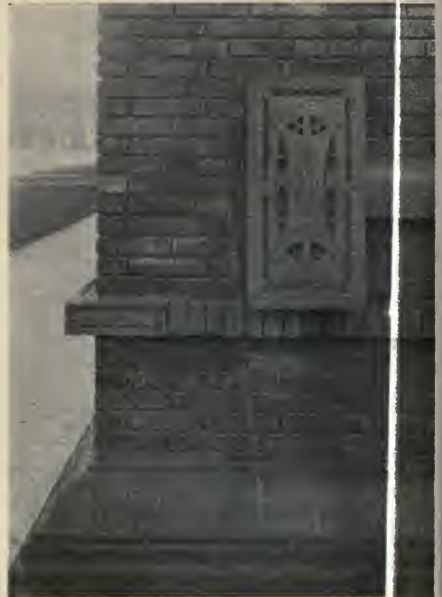
DETAIL—STOP OF SILL COURSE—THE PEOPLE'S SAVINGS BANK. Louis H. Sullivan, Architect.
