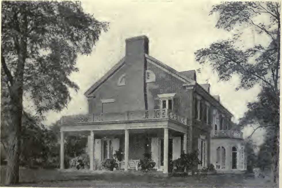
HOUSE AT PORT DEPOSIT, MARYLAND. Parker, Thomas & Rice, Architects.
