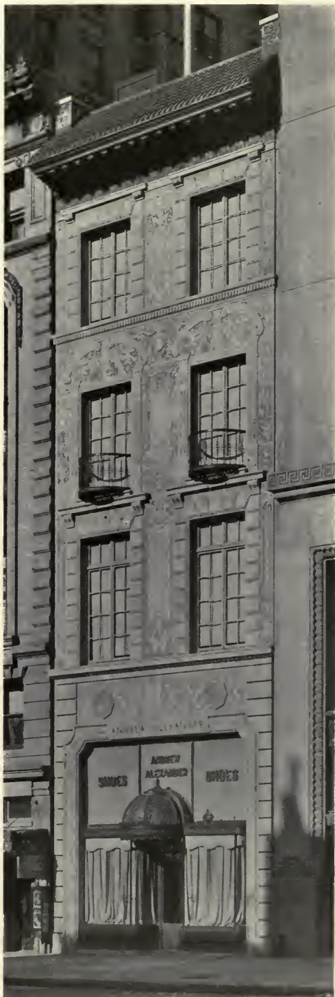
NO. 548 FIFTH AVENUE, N. Y. CITY. Carrère & Hastings, Architects.
