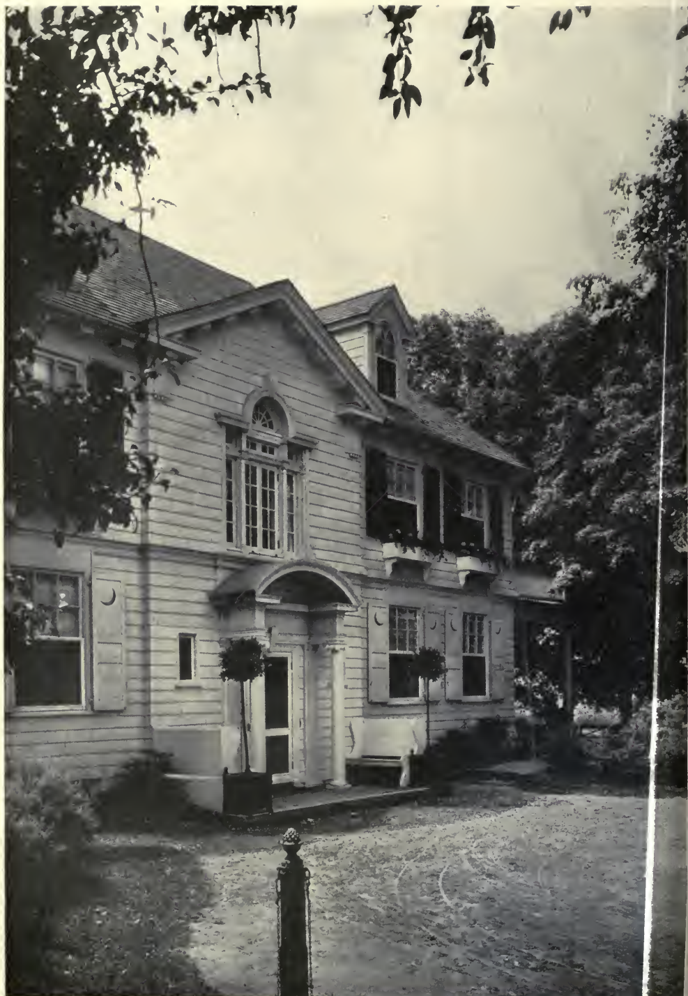
ENTRANCE DETAIL—RESIDENCE OF CARL SCHULTZ PETRASCH, ESQ., AT MT. KISCO, N. Y. LUDLOW & VALENTINE, ARCH'TS.
