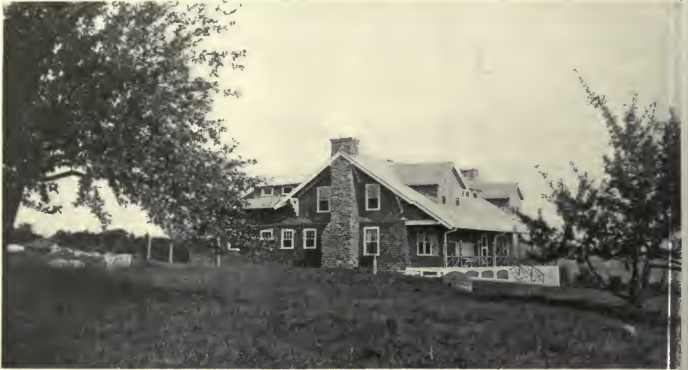
PRESIDENT FINLEY'S BUNGALOW AT TANWORTH, N. H. Kilham & Hopkins, Architects.
