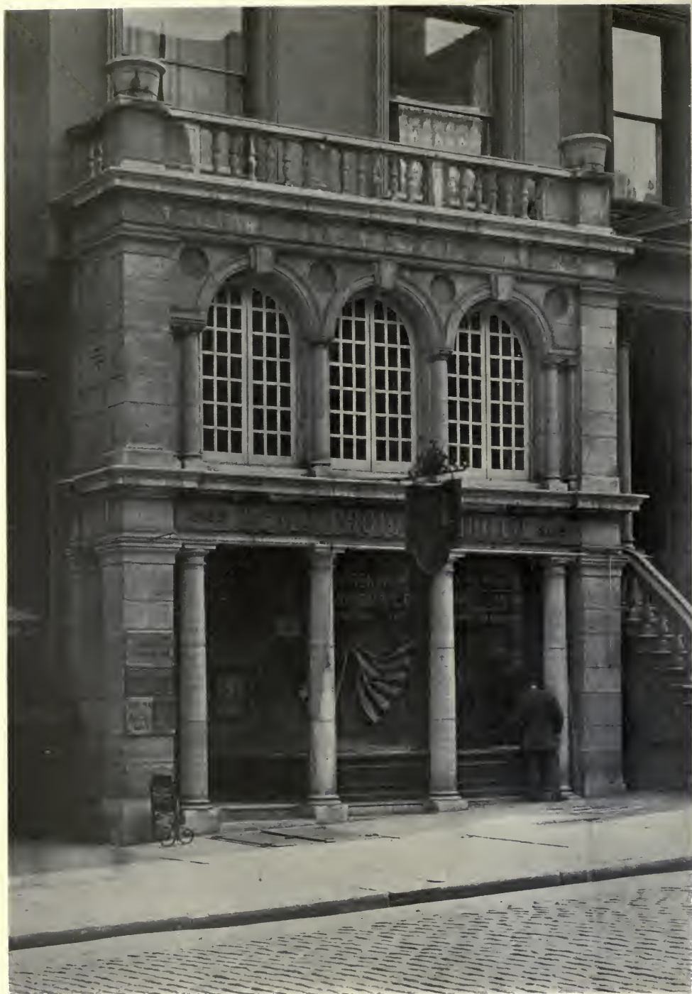
DETAIL OF THE FIRST TWO STORIES, NO. 305 MADISON AVENUE, NEW YORK CITY. HENRY ERKINS, ARCHITECT.
