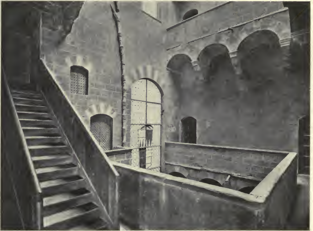
Stairs Leading to Loggia. THE PALAZZO DAVANZATI, FLORENCE, ITALY.
