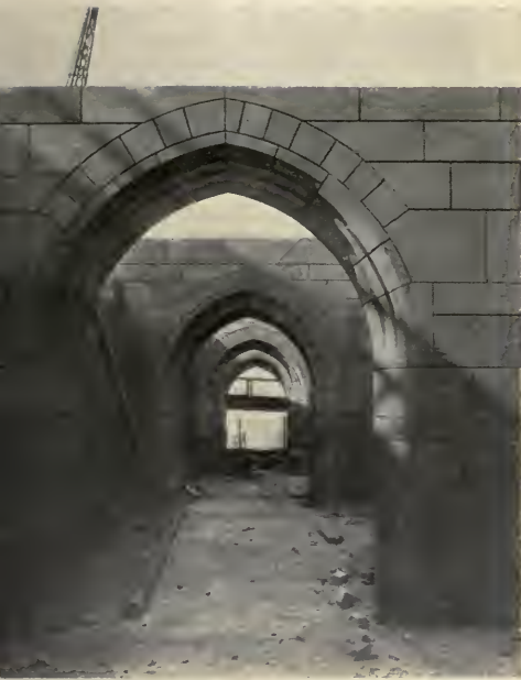
SOUTH TRIFORIUM LOOKING WEST.
