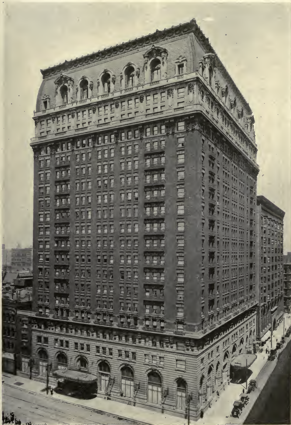
HOTEL LA SALLE, N. W. COR. MADISON AND LA SALLE STS. HOLABIRD & ROCHE, ARCHITECTS.
