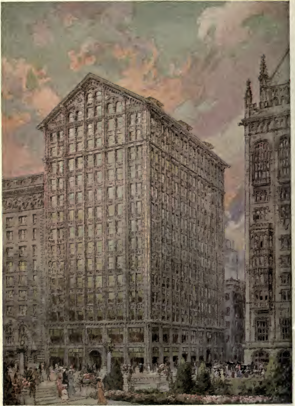
THE MONROE BUILDING, MICHIGAN AVE., CHICAGO, ILLINOIS. HOLABIRD & ROCHE, ARCHITECTS.
