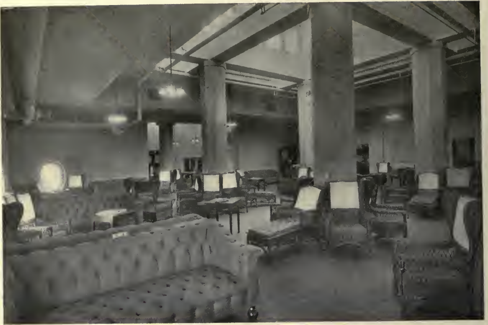
Women's Rest Room.
