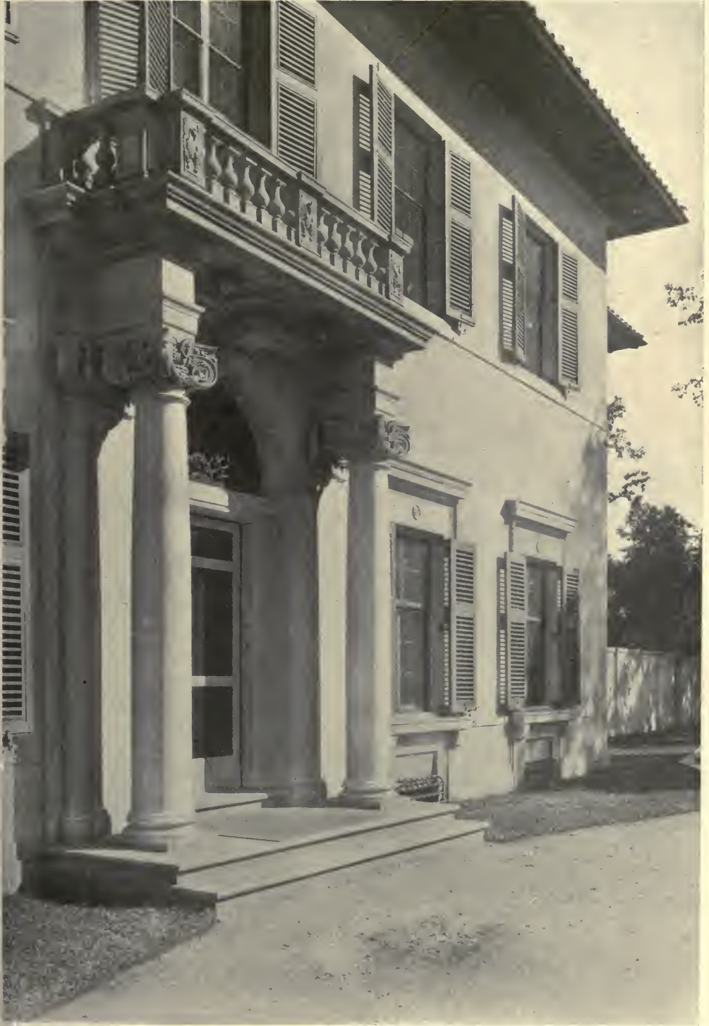
ENTRANCE DETAIL—HOUSE OF HAROLD F. McCORMICK, ESQ., LAKE FOREST, ILL. CHARLES A. PLATT, ARCHITECT.
