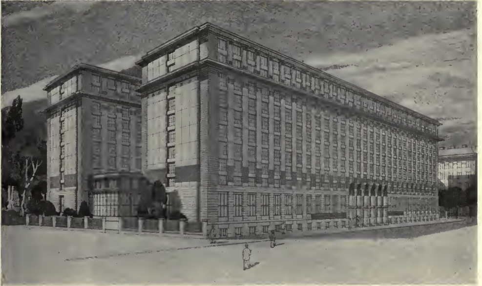
PROJECT FOR A UNIVERSITY LIBRARY IN VIENNA.
