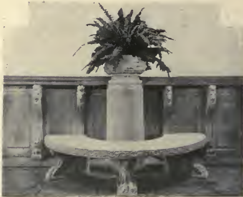
FIG. 20—EXAMPLE OF FINELY MOULDED WORK IN CONCRETE.
