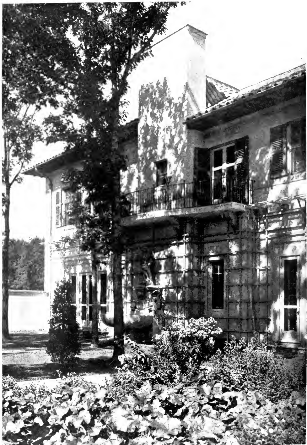
DETAIL OF SOUTH FRONT—HOUSE OF HAROLD F. McCORMICK, ESQ. CHARLES A. PLATT, ARCHT.
