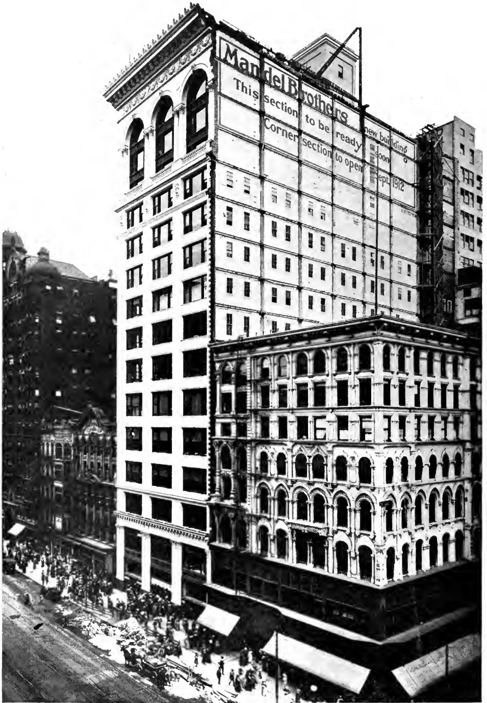
FIRST SECTION MANDEL BROS. BUILDING, N. E. COR. STATE & MADISON STS., CHICAGO, ILL.
