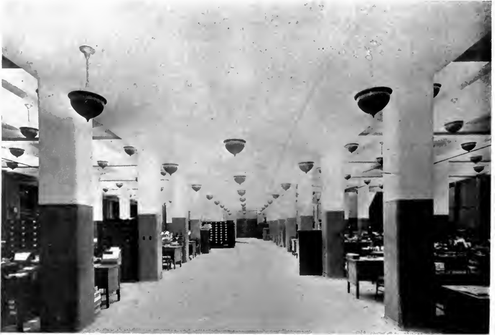
INDIRECT ILLUMINATION IN CIRCULATION DEPARTMENT. THE HOME OF THE CURTIS PUBLISHING COMPANY.
