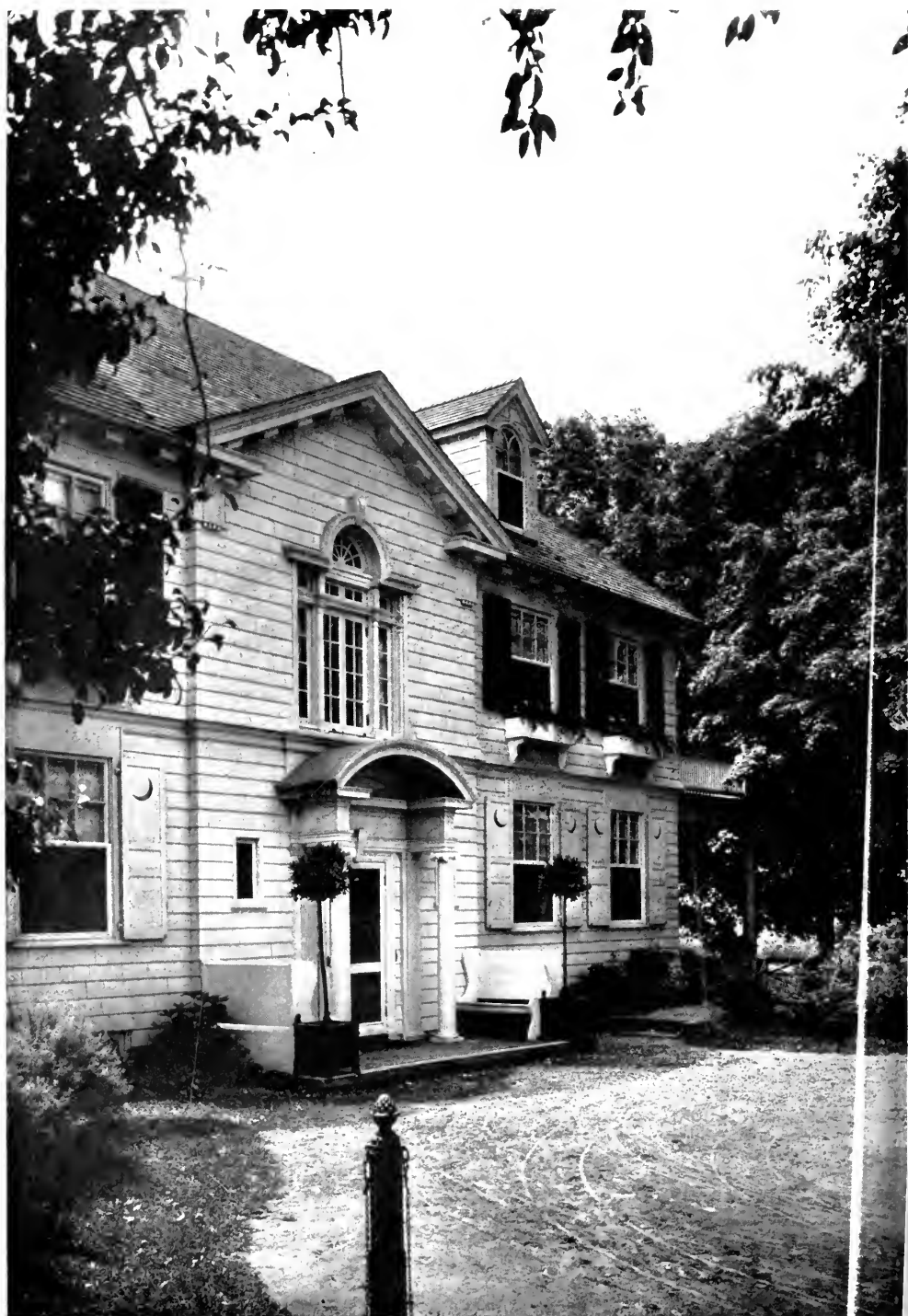
ENTRANCE DETAIL—RESIDENCE OF CARL SCHULTZ PETRASCH, ESQ., AT MT. KISCO, N. Y. LUDLOW & VALENTINE, ARCH'TS.
