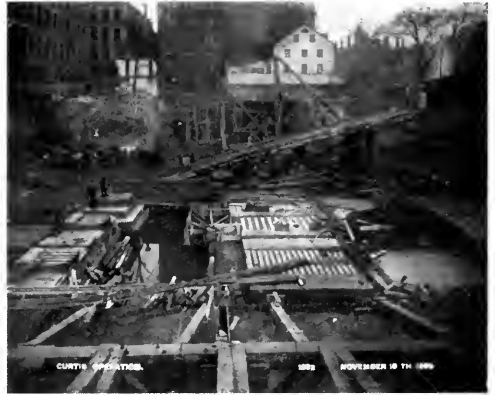
COFFERDAM AND FOUNDATION GRILLAGES.
