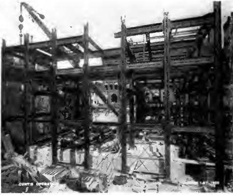
STEEL FRAME OF POWER BUILDING— SHOWING INDEPENDENT FOUNDATION FOR ENGINE ROOM.
