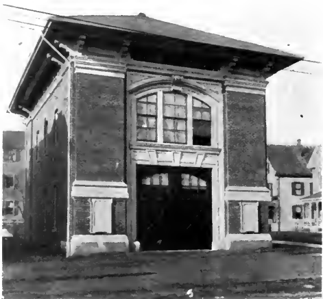
FIRE STATION—BEVERLY, MASS. Kilham & Hopkins, Architects.
