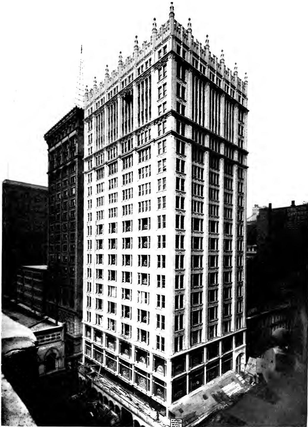
THE NORTH AMERICAN BUILDING, CHICAGO, ILLINOIS. HOLABIRD & ROCHE, ARCHITECTS.
