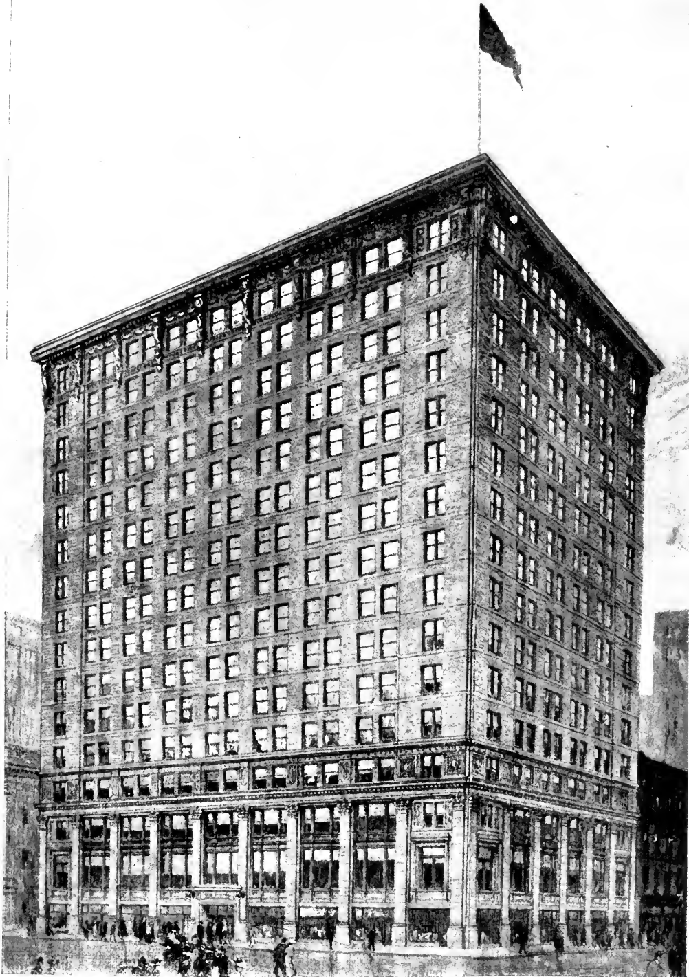
THE OTIS BUILDING, COR. MADISON ST. AND LA SALLE STREET. HOLAPHRD & ROCHE, ARCHITECTS.
