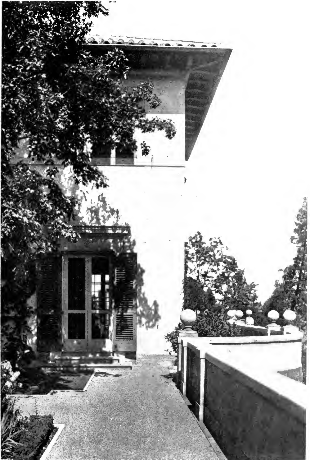
DETAIL OF SOUTHEAST CORNER—HOUSE OF HAROLD F. McCORMICK, ESQ., LAKE FOREST, ILL. CHARLES A. PLATT, ARCHITECT.
