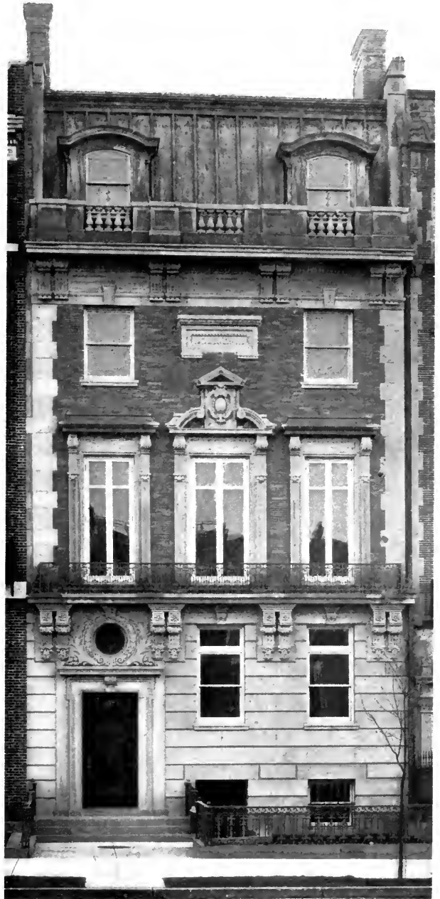
THE C. N. WALLACE HOUSE, Boston, Mass. Kilham & Hopkins, Architects.
