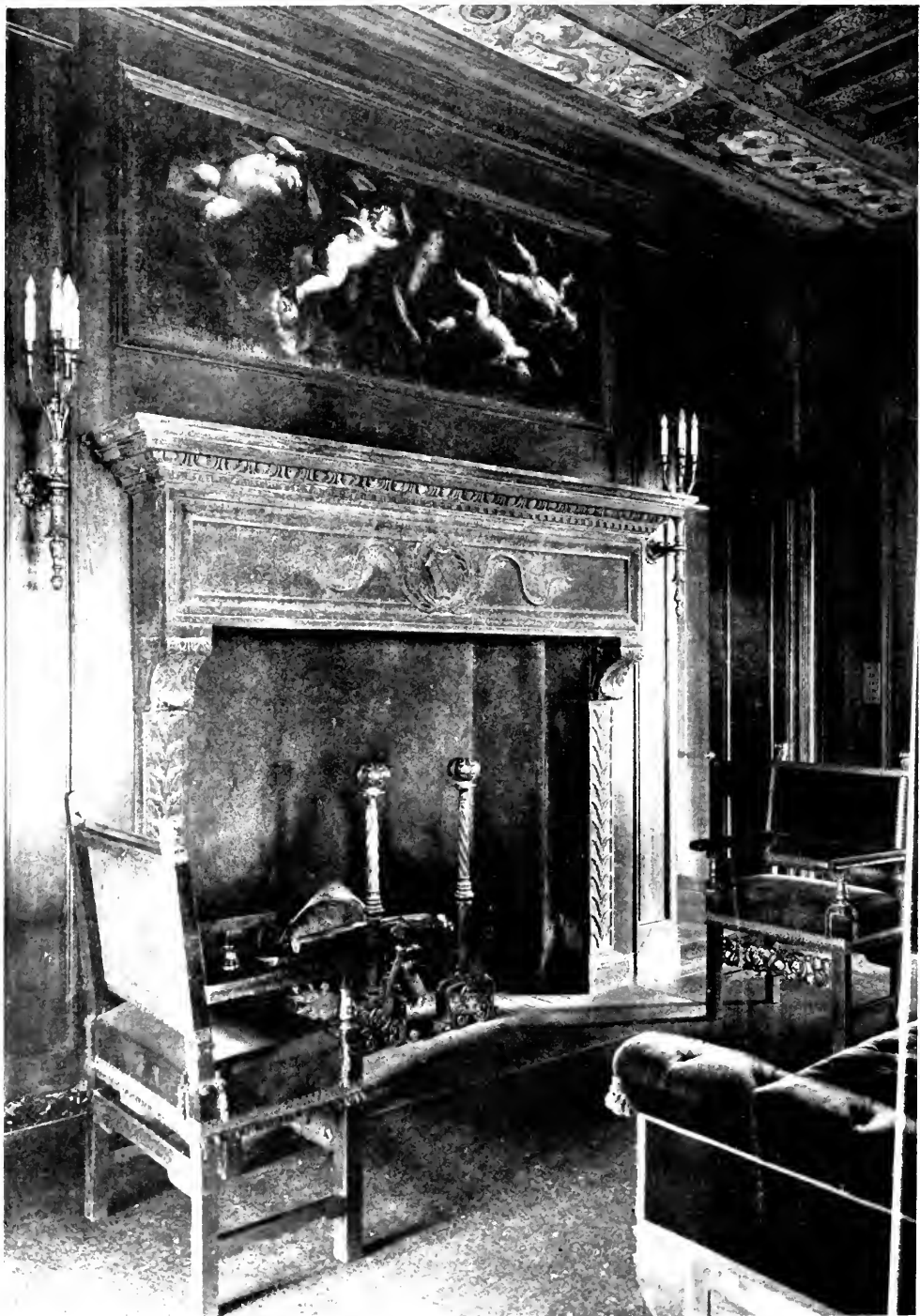
DETAIL OF LIBRARY MANTEL—HOUSE OF HAROLD F. McCORMICK, ESQ., LAKE FOR- EST, ILL. CHARLES A. PLATT, ARCHT.
