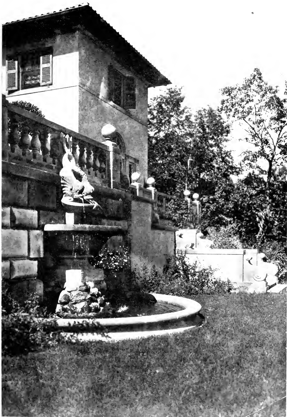
DETAIL OF TERRACE FOUNTAIN—HOUSE OF HAROLD F. McCORMICK, ESQ., LAKE FOREST, ILL. CHARLES A. PLATT, ARCHITECT.
