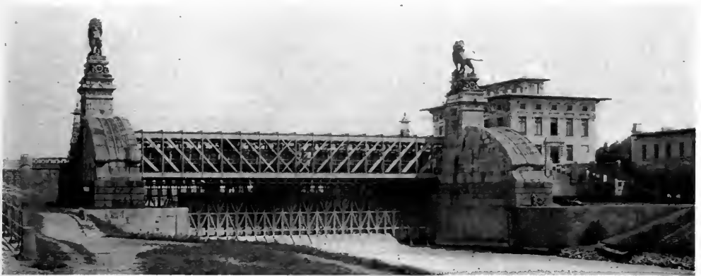
DAM AND GATES AT NUNENDORF.
