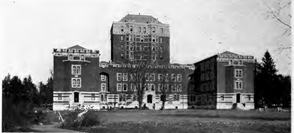
NORTH HALL, VASSAR COLLEGE. Pilcher & Tachan, Architects.
