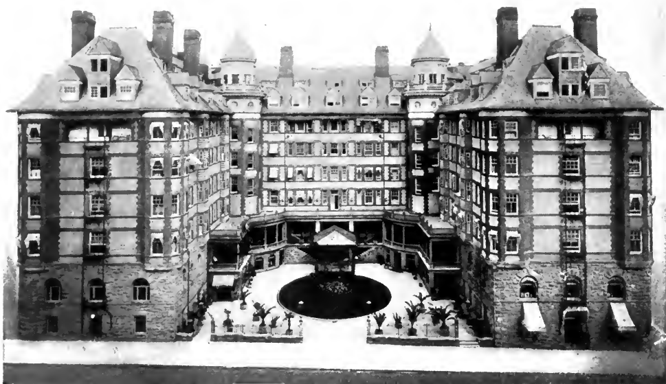
THE PORTLAND HOTEL, PORTLAND, OREGON. McKim, Mead & White, Architects.
