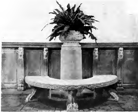
FIG. 20—EXAMPLE OF FINELY MOULDED WORK IN CONCRETE.
