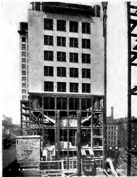
POWER BUILDING FROM COURT, SHOWING COAL-BUNKER FIRING COAL CONVEYORS, SMOKE-STACKS, ASH BINS, BRICK FACING ON COURT SIDE, ETC.
