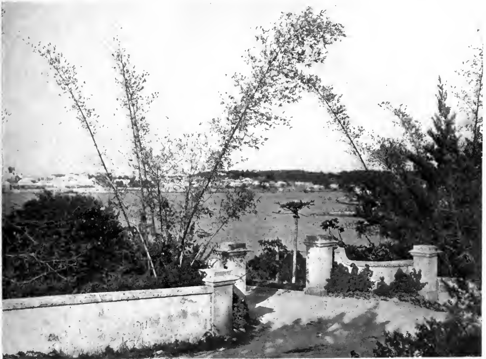
FIG. 10—MONOLITHIC CONCRETE ENTRANCE WAY ON THE ISLAND OF BERMUDA.
