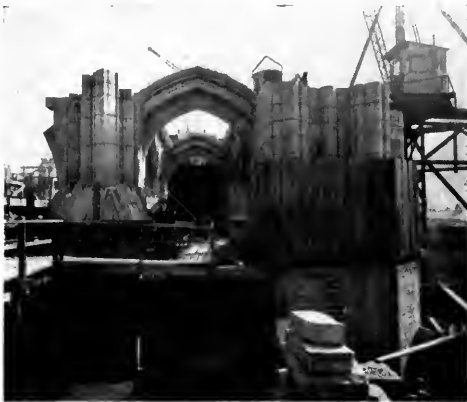
SOUTH CHOIR AISLE LOOKING EAST.
