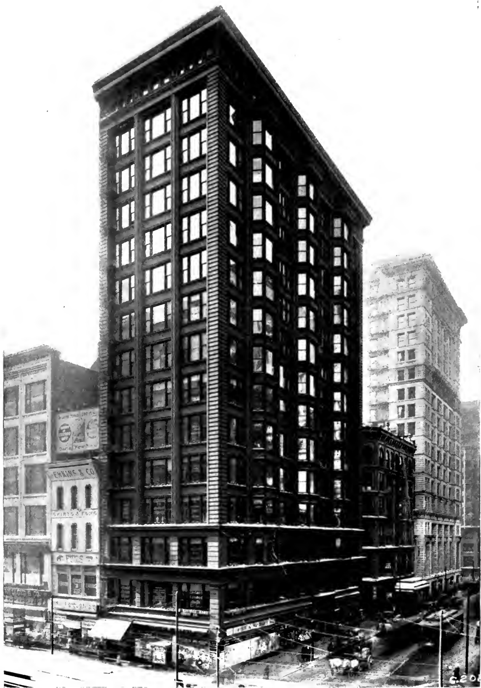
CHICAGO SAVINGS BANK BUILDING. HOLABIRD & ROCHE, ARCHITECTS.
