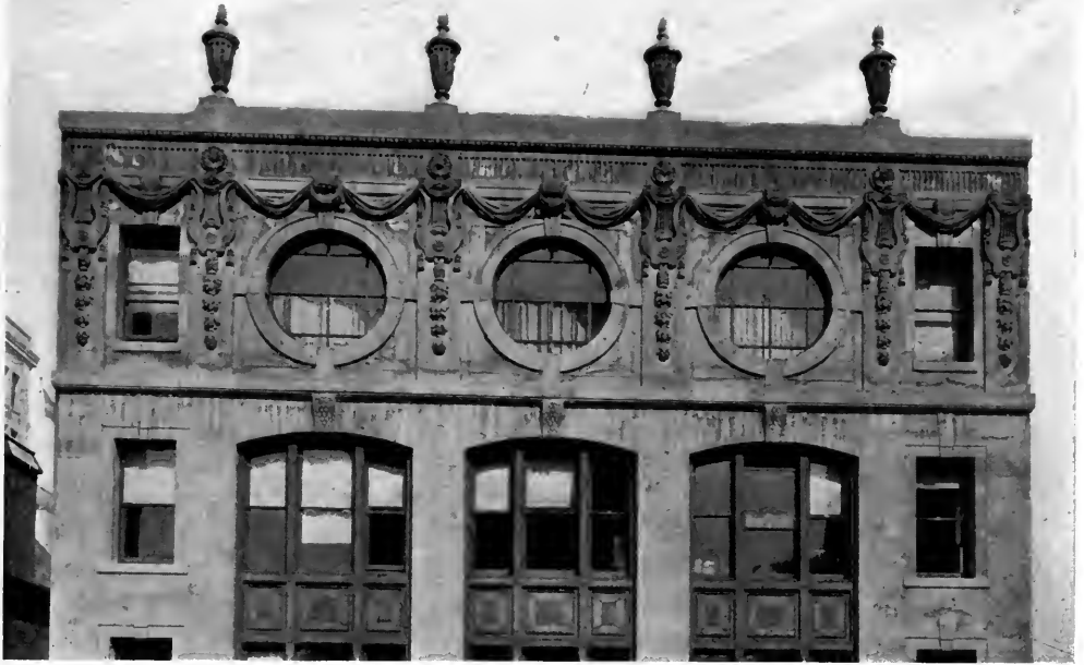
NO. 7 EAST 43D STREET—DETAIL OF UPPER FLOORS. Delano & Aldrich, Architects.
