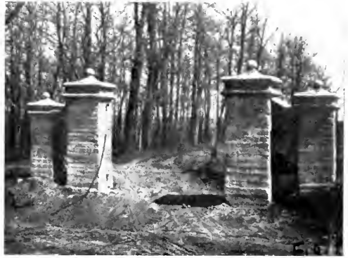
FIG. 8—CONCRETE USED FOR ENTRANCE, ROUGH FINISH.
