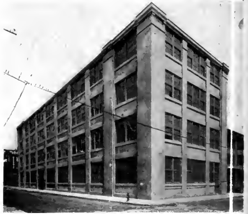
SIMPLEX ELECTRICAL CO. Kilham & Hopkins, Architects.
