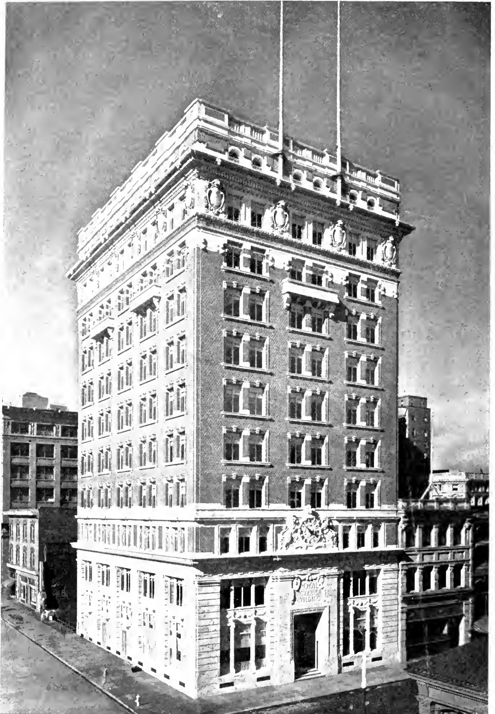
THE ROYAL INSURANCE BUILDING, SAN FRANCISCO, CALIFORNIA. HOWELLS & STOKES, ARCHITECTS.
