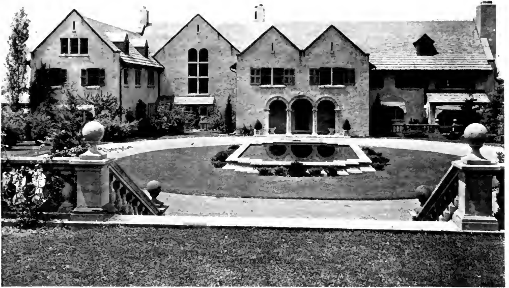
FIG. 31. RESIDENCE OF HORATIO GATES LLOYD, ESQ., HAVERFORD, PA. Wilson Eyre & McIlvaine, Architects.
