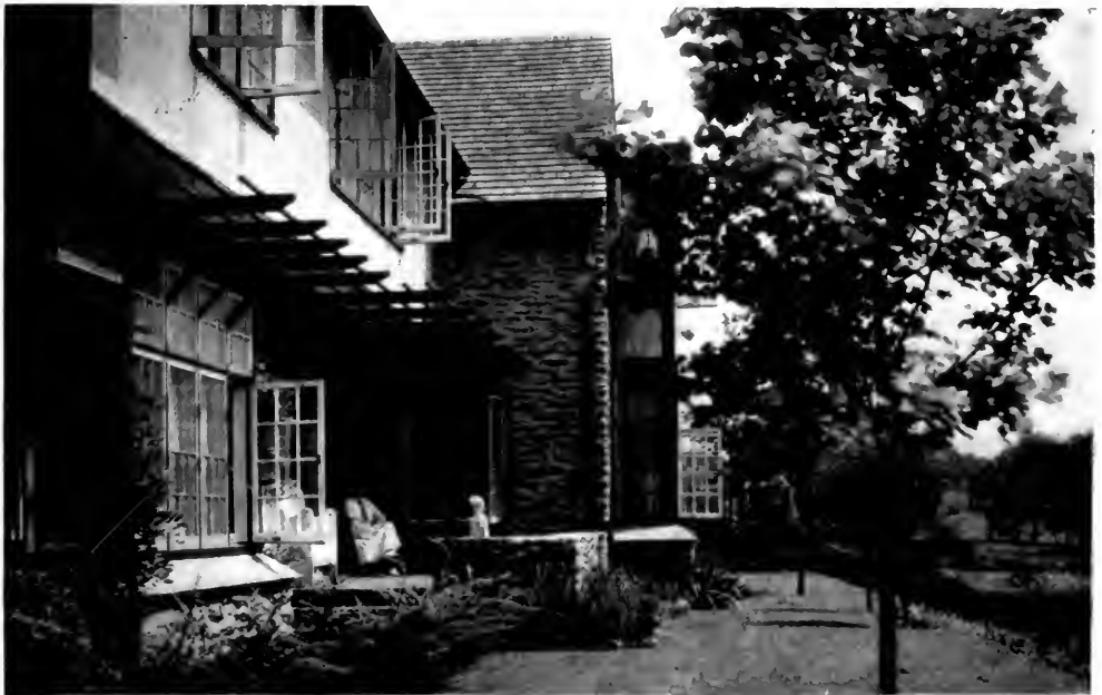
GARDEN TERRACE—RESIDENCE OF LEONARD T. BEALE, ESQ., ST. DAVIDS, PA. Mellor & Meigs, Architects.
