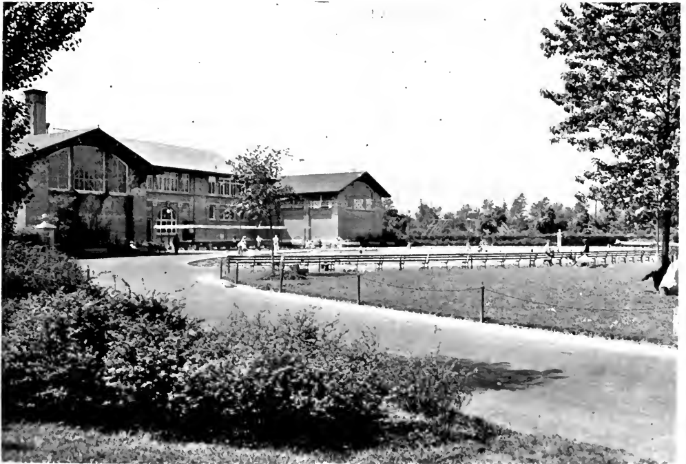
FIELD HOUSE—HAMILTON PARK, CHICAGO.
