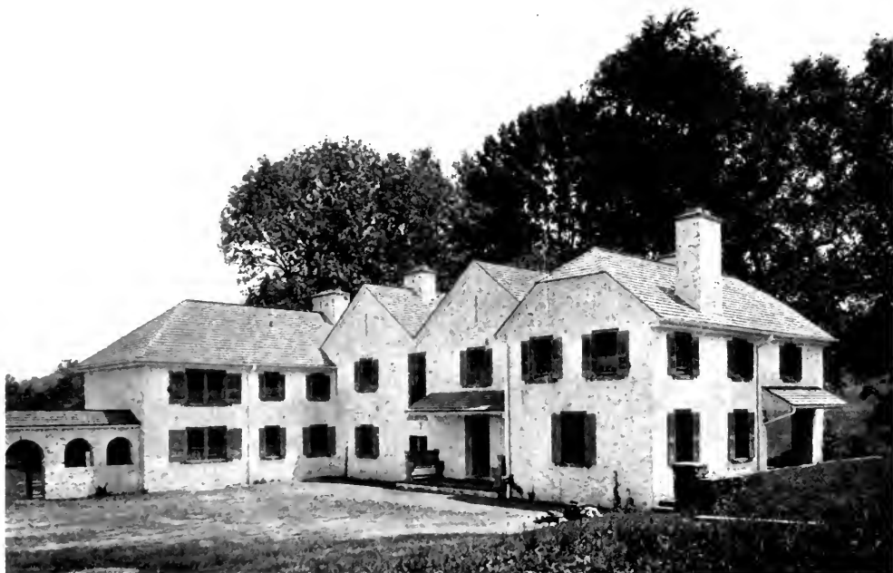
FIG. 57. FORECOURT—RESIDENCE OF MRS. ALBERT B. KELLEY, RADNOR, PA. Wilson Eyre & Mellvaine, Architects.
