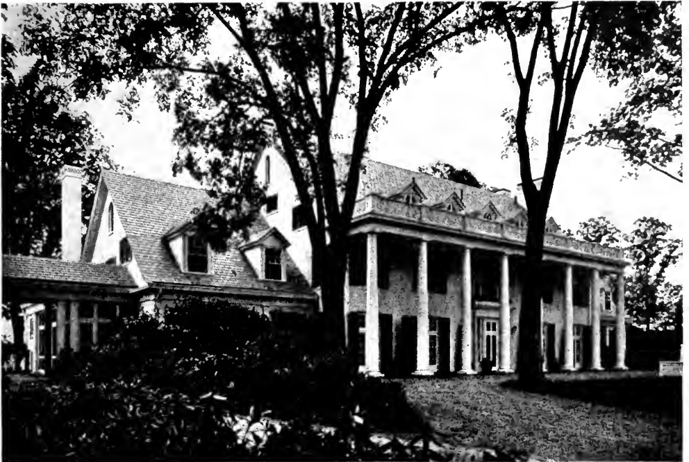
FIG. 6. RESIDENCE OF TRACY DOWS, ESQ., RHINEBECK, N. Y. Albro & Lindeberg, Architects.
