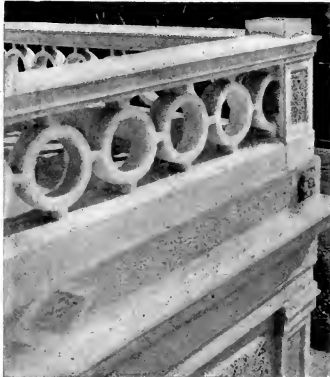
Combination of Smooth Surface Finished With Carborundum Blocks, Pointed Surface, Pebble Dash and Simple Casting Details.
