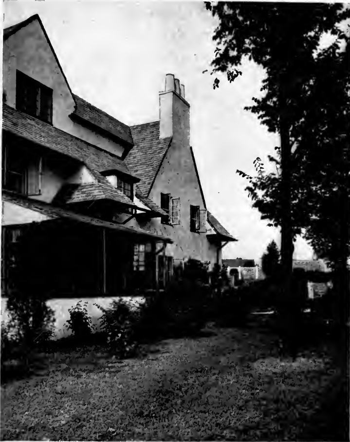
FIG. 28. RESIDENCE OF J. B. VAN HAELEN, ESQ., HARTSDALE, N. Y. Frank J. Forster, Architect.
