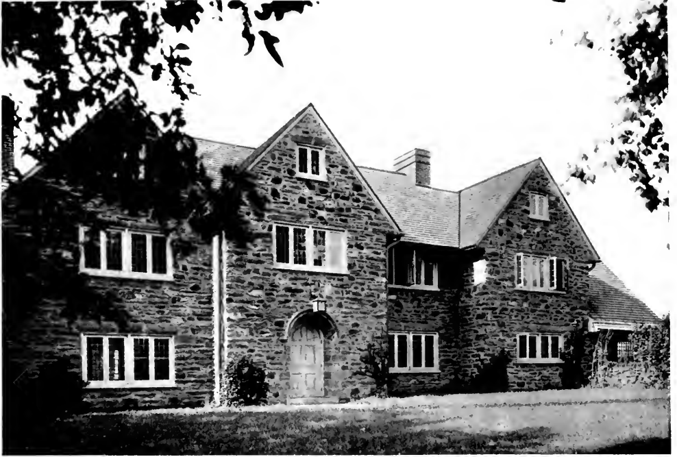
FIG. 33. SOUTH FRONT FROM LAWN—RESIDENCE OF DR. EDWARD B. KRUMBHAAR, WHITEMARSH VALLEY, PA. Arthur H. Brockie, Architect.
