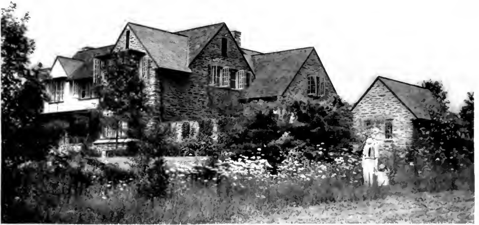
VIEW FROM EAST—RESIDENCE OF LEONARD T. BEALE, ESQ., ST. DAVIDS, PA. Mellor & Meigs, Architects.
