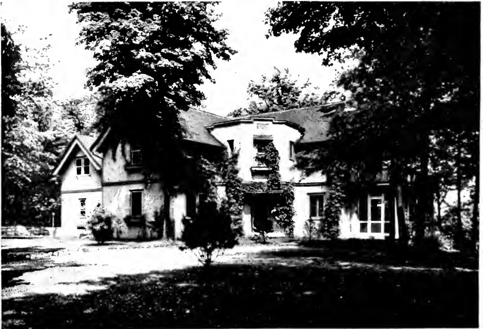
FIG. 101. RESIDENCE OF I. HELLER, ESQ., CEDAR LAKE, WIS. Brust & Philipp, Architects.
