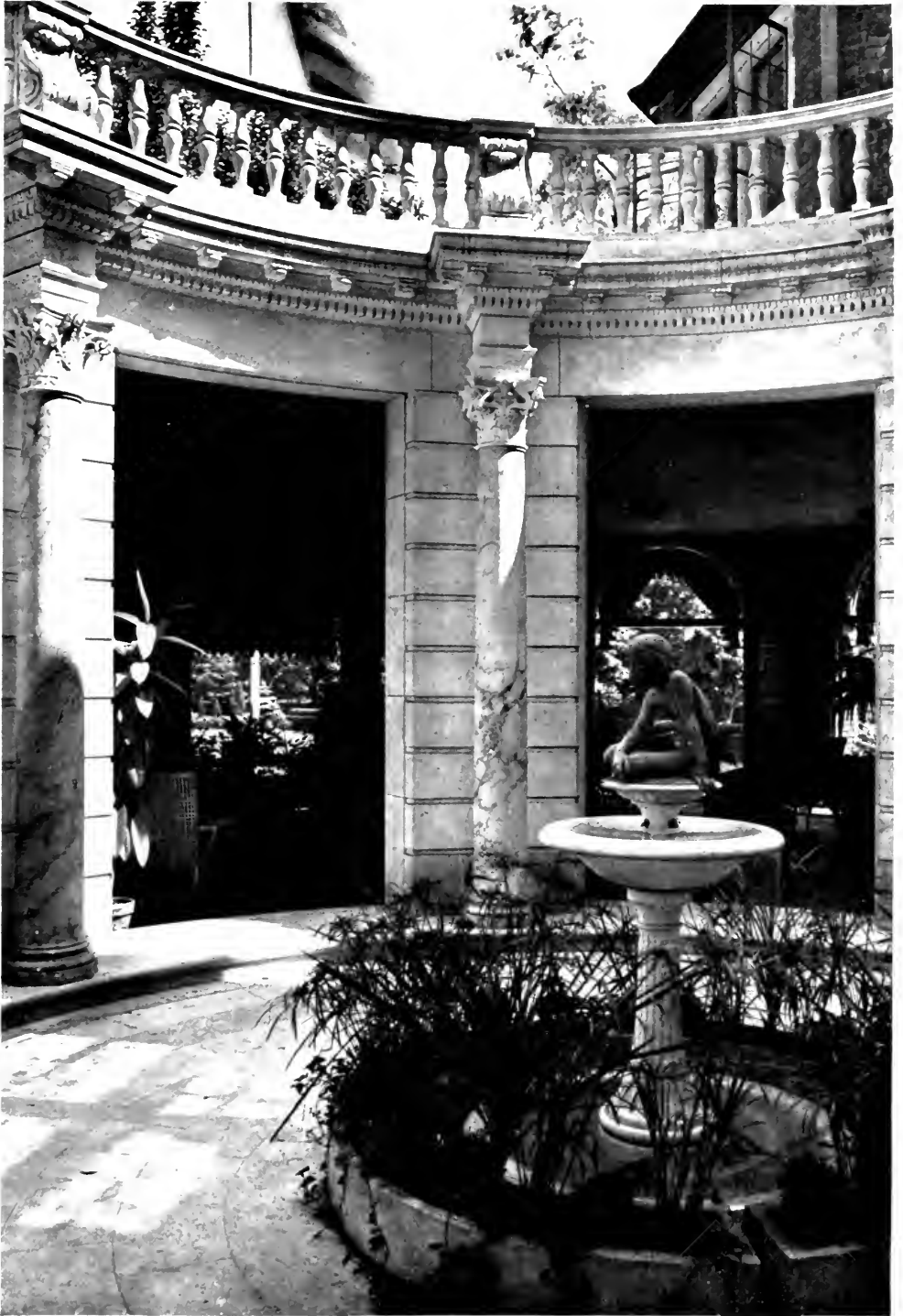
FIG. 17. COURT—RESIDENCE OF CHARLES A. WIMPFHEIMER, ESQ., LONG BRANCH, N. J. HARRY ALLEN JACOBS, ARCHITECT.
