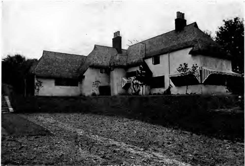
FIG. 24. RESIDENCE OF WALTER B. WALKER, ESQ., ARDSLEY, N. Y. Frank J. Forster, Architect.
