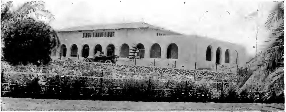
SCRIPPS PLAYGROUND BUILDING, LA JOLLA, CAL. Irving J. & Louis J. Gill, Architects.
