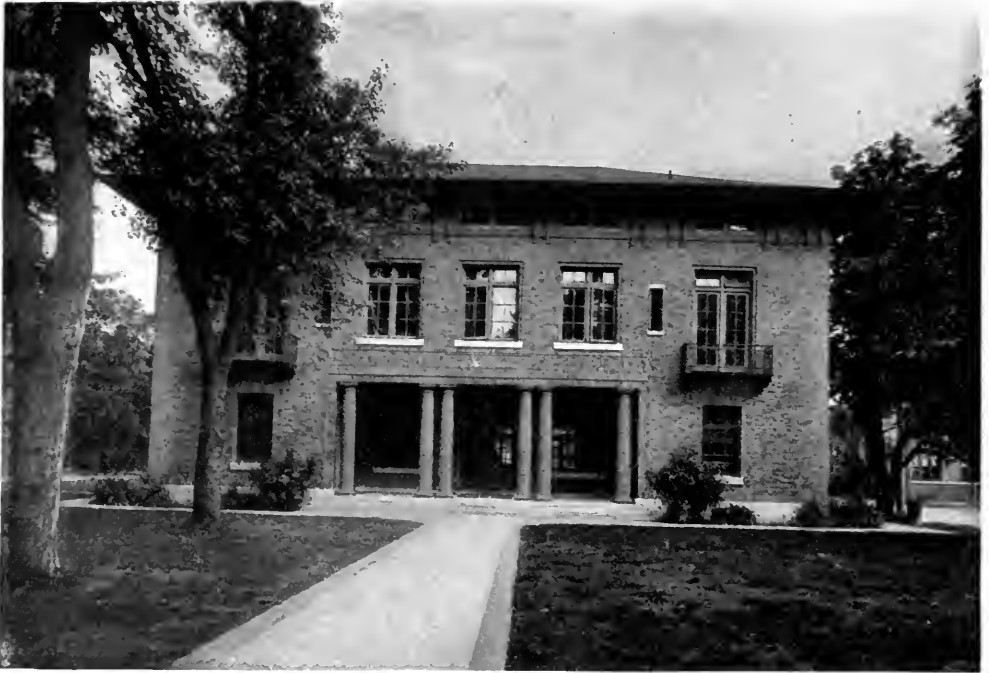
RECREATION BUILDING (CLARKE HALL), HAMPTON NORMAL AND AGRICULTURAL INSTITUTE, HAMPTON, VA. Ludlow & Peabody, Architects.
