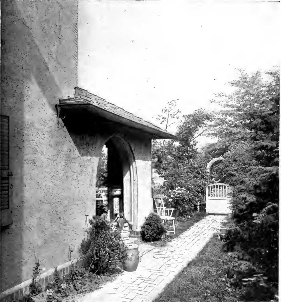
GARDEN GATE—HOUSE OF E. DIGBY BALTZELL, ESQ., ST. MARTIN'S, CHESTNUT HILL, PHILADELPHIA. EDMUND B. GILCHRIST, ARCHITECT.
