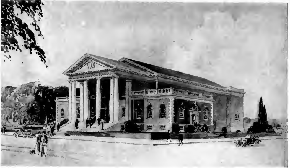
MEMORIAL COMMUNITY BUILDING, GOLDSBORO, N. C. C. Adrian Casner, Architect.
