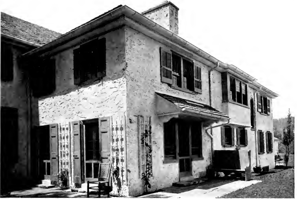
FIG. 60. BREAKFAST TERRACE AND EAST FRONT—RESIDENCE OF MRS. ALBERT B. KELLEY, RADNOR, PA. Wilson Eyre & Melvaine, Architects.
