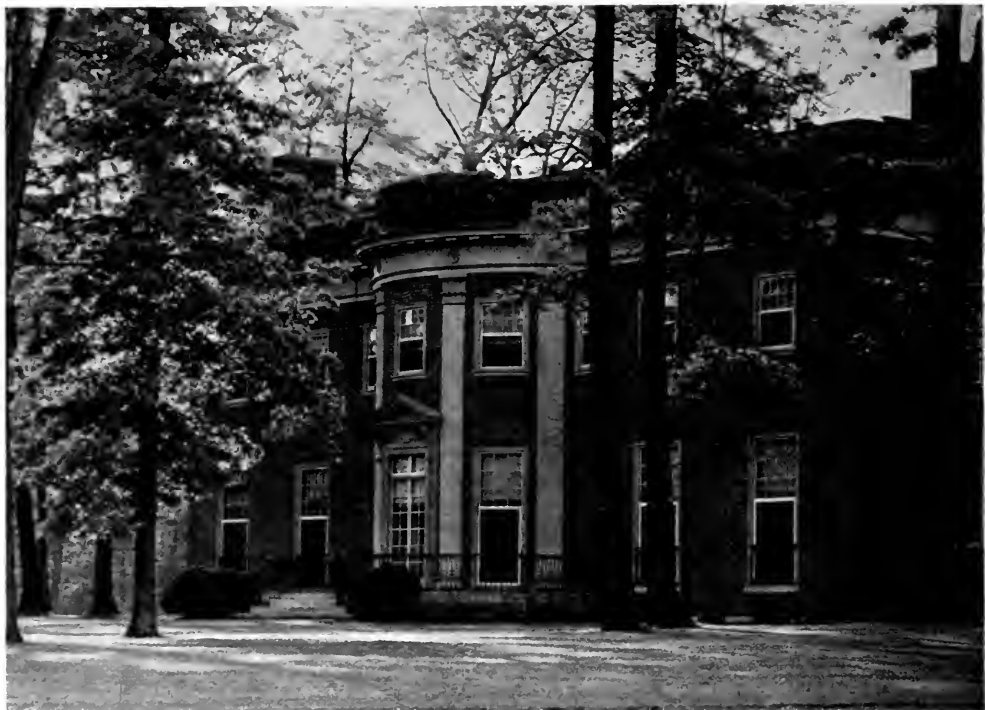
FIG. 8. RESIDENCE OF JAMES SWAN FRICK, ESQ., GUILFORD, BALTIMORE, MD. John Russell Pope, Architect.
