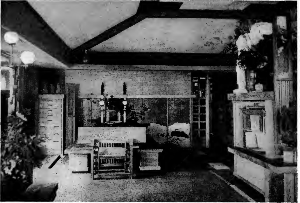
FIG. 16. LIVING ROOM—RESIDENCE OF FRANK LLOYD WRIGHT, SPRING GREEN, WIS. Frank Lloyd Wright, Architect.
