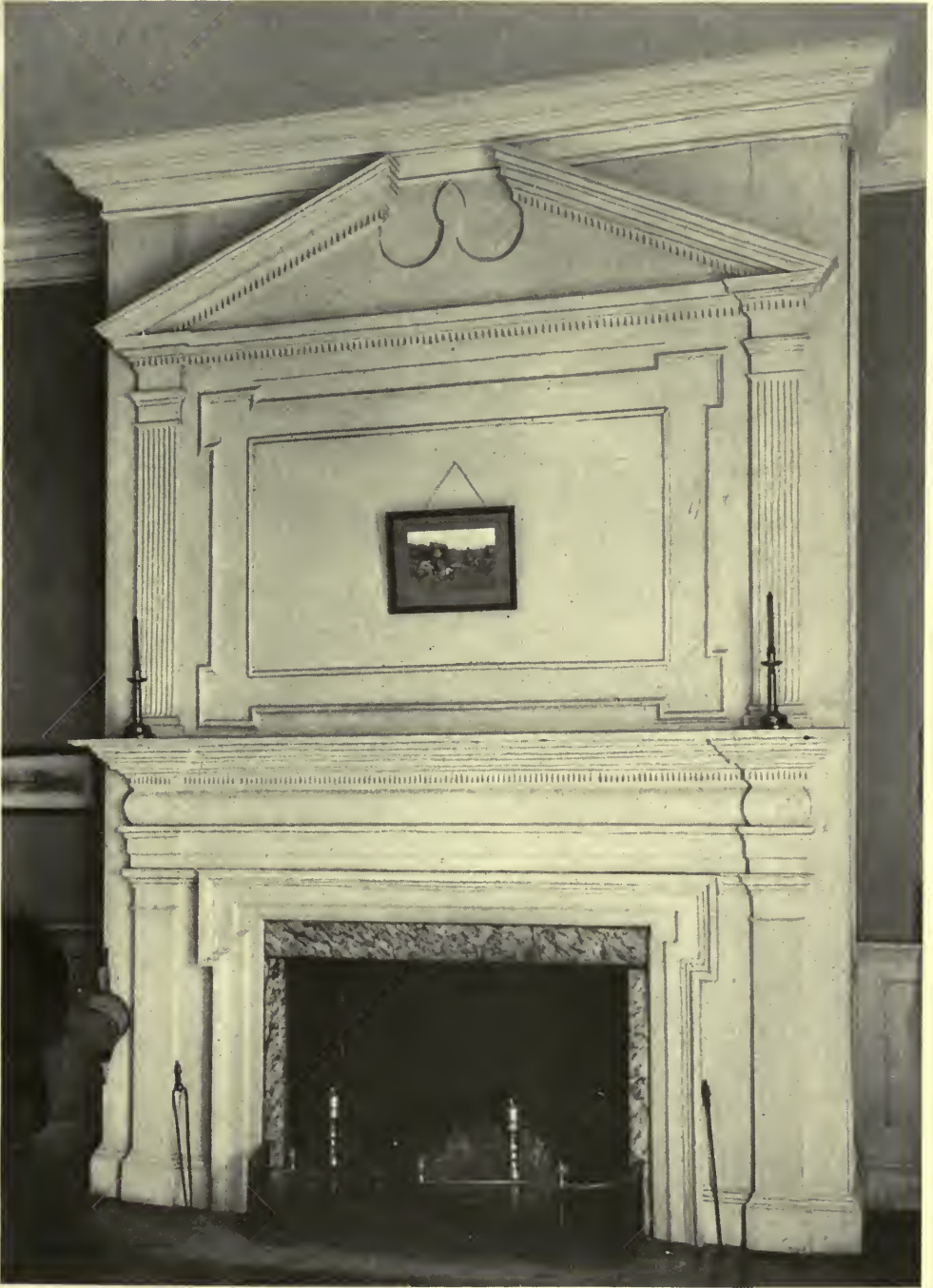
THE STATE BEDCHAMBER MANTELPiece ON SECOND FLOOR OF EPHRAIM BLAINE HOUSE, CARLISLE, PA., 1792-97. EXAMPLE OF HIGH MANTEL WITHOUT ADJOINING WOODWORK.
