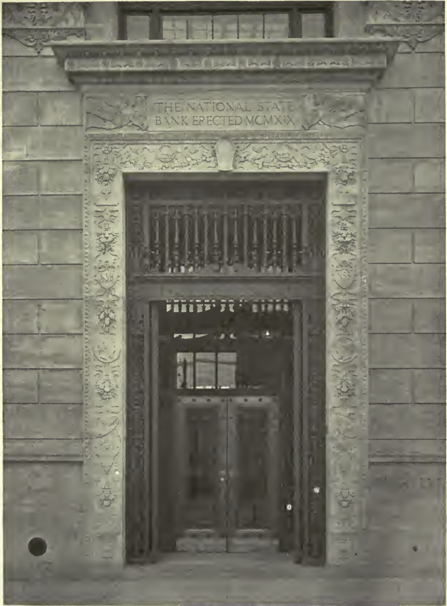
Entrance Gates and Vestibule Enclosure The National State Bank, Elizabeth, New Jersey Dennison & Hiron, Architects
