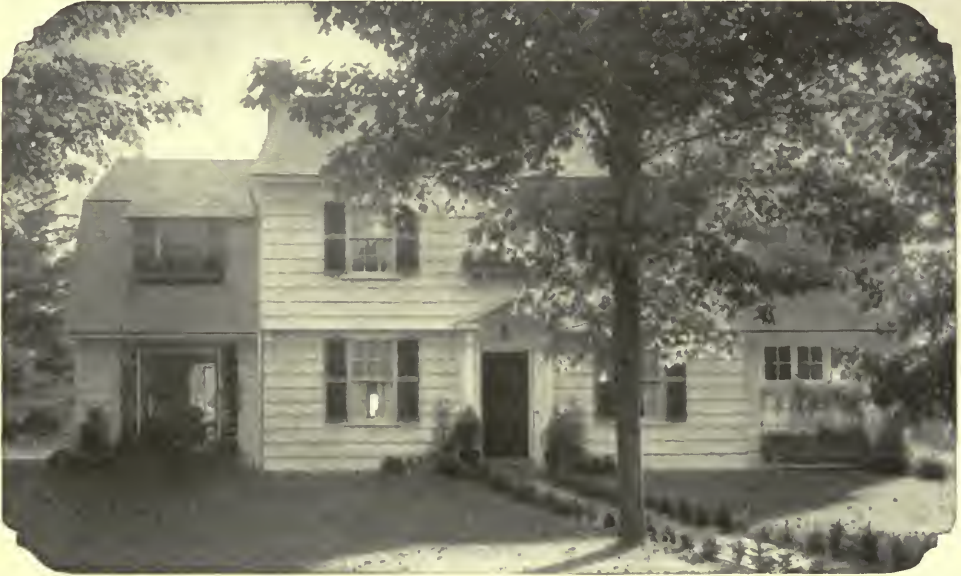
Residence at West Newton, Mass., Davis & Brooks, Architects. Finished throughout with Arkansas Soft Pine
