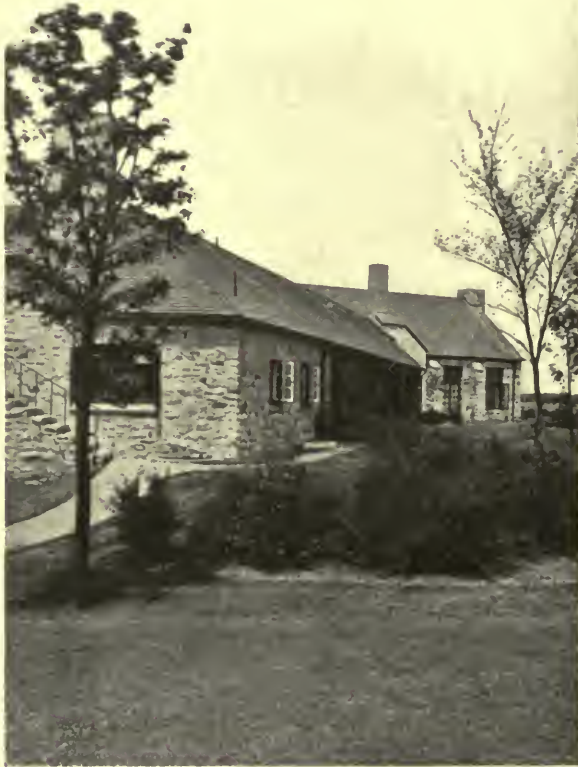
ENTRANCE TO MEN'S LOCKER ROOM, NORWOOD GOLF CLUB, LONG BRANCH, N. J. Harry Allan Jacobs, Architect.
