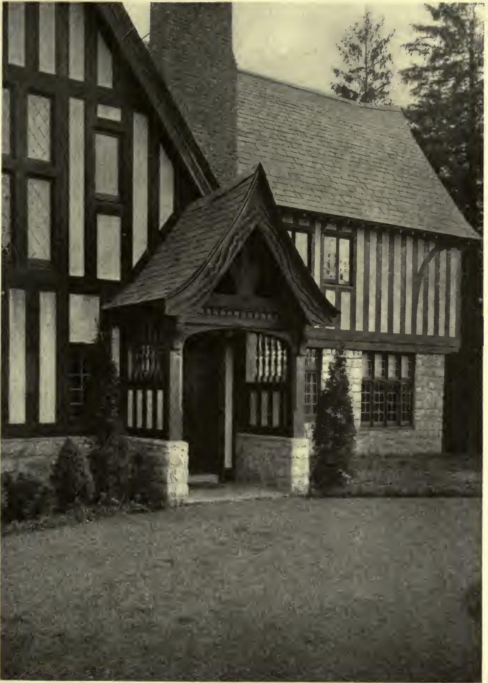
RESIDENCE OF E. C. DE WITT, ESQ., SCARSDALE, N. Y. ALBERT JOSEPH BODKER, INC., ARCHITECTS.
