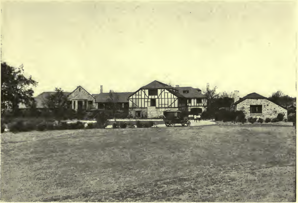
CLUB AND PROFESSIONAL HOUSE—NORWOOD GOLF CLUB, LONG BRANCH, N. J. Harry Allan Jacobs, Architect.
