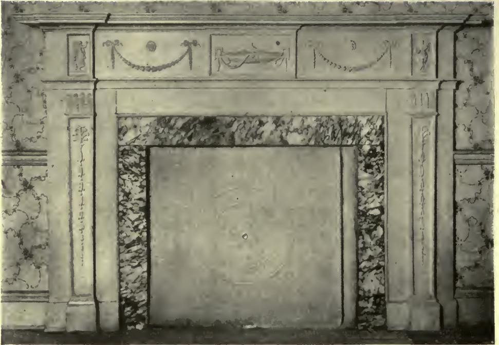
MANTEL NO. 3 IN DILLER HOUSE AT 21 SOUTH QUEEN STREET, LANCASTER.
