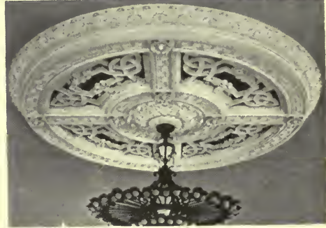
DETAIL OF CENTER OF CEILING
