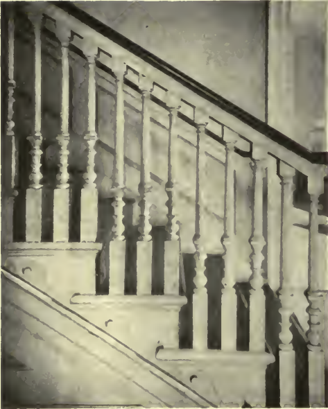
DETAIL OF STAIR BALUSTRADE, CLIVEDEN, GERMANTOWN (1763).
