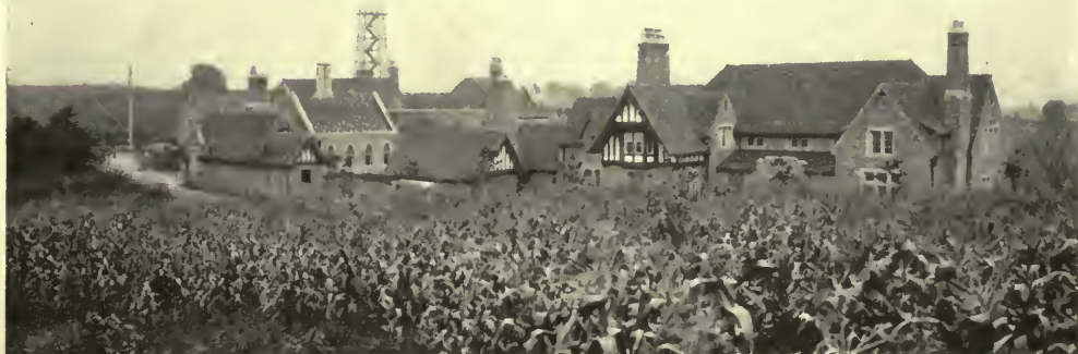
THE STEEL TOWER, A TEMPORARY OBSERVATION PLATFORM, MARKS THE SITE OF THE FUTURE CARSON MEMORIAL TOWER.
