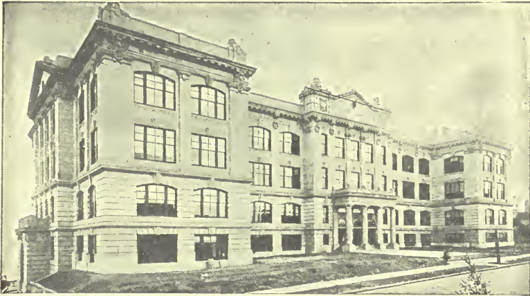
The Queen Anne High School, Seattle, Washington, equipped with a Webster System of Steam Heating.
