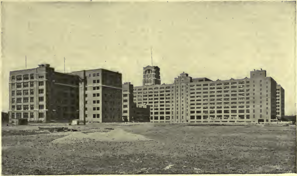
REAR VIEW—EASTERN STORE OF SEARS, ROEBUCK & CO., PHILADELPHIA. George C. Nimmons & Co., Architects.
