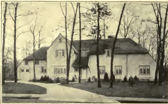
Residence of Geo. W. Klewer, Architect, 36 Crescent Drive, Glencoe, Ill. Bishopric Sheathing used as sub-flooring—on roofs under shingles, and as Sheathing under Bishopric Stucco Base. Bishopric Stucco Base used on all exteriors. Bishopric Plaster Base used on all interiors.
