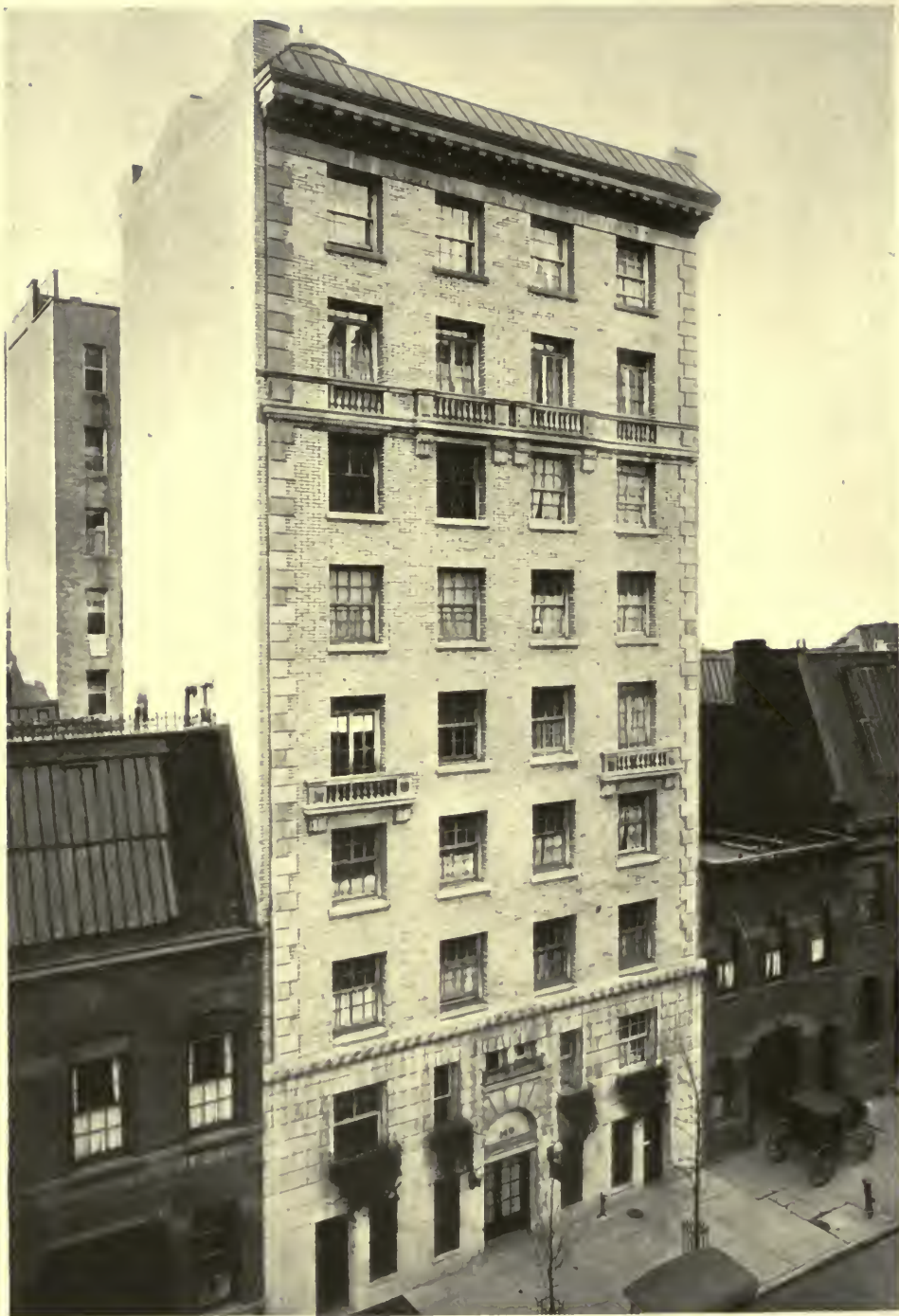
FIG. 38. NOS. 140 AND 142 WEST 55TH STREET, NEW YORK CITY. SCHWARTZ & GROSS, ARCHITECTS.
