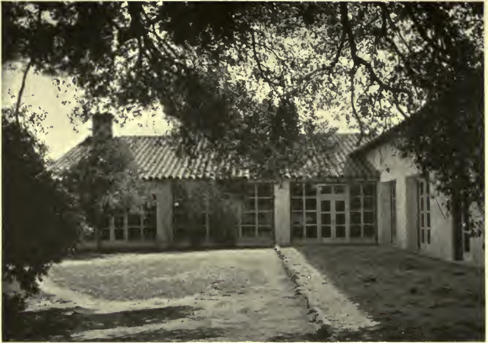
LOOKING SOUTH IN THE PATIO, TOWARD GLAZED PORCH OR TEA-ROOM— FLINTRIDGE COUNTRY CLUB Myron Hunt, Architect
