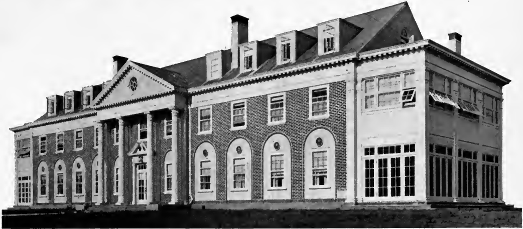
UNION METAL COLUMNS AT ENTRANCE TO ALBERTINA KERR NURSERY HOME, PORTLAND, ORE.
