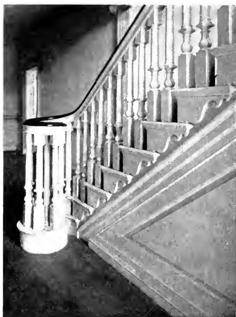
STAIRWAY AT WHITBY HALL, PHILADELPHIA (1754).
