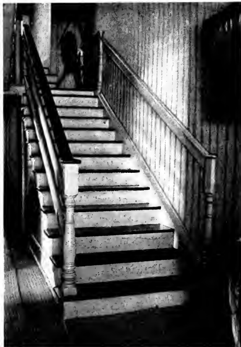
STAIRWAY OF THE C. G. DONNEL HOUSE, SUNBURY (1780).
