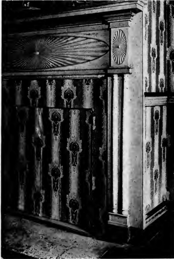
DETAIL OF MANTELPiece FROM A HOUSE NEAR MECHANICSBURG.
