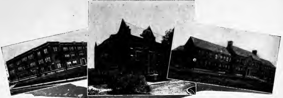
Technical High School, St. Cloud, Minn. Tyrle & Chapman, Architects. Laurence Construction Co., General Contractors.
