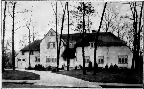
Residence of Geo. W. Klewer, Architect, 36 Crescent Drive, Glencoe, Ill. Bishopric Sheathing used as sub-flooring—on roofs under shingles, and as Sheathing under Bishopric Stucco Base. Bishopric Stucco Base used on all exteriors. Bishopric Plaster Base used on all interiors.
