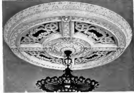
DETAIL OF CENTER OF CEILING
