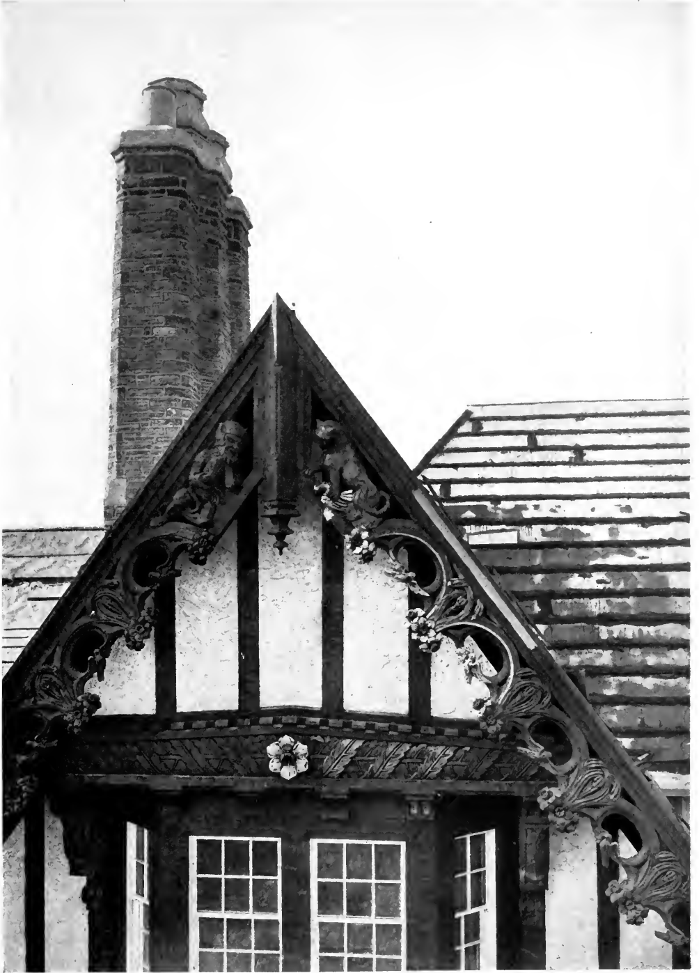
ONE OF THE GABLES OF NARCISSUS COTTAGE BEFORE THE ROOFS WERE TILED, SHOWING EXPERIMENTAL COLORING—THE CARSON COLLEGE FOR ORPHAN GIRLS.
