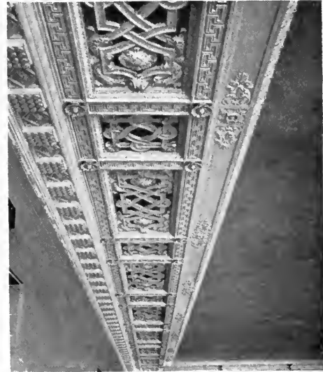
DETAIL OF SIDE OF CEILING
