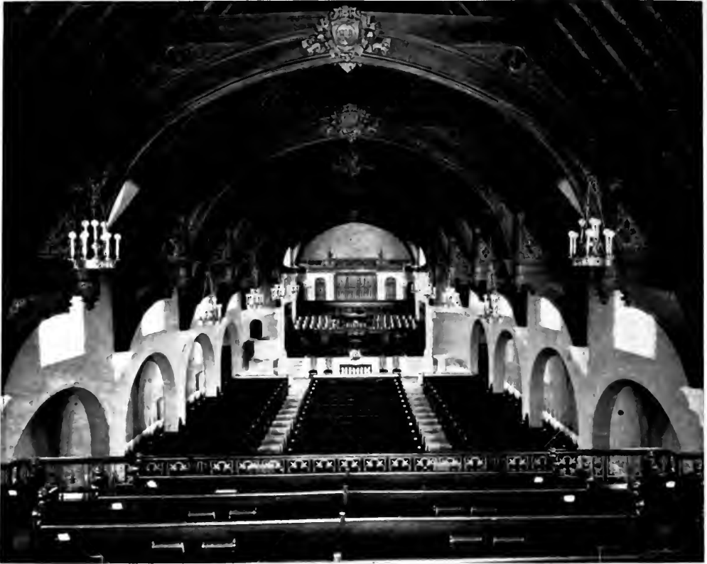
GRACE METHODIST EPISCOPAL CHURCH, DAYTON, OHIO Schenk and Williams, Architects
