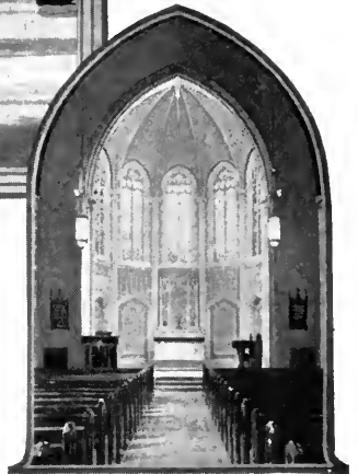
The interior is done in quartered oak; Caen stone walls with Artstone trimming. Aisle and vestibule floors of Faence tile; Chancel floor of Grey Tennessee Marble. The altar is of White Vermont Marble.
