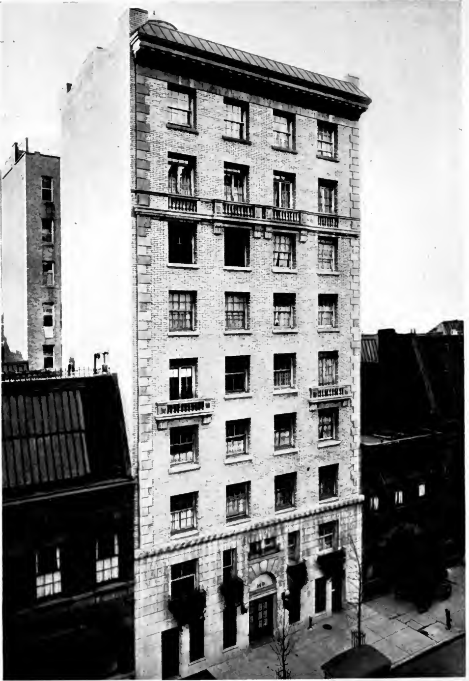
FIG. 38. NOS. 140 AND 142 WEST 55TH STREET, NEW YORK CITY. SCHWARTZ & GROSS, ARCHITECTS.
