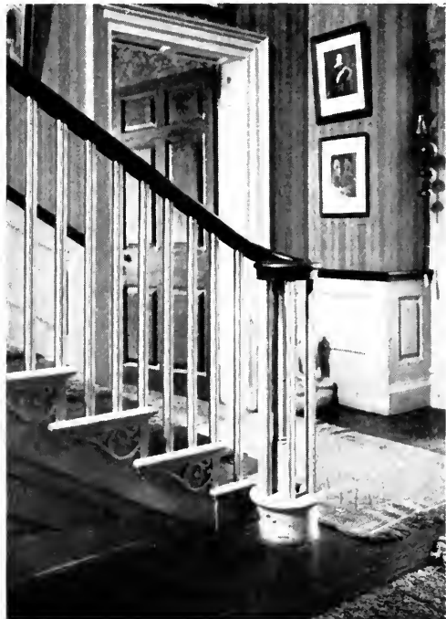
DETAIL OF STAIR BALUSTRADE, UPSALA, GERMANTOWN (1798)
