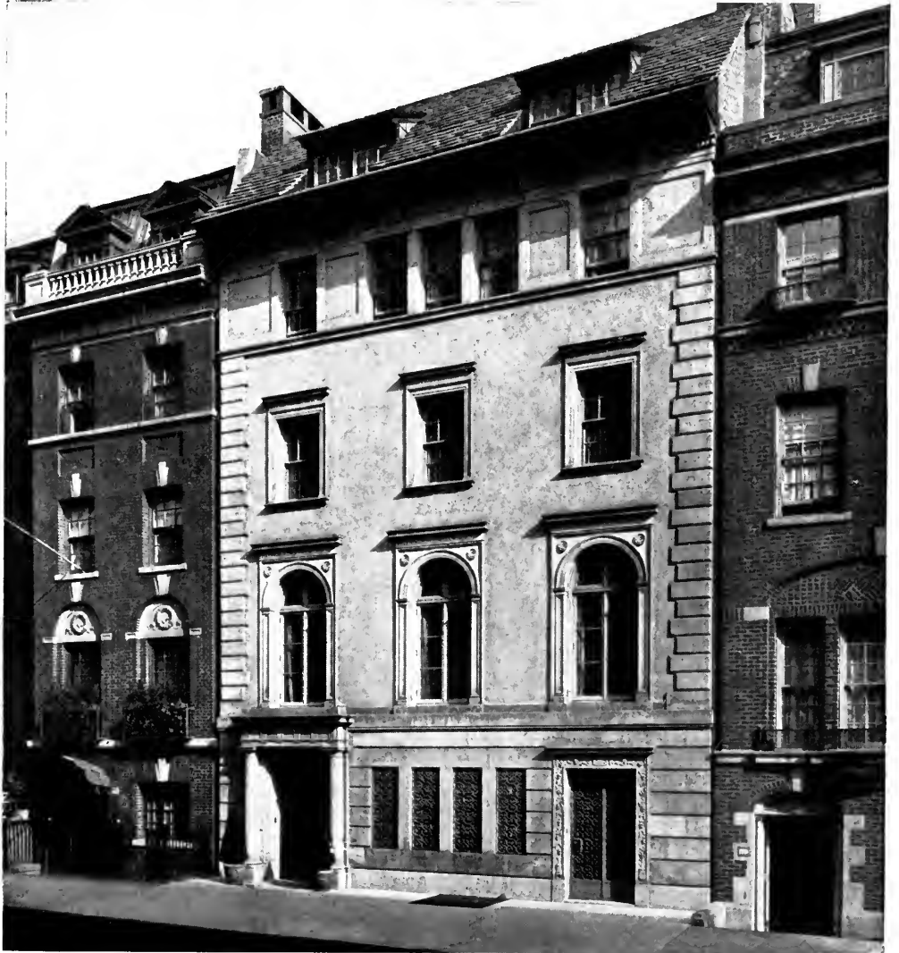
RESIDENCE OF BAYARD DOMINICK, ESQ., 115-117 EAST FIFTY-FOURTH STREET, NEW YORK CITY. WILLIAM F. DOMINICK, ARCHITECT.
