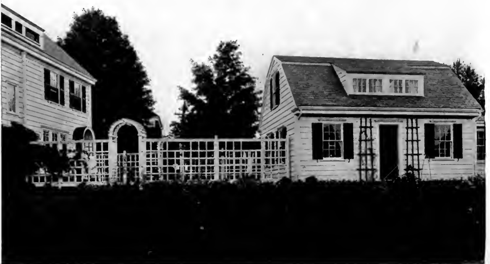
TOOL HOUSE AND GARAGE—RESIDENCE OF MISS E. S. CUSHING, WABAN, MASS. Grandgent & Elwell, Architects.
