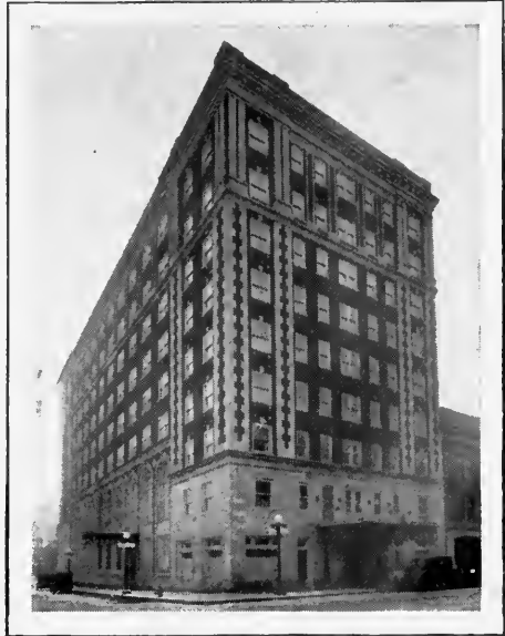
The Fort Steuben Hotel, Steubenville, Ohio: Frederic Webber, Phila., Architect; J. D. Johnson Co., Inc., Phila., Jobbers; Modern Plumbing & Heating Co., Phila., Plumbers
