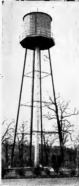
A 30,000 gallon water tank of 3" Redwood. Installed at the Pittsburgh Field Club for club house water system, watering the greens and supplying water for swimming pool.
