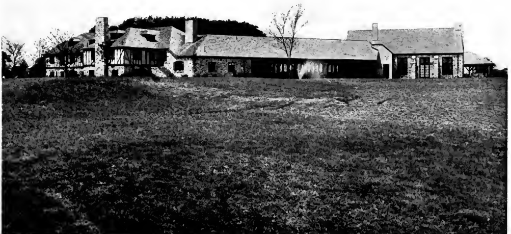
VIEW OVERLOOKING LINKS—NORWOOD GOLF CLUB, LONG BRANCH, N. J. Harry Allan Jacobs, Architect.
