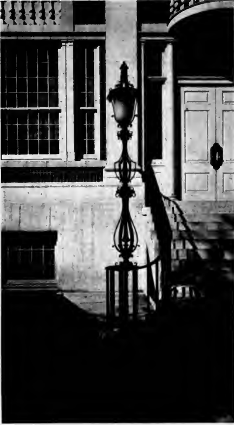
DETAIL OF STEPS—HIGH SCHOOL, PORT CHESTER, N. Y.
