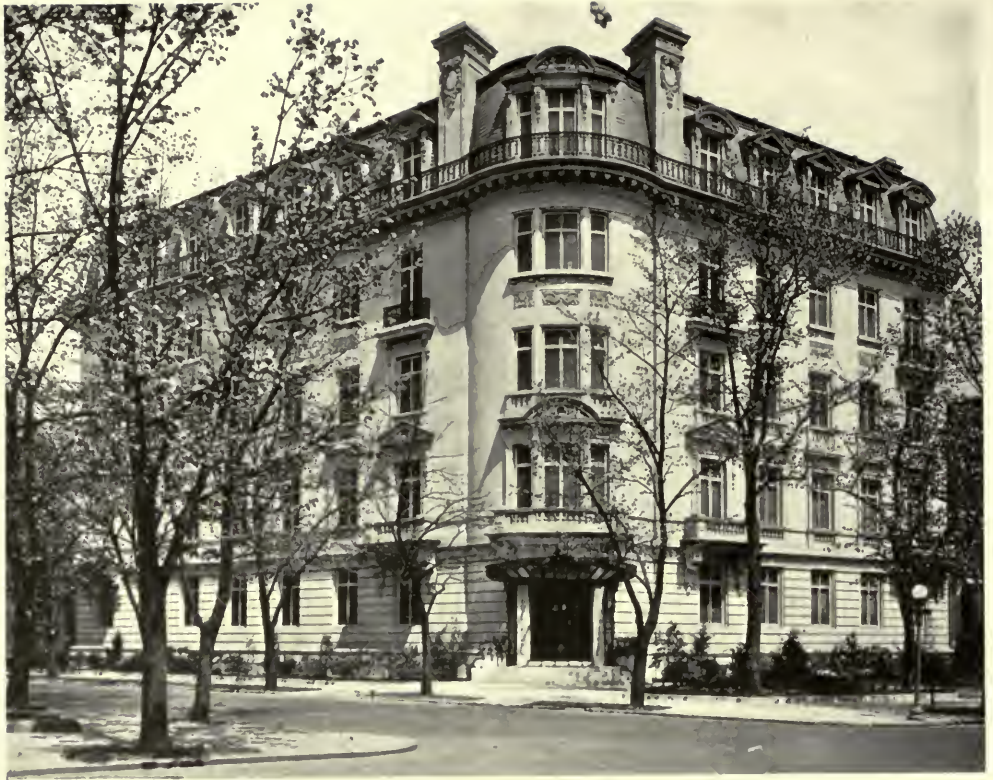
FIG. 130.—APARTMENT HOUSE AT 1785 MASSACHUSETTS AVENUE, WASHINGTON, D. C. J. H. De Sibour, Architect.
