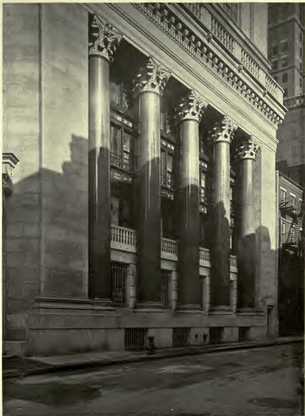
LOWER PORTION OF BEAVER STREET FAÇADE, SEABOARD NATIONAL BANK, NEW YORK CITY. ALFRED C. BOSSOM, ARCHITECT.
