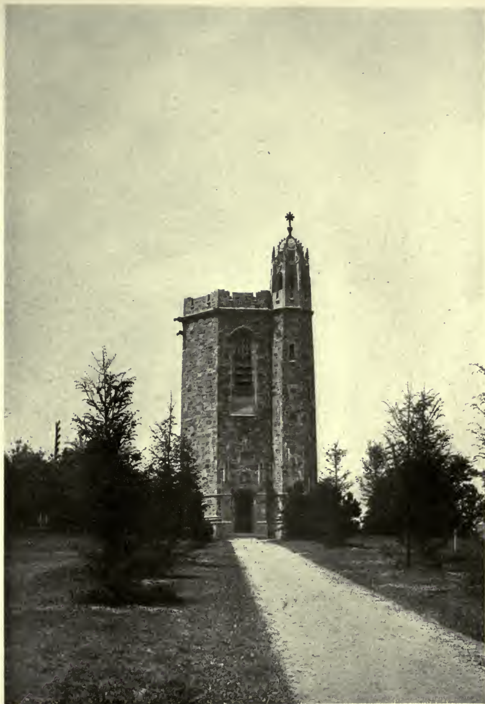
WATER TOWER—CEMETERY OF THE GATE OF HEAVEN. C. W. LEAVITT, ARCHITECT.
