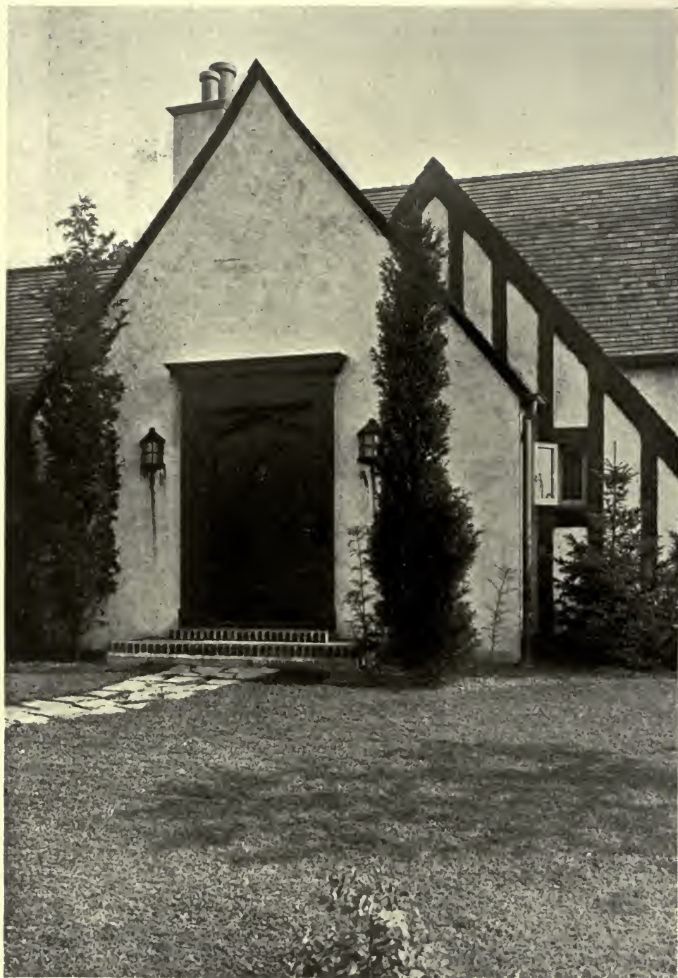
ENTRANCE DETAIL—RESIDENCE OF PAUL SHIELDS, ESQ., GREAT NECK, LONG ISLAND. C. I. PATTERSON, ARCHITECT.
