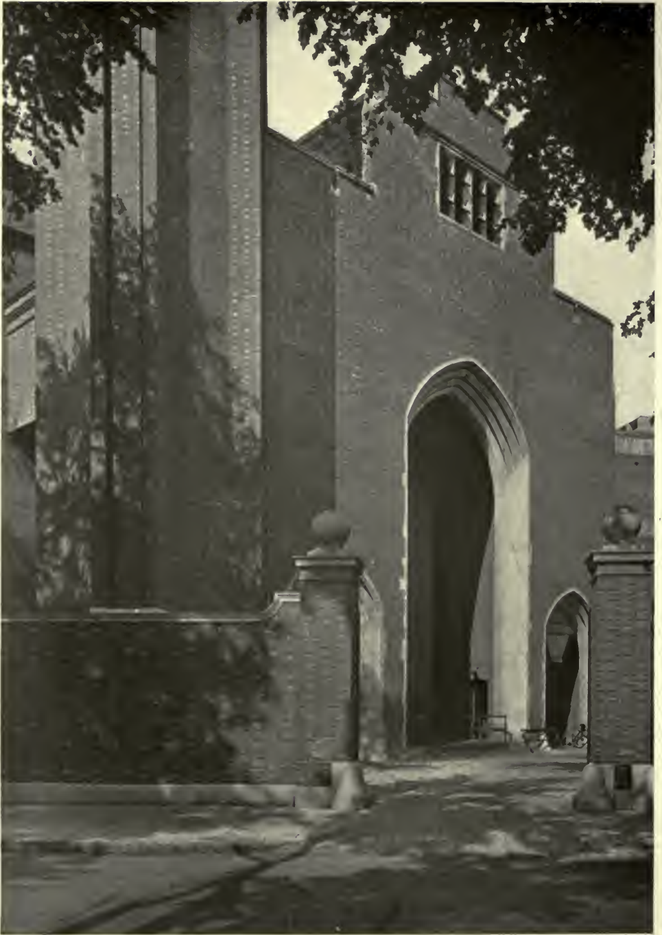
YALE POWER HOUSE, NEW HAVEN, CONN. DAY & KLAUDER. ARCHITECTS.
