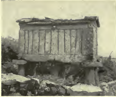
VERY ANCIENT CORNCRIB, NOW ABANDONED; GRANITE ROOF SLABS ARE NINE FEET LONG.
