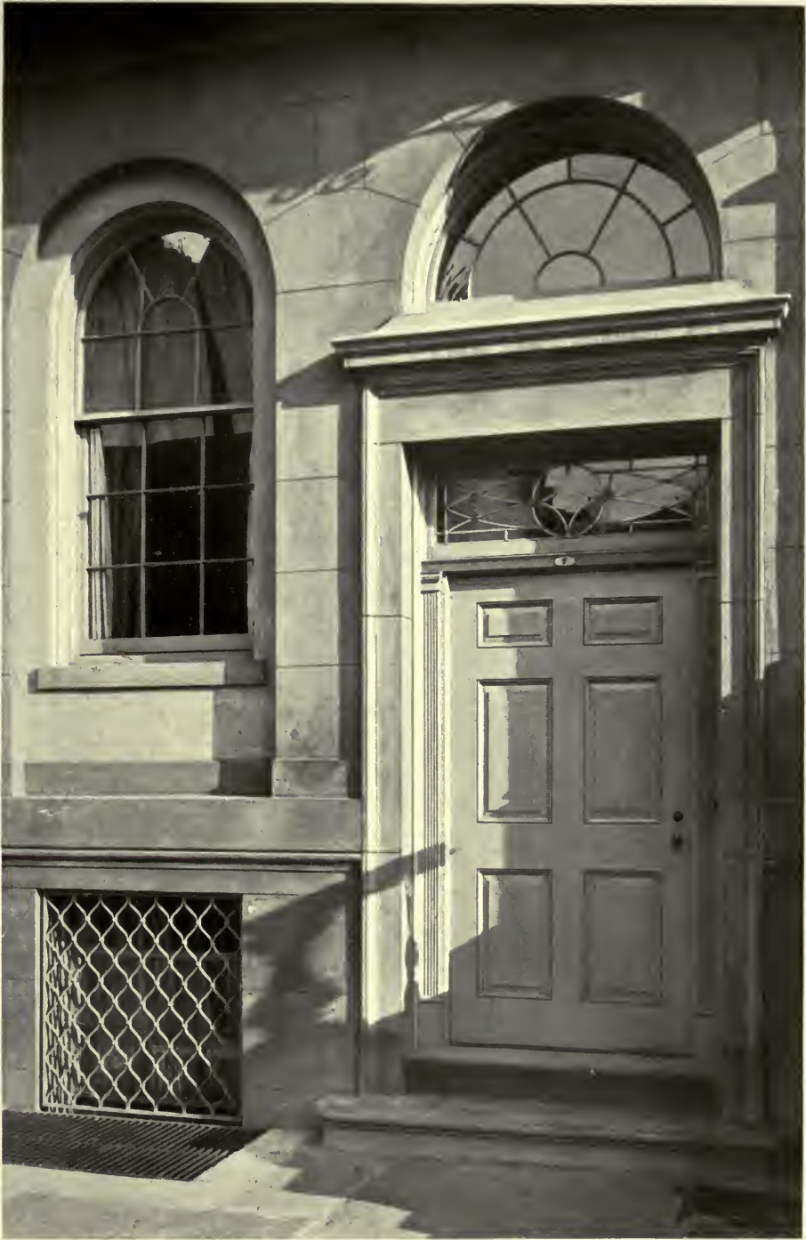
ENTRANCE DOOR—RESIDENCE OF MRS. H. L. CAMMANN, 7 SUTTON PLACE, NEW YORK CITY. WILLIAM F. DOMINICK, ARCHITECT.
