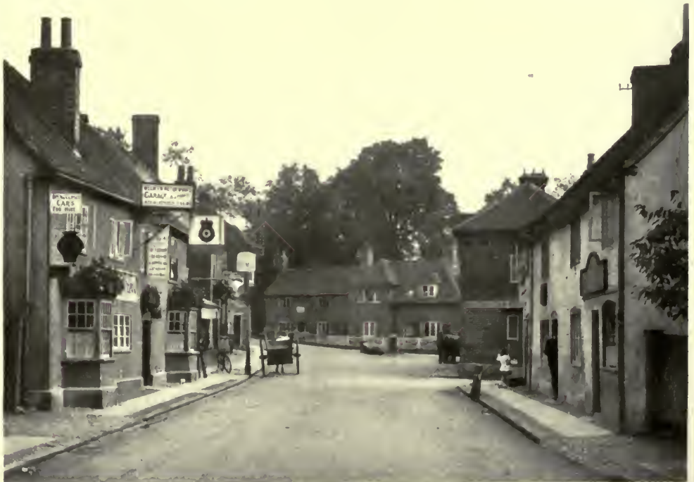
WELWYN OF TODAY, WHERE THE NEW GARDEN CITY WILL BE BUILT.
