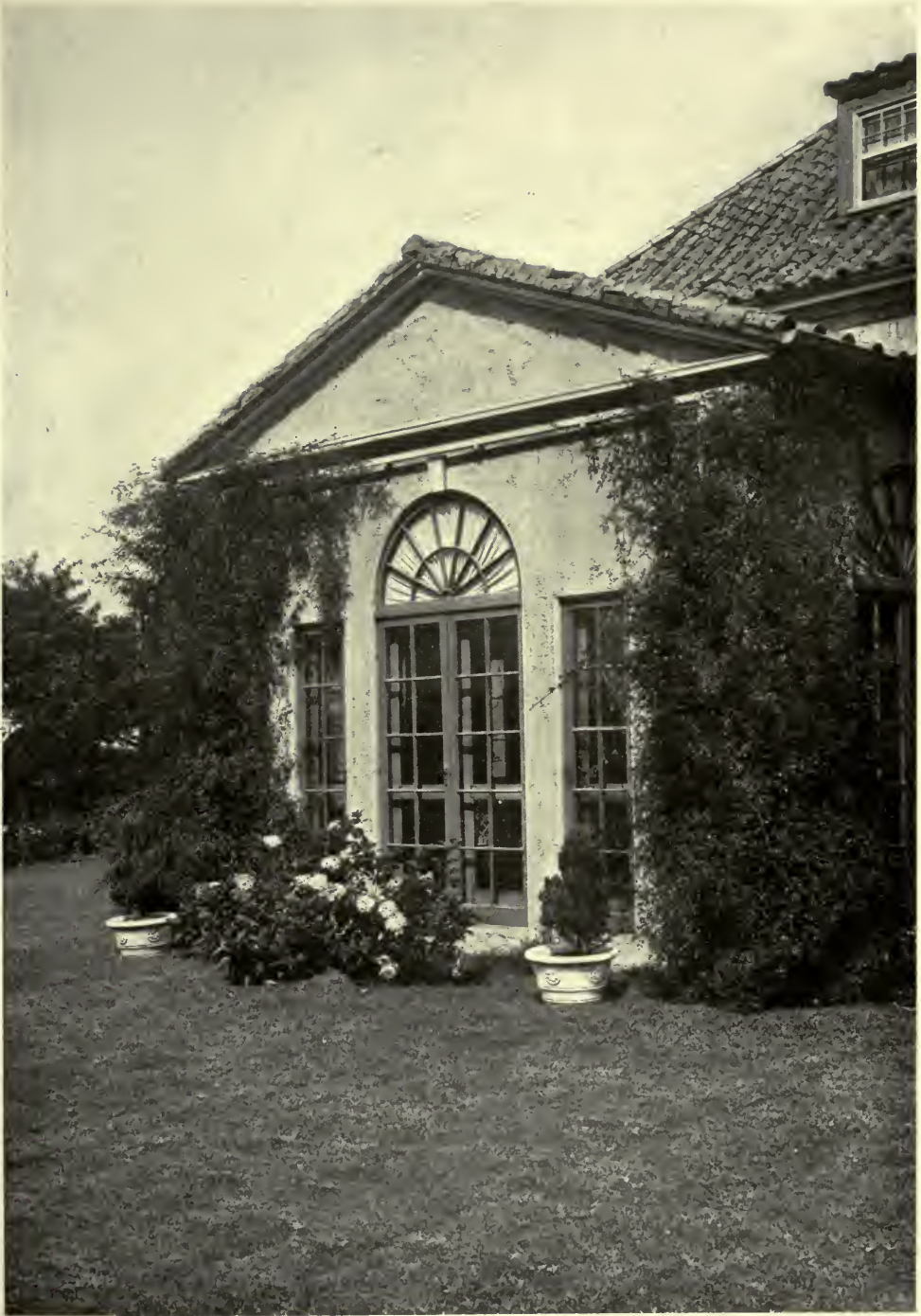
SUN PORCH DETAIL—RESIDENCE OF H. W. HARDINGE, ESQ., FOREST HILLS, LONG ISLAND. WILLIAM LAWRENCE BOTTOMLEY, ARCHITECT.
