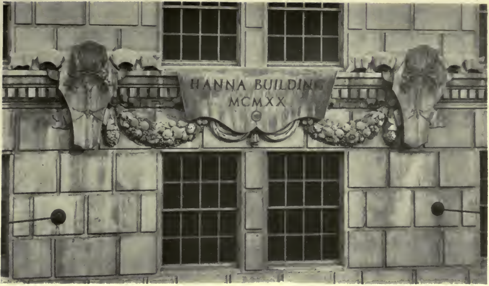
DETAIL OVER MAIN ENTRANCE
