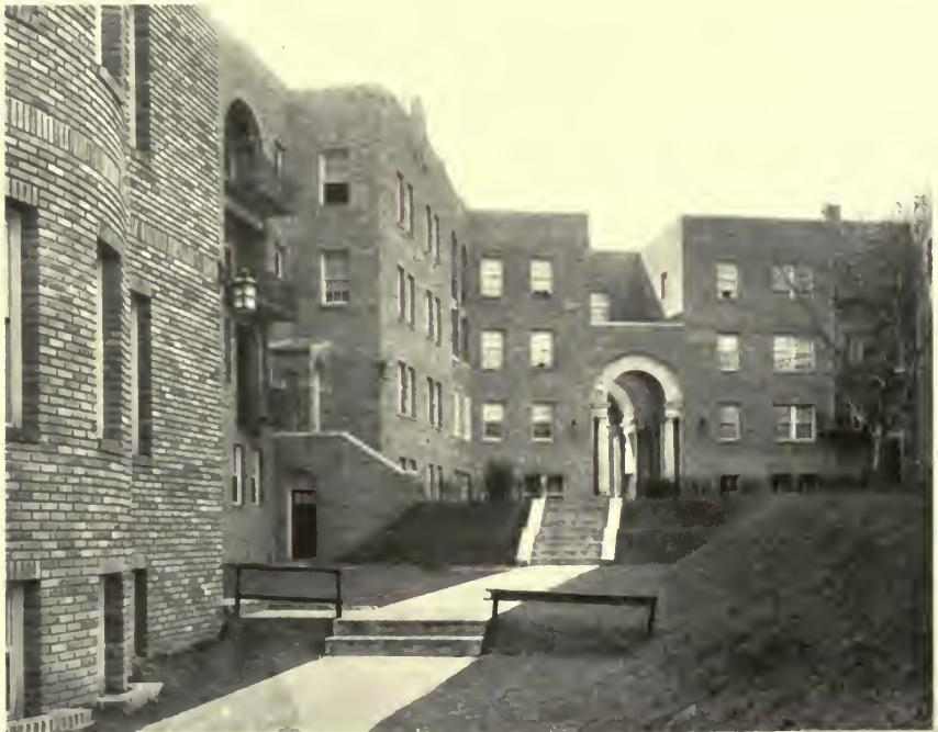
FIG. 111. VIEW IN COURTYARD—WINDSOR COURT APARTMENTS, WALBROOK, BALTIMORE, MD. Clyde N. Friz, Architect.
