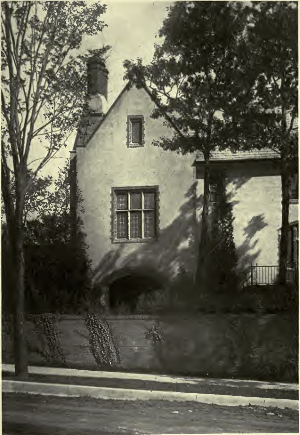
DETAIL OF MAIN FAÇADE—RESIDENCE OF A. L. SEARLE, ESQ., MINNEAPOLIS, MINN. TROWBRIDGE & ACKERMAN, ARCHITECTS.
