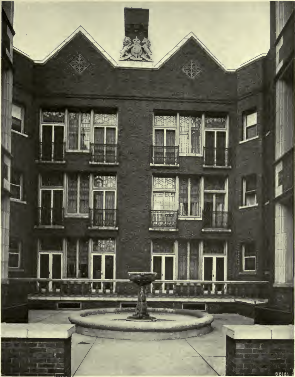
FIG. 91. INTERIOR OF COURTYARD.
