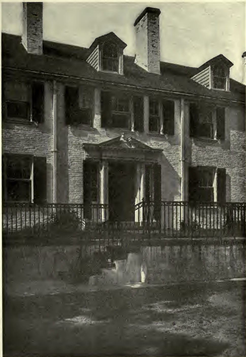
RESIDENCE OF GEORGE DE FOREST LORD, ESQ., WOODMERE, LONG ISLAND. WILLIAM HARMON BEERS, ARCHITECT. FRANK C. FARLEY, ASSOCIATE.
