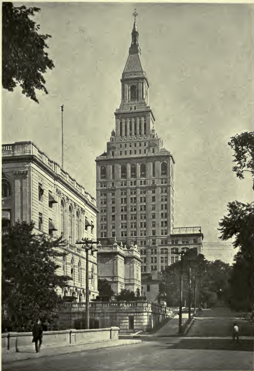
TRAVELERS' INSURANCE COMPANY BUILDING, HARTFORD, CONN. DONN BARBER, ARCHITECT.
