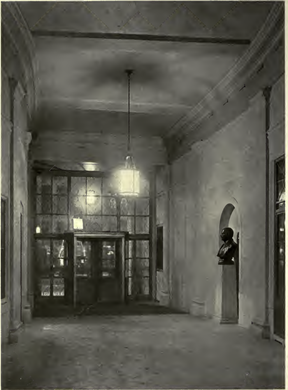
CORRIDOR—HANNA BUILDING, CLEVELAND, OHIO. CHARLES A. PLATT, ARCHITECT.
