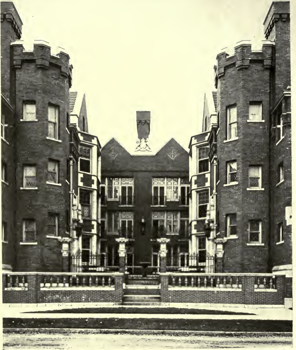
FIG. 89. GENERAL VIEW OF COURTYARD.
