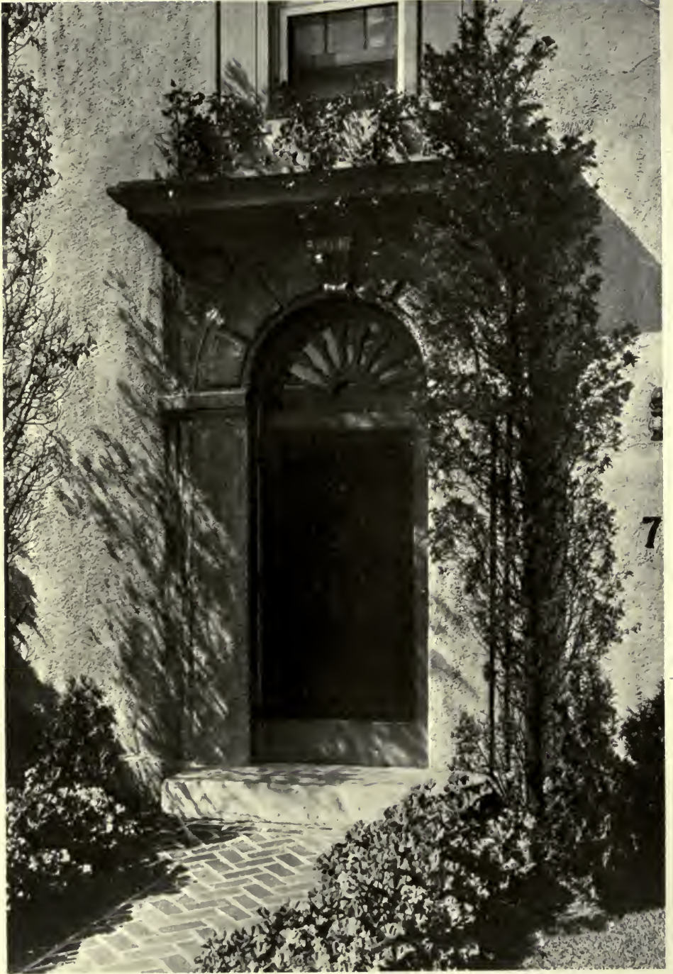
ENTRANCE DETAIL — RESIDENCE OF H. W. HARDINGE, ESQ., FOREST HILLS, LONG ISLAND. WILLIAM LAWRENCE BOTTOMLEY, ARCHITECT.
