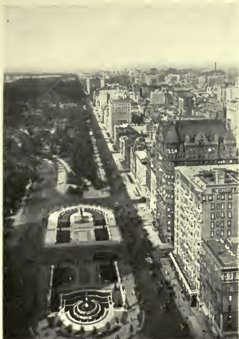
Plaza designed by Mr. Hastings at entrance to Central Park, New York City, co-ordinating the Sherman Monument and the Pulitzer Memorial Fountain, and reflecting the character of the surroundings.
