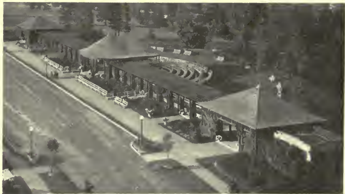
The design and arrangement of this Concert Group with Central Music Pavilion, in Seattle, are admirable. Its location on a through boulevard proved so ill-chosen, however, because of the noise interference and traffic risk, as to necessitate its complete abandonment and the erection of a stand in a new location several hundred yards from the boulevard.
