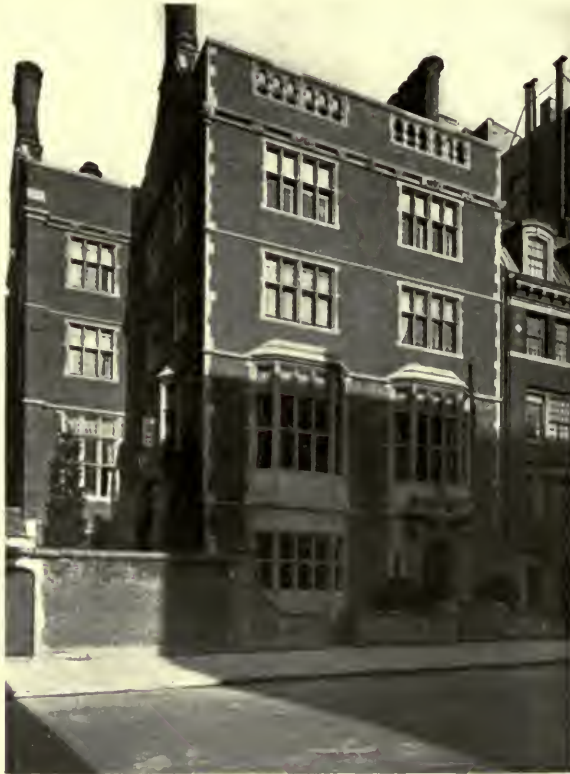
RESIDENCE OF THOMAS W. LAMONT, ESQ., NEW YORK CITY. Walker & Gillette, Architects.
