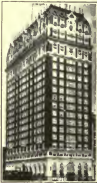
BLACKSTONE HOTEL, CHICAGO, ILL. Marshall and Fox, Architects.
