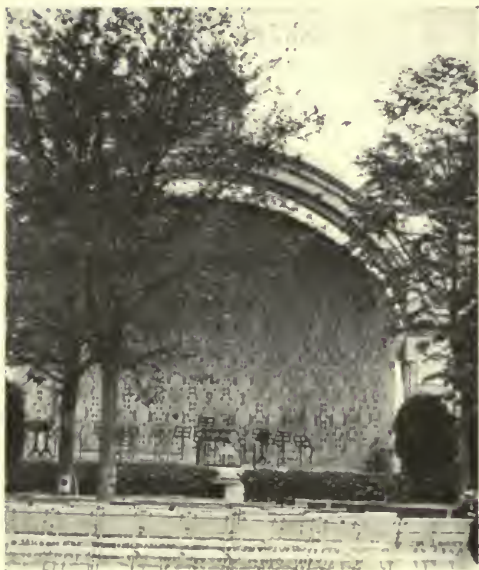
A Shell Type Stand at Lucerne, Switzerland. It shows enough vertical surface below the springing of the half dome and a pleasing overall decoration. Inconspicuous doors lead to rear service room. The stand is flanked by fountains, seats and high hedges, and fronts on the lake promenade.
