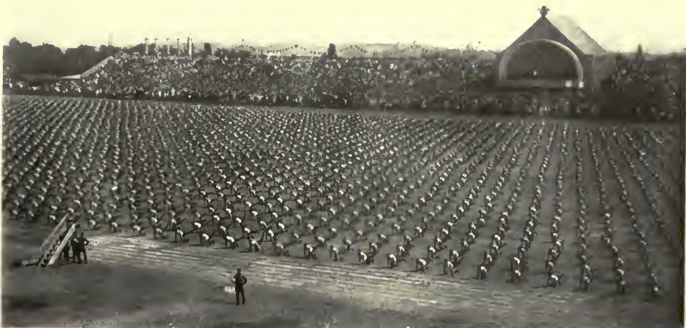
A variation of the shell type at Prague, Czechoslovakia, accommodating one hundred and twenty pieces and providing dressing and service rooms below. It is of rough frame construction with painted decorations.
