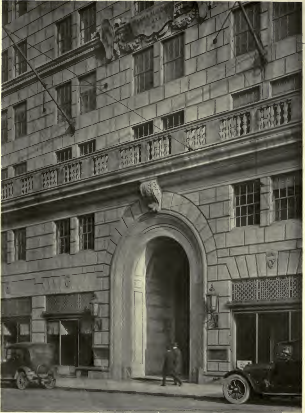
MAIN ENTRANCE—HANNA BUILDING, CLEVELAND, OHIO. CHARLES A. PLATT, ARCHITECT.
