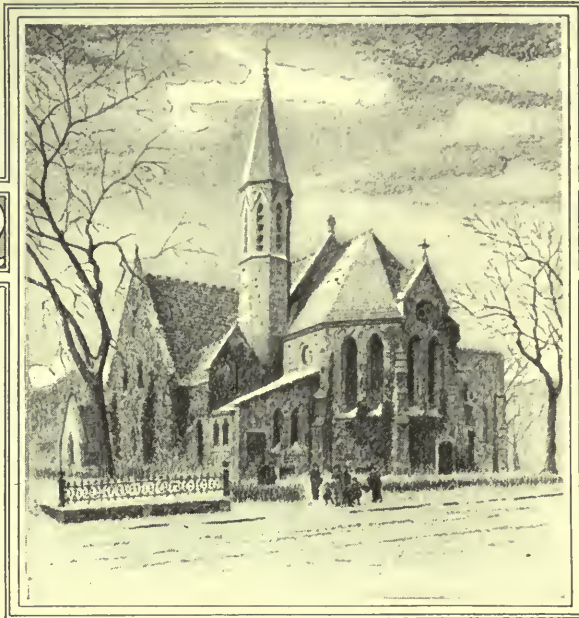
From a drawing by Wesley Bonestell © ARCO 1922 Architects: Henry M. Congdon & Son, New York TRINITY CHURCH, Waterbury, Connecticut, where two IDEAL TYPE A HEAT MACHINES are paying for themselves in the fuel they save.
