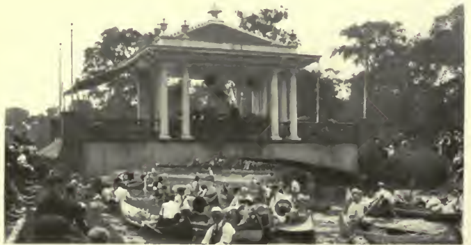
This Detroit pavilion, like most of the Belle Isle features, is a happy incident along one of the canoe channels. The lowered ceiling and lifted cornice form a sounding board without losing the lintel line. Van Leyen & Schilling, Architects.
