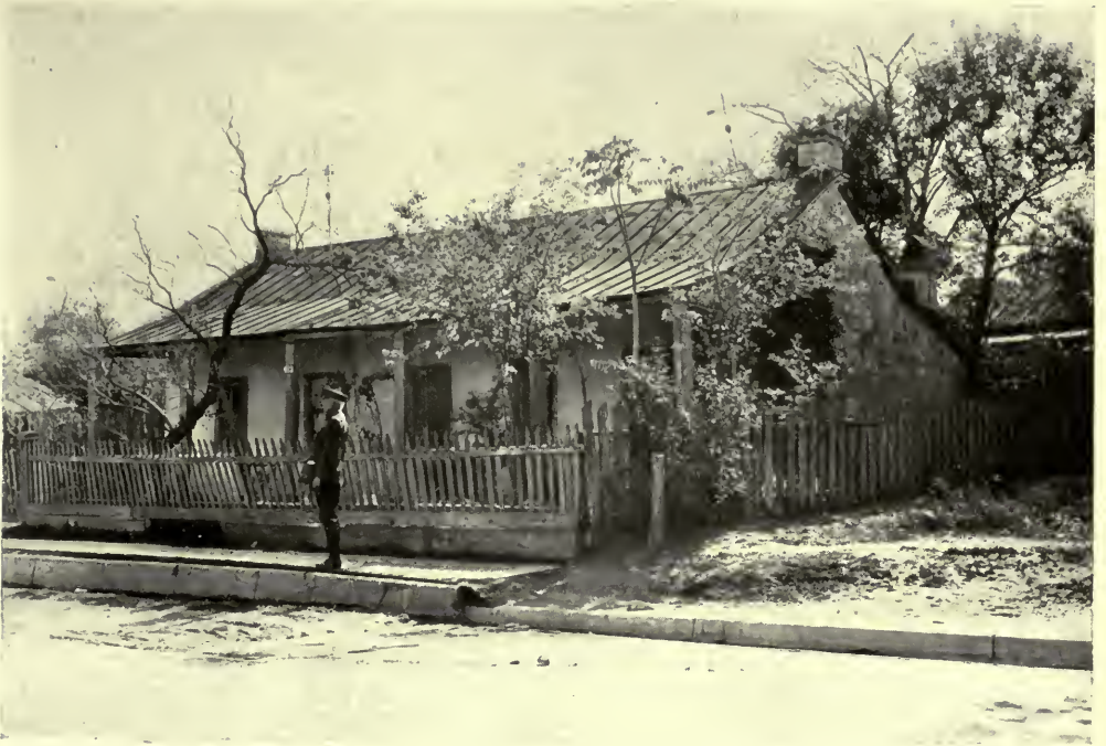
THE OLD ROOF LINE HAS BEEN PRESERVED THOUGH OLD MATERIAL HAS GIVEN WAY TO NEW.
