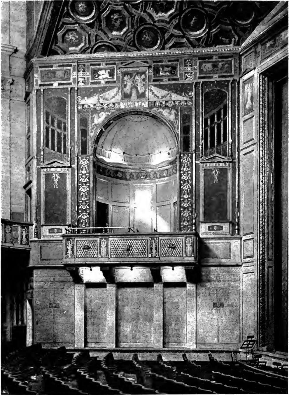
BOX IN HANNA THEATRE—HANNA BUILDING ANNEX, CLEVELAND, OHIO. CHARLES A. PLATT, ARCHITECT.
