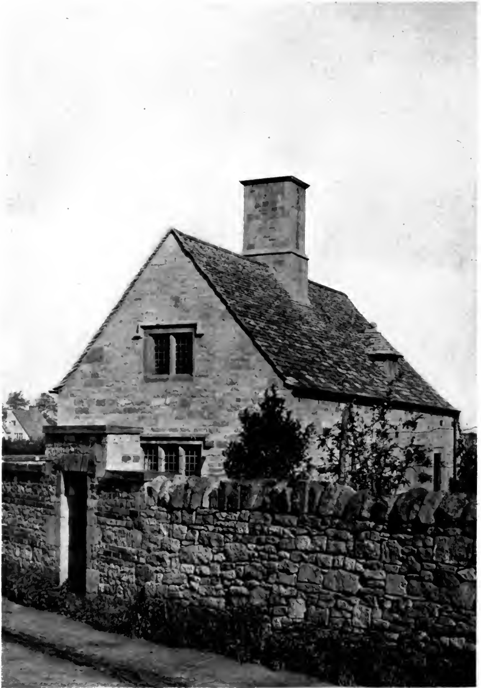
SOUTH AND EAST SIDES—COTTAGE AT LYGON ARMS, BROADWAY, WORCESTERSHIRE, E. S. CARPENTER, ARCHITECT.
