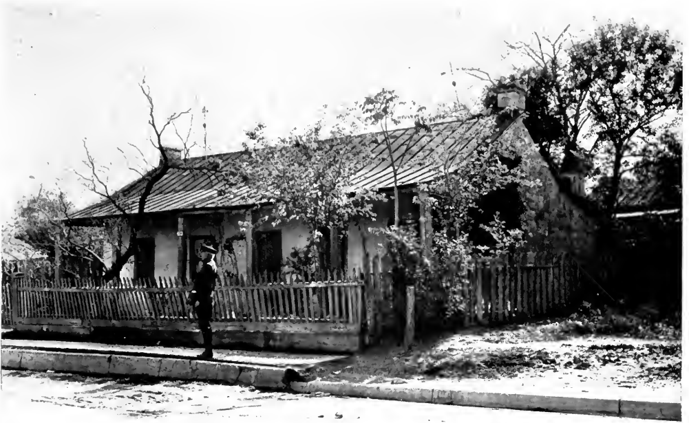
THE OLD ROOF LINE HAS BEEN PRESERVED THOUGH OLD MATERIAL HAS GIVEN WAY TO NEW.
