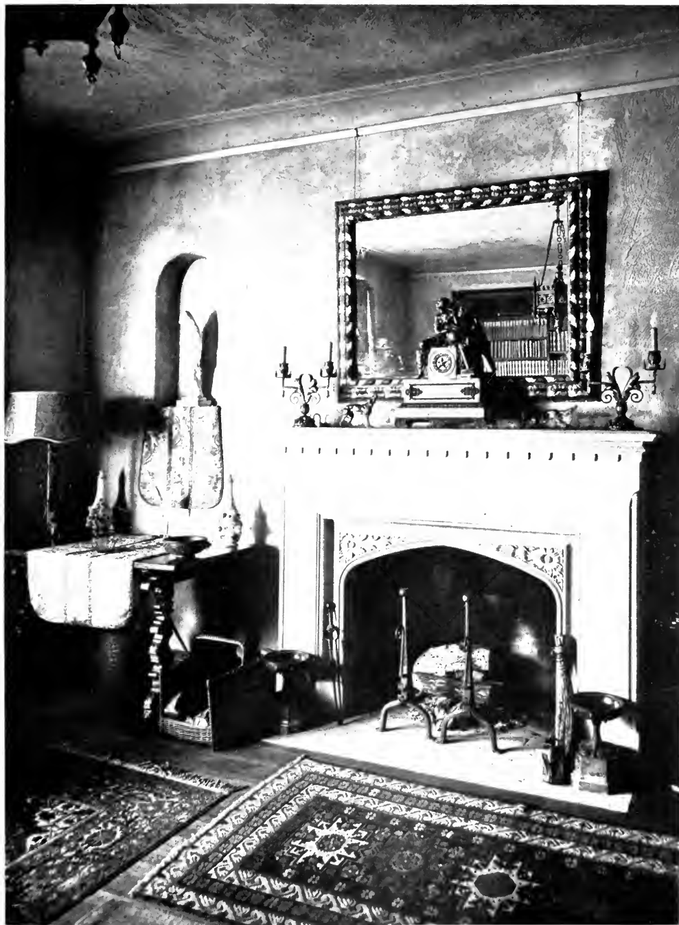
FIREPLACE—RESIDENCE OF MRS. H. L. CAMMANN, 7 SUTTON PLACE, NEW YORK CITY. WILLIAM F. DOMINICK, ARCHITECT.
