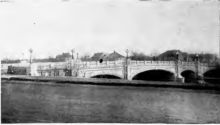
Capital Avenue Bridge, Indianapolis, Ind. The Cleary-Kuert Co., Builders. Geo. E. Kessler, Landscape Artist
