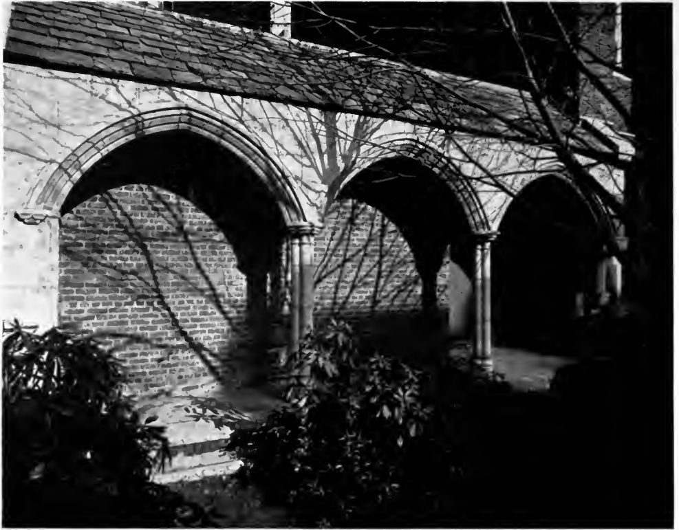
CLOISTER—RESIDENCE OF THOMAS W. LAMONT, ESQ., NEW YORK CITY. Walker & Gillette, Architects.
