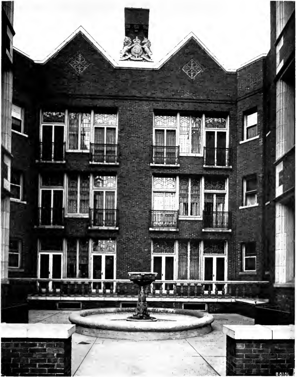
FIG. 91. INTERIOR OF COURTYARD.
