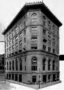
Cotton Exchange Bldg., New Orleans Favrot & Livaudais, Architects Selden Breck Const. Co., Contractors
