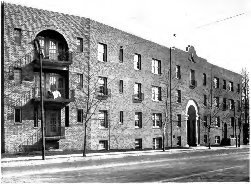
FIG. 110. VIEW OF EXTERIOR WINDSOR COURT APARTMENTS, WALBROOK, BALTIMORE, MD. Clyde N. Friz, Architect.
