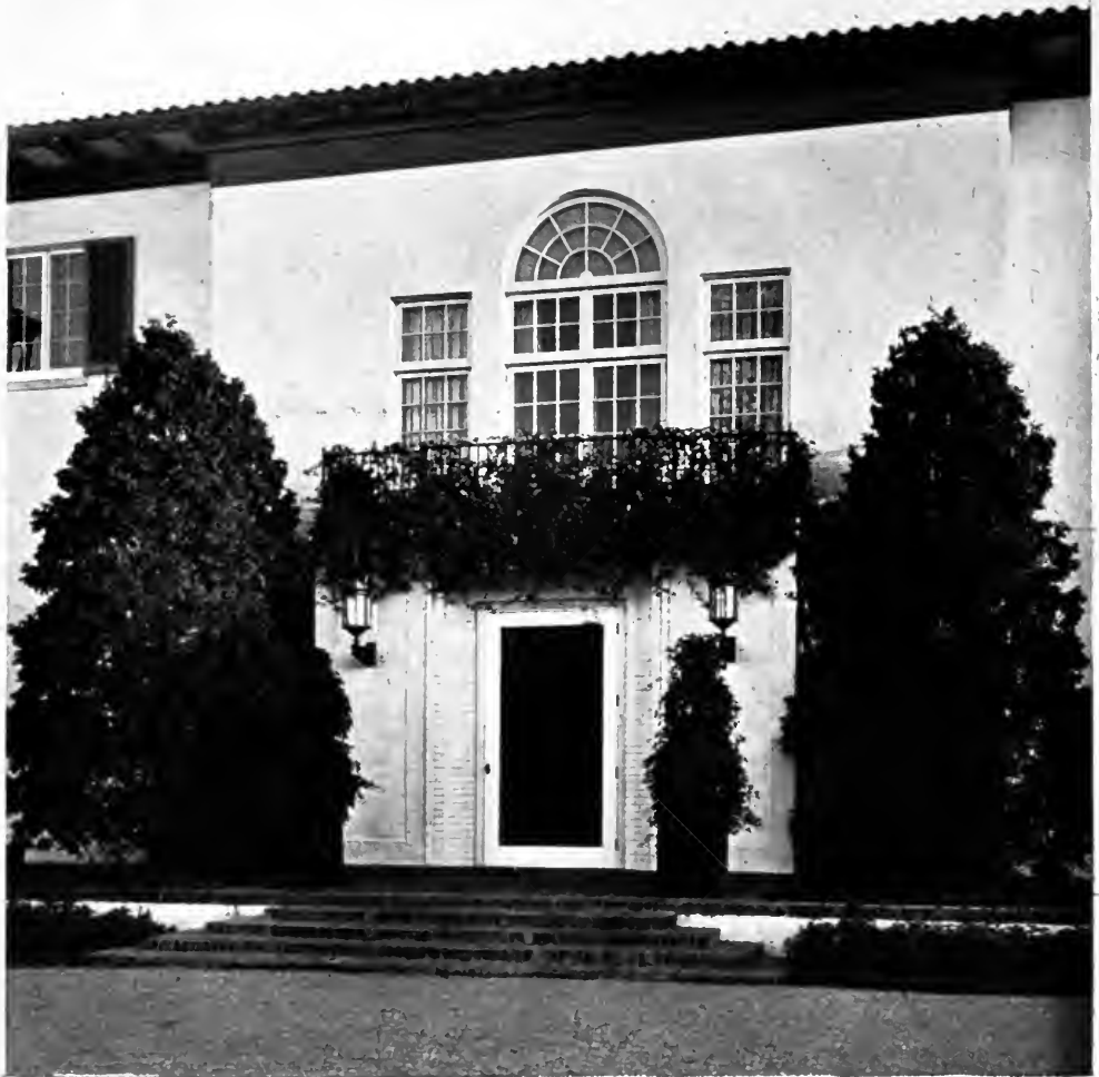
DETAIL OF ENTRANCE—RESIDENCE OF JOHN L. BUSHNELL, ESQ., SPRINGFIELD, OHIO. Lewis Colt Albro, Architect.
