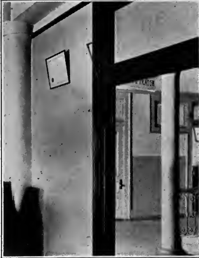
Moore Building, San Antonio. Partitions are made of 27-gauge Kno-Burn with channels 12" on centers.
