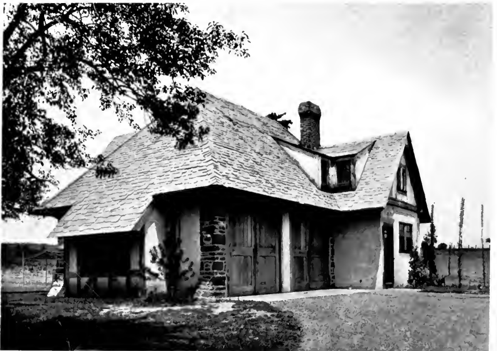
GARAGE—HOUSE OF MRS. WILLIAM K. RYAN, HAVERFORD, PA. Emil H. Kleeman, Architect.
