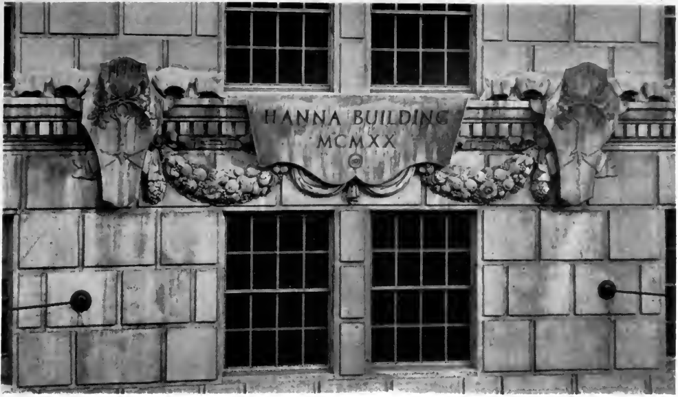
DETAIL OVER MAIN ENTRANCE
