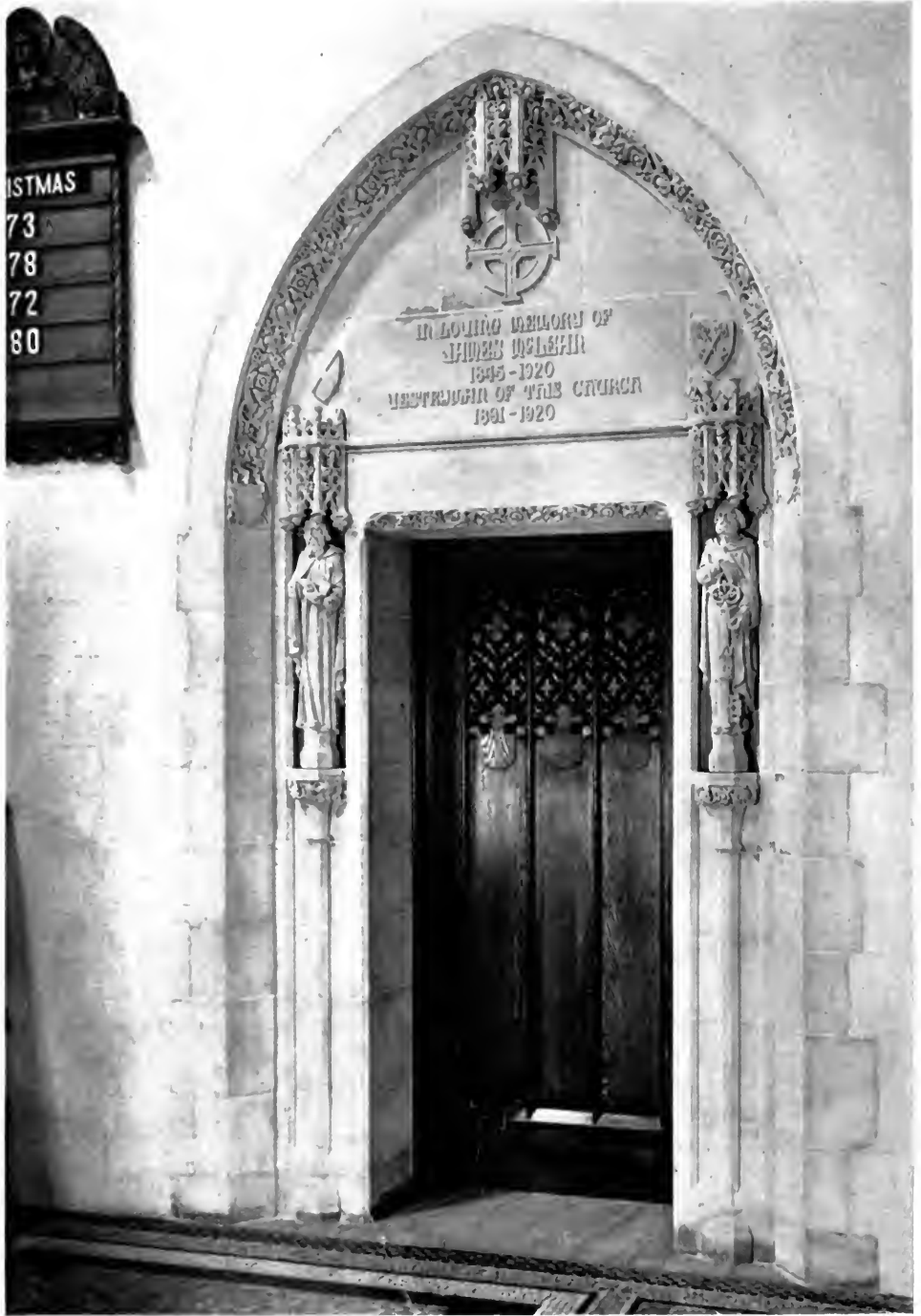
DOORWAY — CHURCH OF THE INCARNATION, NEW YORK CITY. ALLEN & COLLENS, ARCHITECTS.
