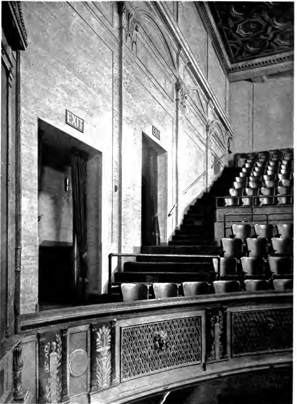
WALL AND BALCONY IN HANNA THEATRE—HANNA BUILDING ANNEX, CLEVELAND, OHIO. CHARLES A. PLATT, ARCHITECT.
