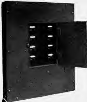
Type T—Safety Panel Board with Inner Door open, giving access to switches.
