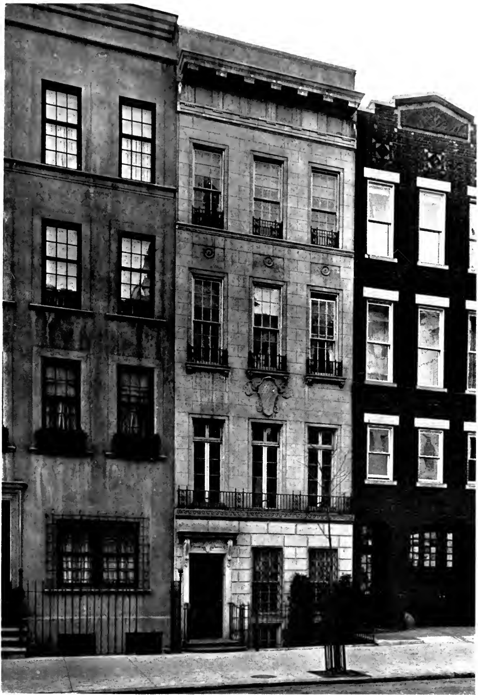
GENERAL ELEVATION—RESIDENCE ON 75TH STREET, NEW YORK CITY. HARRY M. CLAWSON, ARCHITECT.
