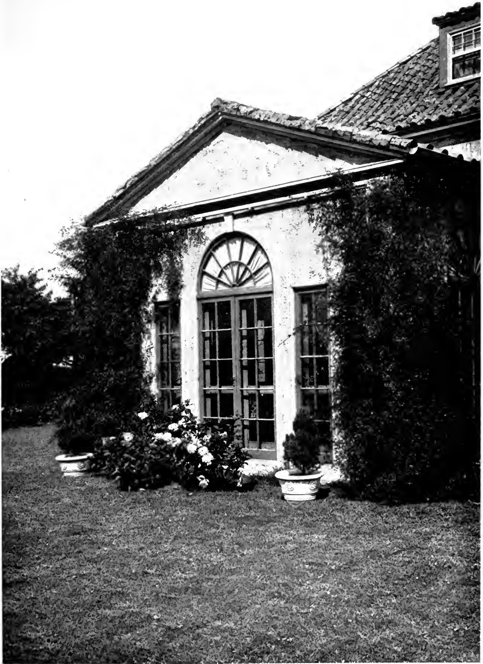
SUN PORCH DETAIL—RESIDENCE OF H. W. HARDINGE, ESQ., FOREST HILLS, LONG ISLAND. WILLIAM LAWRENCE BOTTOMLEY, ARCHITECT.
