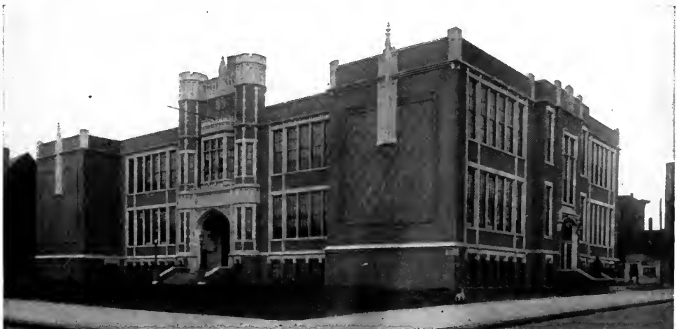
CENTRAL SCHOOL, UNIONTOWN, PA. TRUSCON STEEL SASH AND TRUSCON REINFORCING STEEL. Andrew P. Cooper, Archt. Geo. M. Hall Co., Contractors.
