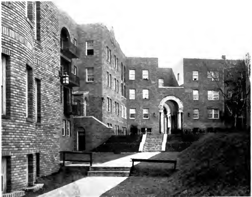
FIG. 111. VIEW IN COURTYARD—WINDSOR COURT APARTMENTS, WALBROOK, BALTIMORE, MD. Clyde N. Friz, Architect.
