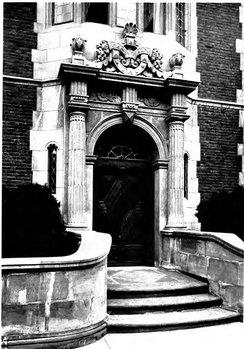
ENTRANCE—RESIDENCE OF THOMAS W. LAMONT, ESQ., NEW YORK CITY. WALKER & GILLETTE, ARCHITECTS.
