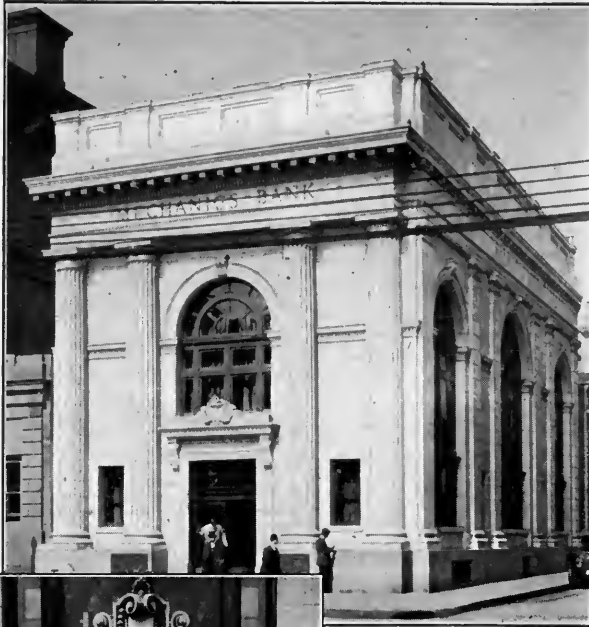
The Mechanics Bank, New Haven, Connecticut. L. W. Robinson, Architect. Constructed of Vermont Mountain White Marble.
