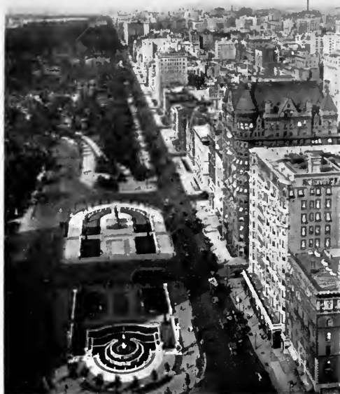
Plaza designed by Mr. Hastings at entrance to Central Park, New York City, co-ordinating the Sherman Monument and the Pulitzer Memorial Fountain, and reflecting the character of the surroundings.
