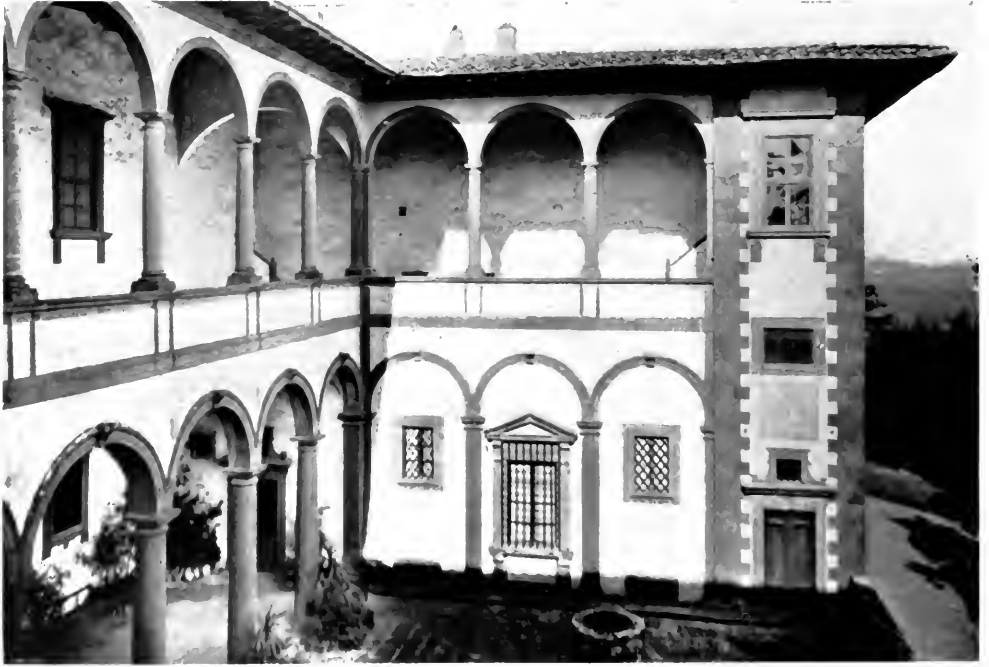
GROUND AND FIRST FLOOR LOGGIAS VILLA DEI COLLAZZI, TAVARNUZZE, TUSCANY.
