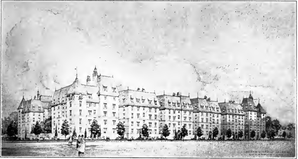
GROUPED APARTMENT BUILDINGS FOR THE QUEENSBORO CORPORATION AT JACKSON HEIGHTS, NEW YORK CITY.
