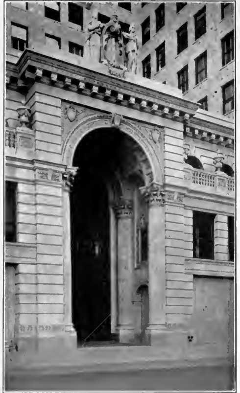
PACIFIC MUTUAL BUILDING LOS ANGELES, CALIF.
