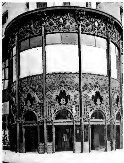
CORNER ENTRANCE, THE SCHLESINGER & MAYER BUILDING, CHICAGO, ILL. LOUIS H. SULLIVAN, ARCHITECT.
