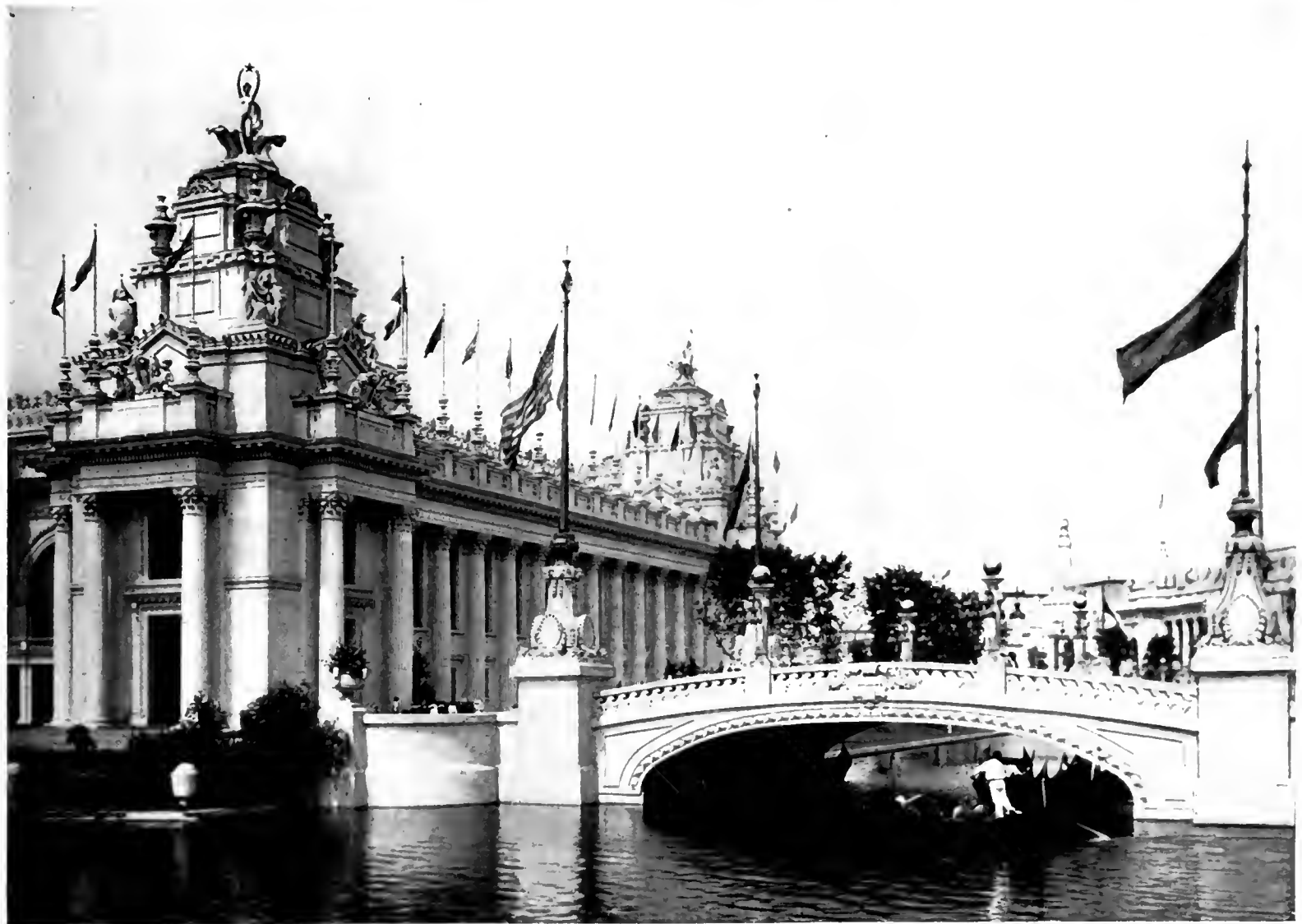
XVIII. NORTH SIDE OF THE ELECTRICITY BUILDING FROM THE EAST.
