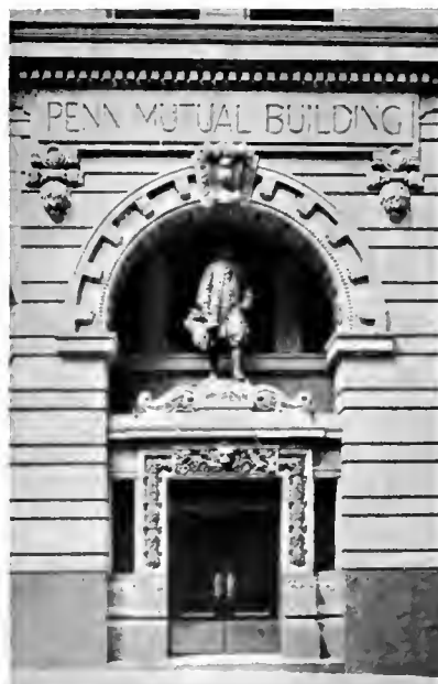
ENTRANCE TO PENN MUTUAL BUILDING, BOSTON. E. V. SEELER, ARCHITECT.
