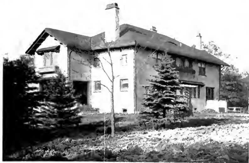
VIEW FROM THE SOUTHWEST
