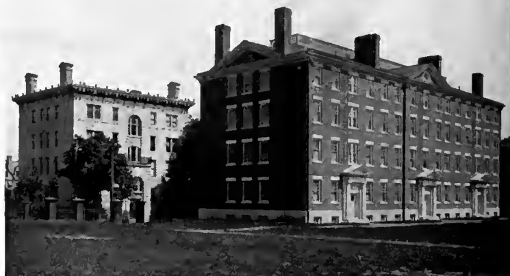
BRUNONIA PRIVATE DORMITORY AND CASWELL. THE LATTER BY HOPPIN & ELY, ARCHITECTS.
