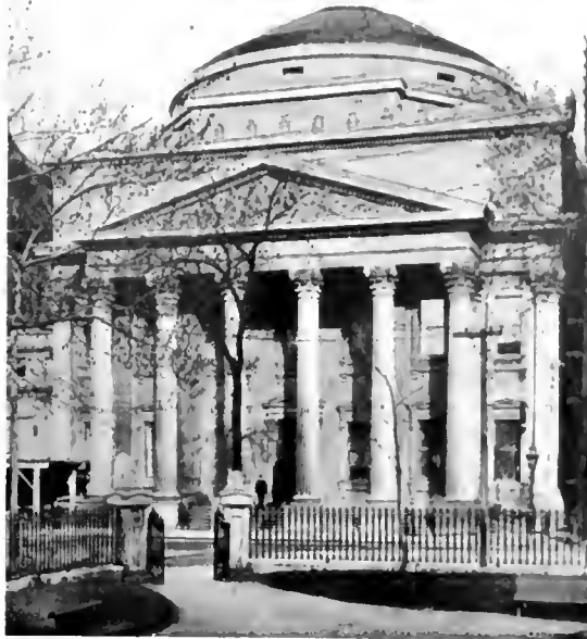
HEAD OFFICES OF THE BANK OF MONTREAL. MCKIM, MEAD & WHITE, TAYLOR, HOGLE & DAVIS, ASSOCIATE ARCHITECTS.
