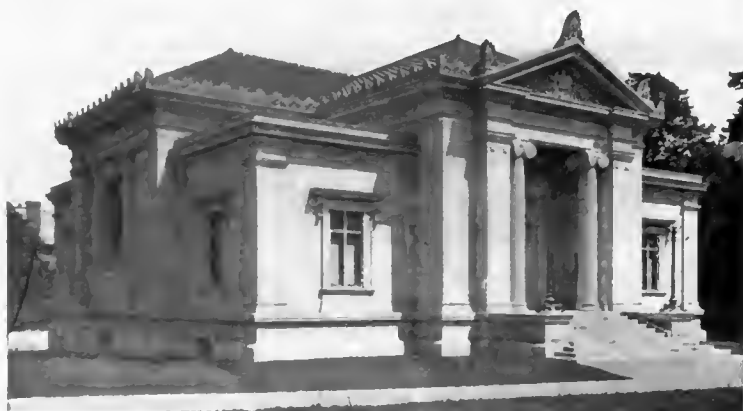
THE JOHN CARTER BROWN MEMORIAL LIBRARY. SHEPLEY, RUTAN & COOLIDGE, ARCHITECTS.
