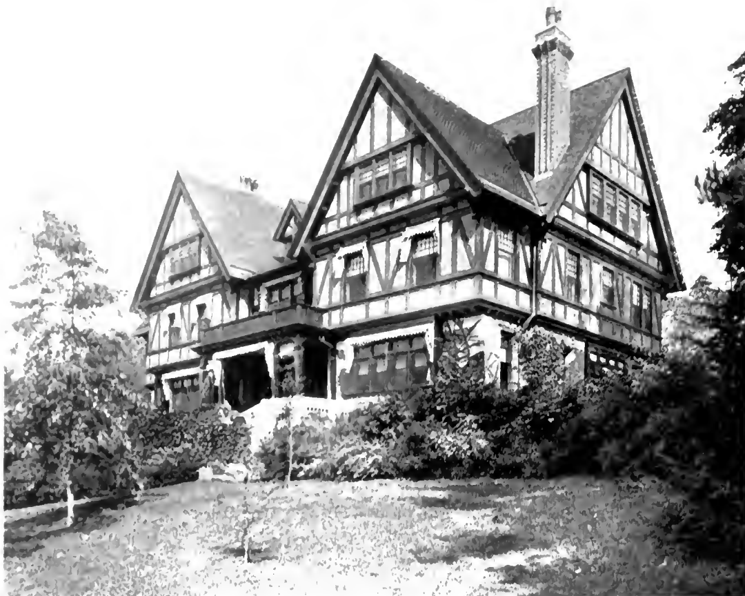
VIEW FROM THE SOUTH.
