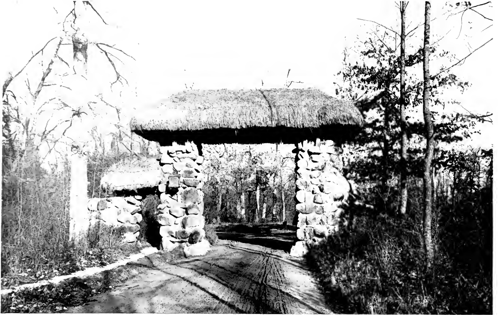
"STONE GATE" ENTRANCE TO THE PRIVATE ROAD TO THE ESTATES OF CYRUS H. McCORMICK, JOHN V. FARWELL, Jr., AND FRANCIS C. FARWELL, LAKE FOREST, ILL. JAMES GAMBLE ROGERS, ARCHITECT, CHICAGO.
