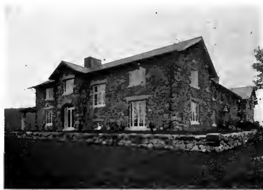
VIEW OF THE NORTH FRONT
