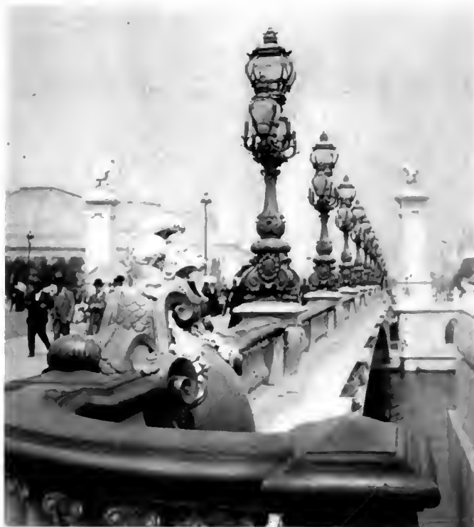
FIG. 9. THE ALEXANDER BRIDGE, PARIS.
