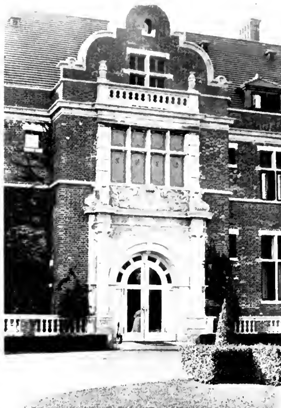
CENTRE MOTIVE OF ENTRANCE FRONT
