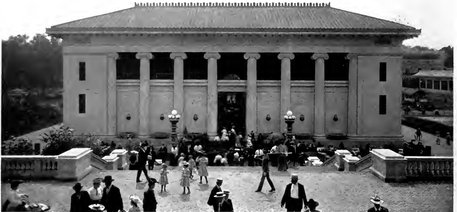
XXXVI. FISHERIES BUILDING FROM THE NORTHEAST.
