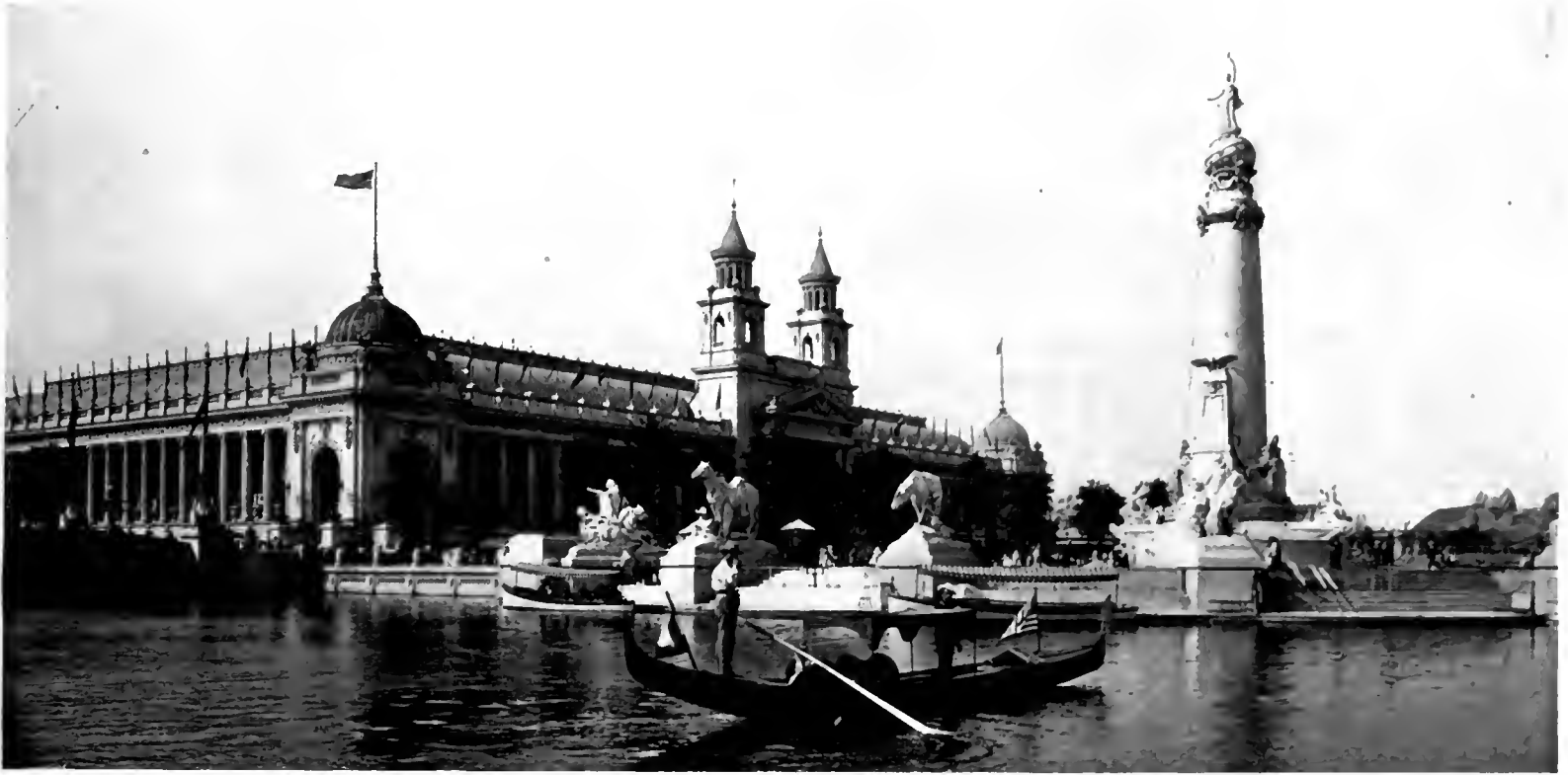
XXVI. EAST SIDE OF THE VARIED INDUSTRIES BUILDING.
