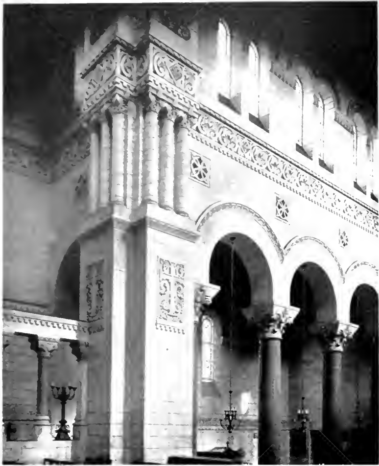
TRANSEPT PIER AND NAVE ARCADE.
