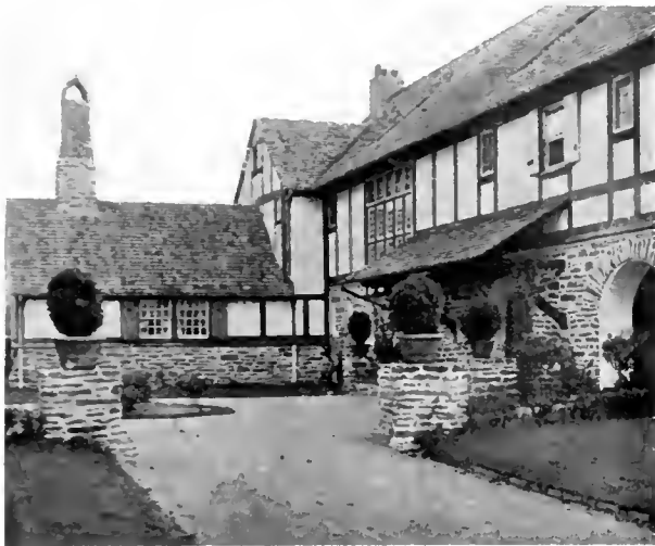
THE COURT, "MILL-BROOK," BRYN MAWR, PA. CHARLES BARTON KEEN, ARCHITECT.
