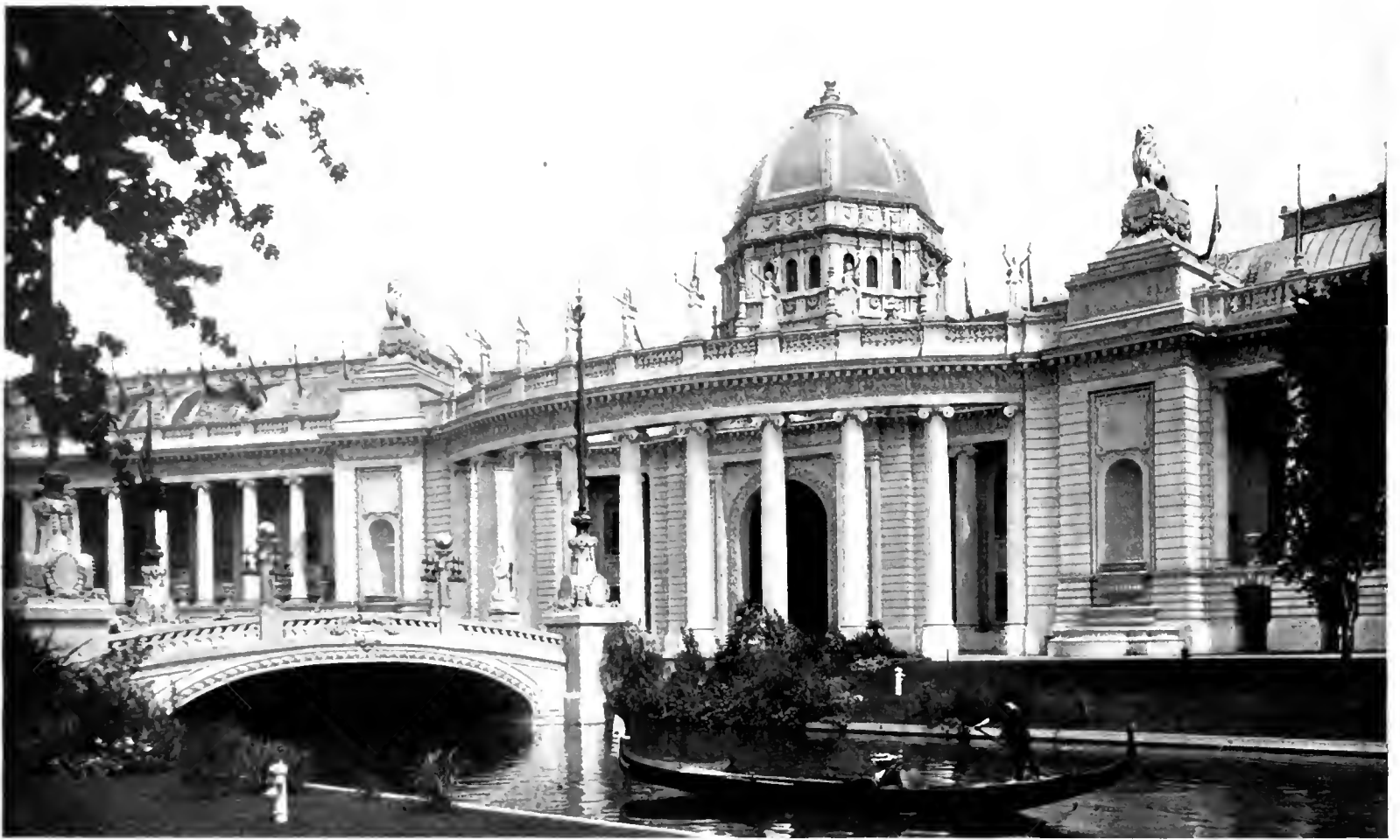
XXVIII. SOUTH ENTRANCE OF VARIED INDUSTRIES BUILDING.
