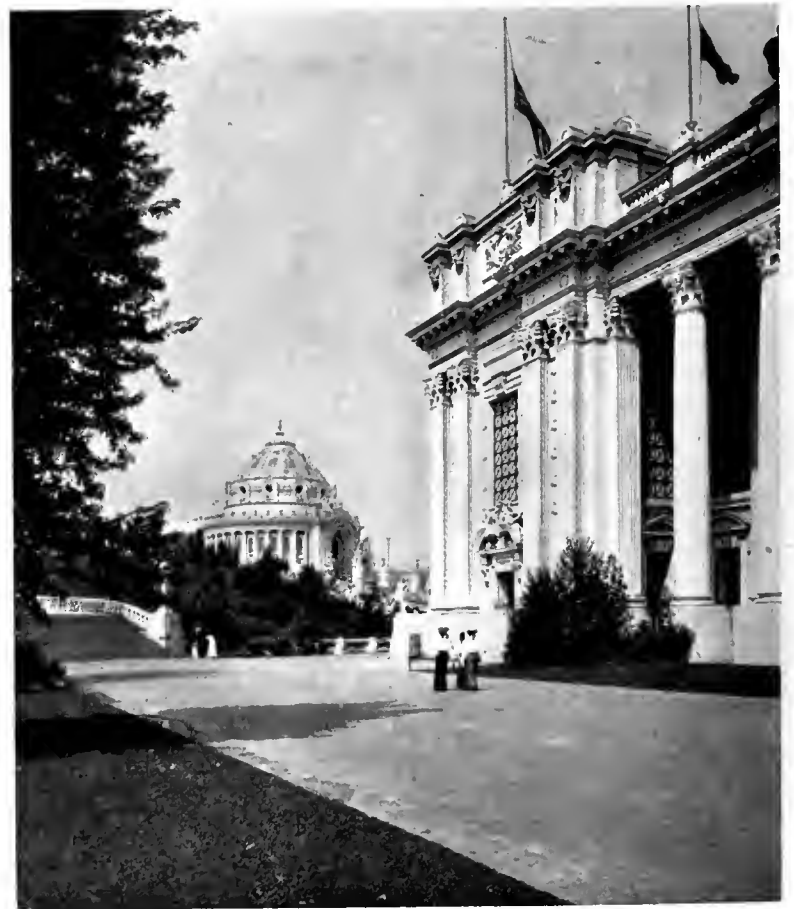
XII. VISTA SOUTHWEST ALONG THE EDUCATION BUILDING.
