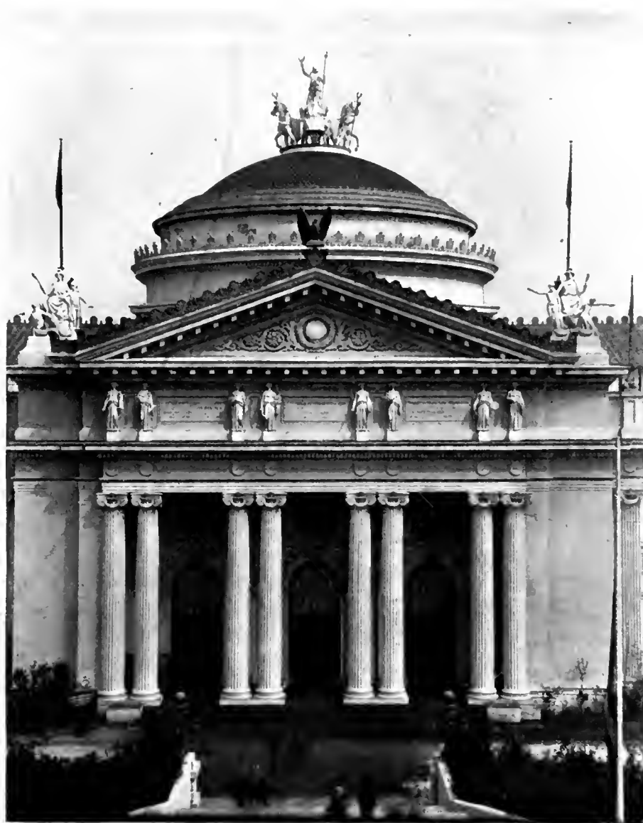
XXXV. U. S. GOVERNMENT BUILDING ENTRANCE DETAIL.
