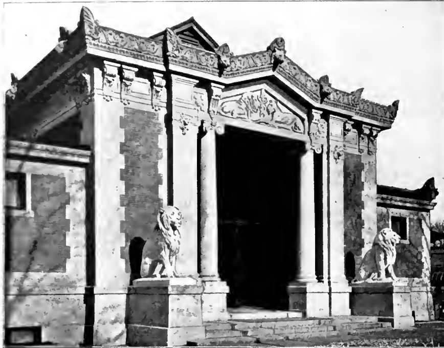
DETAIL OF MAIN ENTRANCE, LION HOUSE, BRONX PARK, NEW YORK CITY. HEINS & LAFARGE, ARCHITECTS.
