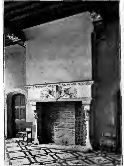
CHIMNEY-PIECE, "HOTEL GRUUTHUUS," BRUGES.
