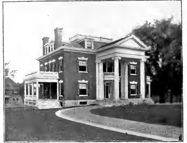
HOUSE AT CINCINNATI, O. ELZENER & ANDERSON, ARCHITECTS.
