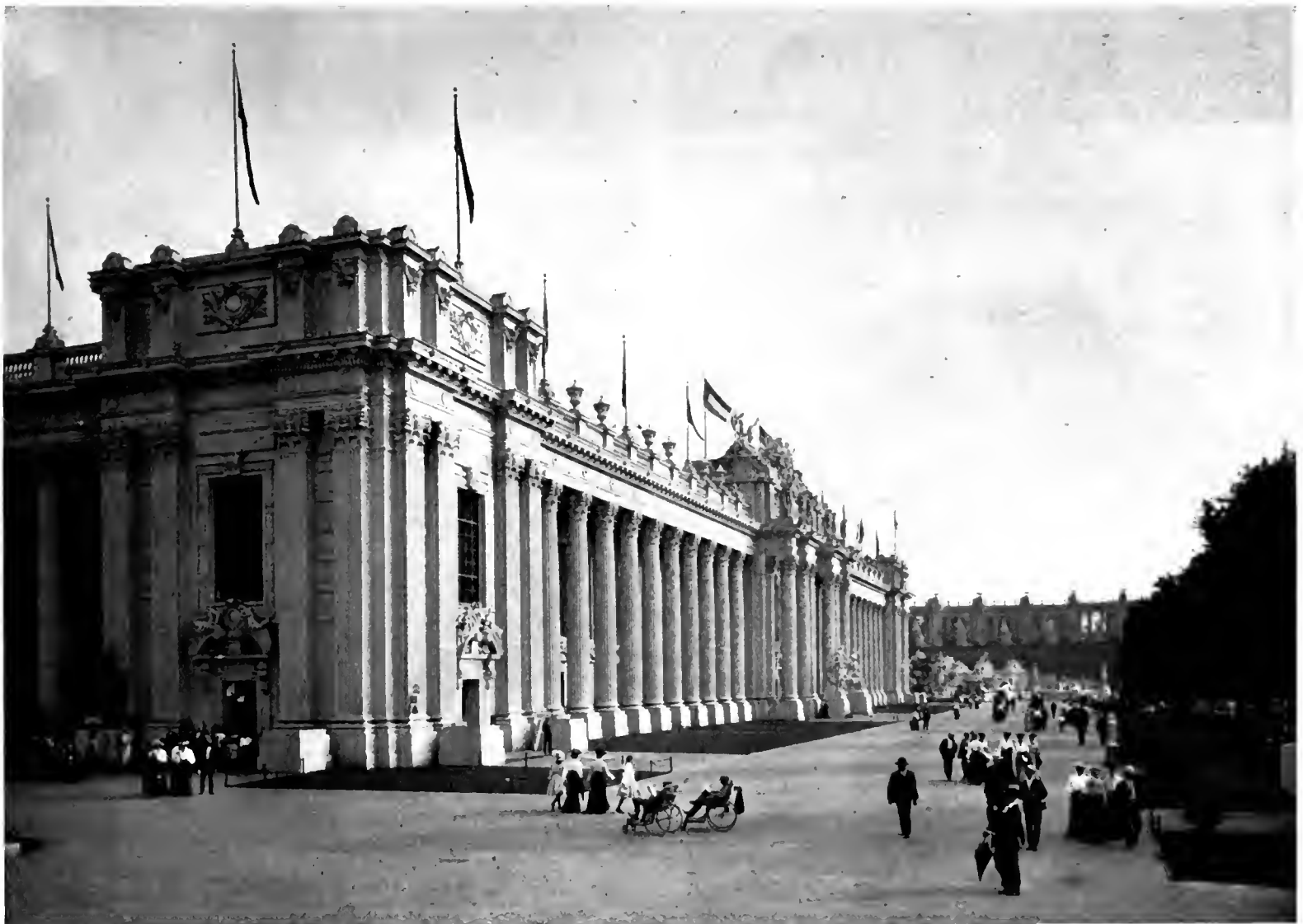
XIV. EDUCATION AND SOCIAL ECONOMY BUILDING, LOOKING SOUTH FROM JOLIET BRIDGE.
