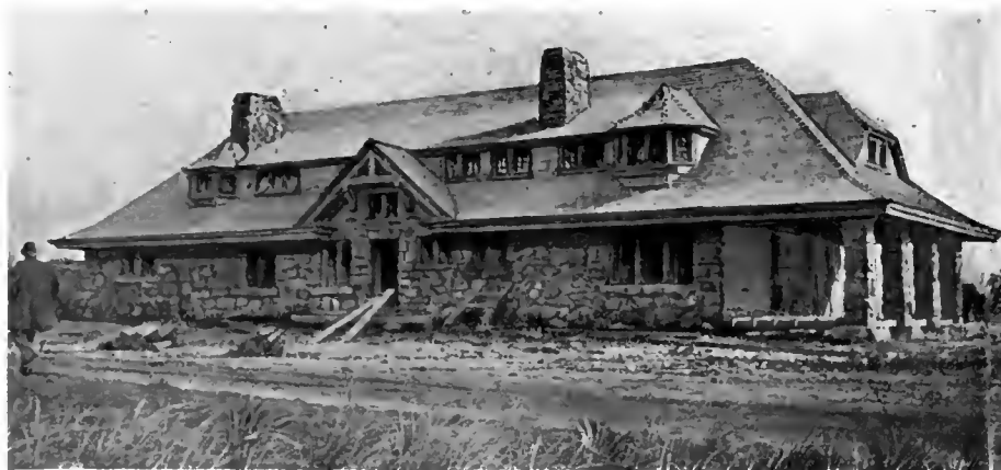
A BUNGALOW BEFORE COMPLETION.
