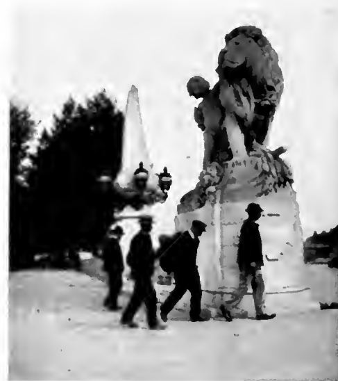
FIG. 13. APPROACH TO THE ALEXANDER BRIDGE.
