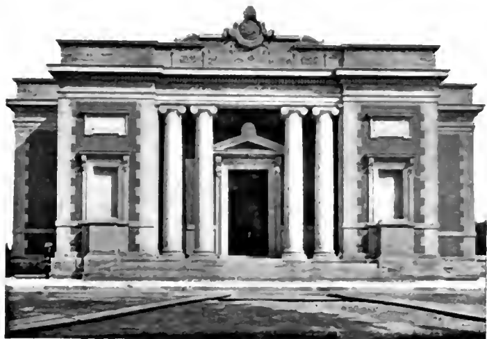
PUBLIC LIBRARY, MILTON, MASS. SHEPLEY, RUTAN & COOLIDGE, ARCHITECTS.
