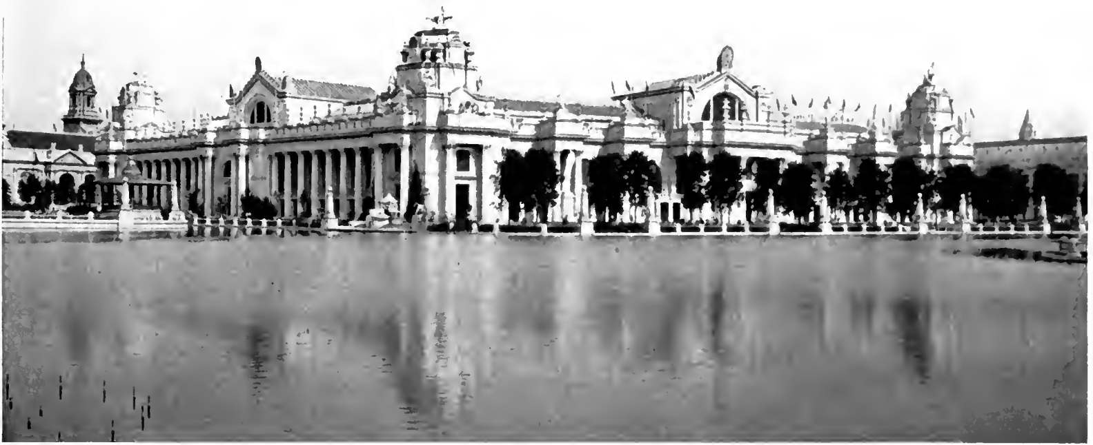
XVII. ELECTRICITY BUILDING FROM THE SOUTHEAST.
