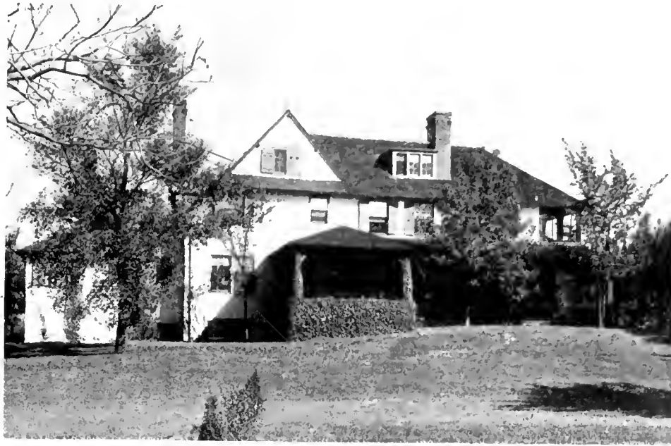
THE WEST SIDE OF THE HOUSE.
