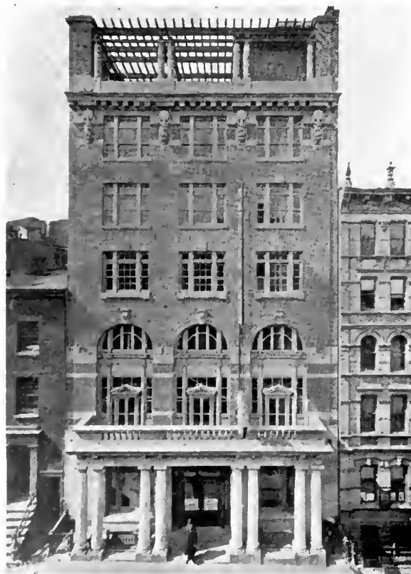
CLINTON HALL, NEW YORK CITY. HOWELLS & STOKES, ARCHITECTS.
