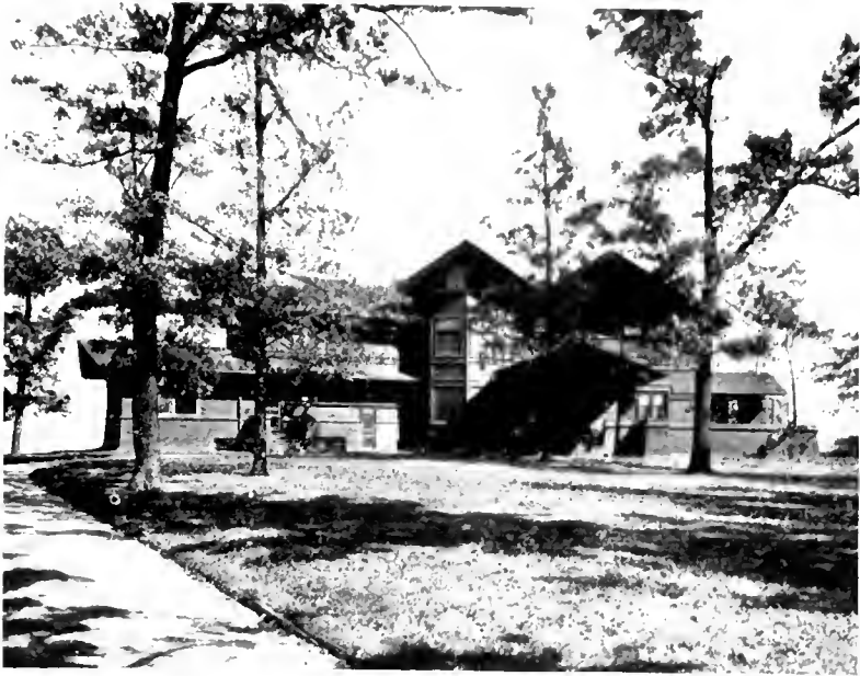
THE WEST SIDE
