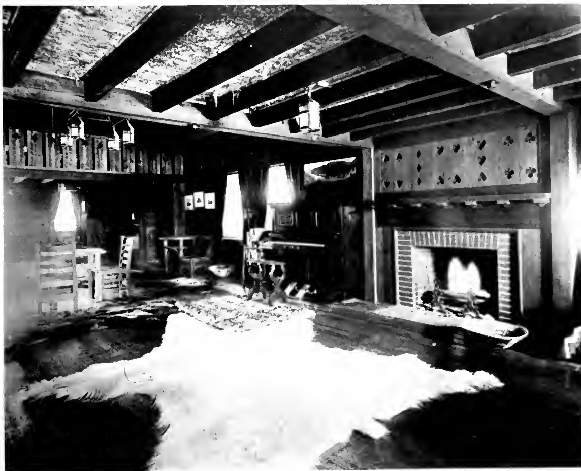
THE ATTIC ROOM
