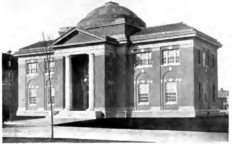
THE COLLIS P. HUNTINGTON MEMORIAL LIBRARY, HAMPTON, VA. DAVIS & BROOKS, ARCHITECTS.
