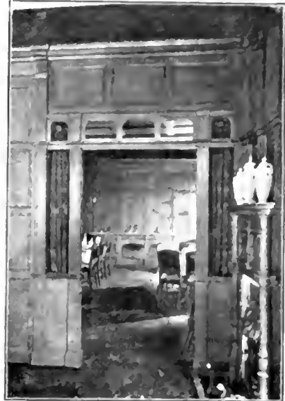
ROYAL EXCHANGE CLUB, LEEDS. BUTLER WILSON & OGLESBY, ARCHITECTS.
