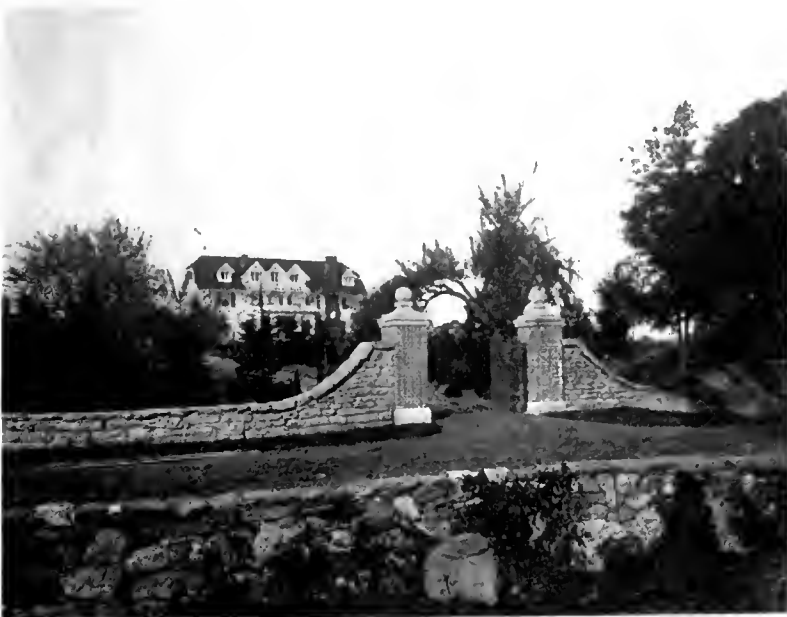
THE ENTRANCE GATES
