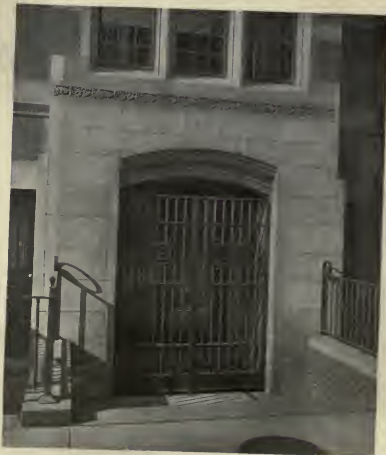
DETAIL OF ENTRANCE GATES.
