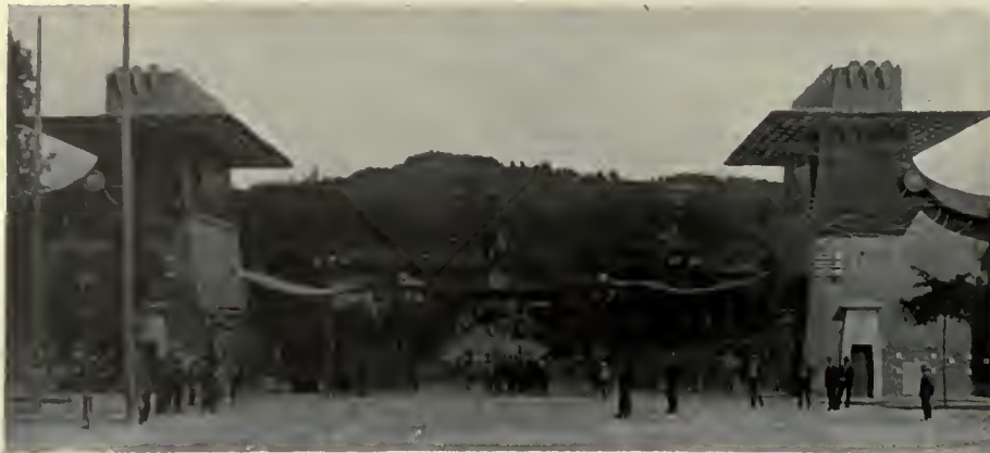
Turin Exposition, 1902. Main Entrance. Raim. d'Aronco, Architect.
