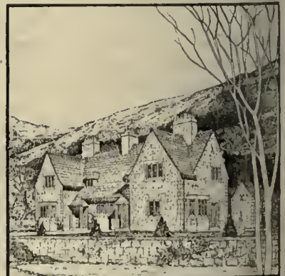
Double Cottage, Elan Valley. Buckland and Haywood-Farmer, Architects.
