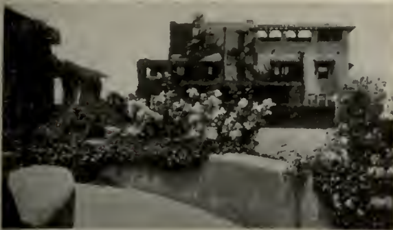
House at "Bayberry Point," Islip, L. I. Grosvenor Atterbury, Architect.
