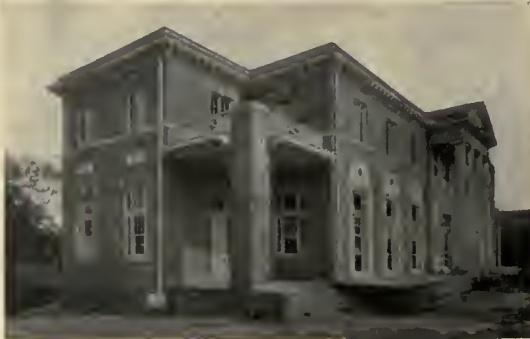
Dining-Hall and Dormitory, Auburn, Ala. Warren & Welton, Architects. (From "The American Architect.")
