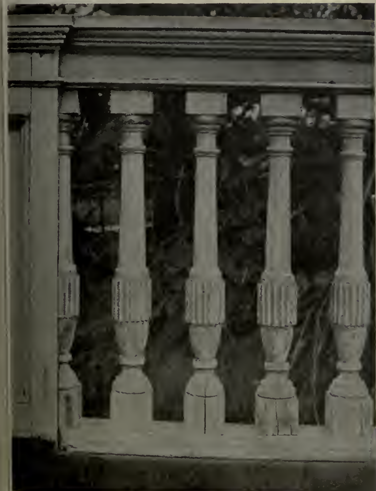
Detail, Porch, Roof Balustrade.
