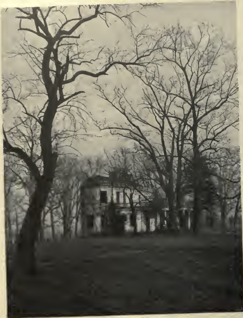
General View from the West.
