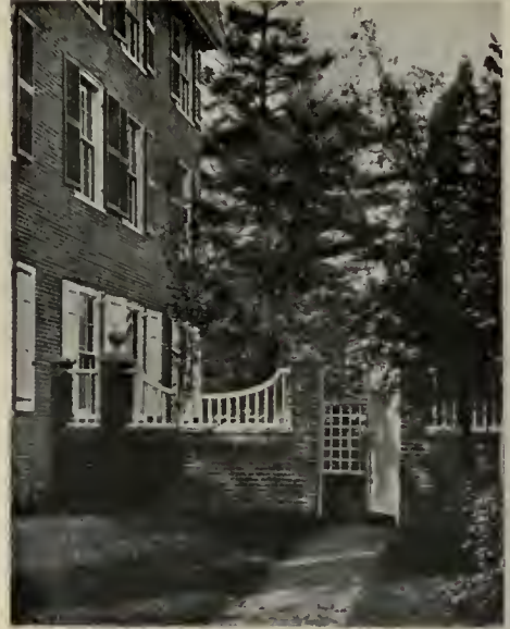
Garden Gateway, Dedham, Mass. Frank Chouveau Brown, Architect.
