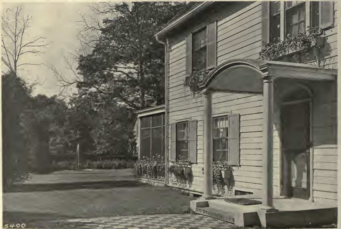
DETAIL OF PORCH.
