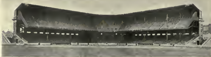
"Inside View," Pavilion for Am. League Baseball Club, Philadelphia, Pa. William Steele & Sons Co., Architects and Builders.
