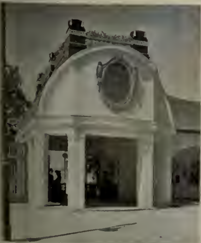
First Exposition Hall, Munich. Wilhelm Bertsch, Architect.
