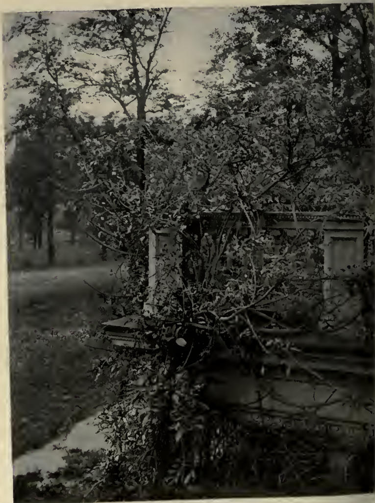
Corner of Porch Entablature and Balustrade.
