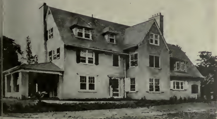
Residence at Germantown, Pa. Thomas, Churchman & Molitor, Architects.
