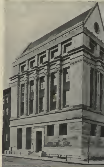
School of Applied Design for Women New York City. Pell & Corbett, Architects.
