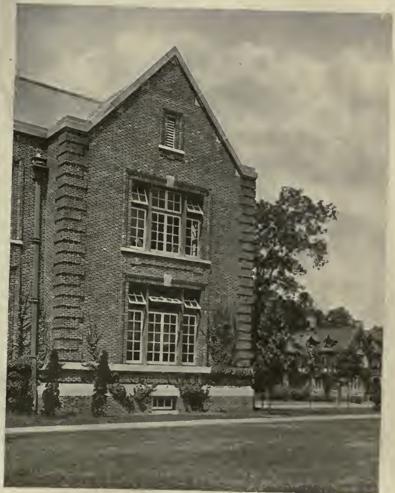
Detail of End Gable.
