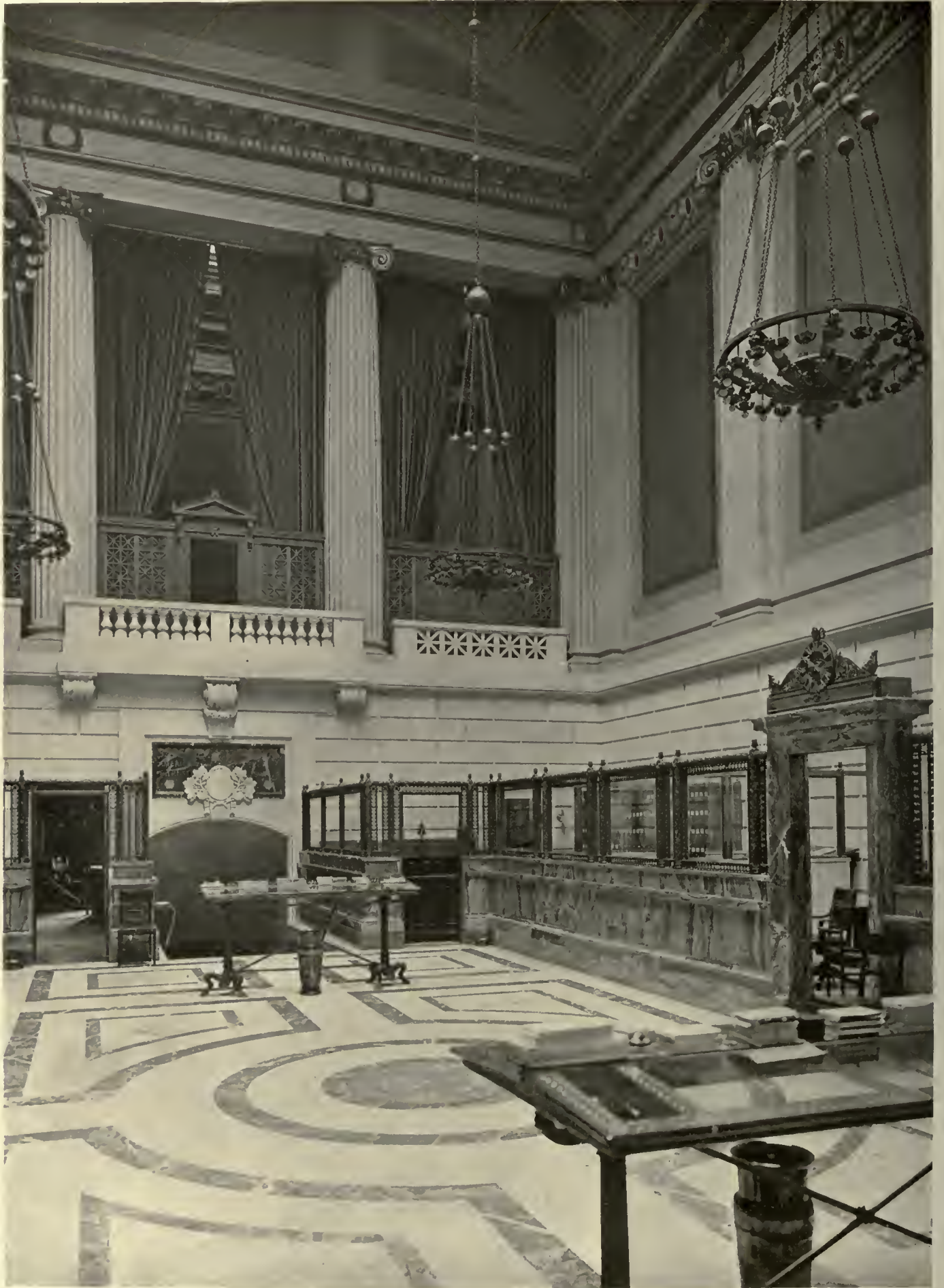
INTERIOR, LOOKING TOWARD ENTRANCE OF SAFE DEPOSIT VAULTS, AMERICAN SECURITY AND TRUST COMPANY, WASHINGTON, D. C.
