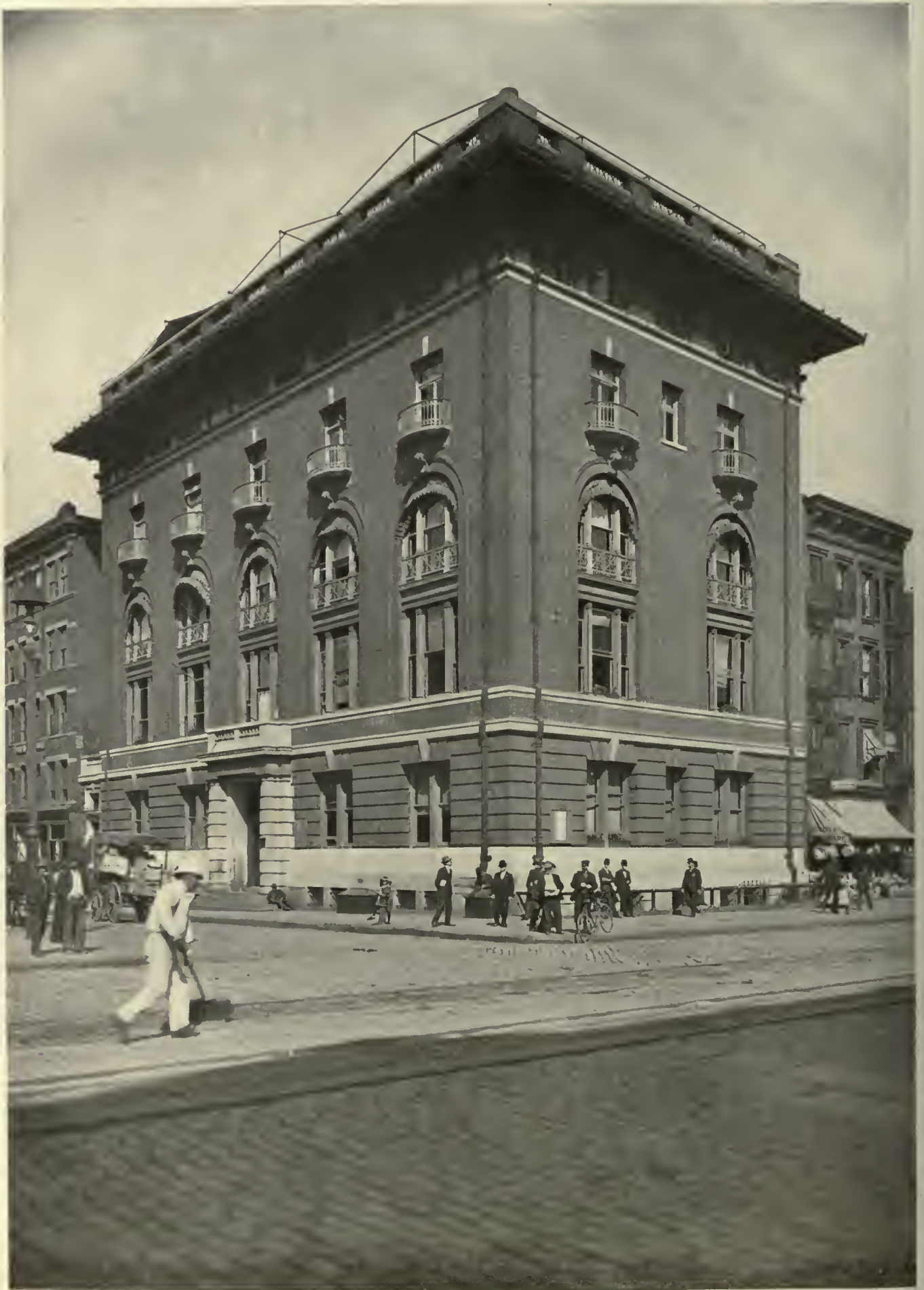
SETTLEMENT HOUSE, TENTH AVE. AND FIFTIETH ST., NEW YORK CITY.
