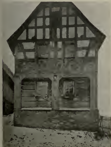
Fig. 25. Farmhouse in Block Framing, Liebschütz, 18th Century.
