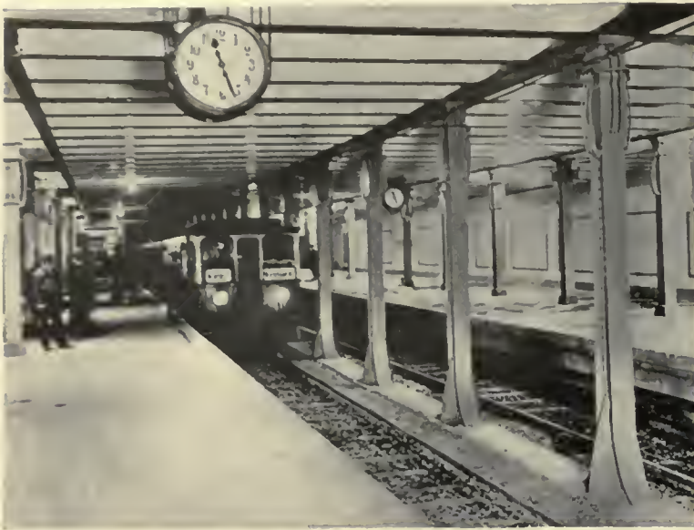
Typical Station Treatment of Supports.
