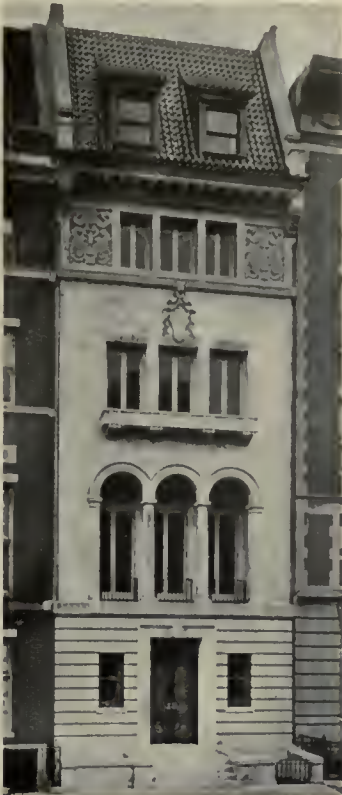
Residence, C. S. Guggenheim, N. Y. Harry Allen Jacobs, Architect. (From "Architecture.")
