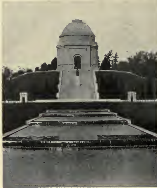
The McKinley National Memorial, Canton, Ohio. H. Van Buren Magonigle, Architect. (From "The New York Architect.")
