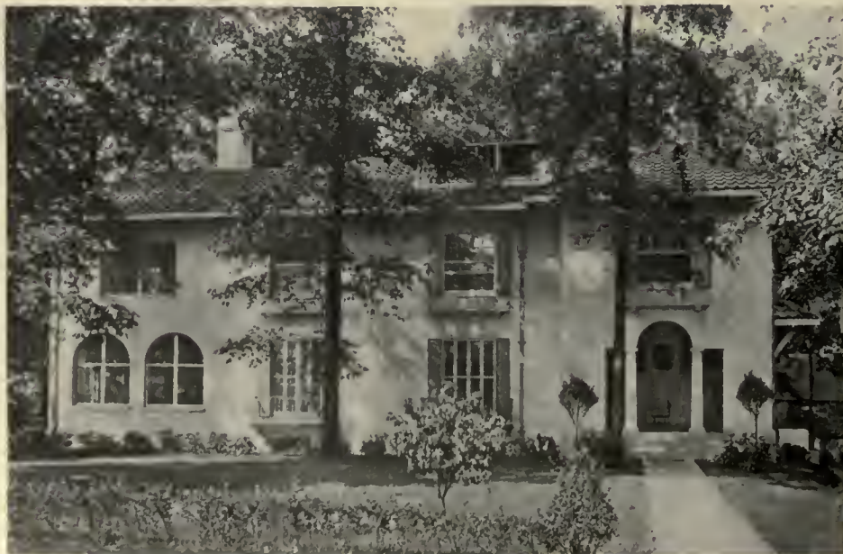
House of W. H. Crowell, Esq., Glenridge, N. J. Davis, McGrath & Kiessling, Architects.
