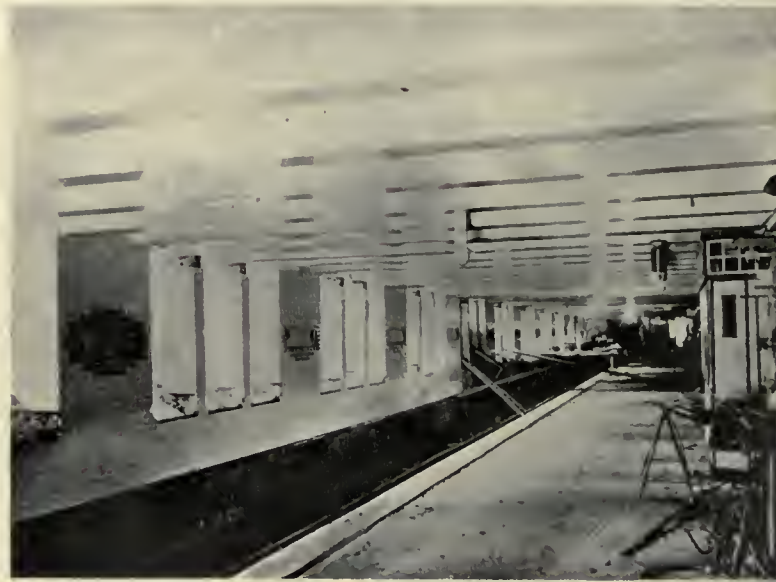
Station Underneath Spree Embankment.
