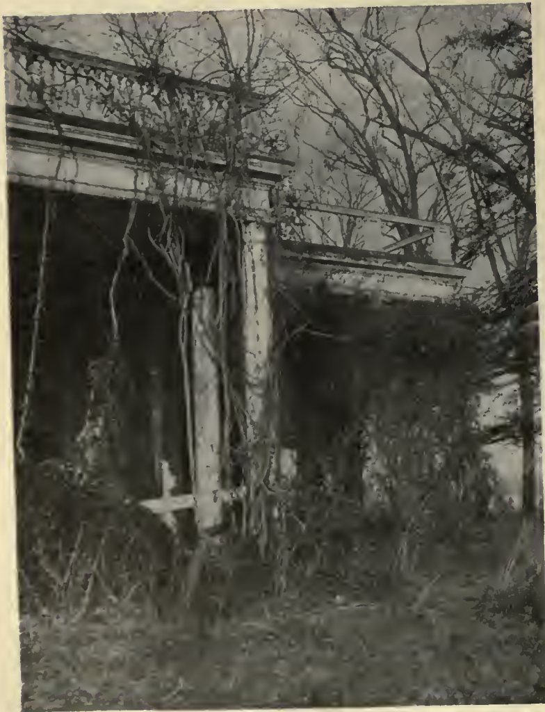
A Detail of the Porch.
