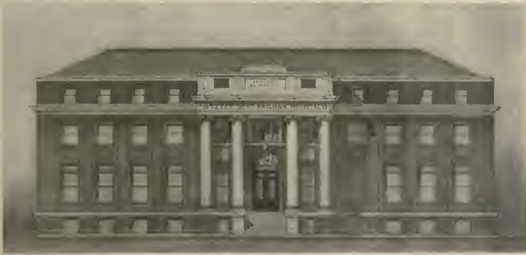
ADMINISTRATION BUILDING, PARKER, THOMAS & RICE, ARCHITECTS.
