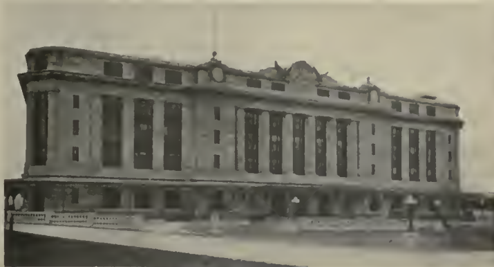
D., L. & W. R.R. Station, Scranton, Pa. Kenneth Murchison, Architect. (From "The Brickbuilder.")
