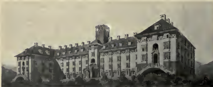
Government Offices, Simla. James Ransome, Architect.
