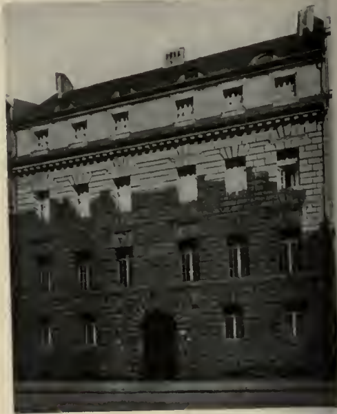
School Administration Building, Berlin. Ludwig Hoffmann, Architect.
