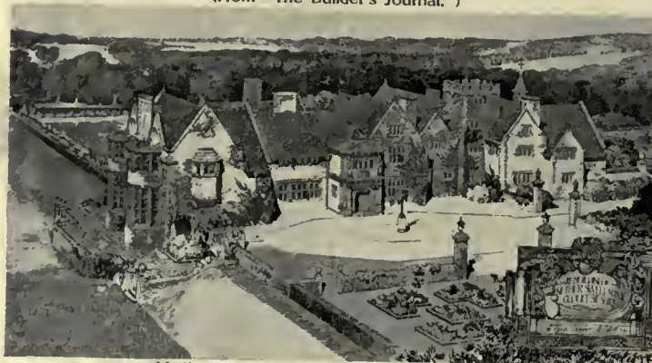
Nether Swell Manor, Gloucestershire. E. Guy Dawber, Architect. (From "The Builder's Journal.")
