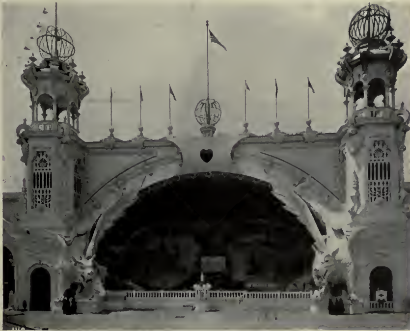
Entrance to the "Dragon's Gorge," Luna Park. One of the best "fronts" on the island, and showing the scale of the architecture.
