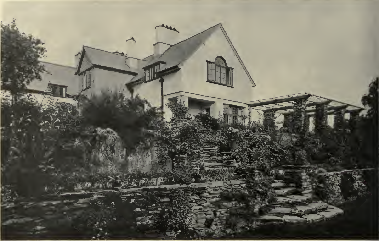
Rustic Steps, Terrace, and Pergola.
