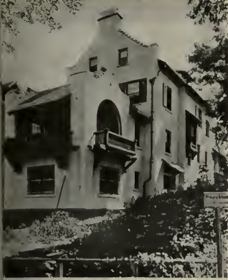
House for A. L. Schaeffer, University Hts., N.Y. Squires & Wynkoop, Architects.
