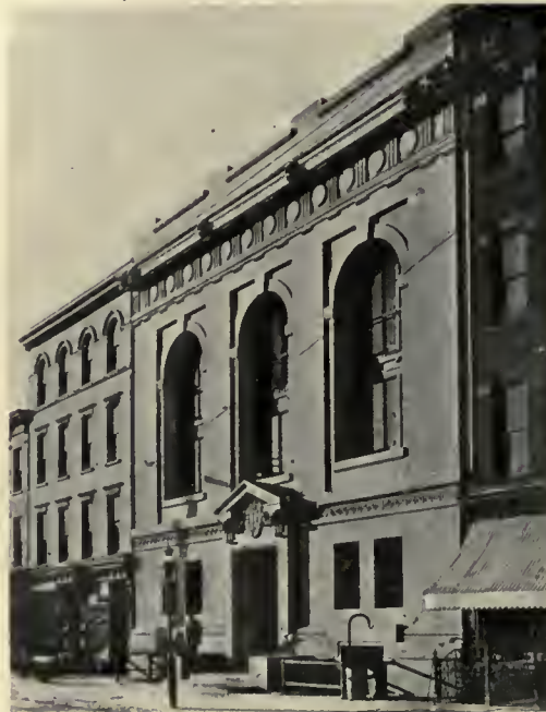
Gates Avenue Court-house, Brooklyn, N. Y. H. Van Buren Magonigle, Wilkinson & Magonigle, Architects. (From "The New York Architect.")
