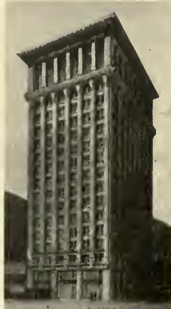
Milbank Bldg., New York City. Geo. B. Post & Sons, Architects.
