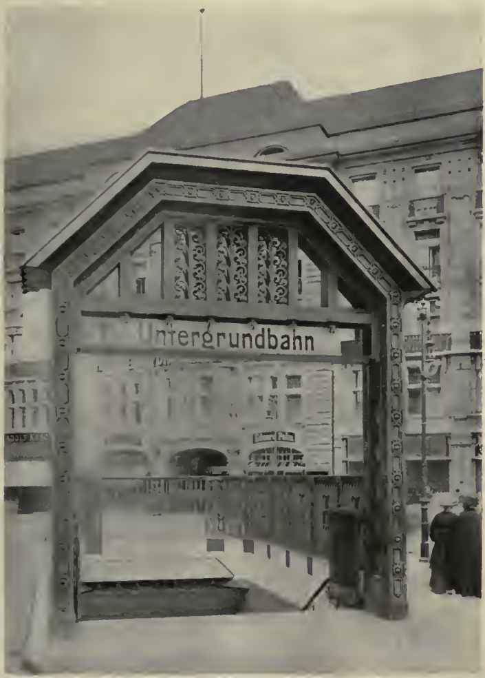
Ironwork of Typical Station Entrance.
