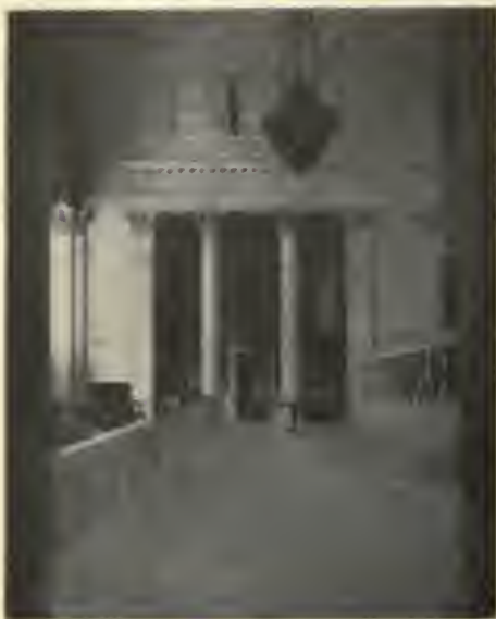
View of Southeast Alcove, National City Bank of New York. McKim, Mead & White, Architects.
