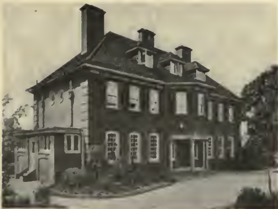
House at Kingston Hill. A. Jessop Hardwick, F. R. I. B. A., Architect.
