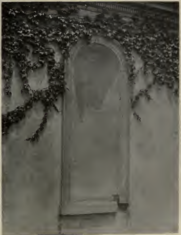
Detail of Niche and Cornice.
