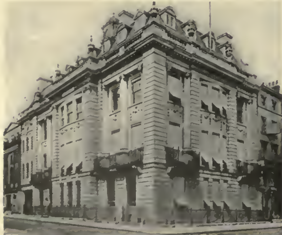
United University Club, Pall Mall East. Reginald Blomfield, A.R.A., Architect.
