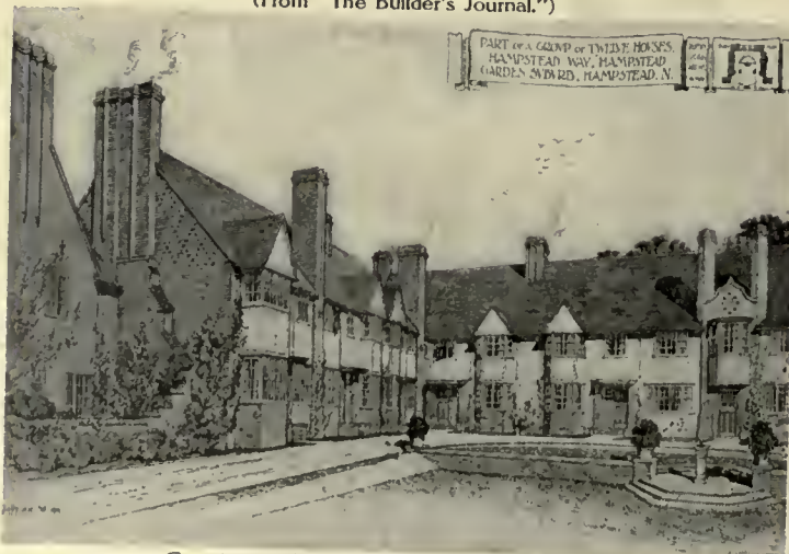
Courtyard, House Group, Hampstead, N. Geoffry Lucas, Architect.
