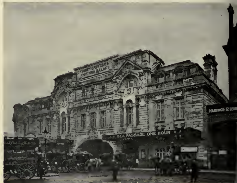
The Victoria Station, S. E. & C. Railway. Principal Frontage, Facing Forecourt.
