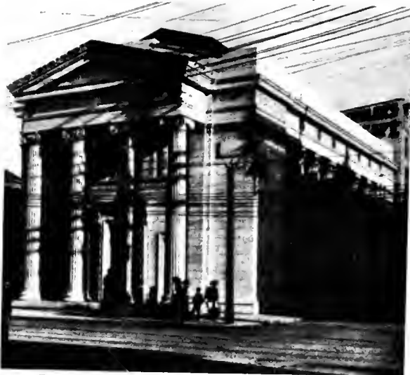
Connecticut Savings Bank, New Haven, Conn. Gordon, Tracy & Swartwout, Architects. (From "The Architectural Review," London.)
