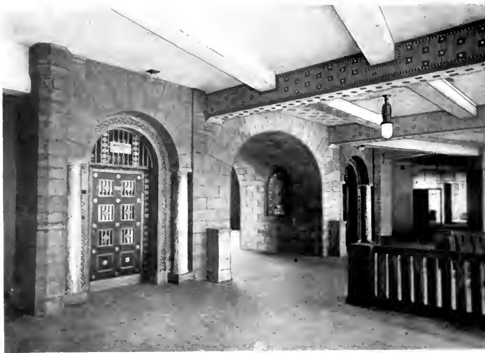
View within the Outside Corridors, Showing Stairways and Elevator Enclosures.
