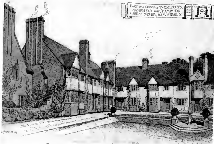
Courtyard, House Group, Hampstead, N. Geoffry Lucas, Architect.
