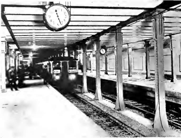
Typical Station Treatment of Supports.
