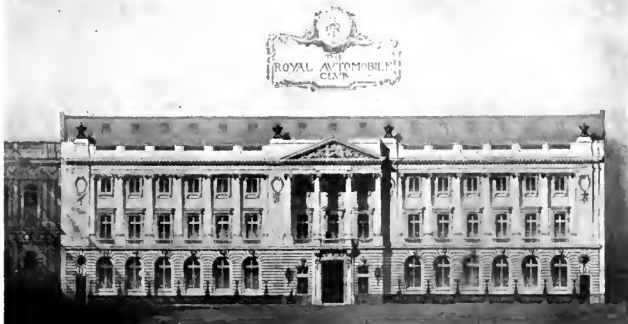
The Façade at Pall Mall. Mewès & Davis and E. Keynes Purchase, Associate Architects.
