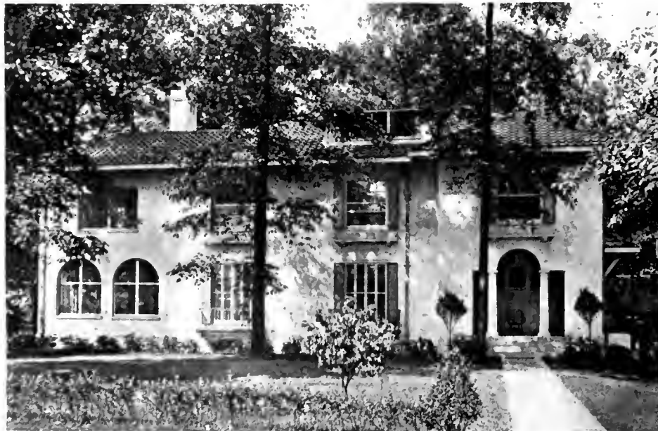
House of W. H. Crowell, Esq., Glenridge, N. J. Davis, McGrath & Kiessling, Architects.
