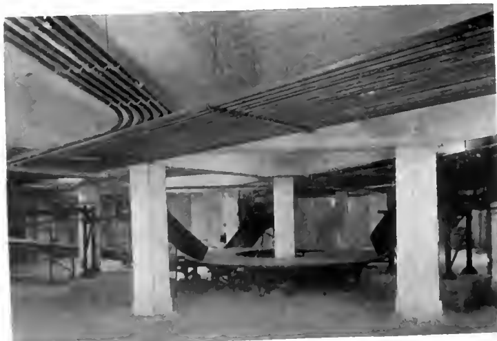
Parcel Conveyers and Rotating Table in Basement. Cash-system tubes are to be seen hung from the ceiling above.
