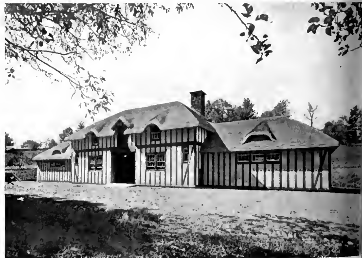
Stable for Charles S. Brown, Esq., Mt. Kisco, N. Y. Albro & Lindeberg, Architects.
