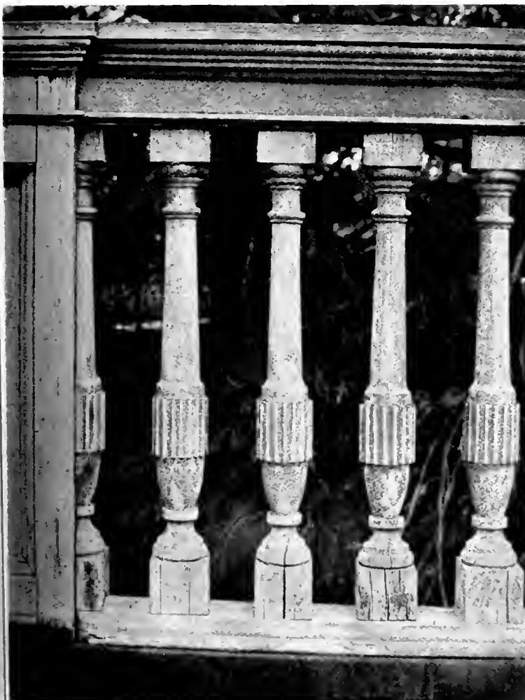
Detail, Porch, Roof Balustrade.
