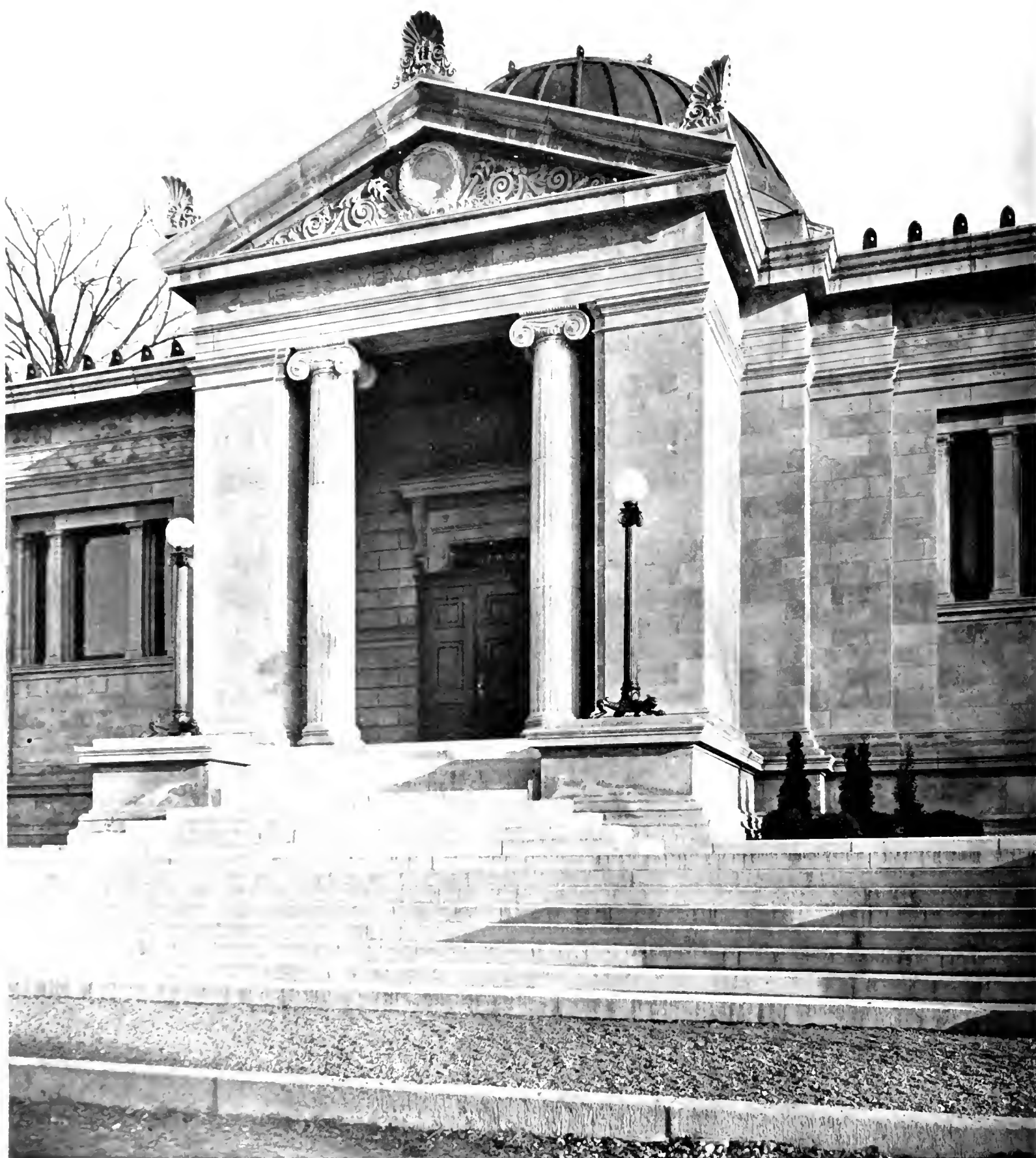
DETAIL OF ENTRANCE, FIELD MEMORIAL LIBRARY, CONWAY, MASS.
