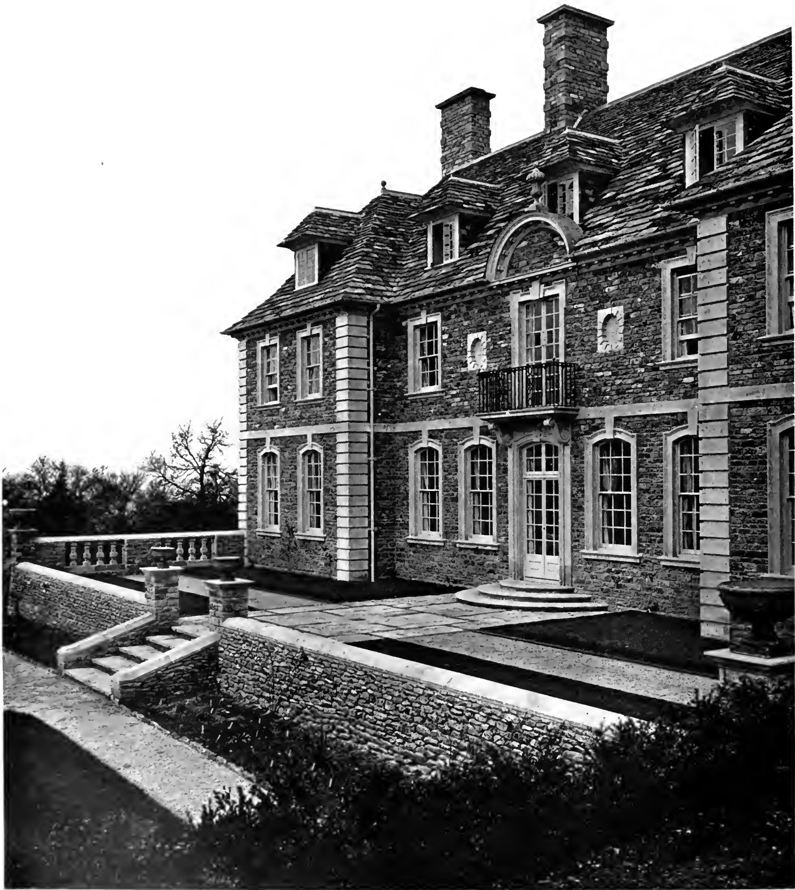
DETAIL, GARDEN TERRACE AND ENTRANCE, CONKWEIL GRANGE, WILTSHIRE, ENGLAND.
