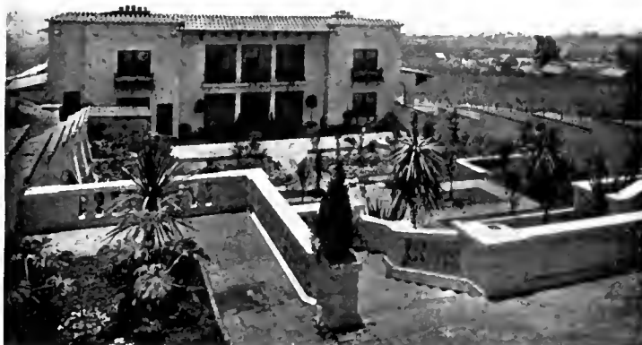
Garden from Terrace, House at Hollywood, Cal. Myron Hunt & Elmer Grey, Architects.
