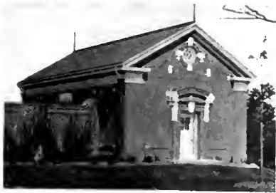
Squash Court, North Easton, Mass. Coolidge & Carlson, Architects.
