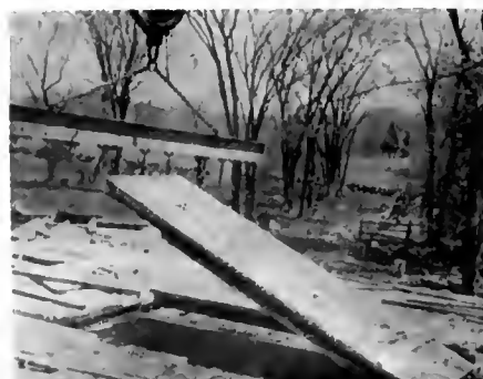
Raising Section of Wall with Special Derrick.
