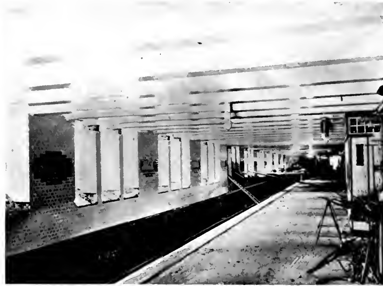
Station Underneath Spree Embankment.
