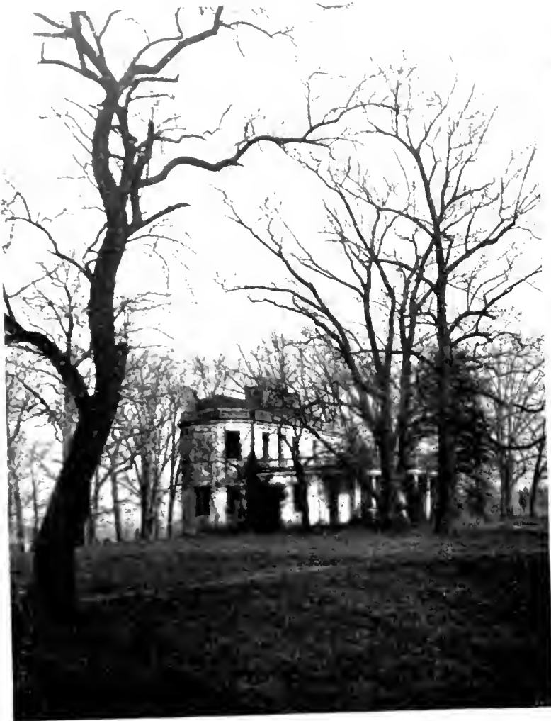
General View from the West.
