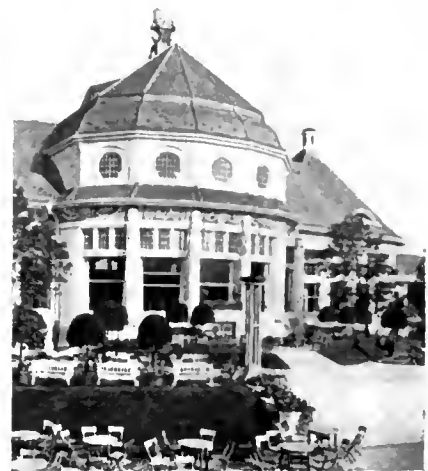
Restaurant in Munich Exposition Park. Imanuel Von Seidl, Architect.
