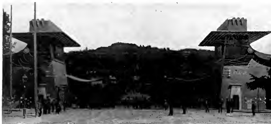
Turin Exposition, 1902. Main Entrance. Raim. d'Aronco, Architect.
