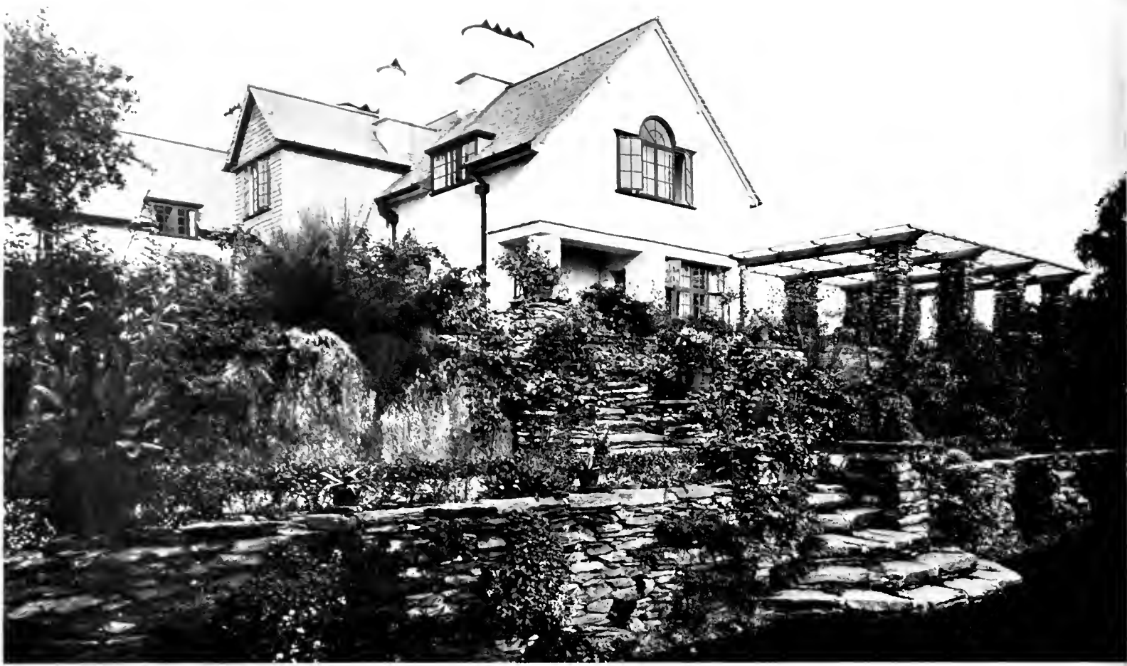
Rustic Steps, Terrace, and Pergola.
