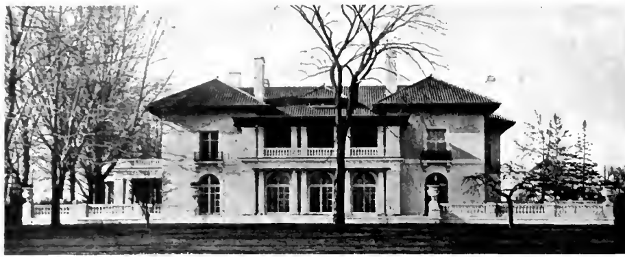
Residence of A. L. Stephens, Grosse Pointe, Mich. Albert Kahn, Architect.
