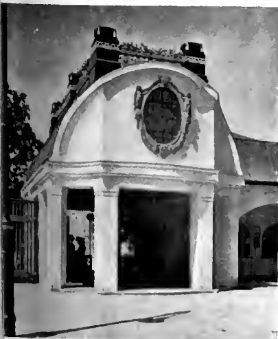
First Exposition Hall, Munich. Wilhelm Bertsch, Architect.
