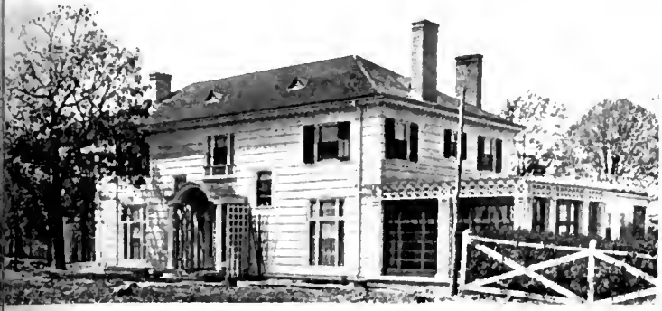
House at Birmingham, Ala. Warren & Welton, Architects.
