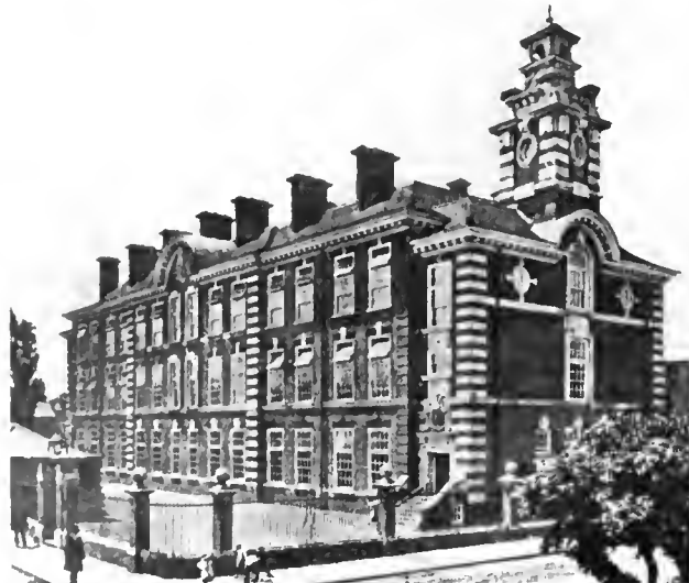
Pelham School, Wimbledon. H. P. Burke Downing, F. R. I. B. A., Architect.
