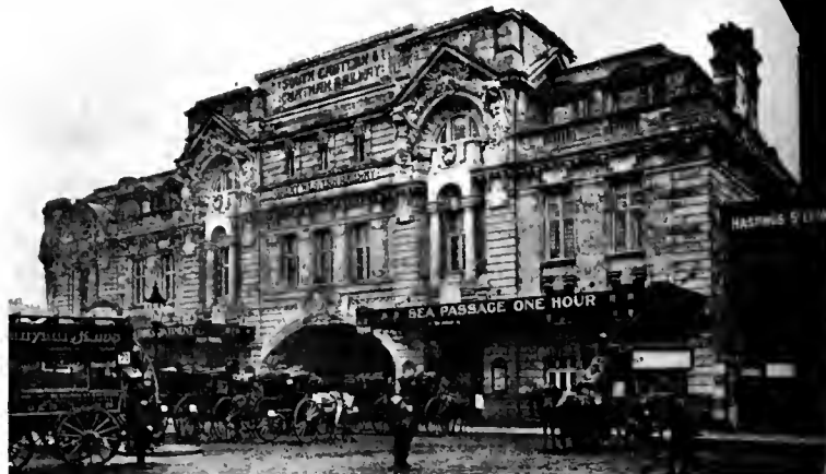
The Victoria Station, S. E. & C. Railway. Principal Frontage, Facing Forecourt.
