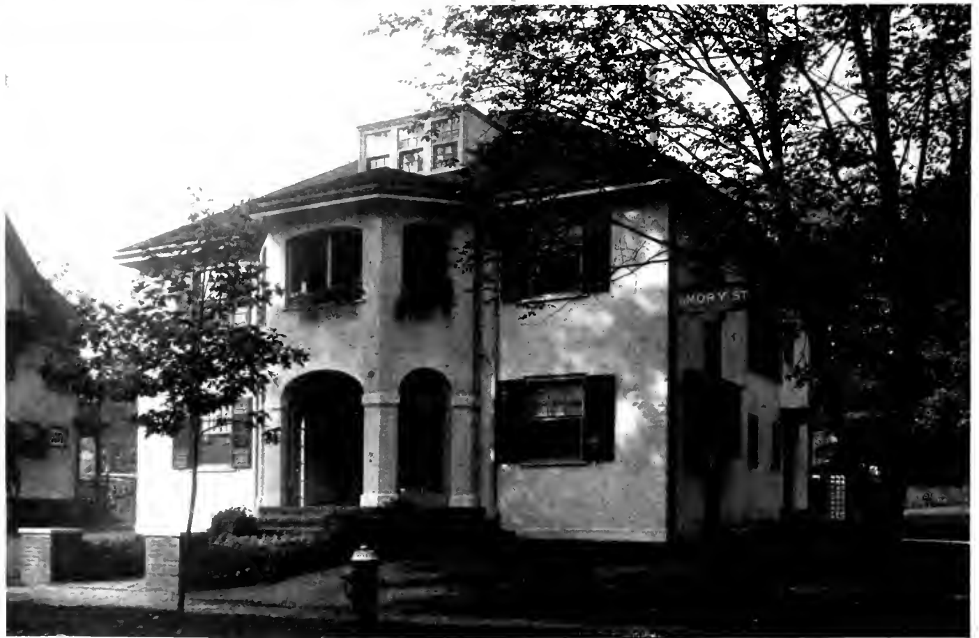
HOUSE CORNER AMORY AND FREEMAN STREETS, BROOKLINE, MASS. FRANK CHOUTEAU BROWN, ARCHITECT.
