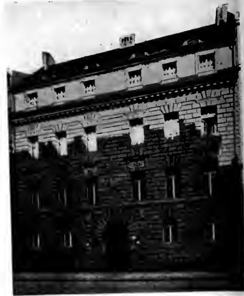
School Administration Building, Berlin. Ludwig Hoffmann, Architect.
