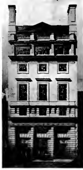
Façade in Kingsway, London. Edwin L. Lutyens, Architect.
