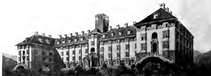
Government Offices, Simla. James Ransome, Architect.
