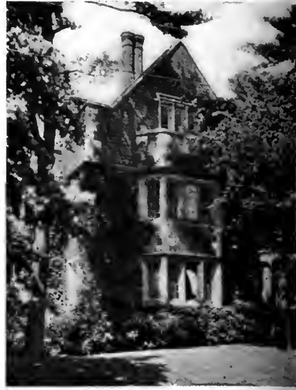
Seventy-Nine Dormitory, Princeton Univ. Cram, Goodhue & Ferguson, Architects.
