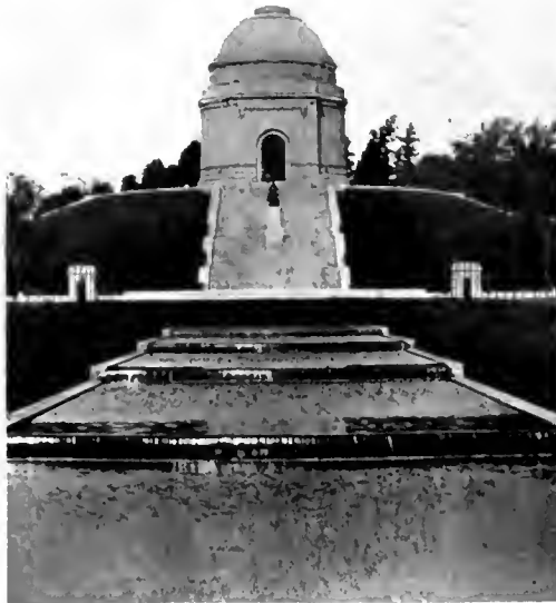
The McKinley National Memorial, Canton, Ohio. H. Van Buren Magonigle, Architect. (From "The New York Architect.")
