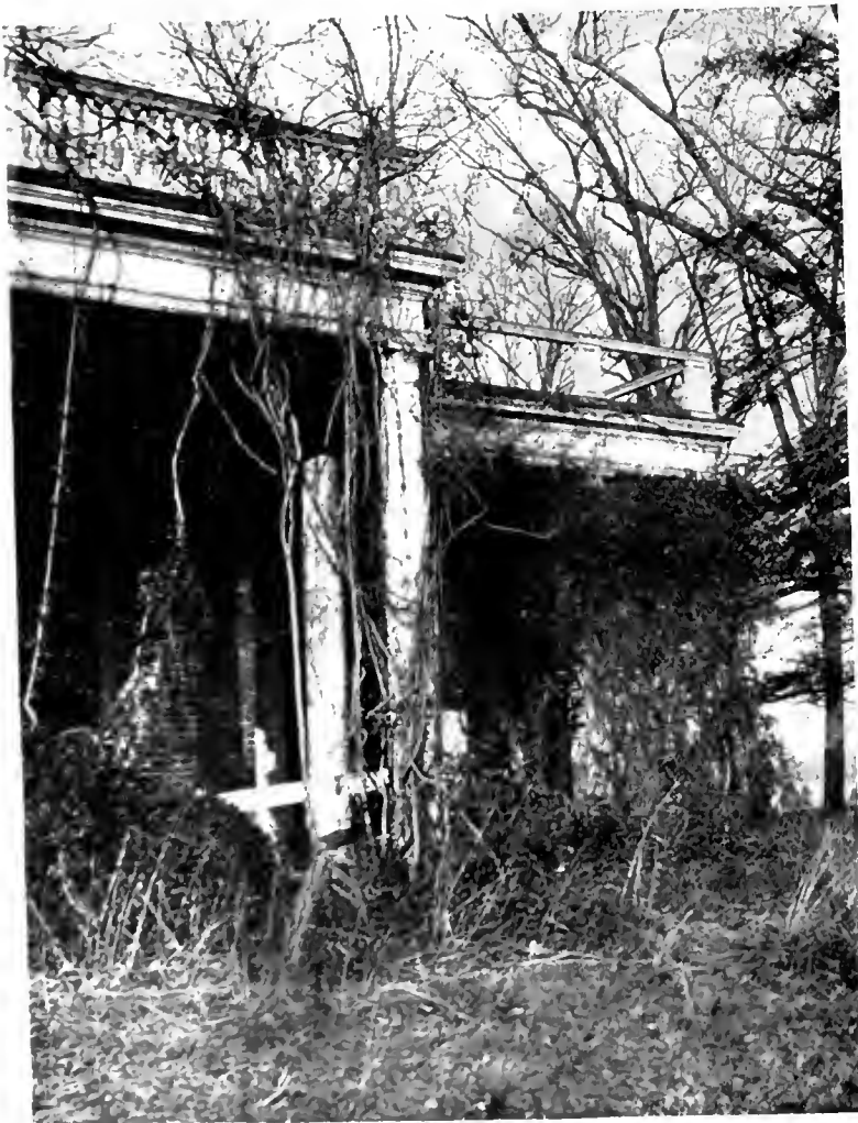
A Detail of the Porch.
