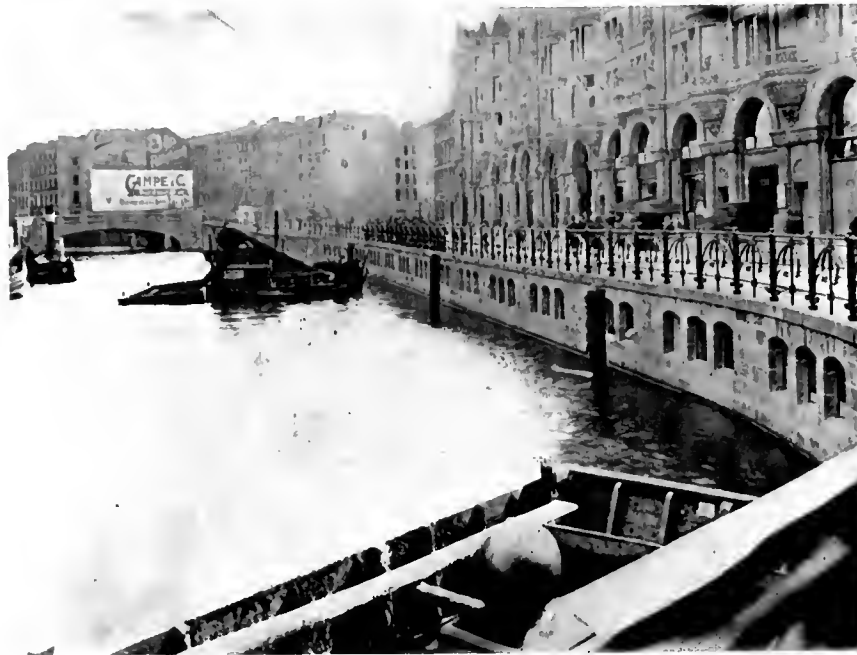
Windows Along the Spree Embankment, from Without.
