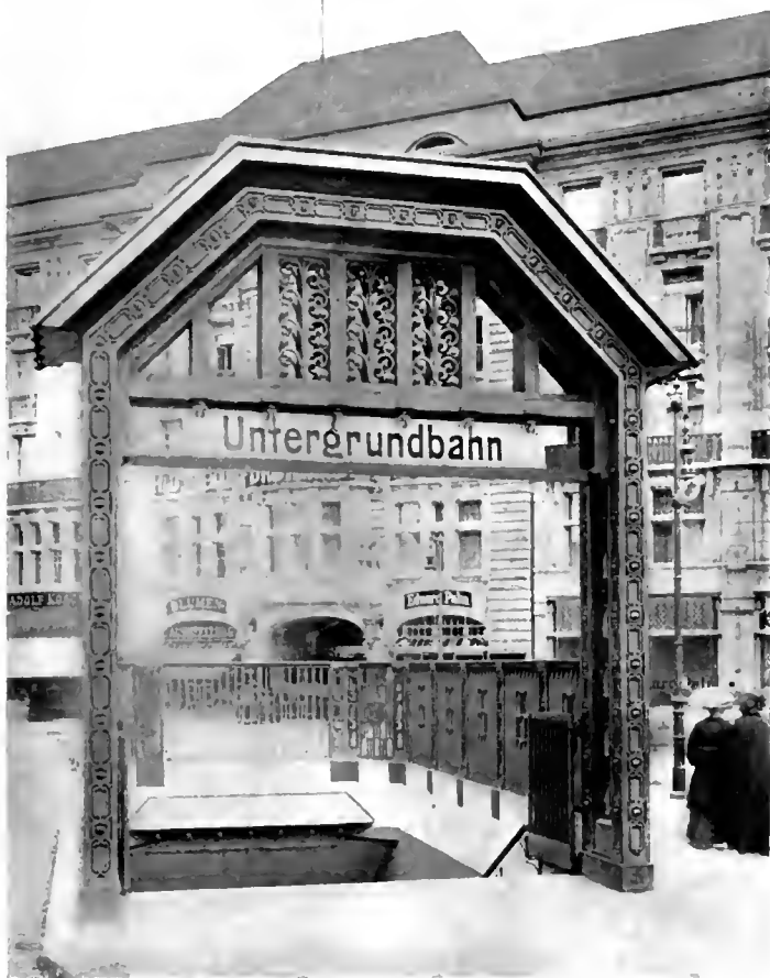
Ironwork of Typical Station Entrance.
