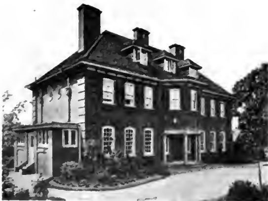
House at Kingston Hill. A. Jessop Hardwick, F.R.I.B.A., Architect.
