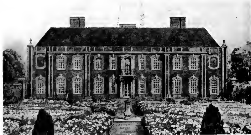
New West Wing, Temple Dinsley, Herts. Edwin L. Lutyens, F. R. I. B. A., Architect.
