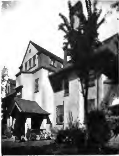
Residence, La Crosse, Wis. Handy & Cady, Architects.
