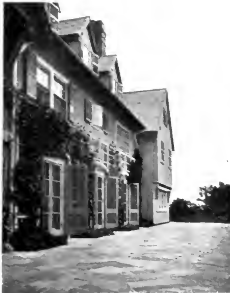
Terrace, House at Cohasset, Mass. Andrews, Jacques & Rantoul, Architects.
