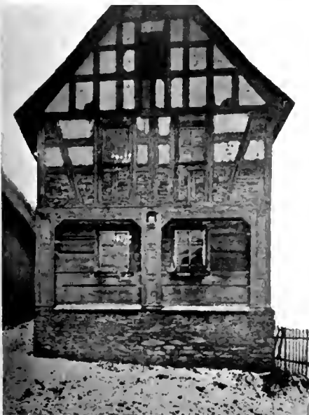
Fig. 25. Farmhouse in Block Framing, Liebschütz, 18th Century.
