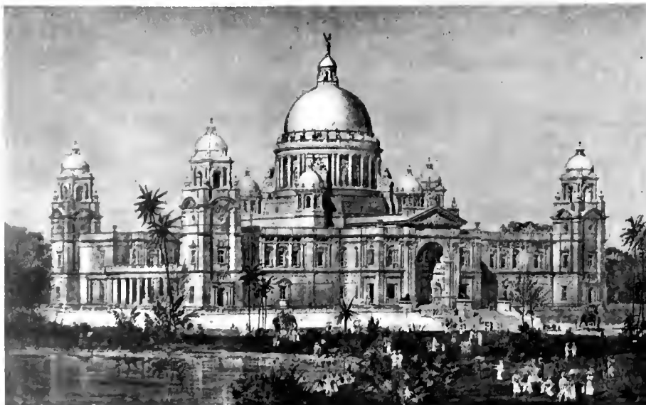
The Queen Victoria Memorial Hall, Calcutta. Sir William Emerson, F.R.I.B.A., Architect.
