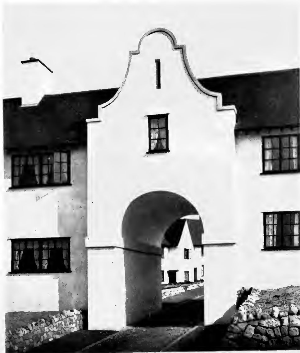
THE ENTRANCE ARCH.
