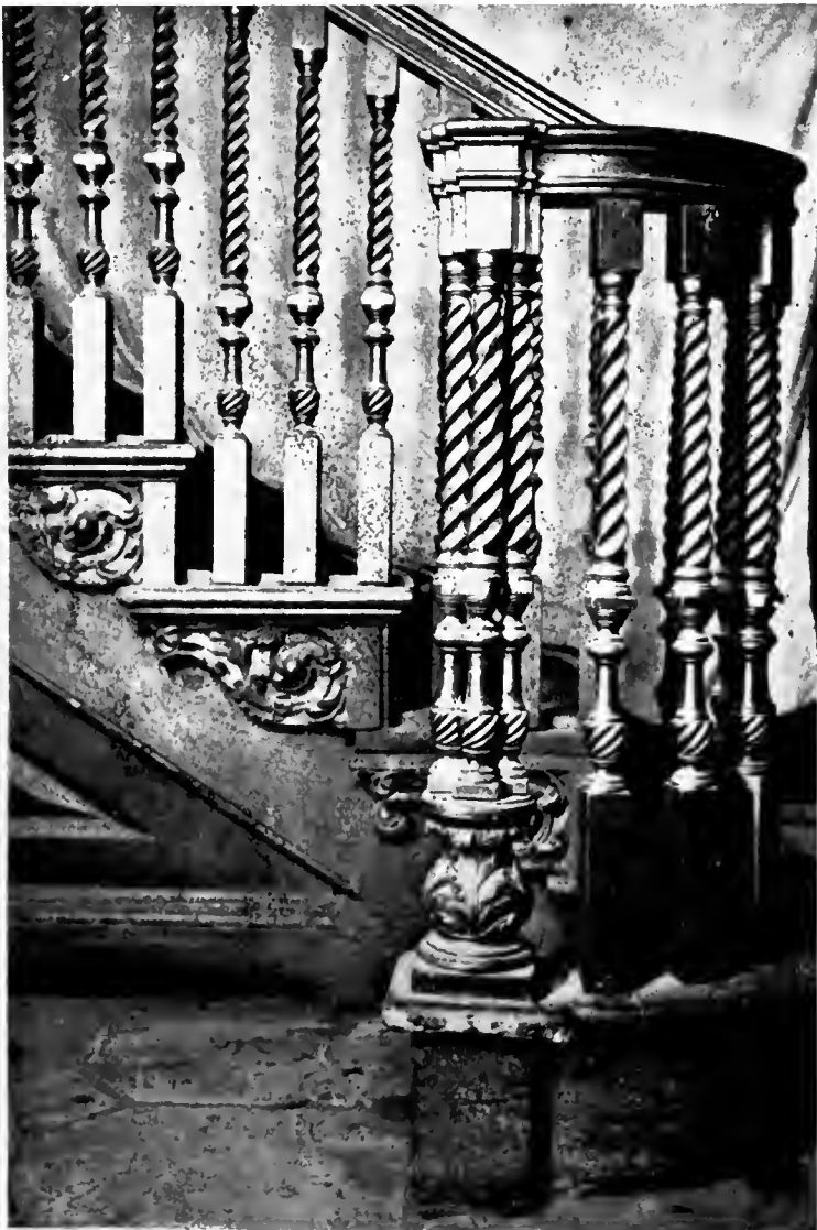
DETAIL OF STAIRCASE, No. 15 QUEEN SQUARE.
