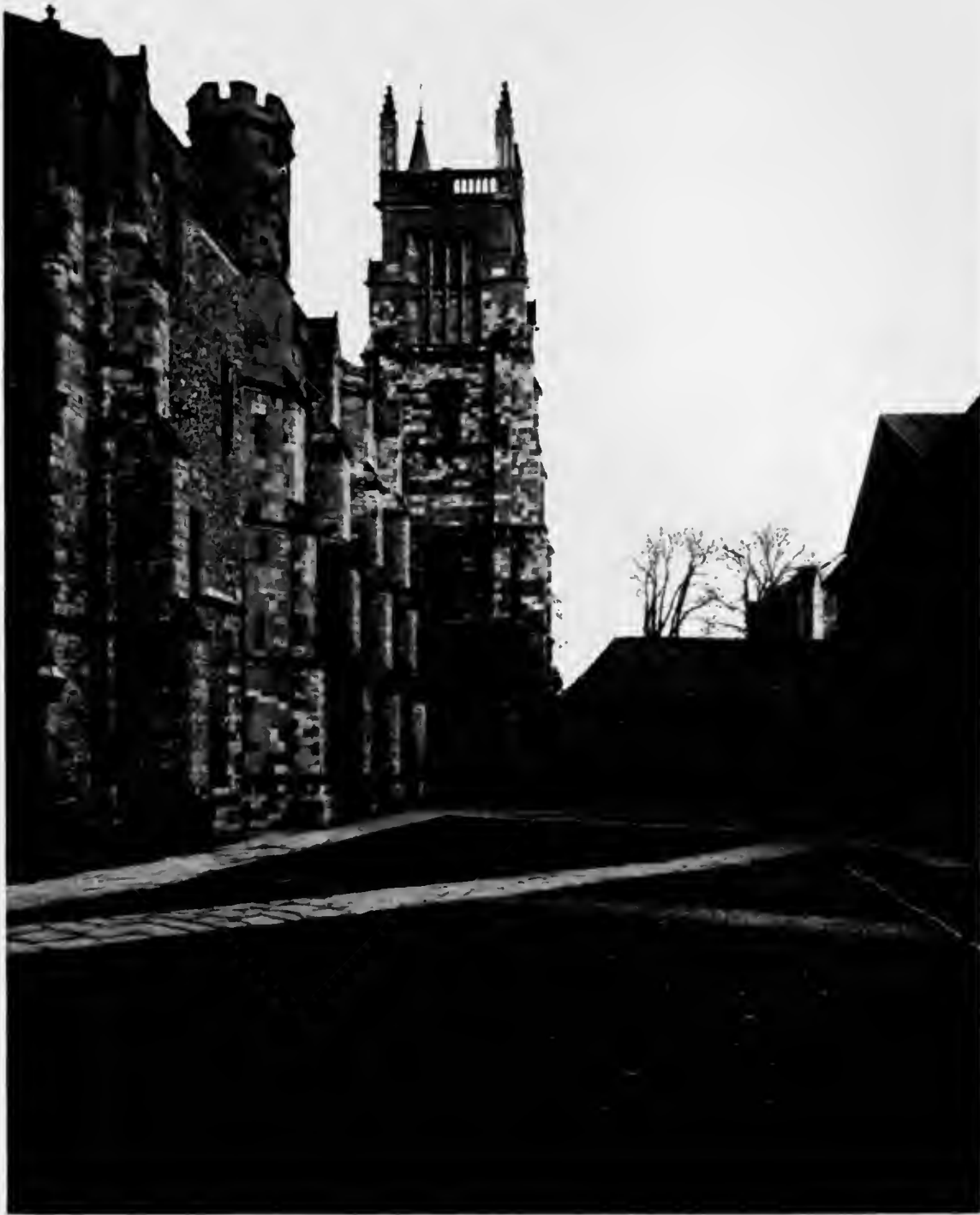
CHAPEL TOWER AND CORNER OF SCHOOL.
