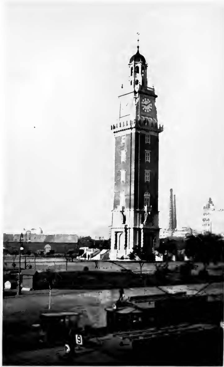
GENERAL VIEW OF TOWER.
