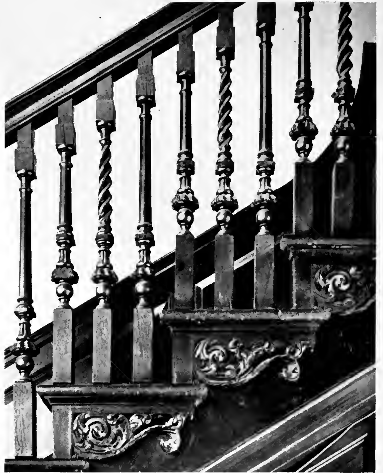
DETAIL OF STAIRCASE, No. 15 QUEEN SQUARE.
