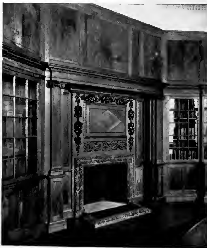
PANELLING ETC., TO BOARD ROOM—IN ENGLISH WALNUT. MESSRS. H. B. CRESWELL & W. A. FORSYTH, ARCHITECTS.
