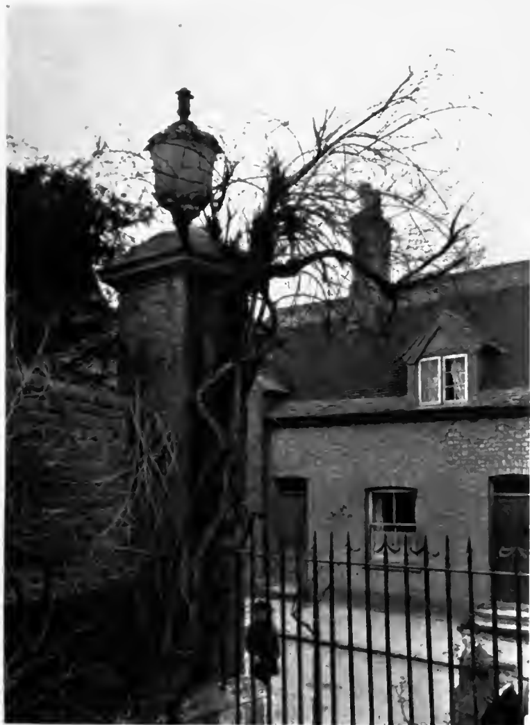
VASE ON POST FORMERLY AT HOUGHTON TOWERS.
