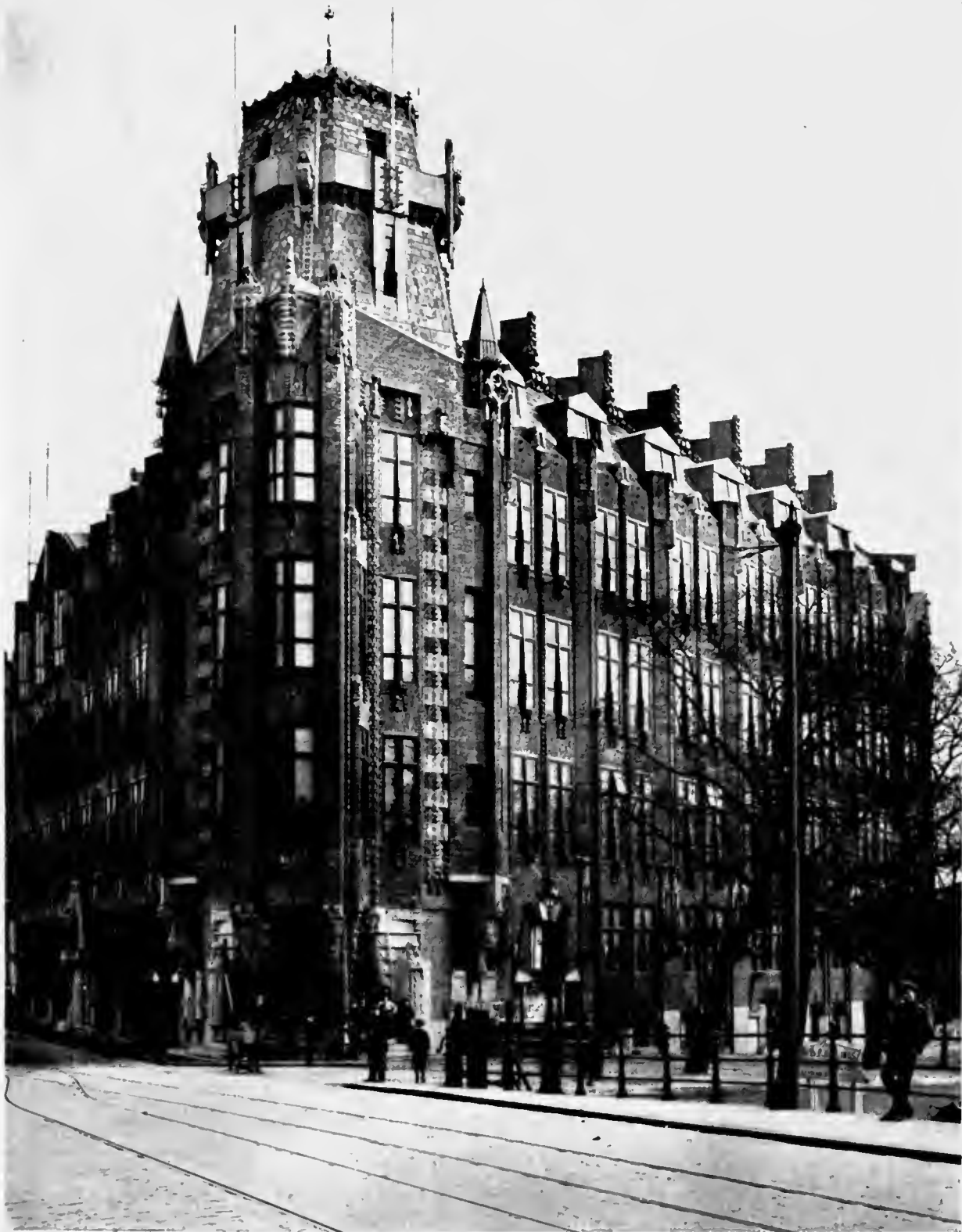
MARINE HOTEL, AMSTERDAM: GENERAL VIEW.
